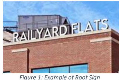
Figure 1: Example of Roof Sign Source: Pride Neon Sign Solutions
