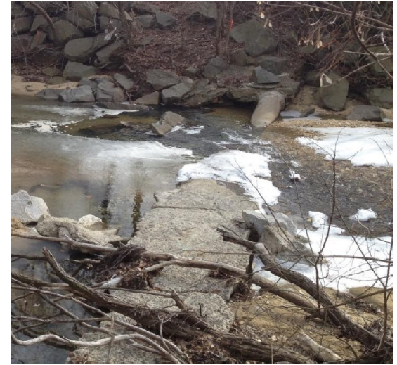
South Van Dorn Emergency Repair – 120 feet of 20 inch sewer line sagged due to stream erosion
