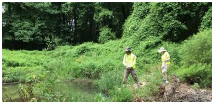
Figure 12: Staff inspecting and treating a storm water pond.
