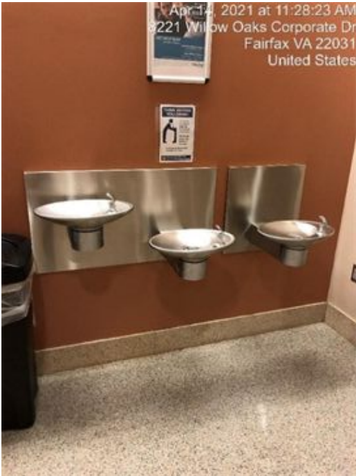
Figure 2-12. Standard Water Fountain.
