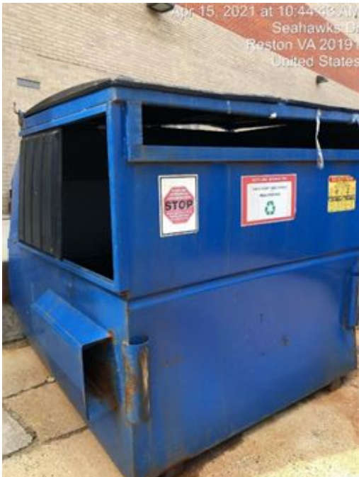
Figure 2-9. Cardboard slots on exterior dumpsters makes user believe only cardboard is accepted. Suggest replacing or enhancing existing exterior recycling dumpsters to not have or indicate cardboard slots.
