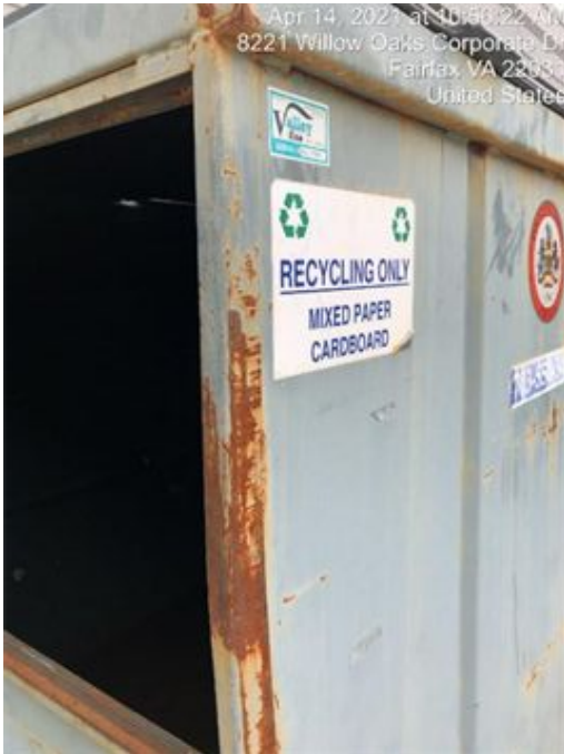
Figure 2-8. Incorrect labeling of exterior County dumpster; the County has single-stream recycling and also collects bottles/cans. The dumpster could also be painted blue to clearly indicate it is a recycling receptacle.
