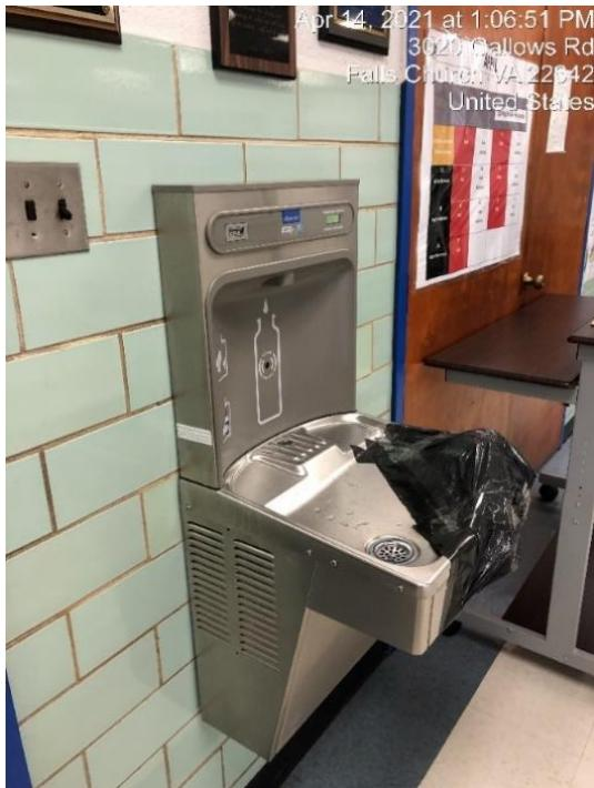
**Figure 2-11. Installed Bottle Filling Station at a Current FCPS Middle School (spout currently inoperable due to COVID-19 health and safety regulations).**
