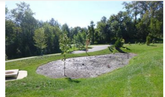
Bioretention Missing Mulch/Plants
