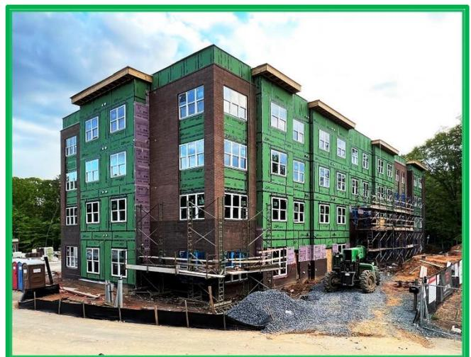
Installation of the brick façade on the building is underway. The developer has been applying insulation and has begun installing mechanical equipment on the rooftop. This work, along with additional mechanical-electric-plumbing work, will continue during May.
