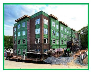
Installation of the brick façade on the building is underway. The developer has been applying insulation and has begun installing mechanical equipment on the rooftop. This work, along with additional mechanical-electric-plumbing work, will continue during May.
