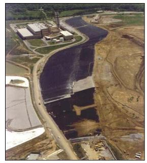
The ash landfill was designed in four phases and meets federal and state standards for the construction of new landfills, which requires a double liner with a leachate collection system for the prevention of groundwater degradation. Phases I and II have reached capacity and have been covered with an intermediate cover system. Phase III is currently being used for ash disposal and has at least five years of capacity remaining. Phase IV has not yet been constructed.
