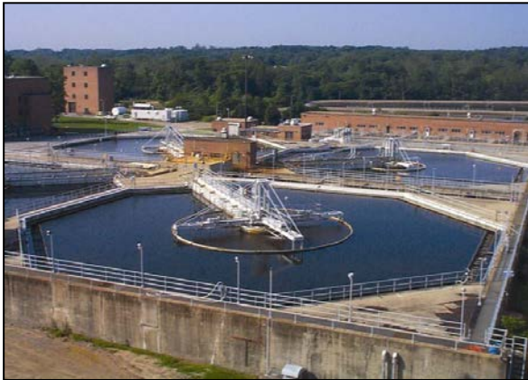
Photo of the Noman M. Cole Jr. Pollution Control Plant
