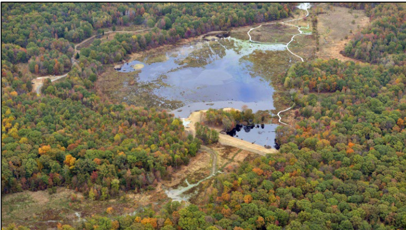
Photo of the Huntley Meadows wetland restoration project
