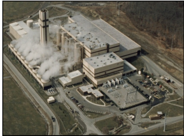
I-95 Energy/Resource Recovery Facility
