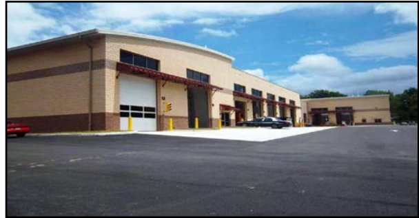
Newington DVS Facility
