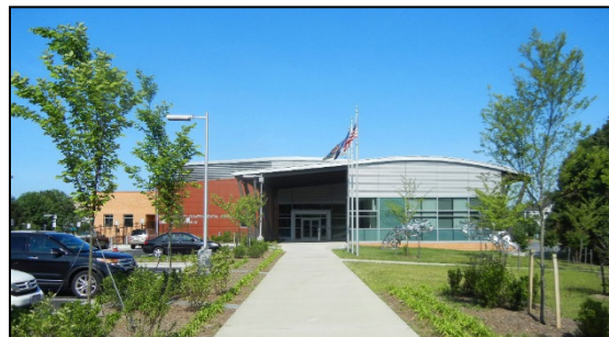
Reston Police Station
