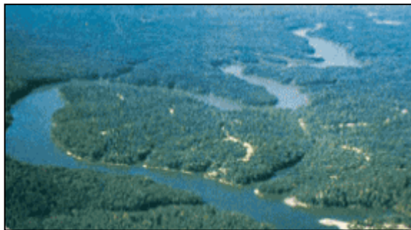
Picture of the Occoquan Reservoir, one of Fairfax County's two principal sources of water.
