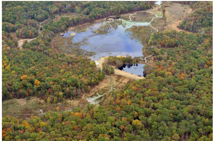
Photo of the Huntley Meadows wetland restoration project
