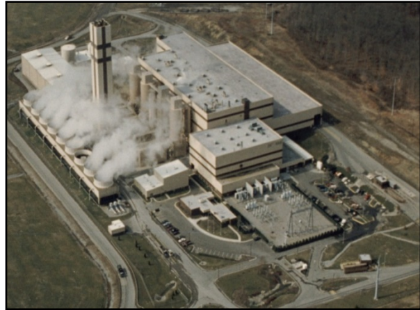
I-95 Energy/Resource Recovery Facility
