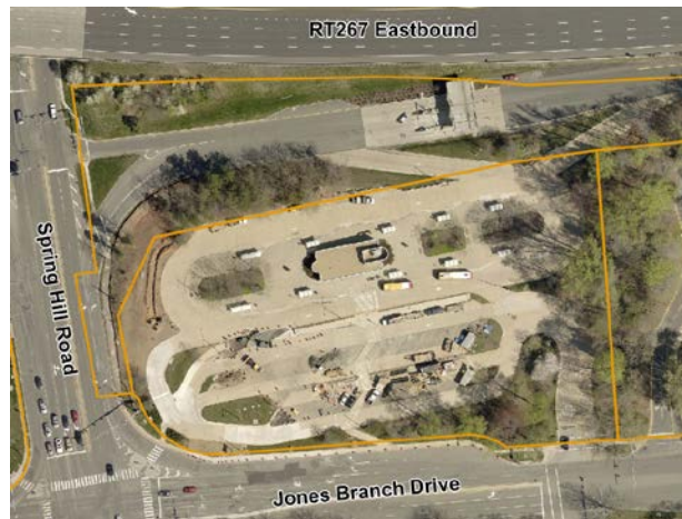
Current Transit Site
