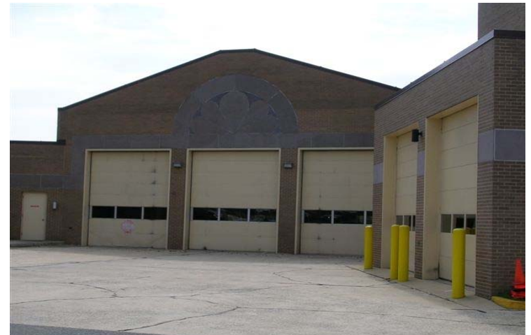
Fair Oaks Fire Station
