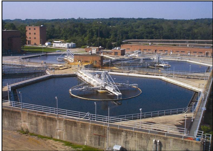
Photo of the Norman M. Cole Jr. Pollution Control Plant
