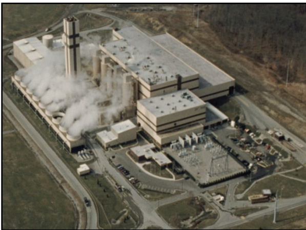
I-95 Energy/Resource Recovery Facility
