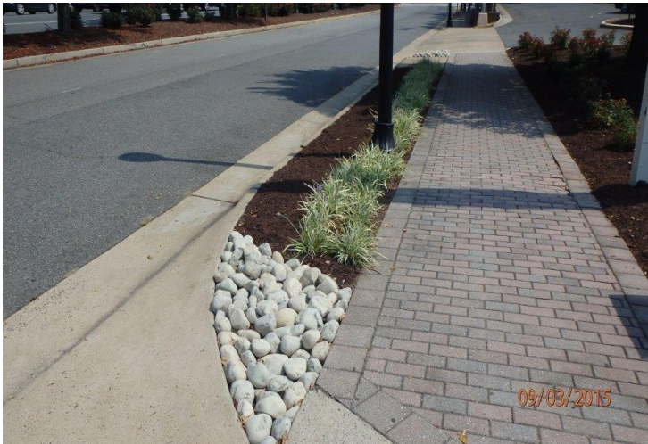
Annandale Service Road - After
