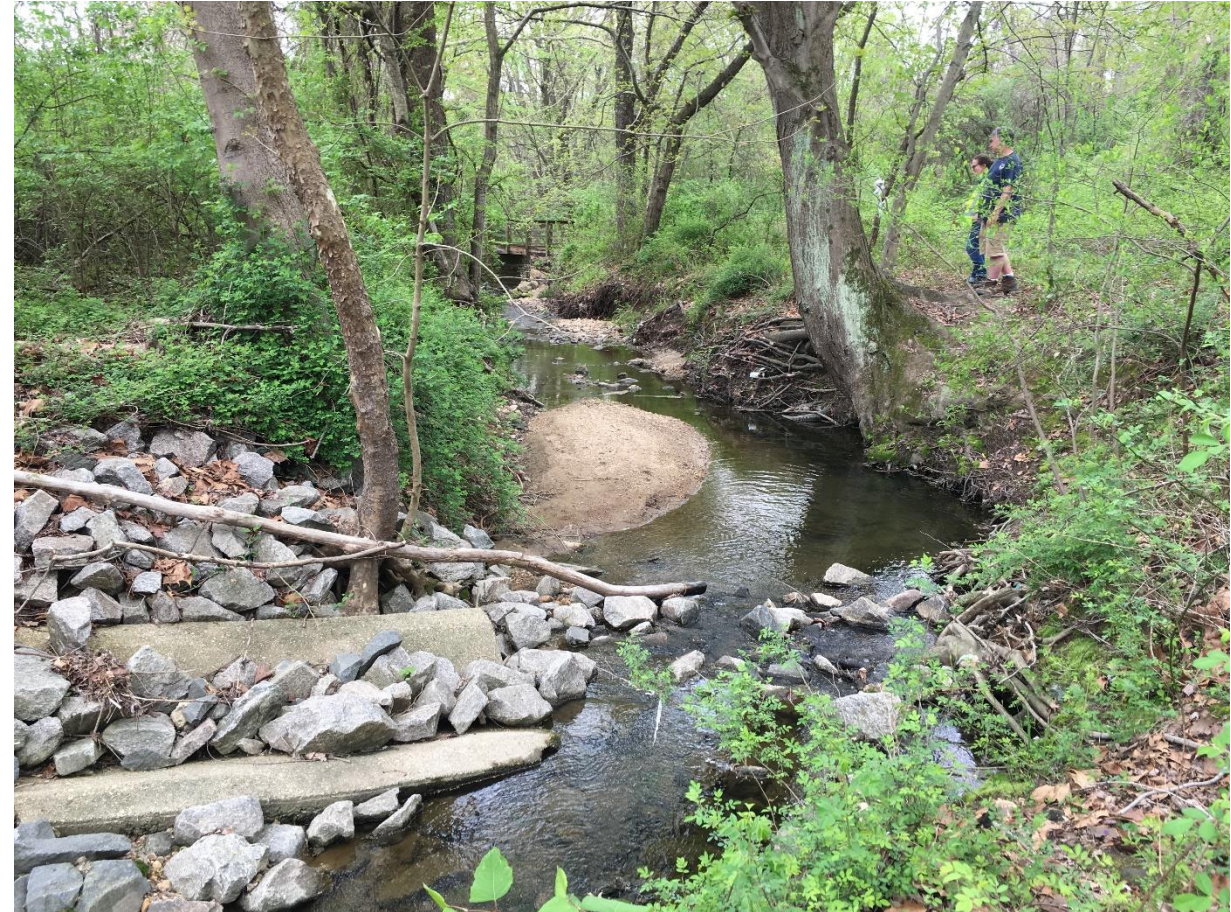
Undermined Concrete Ditch: Long Branch in Smokewood Park Downstream of Whiteacre Dr
