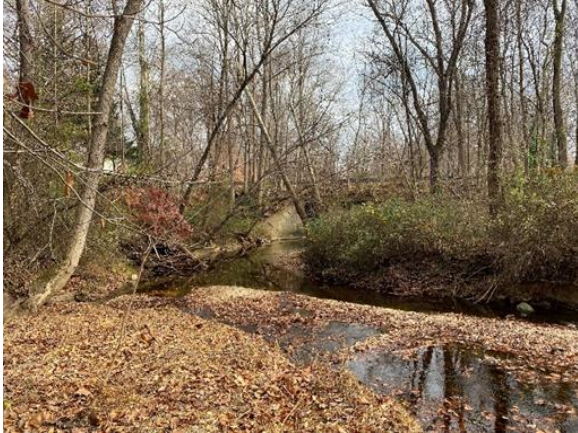
Widening stream channel with poor alignment into downstream culvert; large supply of sediment and streambed material in front of two culvert openings.
