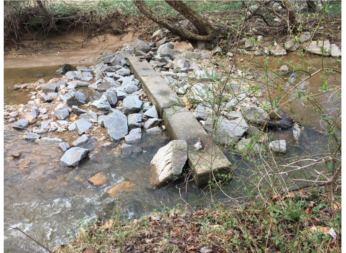
Old Grade Control Structure: Long Branch Main Stem Canterbury Woods Downstream of Woodland Way
