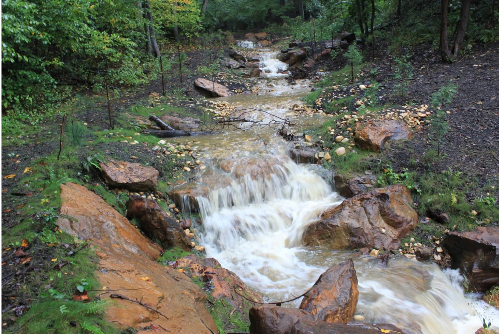
Regenerative Stormwater Conveyance (RSC) Carriage Hills Anne Arundel County, MD
