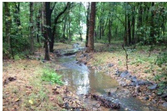
Government Center Stream Restoration Before and After
