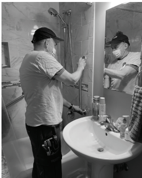
Installing shower grip bars.
