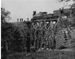
Orange and Alexandria Railroad Trestle
