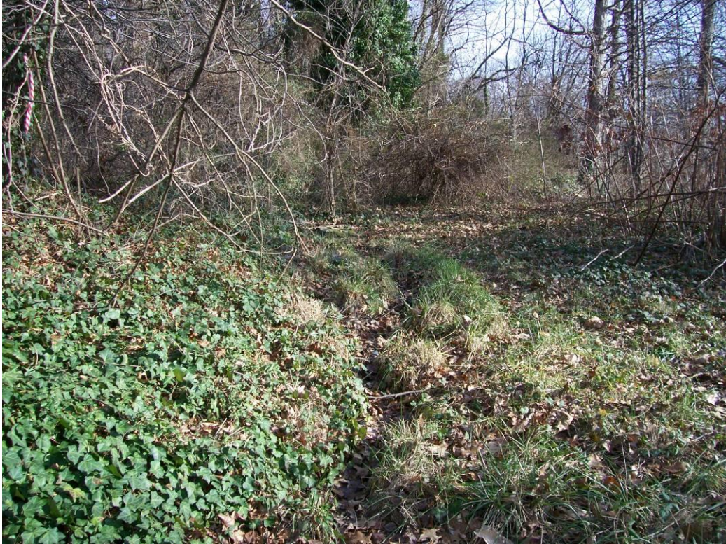
Photograph 4. Drainage pattern created from a culvert, located near Route 1. Photograph Direction: East
