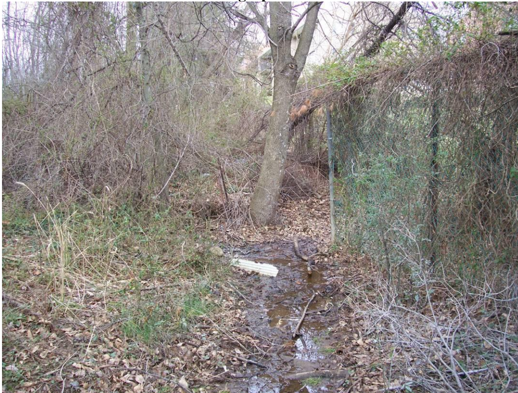
Photograph 15. View of an on-site drainage swale near the eastern property boundary at DP-1. Photograph Direction: Northeast
