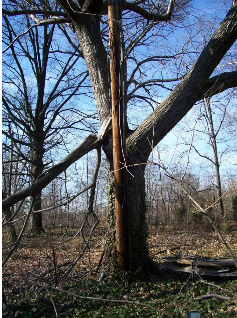
Photograph 7. View of tree number 339 with broken limbs and adjacent utility pole. Photograph Direction: West
