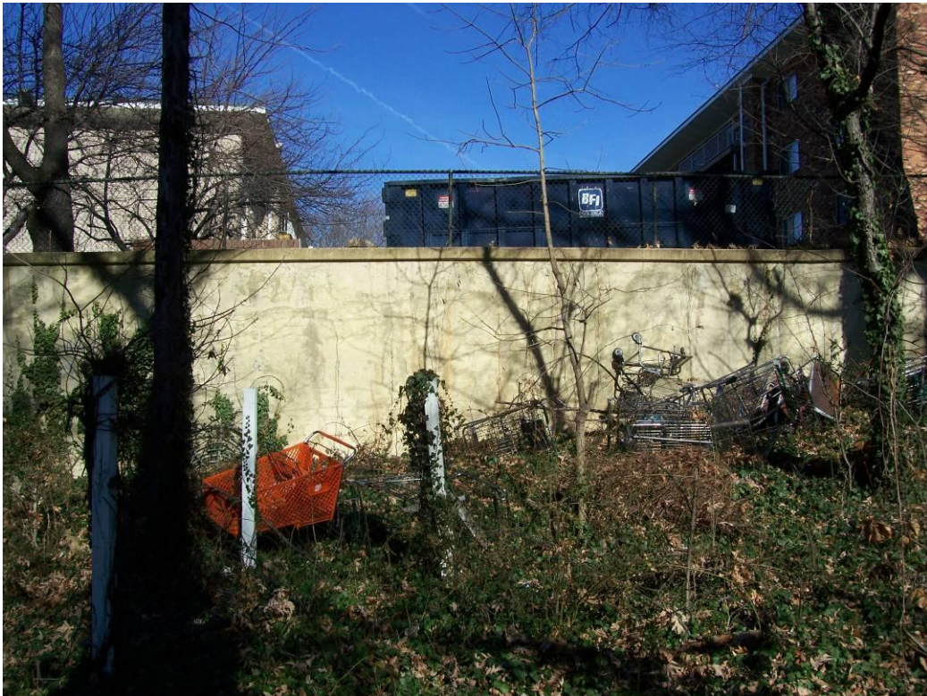
Photograph 9. Shopping carts and debris located along the northern site boundary. Photograph Direction: North
