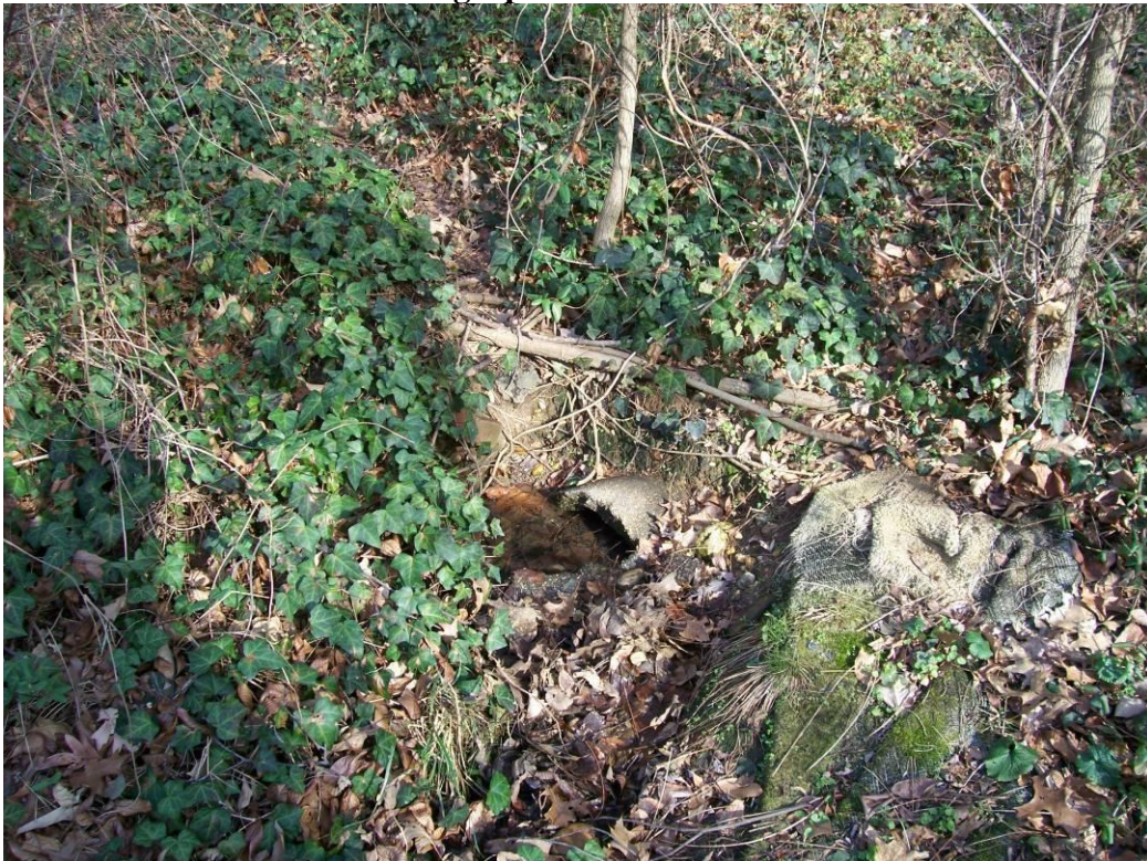
Photograph 5. Underground concrete culvert which empties into the drainage pattern, as shown in Photograph 4. Photograph Direction: Northeast
