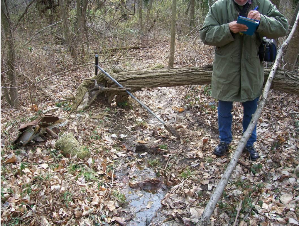
Photograph 18. View of on-site drainage swale at DP-2. Photograph Direction: South
