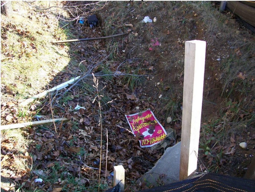
Photograph 2. View of a culvert with silt fencing directly adjacent to Route 1. Photograph Direction: East
