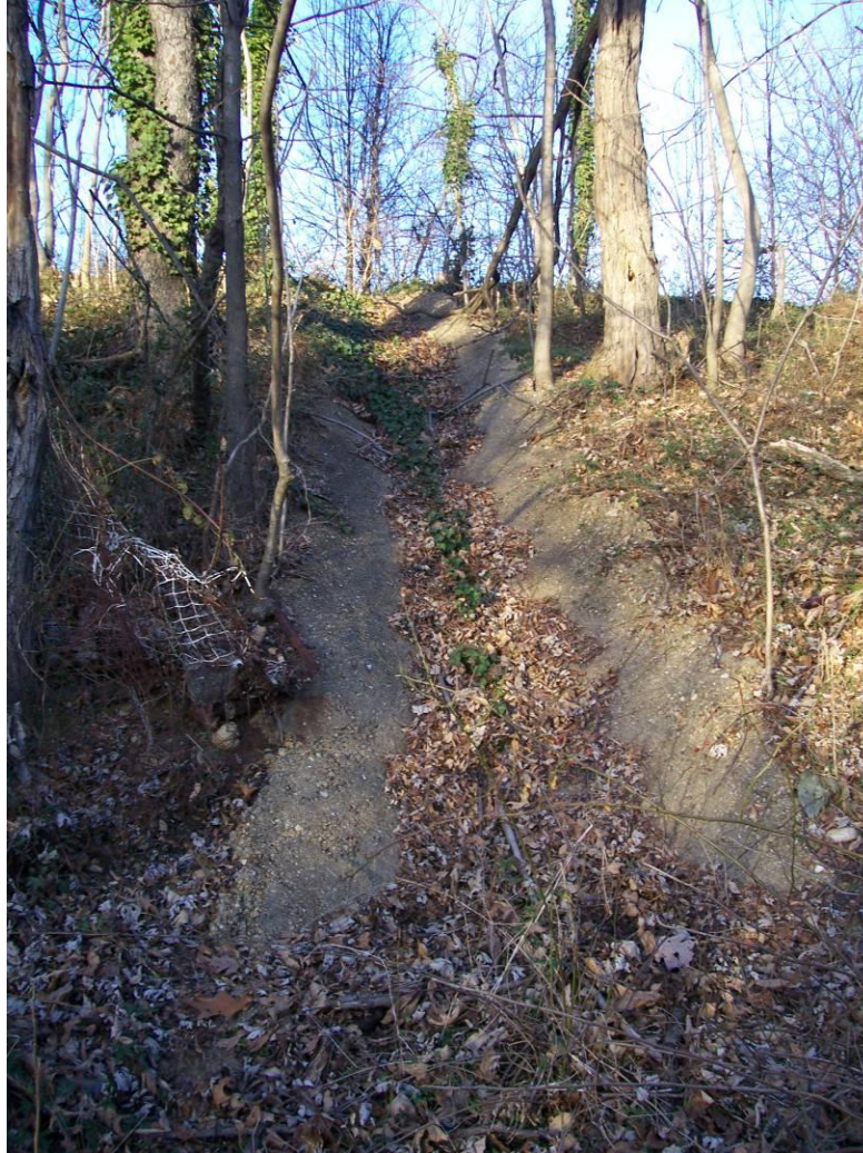
Photograph 11. View of a concrete drainage, which leads into a ground grate. Photograph Direction: Northeast
