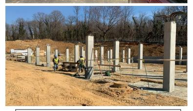
*Pictured From Top to Bottom:* Rendering of the Residences at North Hill Development; Dart Drive looking west toward Richmond Highway; Building 3a structural columns to first floor.
