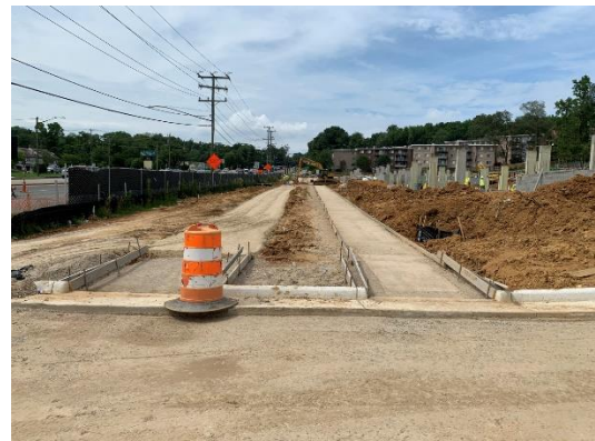
Pictured From Top to Bottom: Rendering of the Residences at North Hill Development; view from right to left of building 1A columns and building 2A podium slab and elevator shaft; bike trial and sidewalk along Richmond Highway
