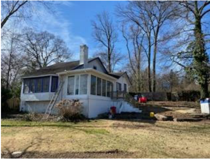
Rear of existing house
