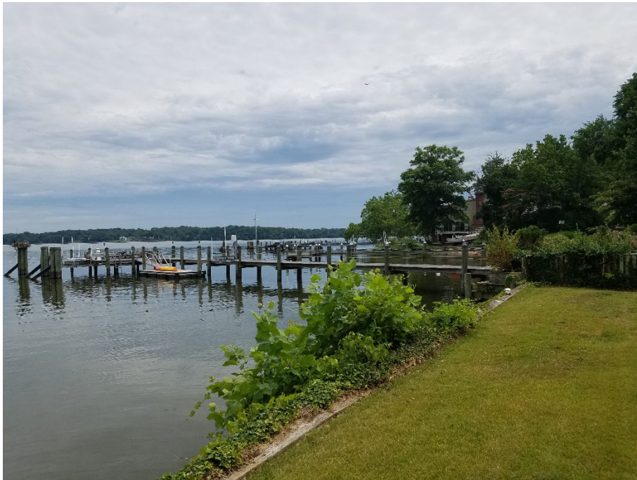
View of Bulkhead wall looking south. Pier on adjacent property
