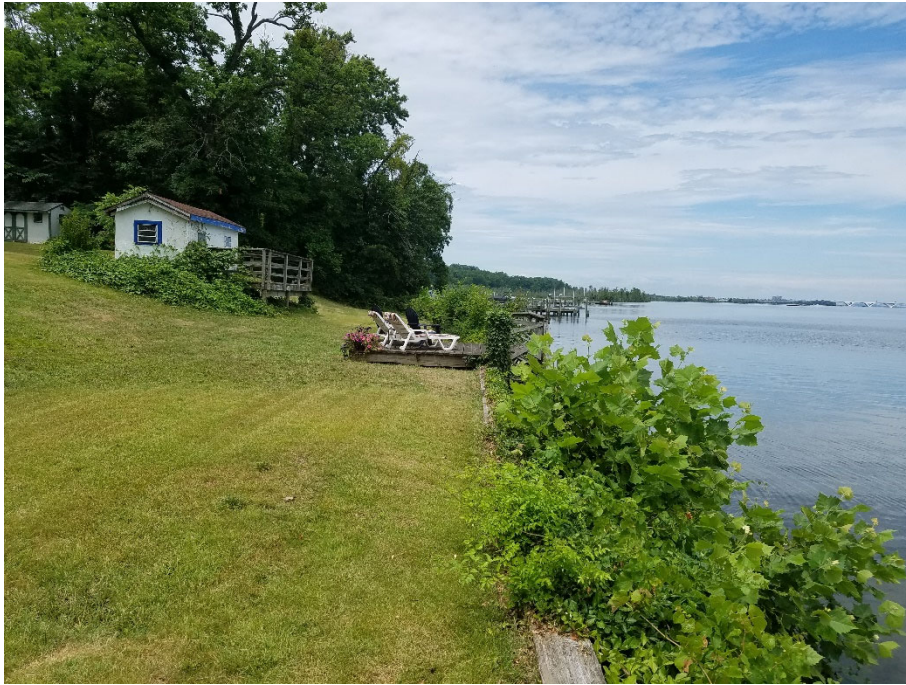
View of Bulkhead wall looking North
