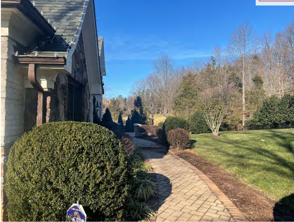
Photograph 3: View to the north showing the front walkway and house.
