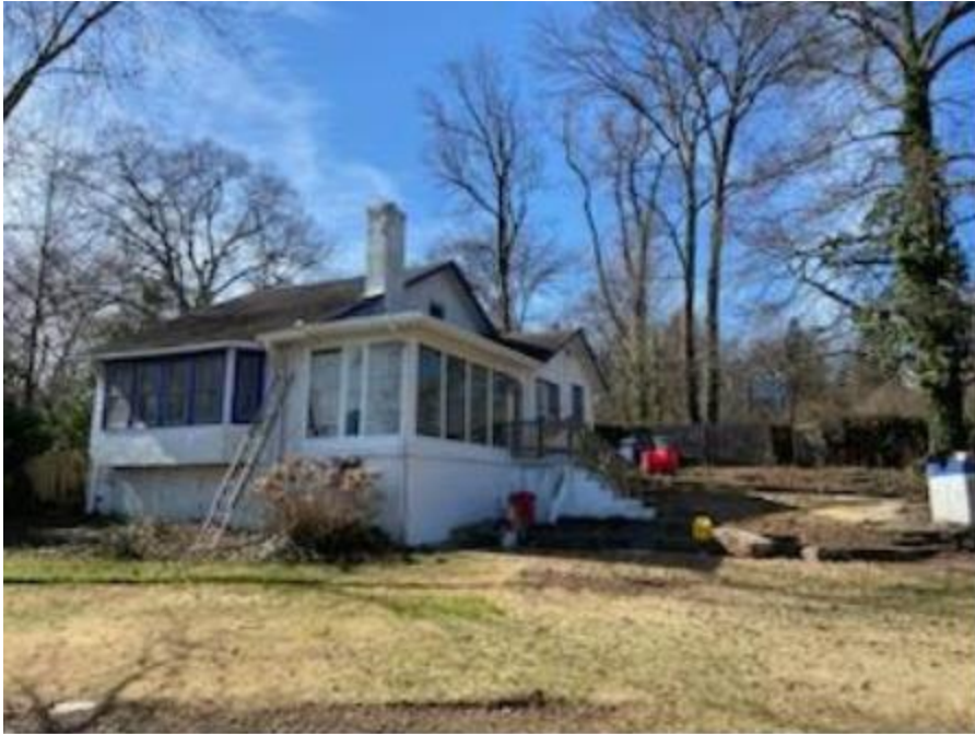
Rear of existing house
