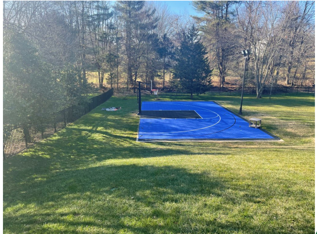
View of the existing sport court facing west
