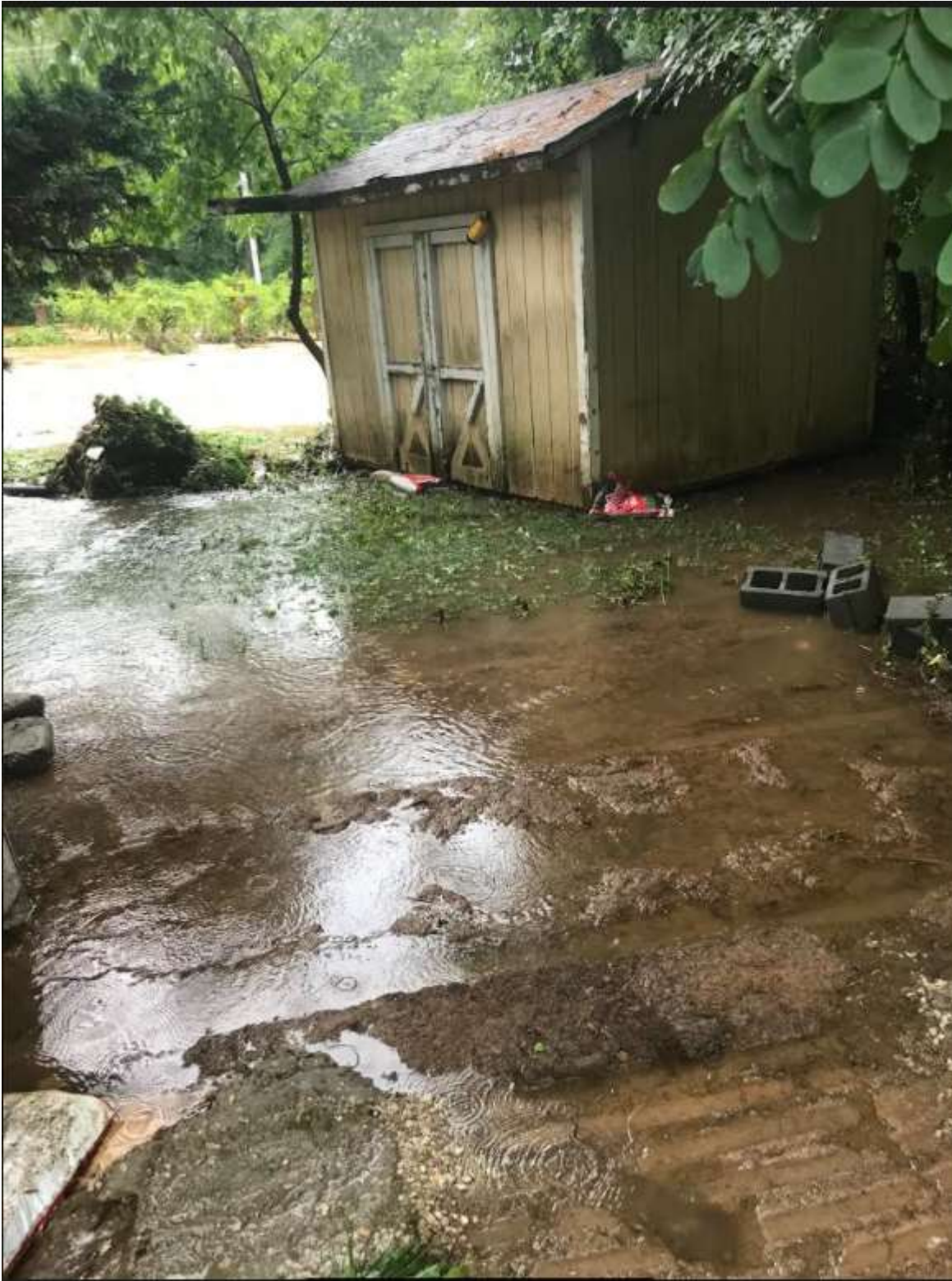
PHOTO 1: POINTING NORTH, PHOTO OF 10' x 12' SHED MOMENTS AFTER FLOODING EVENT ON JULY 8, 2019. NOTE THE BARE EARTH NEAR BOTTOM OF PHOTO WHERE SHED EXISTED PRIOR TO MOVEMENT VIA FLOATATION.
