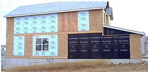
FIGURE 6: INTERMITTENT BRACING
