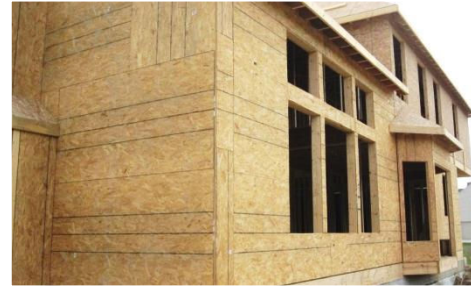
FIGURE 7: CONTINUOUS-SHEATHING
