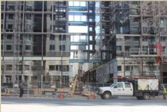
Project Under Construction
