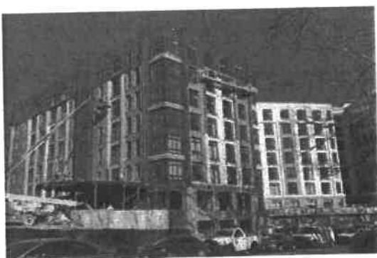
Lake Anne House Construction Progress as of Winter 2021
