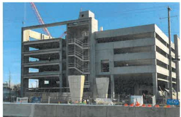
Commuter parking facility under construction
