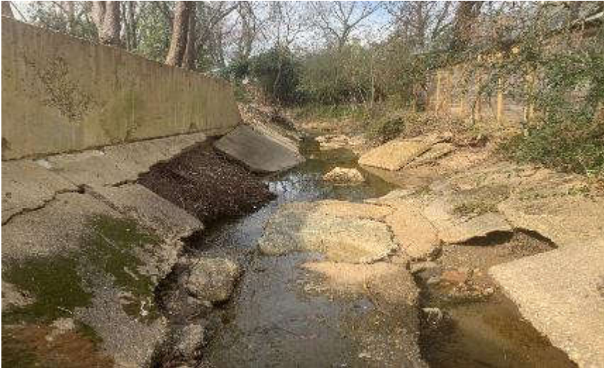
Stormwater Conveyance Channel In Kent Gardens Neighborhood Dranesville District Pimmit Run WS
