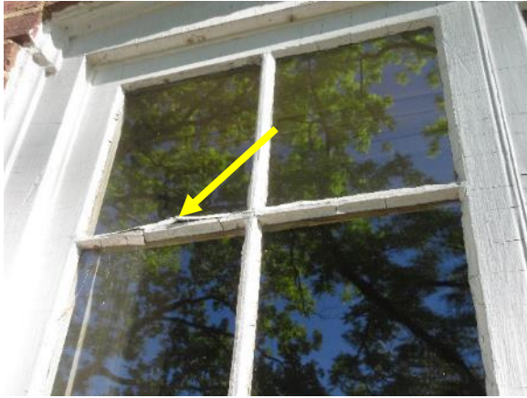
Figure 127. Typical cracked glazing putty at exterior windows.
