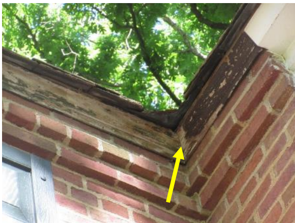
Figure 119. Typical paint deterioration of wood trim underneath roof.
