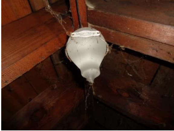
Figure 293. "Sure stop" fire grenades found attached to ridge of attic. These were used to extinguish fires.
