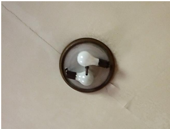
Figure 201. Typical bedroom light fixture with missing glass globe.
