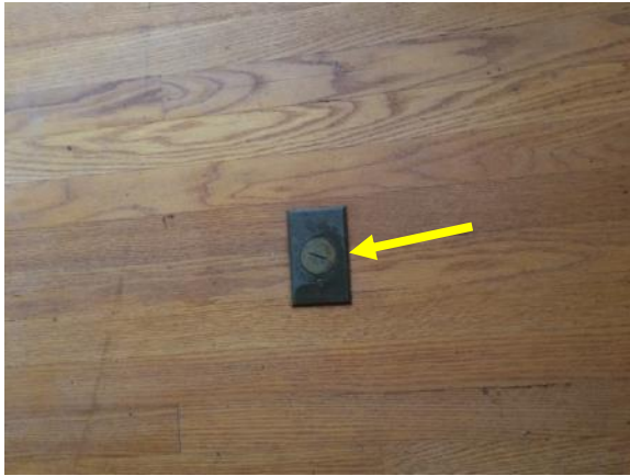
Figure 177. Metal outlet plate on floor of dining room.
