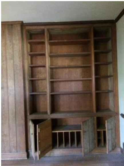
Figure 225. Built-in shelving and cabinets on north wall of living room adjacent to fireplace.
