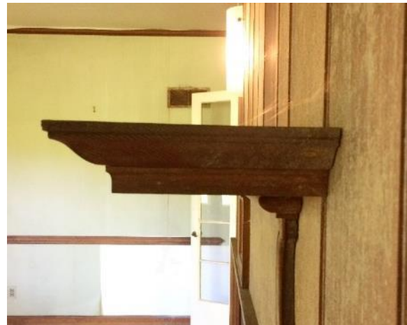
Figure 222. Detail view of mantle over fireplace.
