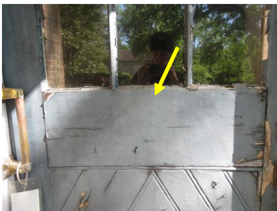
Figure 135. Typical faded and peeling paint at exterior doors.
