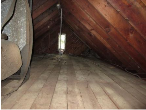
Figure 287. Wood attic floors above center core of home, looking south.
