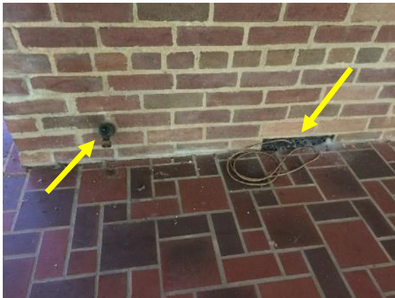
Figure 243. Spigot and decorative metal vent register located on the south wall of the glass porch. These appear to be original to the house and were enclosed with the addition of the porch.
