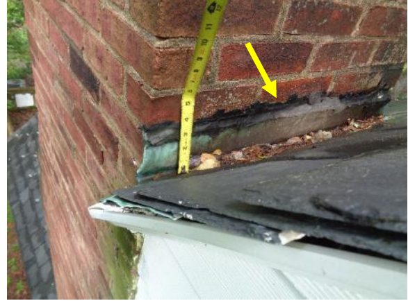
Figure 110. Copper chimney flashing on south chimney with mastic repairs.
