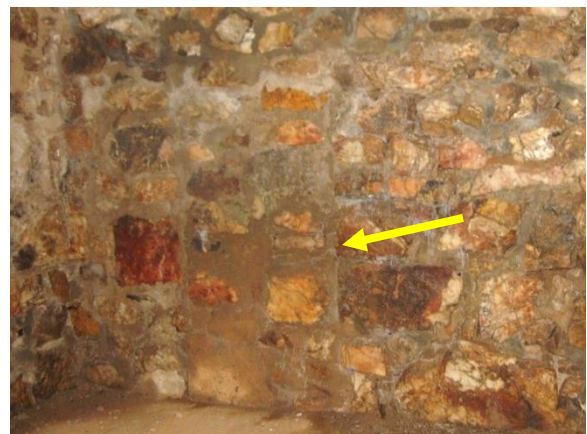
Figure 405. A rectangular opening can be seen in fieldstone wall at the northwest corner of the basement interior wall.
