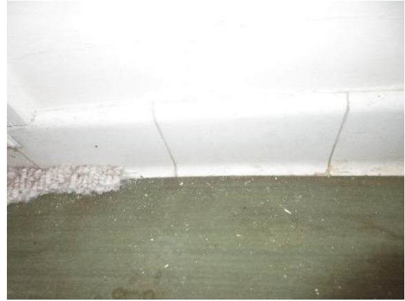
Figure 329. Subflooring under debonded carpet in Bathroom B.
