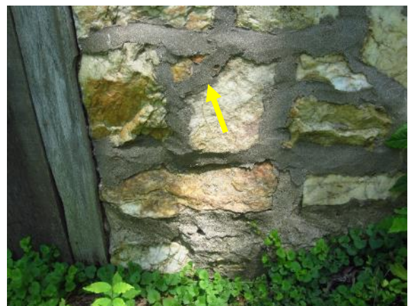
Figure 345. Dark gray mortar on south side of the barn.
