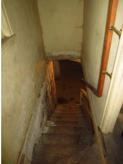
Figure 149. View of basement staircase from top of stair.
