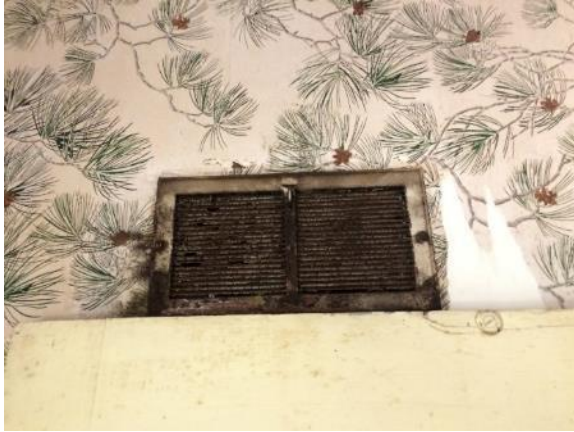
Figure 334. Typical blocked and corroded vent register.
