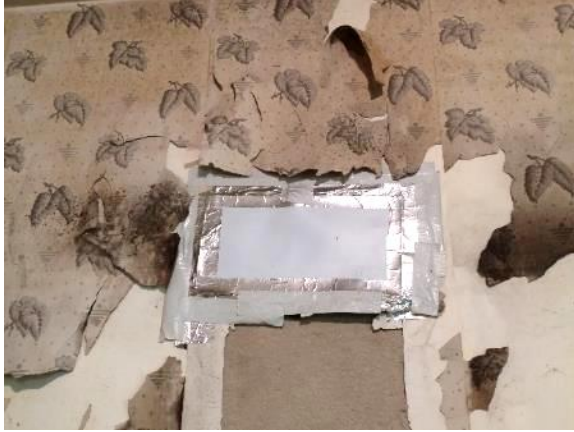
Figure 203. Vent on south wall taped over in Bedroom D.
