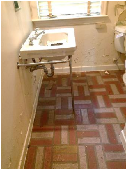
Figure 205. View of typical finishes in first floor bathroom looking north. Side view of original console sink.
