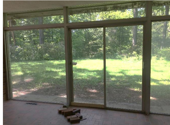
Figure 234. Sliding glass doors located on north wall of glass porch,
