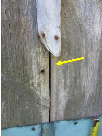
Figure 370. Missing wood batten.
