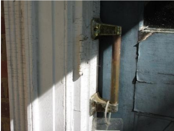
Figure 67. Retrofit handle added to front door frame, typical of other exterior retrofit handles.
