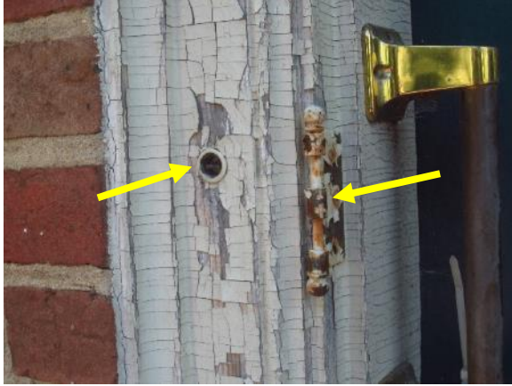
Figure 73. Missing doorbell and abandoned hinges located on frame of west exterior door.
