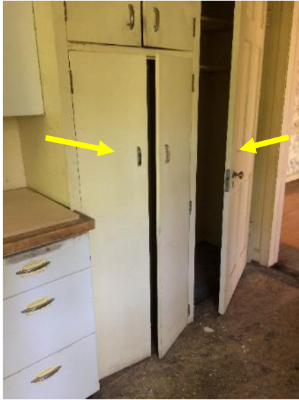
Figure 193. View of large cabinet on north wall and pantry door.
