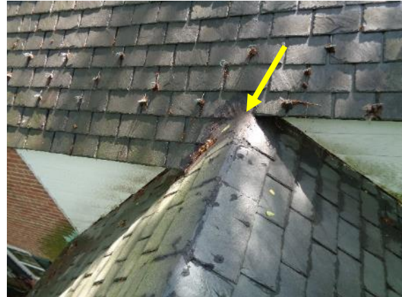
Figure 104. Intersection of west wing roof to main north-south gable roof. Note the repair with mastic at the ridge and meeting point.
