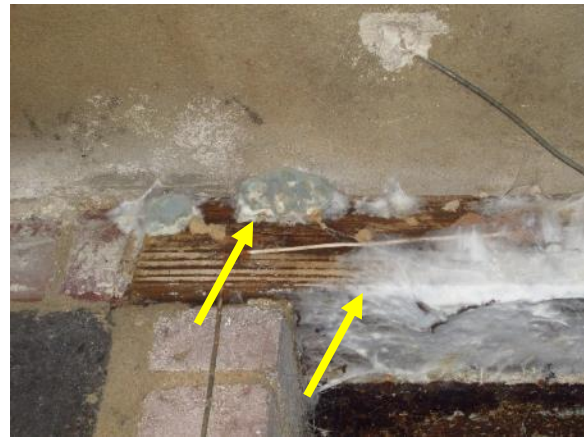
Figure 134. Potential microbial growth and rot on wood lintel in basement.
