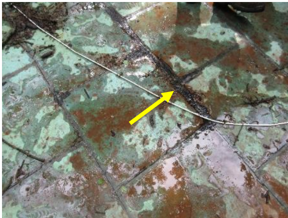
Figure 113. Copper flat-lock soldered seam roof. Note the seams that have been repaired with mastic.
