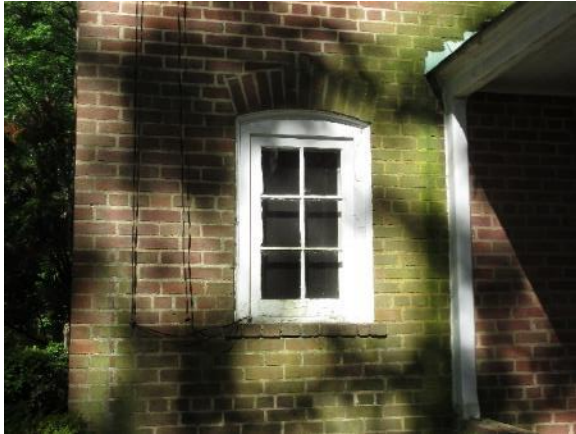
Figure 51. Typical six-paned single casement window (east facade).
