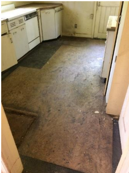
Figure 179. View of kitchen floor, looking west.
