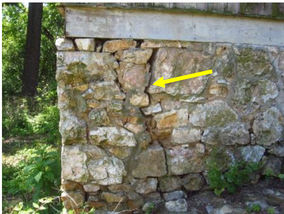
Figure 362. Displaced stone foundation and cracked mortar on north side.
