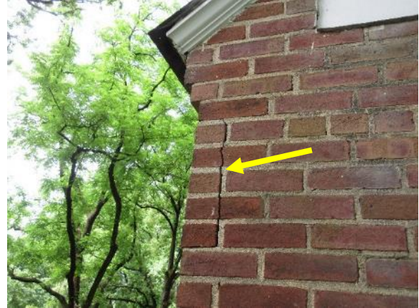
Figure 80. Vertical cracking at south east corner.
