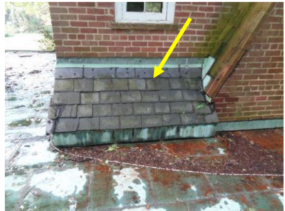
Figure 34. Small roof located adjacent to the north chimney.
