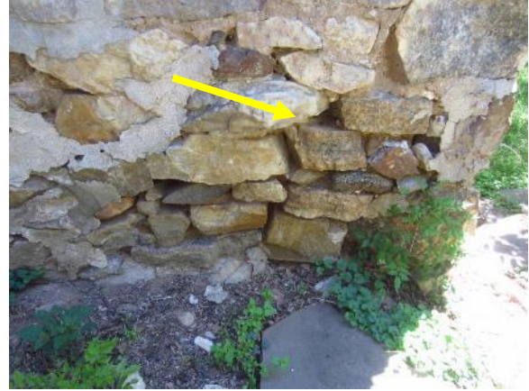
Figure 365. Missing mortar on west end.
