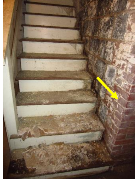
Figure 150. View of basement staircase from bottom of stair at basement. Note brick at corner.
