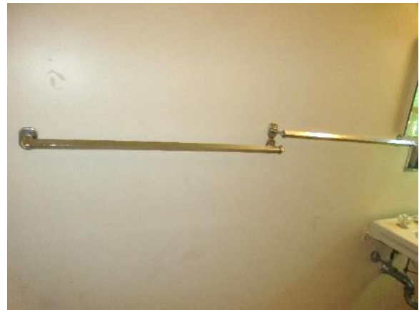
Figure 272. Metal towel bars on west wall of Bathroom B.
