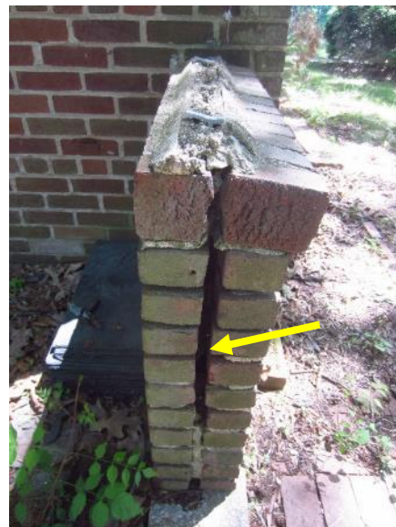
Figure 84. Missing mortar from greenhouse wall collar joint and bed joints.
