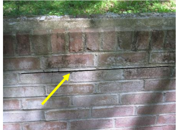
Figure 86. Horizontal crack through mortar on greenhouse wall. Crack traced for clarity.
