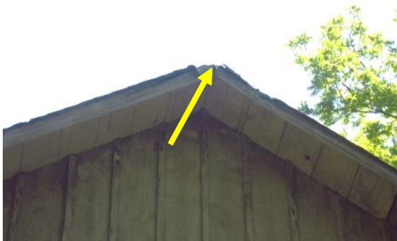
Figure 386. Missing shingles along ridge of barn at west gable end.
