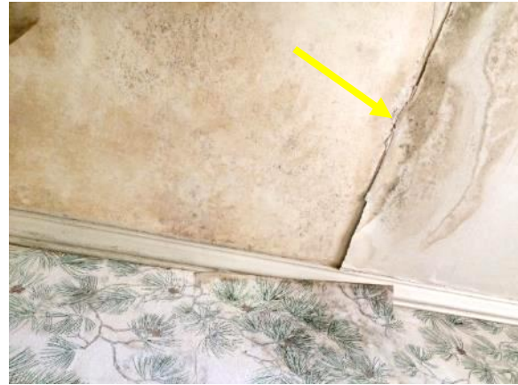
Figure 299. Potential microbial growth at ceiling due to water infiltration in dining room.
