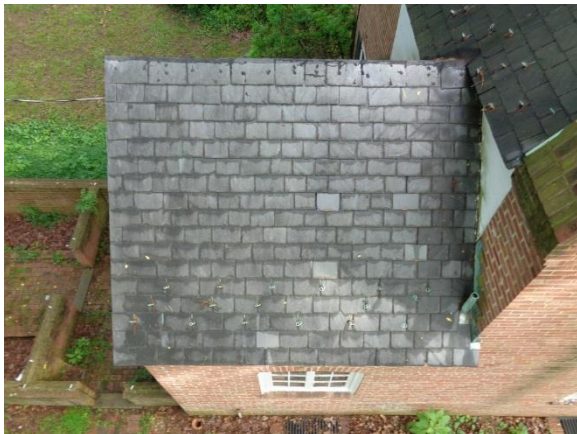
Figure 33. Roof above west wing that terminates into north-south core of home.
