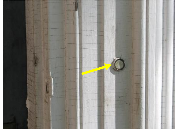
Figure 68. Front door doorbell, painted white, located on door frame.
