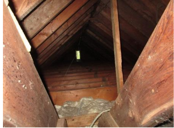
Figure 288. Floor joists are exposed in attic space above east wing. Note the attic window under the east gable end.
