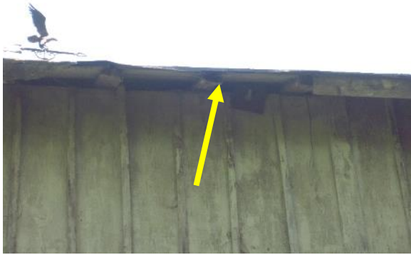
Figure 388. Missing wood along south eave.
