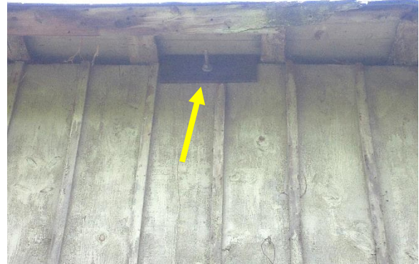
Figure 341. Typical tie-rod metal plate, threaded rod and nut.
