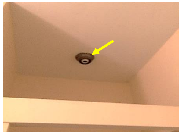
Figure 214. First floor bathroom light fixture above shower missing bulb and glass globe. The fixture is typical for Bathroom B as well.
