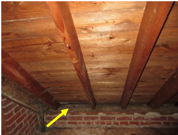
Figure 281. View of south wall of storage room. The wood rafters meet a wood nailer on top of the brick wall.
