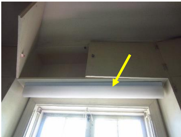
Figure 195. Fluorescent light above sink in kitchen.
