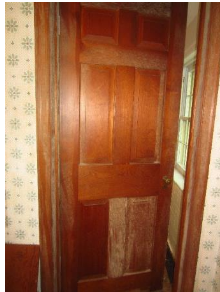
Figure 258. Stained wood door to Bathroom A from Bedroom A.
