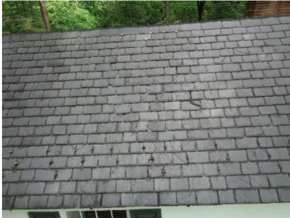
Figure 103. View of east portion of slate roof, typical roof condition for entire roof.
