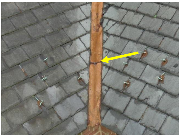
Figure 105. Copper valley between east-west and north-south gable roofs.
