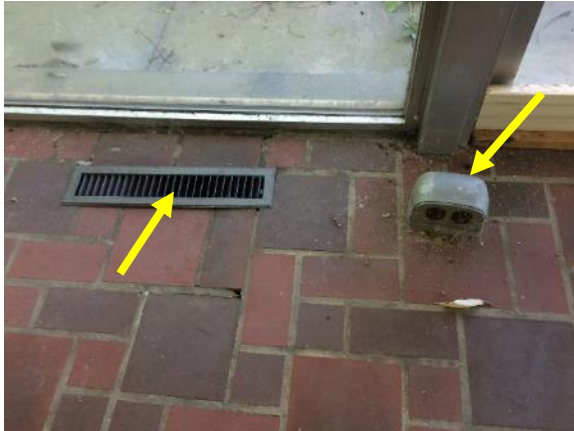
Figure 241. Typical rectangular metal registers and utility ports located along approximately every other IGU in the glass porch.
