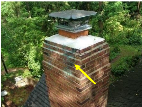
Figure 89. Copper staining due to chimney cap.
