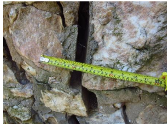
Figure 363. Displaced stone foundation on north side.
