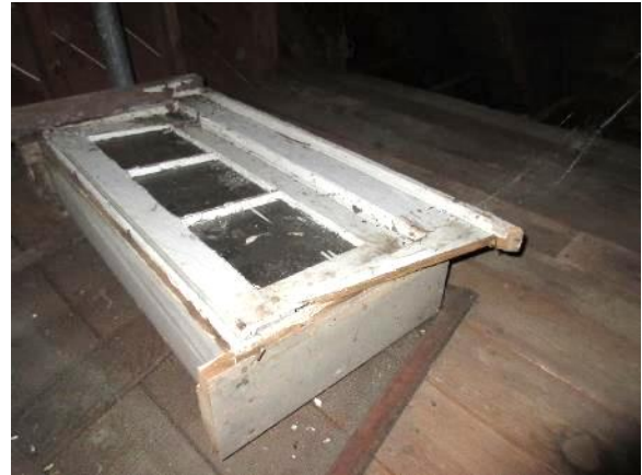
Figure 56. Original casement window that was located in the attic.
