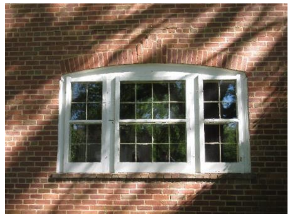
Figure 60. Double hung window assembly on south facade.
