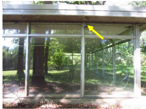
Figure 26. Typical aluminum-framed storefront windows at the glass porch. Note typical floodlight at soffit (yellow arrow).
