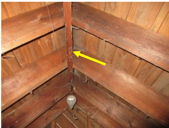
Figure 291. Typical attic ridge beam.
