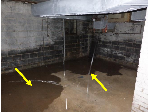
Figure 294. Water infiltration in the basement during an active rain event.
