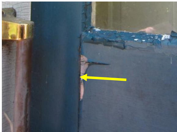
Figure 137. Typical separation of wood between stile and rail on door.
