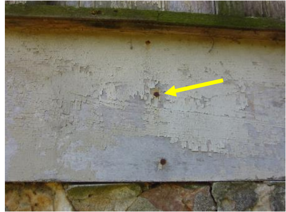
Figure 379. Typical corroding fasteners in wood.
