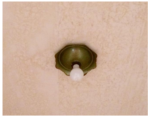
Figure 168. Hallway light fixture with decorative circular metal base and missing globe.
