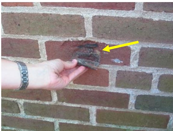
Figure 83. Localized face spall on west facade near exterior door.
