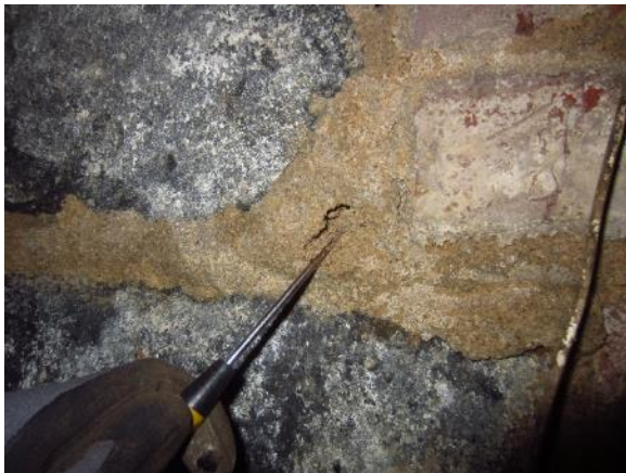
Figure 296. Soft, wet mortar on basement walls.
