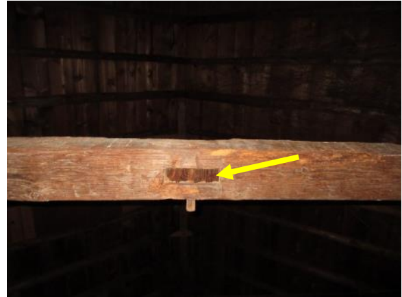
Figure 395. Slot for previous supporting center post on east side of barn. Note the wood dowel that remains from the connection.
