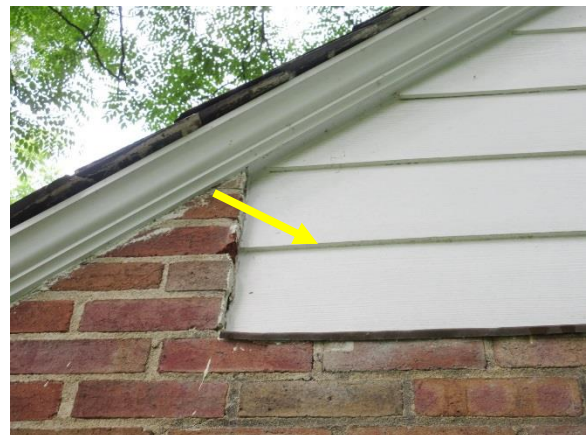
Figure 102. Fiber-cement siding in good condition.
