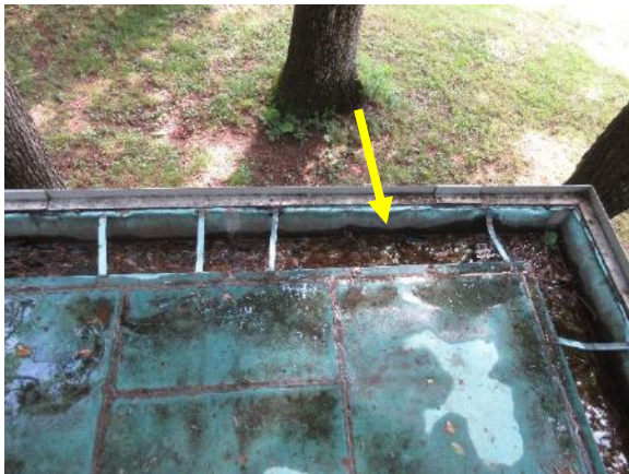
Figure 117. Missing and broken gutter straps along gutter of glass porch.
