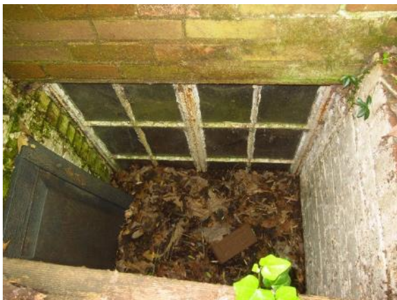
Figure 125. North window with well missing covering grate and debris accumulation. Note miscellaneous shutter stored in window well.
