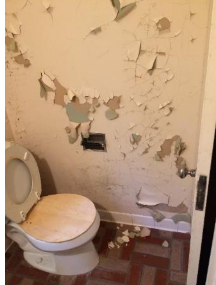
Figure 212. First floor bathroom toilet and toilet paper holder.
