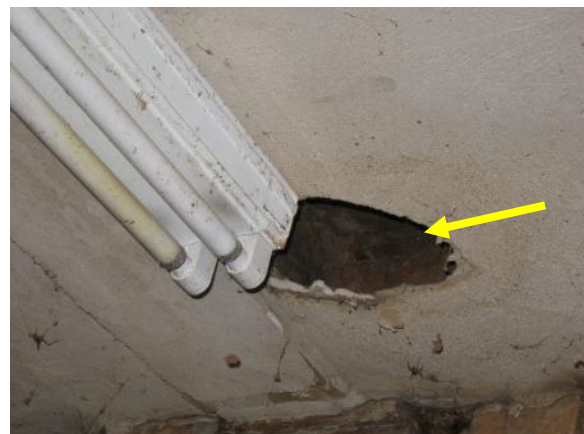
Figure 418. Hole in basement ceiling near east wall.
