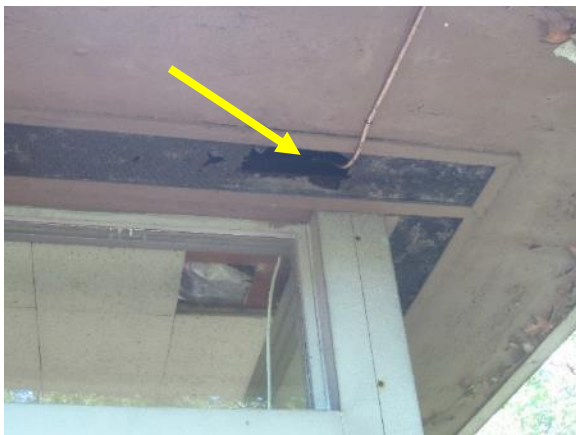
Figure 101. Hole in screen of glass porch soffit with cable fed through opening.
