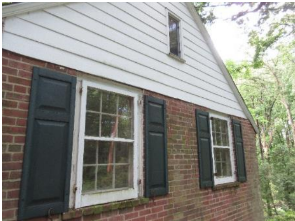
Figure 63. North facade second floor windows are typical 6/6 double hung windows with shutters and exterior storm windows.
