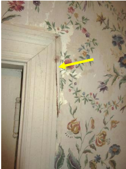
Figure 322. Cracked window casing in Bedroom B.
