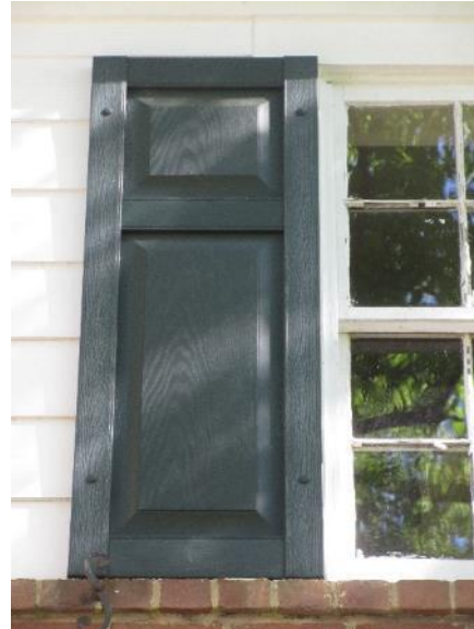
Figure 132. Typical fixed replacement shutter on exterior of home.
