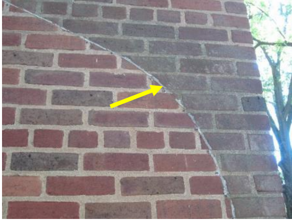
Figure 91. Surface staining and residual sealant and fasteners around previously-attached greenhouse on west facade.
