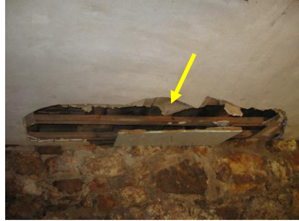
Figure 414. Hole in basement ceiling at north wall.
