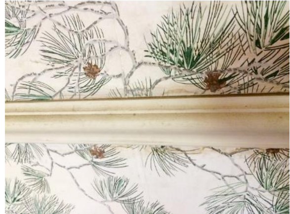
Figure 174. Chair rail in dining room. The profile is typical for all other chair rails in the home.
