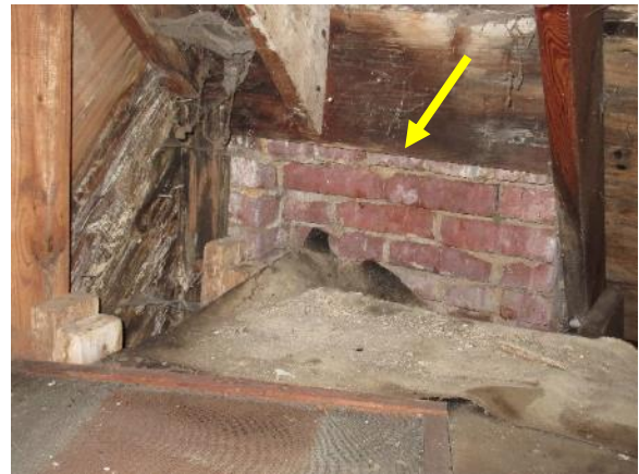
Figure 290. Brick chimney wall at southwest corner of attic above center core. Note moist wood above and adjacent to brick indicating water infiltration.
