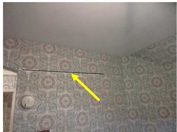
Figure 319. Horizontal crack through plaster in second floor hallway. Crack traced for clarity.
