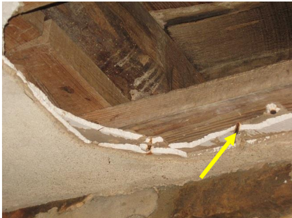
Figure 415. Hole in plaster ceiling at north wall.
