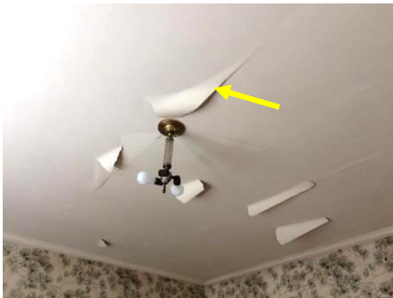
Figure 312. Typical peeling wallpaper on ceiling.
