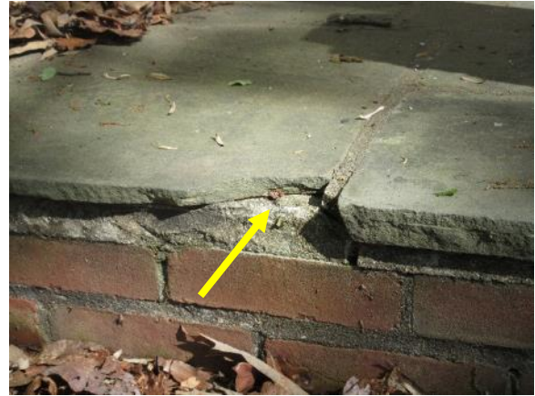
Figure 94. Spalled stone paver on front porch (south projection).
