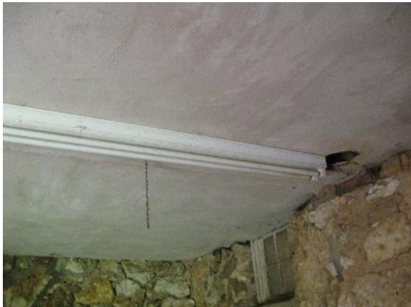
Figure 408. Typical fluorescent lights located in basement of barn.
