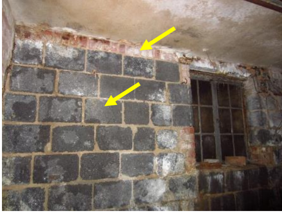
Figure 153. Basement CMU wall with brick course at top.
