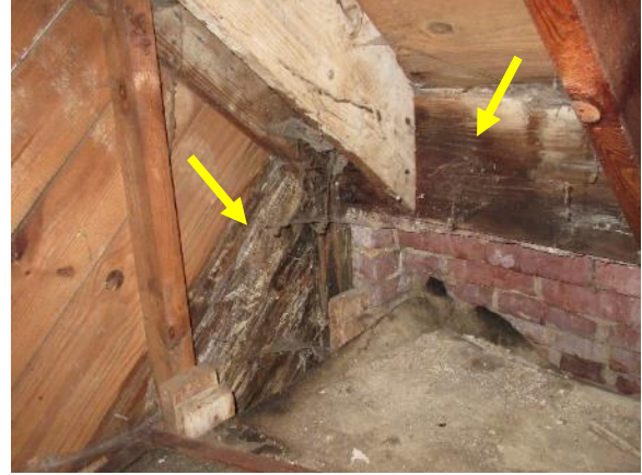
Figure 303. Soft stained wood in attic at southwest corner of house.
