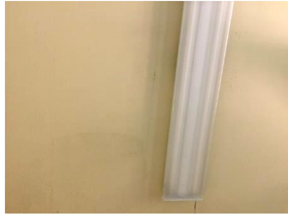
Figure 194. Fluorescent light on ceiling in kitchen.
