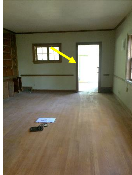
Figure 220. View of east wall of living room and doorway to glass porch. Doors have been removed, but hinges are still in place.
