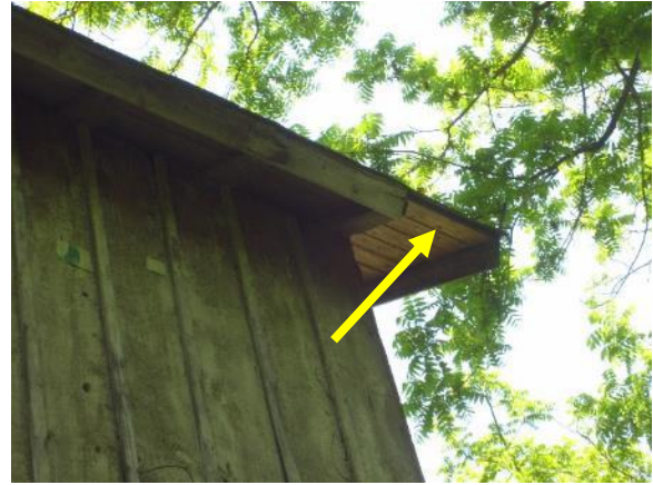
Figure 389. Missing fascia board along south eave.
