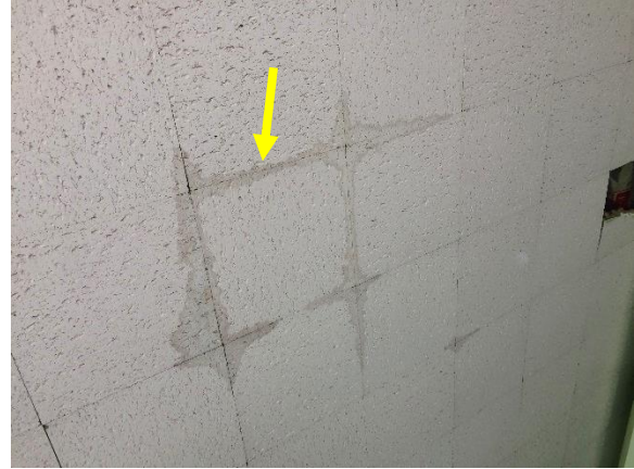
Figure 307. Moisture stains on ceiling tiles in center of glass porch.
