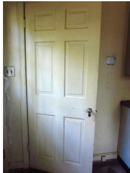
Figure 148. Typical six-paneled wood door with metal doorknob and key escutcheon (kitchen to basement staircase).
