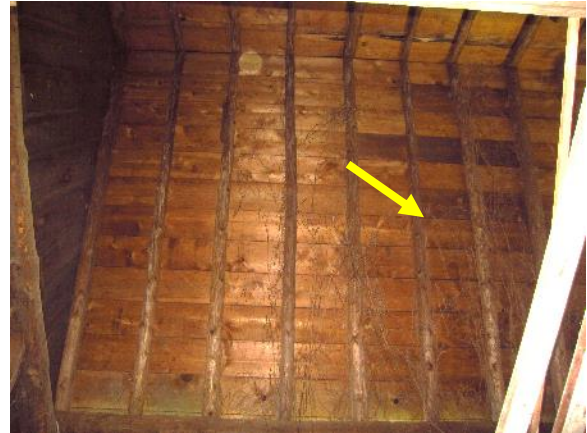
Figure 422. Vegetation on northern roof interior.
