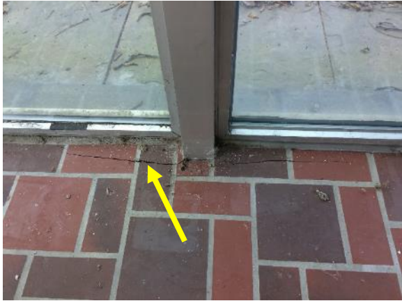
Figure 330. Cracked brick pavers around aluminum frame in glass porch.
