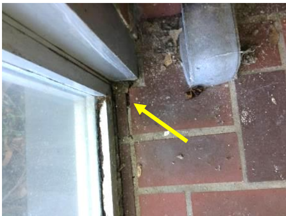
Figure 332. Missing mortar between brick pavers in glass porch.
