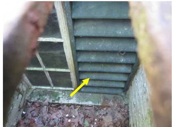
Figure 42. Basement casement window with one sash replaced with a louver.
