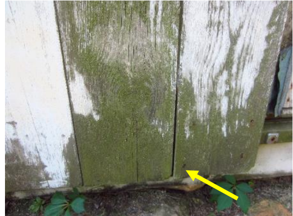
Figure 385. Vegetation growing on bottom of sliding door.
