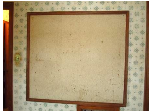
Figure 256. Cork board on west wall of Bedroom A.
