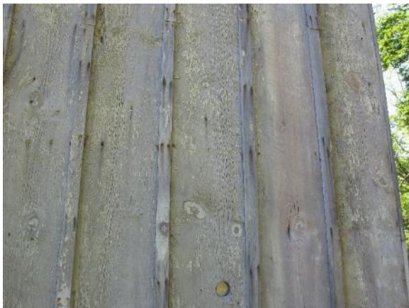
Figure 338. Typical faded wood color on exterior of barn. Remains of white coating can be seen.
