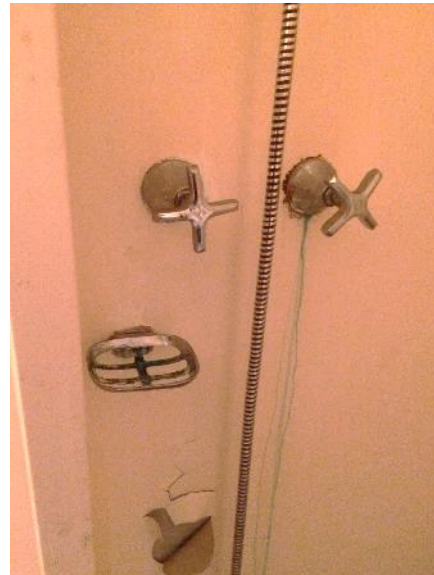
Figure 210. First floor shower faucets and soap holder. Note staining and peeling paint on shower wall.
