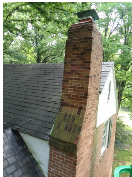
Figure 30. Interior chimney located on the south gable end of the center core.
