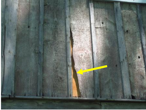
Figure 376. Wood plank attached to interior to cover hole on south side.
