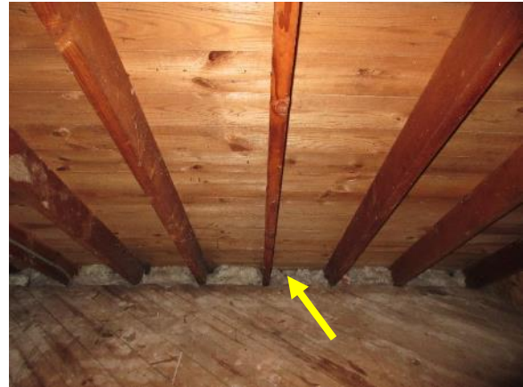
Figure 280. View of north wall of storage room. The wood rafters meet insulation next to the wood floors.
