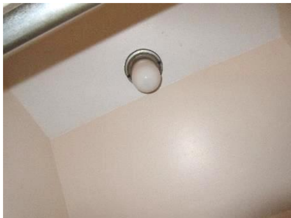
Figure 273. Light fixture located above shower in Bathroom B. Note this fixture's glass globe is still intact.
