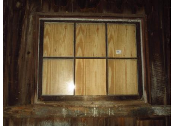
Figure 347. Typical main level barn awning window, viewed from the interior.
