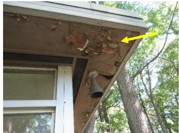
Figure 100. Typical peeling paint on the glass porch soffit.
