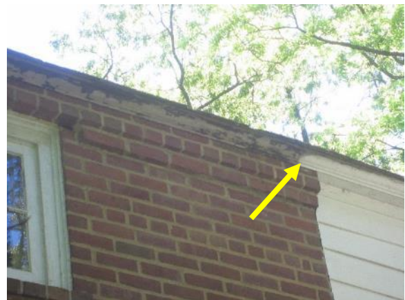
Figure 120. Painted wood trim above siding (west elevation).
