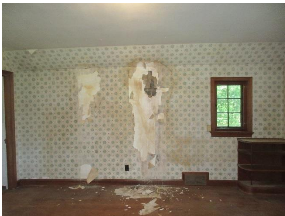
Figure 300. Extensive water staining at plaster, wallpaper and wood floors at north wall in Bedroom A.
