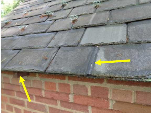
Figure 115. Cut gutter strap hanger and wood block.
