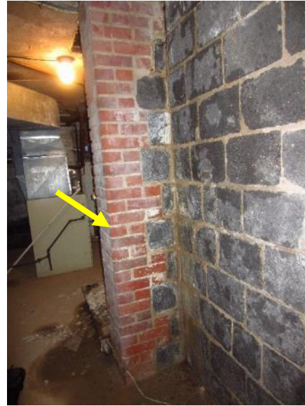
Figure 156. Western-most brick column with CMU tie-in to wall.
