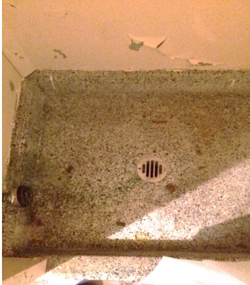
Figure 211. Terrazzo floor and drain in first floor shower. Typical for Bathroom B as well.
