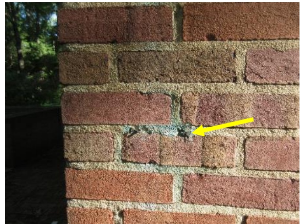
Figure 88. Typical copper staining due to metal fasteners (south facade).
