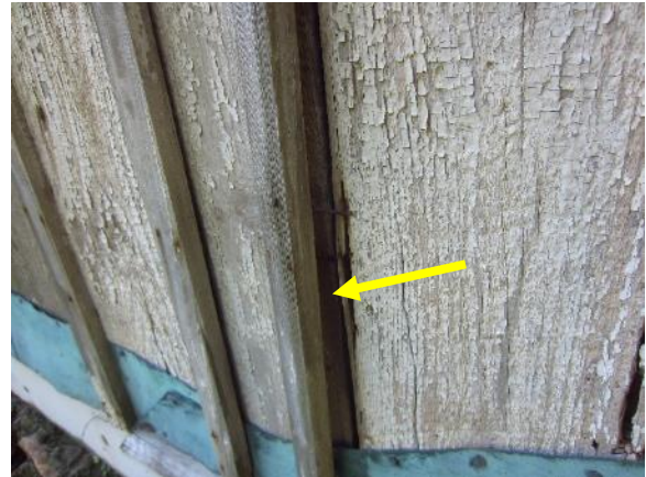
Figure 371. Partially detached batten.
