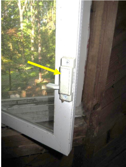
Figure 55. Typical plastic lock on the interior of an attic window.
