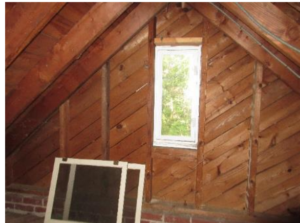
Figure 282. West wall of storage room, under gable. Note the diagonal wood boards and attic casement window.
