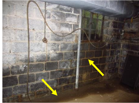
Figure 295. Damp area below window sill and at interface with floor slab several days after a rain event.
