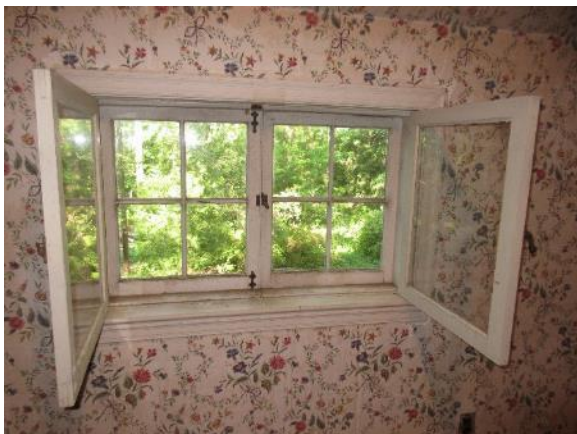
Figure 49. Interior paired casement storm windows on west window in Bedroom B.
