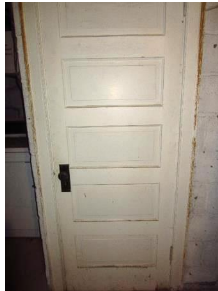
Figure 152. Five-paneled closet door located in the basement.
