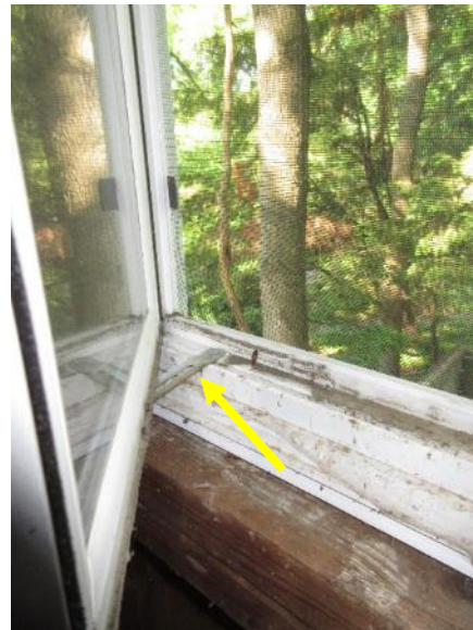
Figure 54. Typical metal hinges for operation of an attic window. The window opens to the interior and has an exterior screen.
