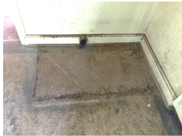
Figure 180. Stained linoleum flooring where kitchen appliance once sat.
