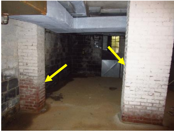
Figure 155. Typical brick columns in basement. Note the white coating on the brick.
