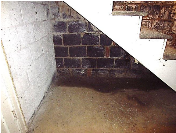
Figure 151. Side view of basement staircase. Note moisture in CMU and edge of slab beyond.
