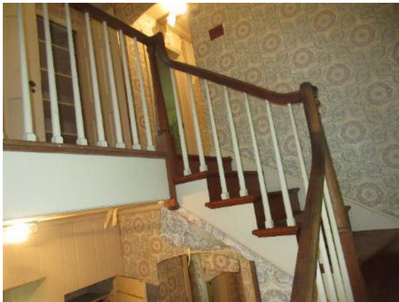
Figure 147. View of landing from staircase.
