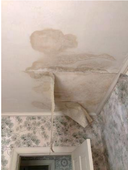
Figure 298. Staining and peeling of wallpaper on ceiling due to water damage in dining room.
