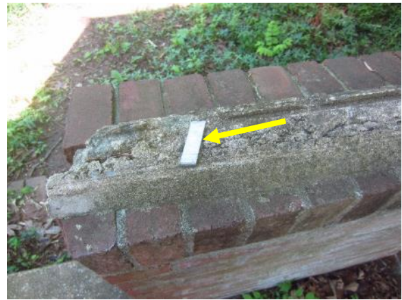
Figure 22. Metal clips remain embedded in the greenhouse walls
