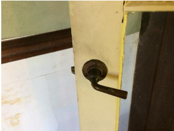
Figure 219. Detail view of the original handle used to open the French doors to the living room.
