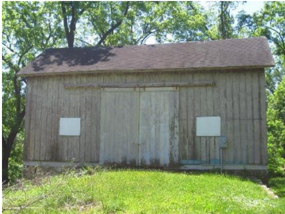
Figure 336. View of barn north side.
