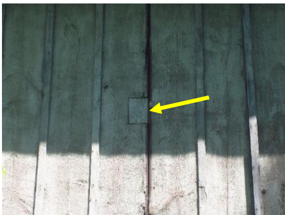
Figure 374. Existing wood dutchman on south side.
