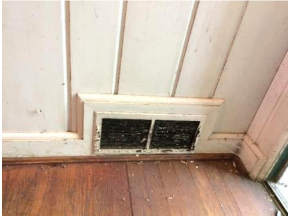
Figure 165. Typical white painted metal vent.
