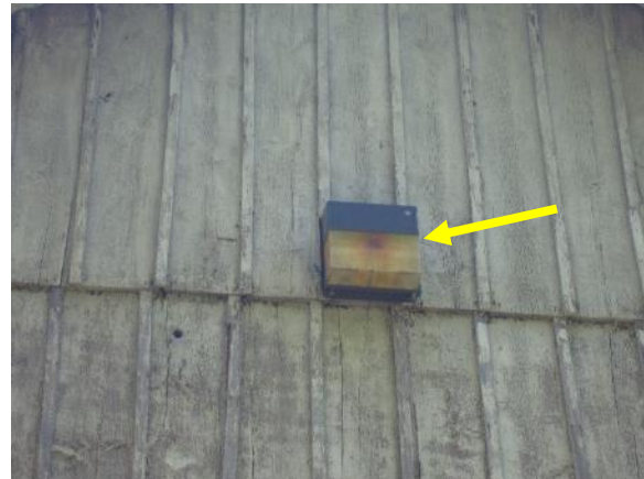
Figure 361. Plastic security light fixture on west end of barn.
