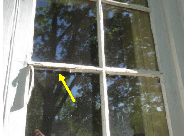
Figure 128. Typical missing glazing putty at exterior windows.
