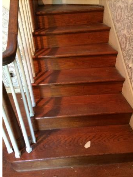
Figure 142. Stained wood treads, risers, and nosings.
