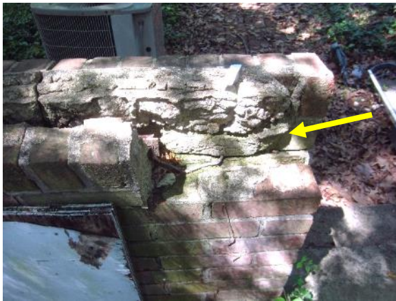
Figure 87. Missing brick units at west end of greenhouse wall.
