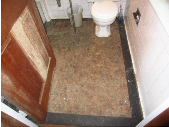
Figure 259. Tan and black marbled linoleum floor with a black border in Bathroom A.
