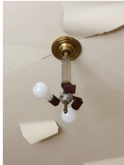
Figure 176. Dining room hanging light fixture. Glass globe and one bulb currently missing.
