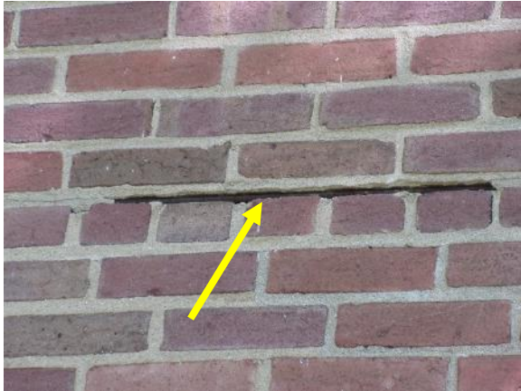
Figure 81. Cracks in mortar at floor line, revealing minor surface corrosion at steel shelf angle behind.
