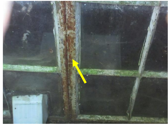
Figure 124. Corroded window casing and sash in basement.
