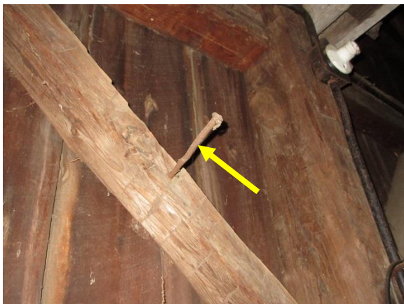
Figure 398. Miscellaneous metal nail extending from typical rough-hewn brace.
