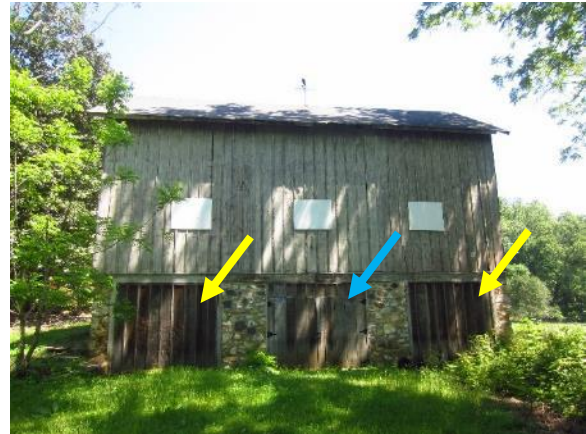
Figure 337. View of barn south side. Note the board and batten infill panels (yellow arrows) and stone columns on either side of the hinged double doors (blue arrow) at the basement level.
