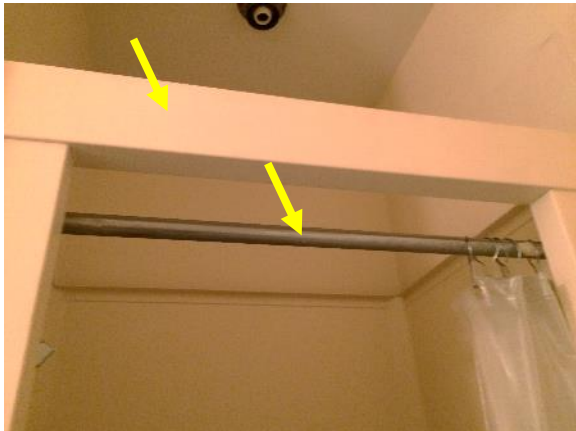
Figure 209. First floor bathroom shower curtain rod and plastic frame.
