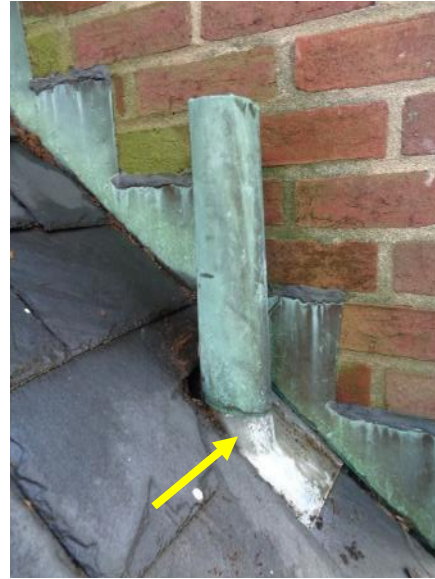
Figure 112. Failed copper counterflashing at pre-fabricated lead flashing boot.
