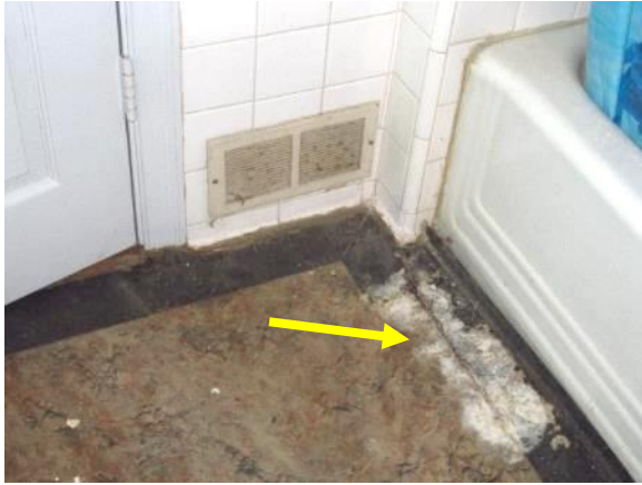
Figure 328. Cracked and blistered linoleum in Bathroom A.
