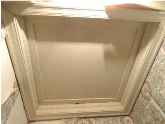
Figure 247. Access hatch located on the ceiling of the second floor hallway.
