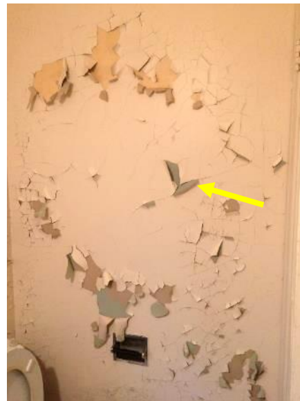
Figure 313. Typical peeling and blistering paint on walls.
