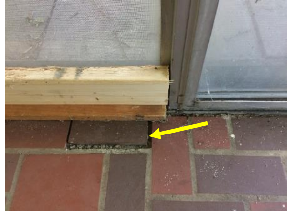
Figure 331. Loose brick paver in glass porch.
