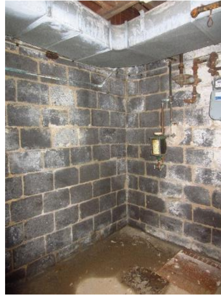
Figure 24. Typical CMU foundation walls.
