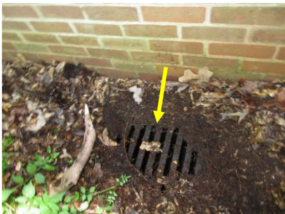
Figure 43. View of west basement window well that has been covered with dirt and foliage.
