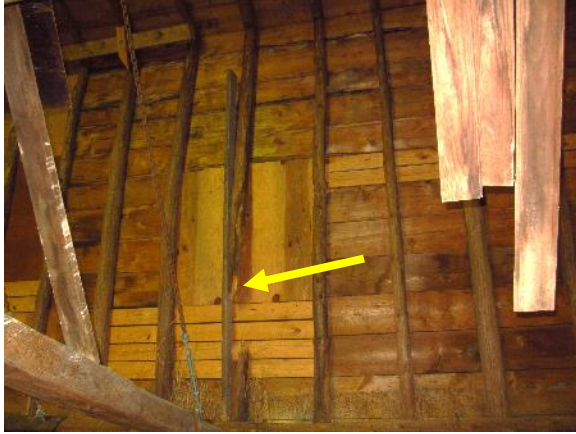
Figure 419. Sistered rafter on southern roof face.
