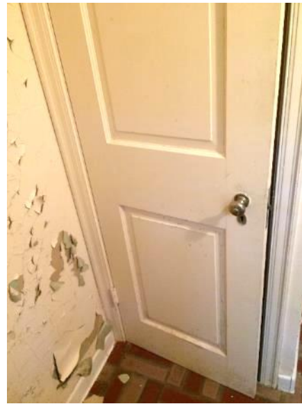
Figure 206. Typical white two-paneled door to bathroom closets.
