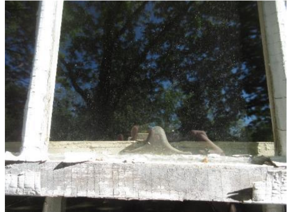
Figure 122. Typical displaced upper and lower sash on double hung windows.
