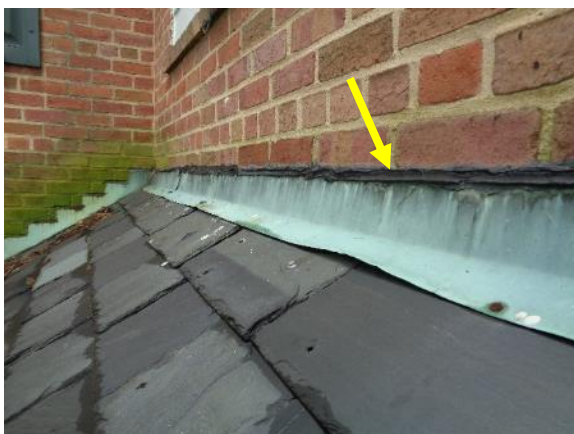
Figure 107. Copper flashing at porch roof. Note the mastic repair at the interface between the copper and the brick masonry.
