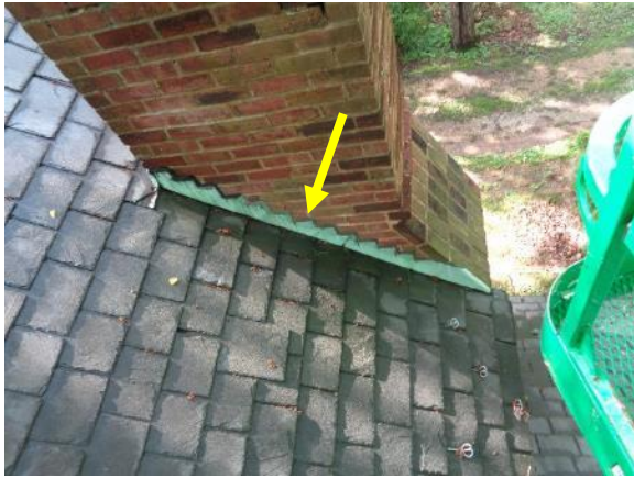
Figure 111. Copper chimney flashing on south chimney.
