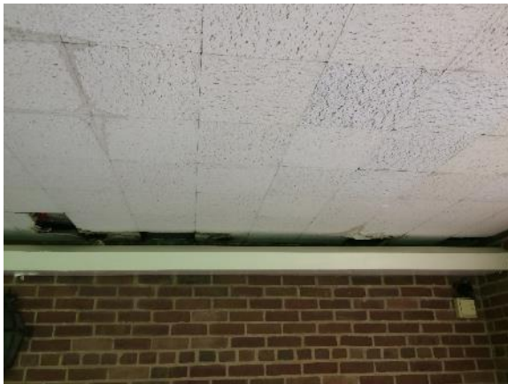
Figure 239. View of the acoustic ceiling tiles, "lighting cove," and brick wall on the south interior wall of the glass porch.
