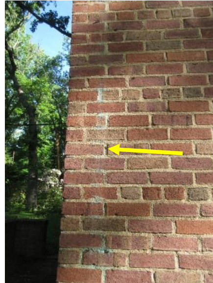
Figure 36. Abandoned fasteners from downspout connections.
