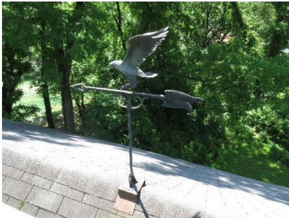
Figure 360. Metal weather vane on ridge of roof.
