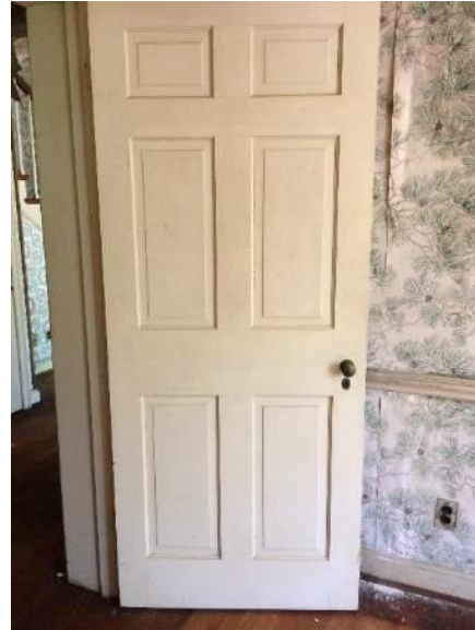
Figure 170. Six -paneled door between hallway and dining room. Door is wider than typical door in home.
