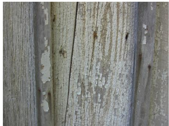
Figure 369. Typical deteriorated coating on exterior of barn.
