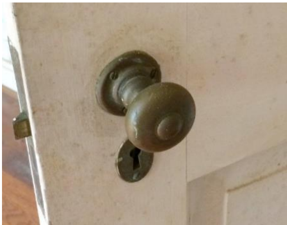
Figure 171. Typical metal door knob and metal key escutcheon.
