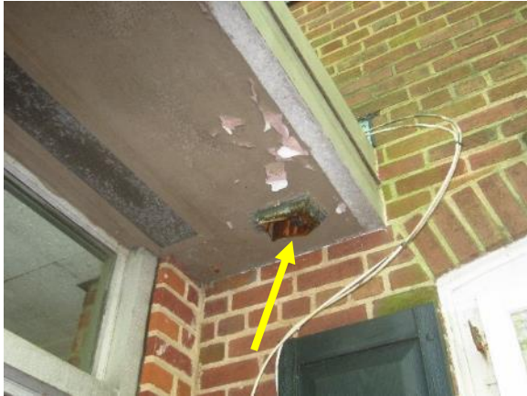
Figure 39. Downspout has been detached from location of previous drainage.
