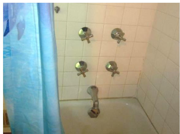
Figure 264. Silver metal faucets located in Bathroom A shower.
