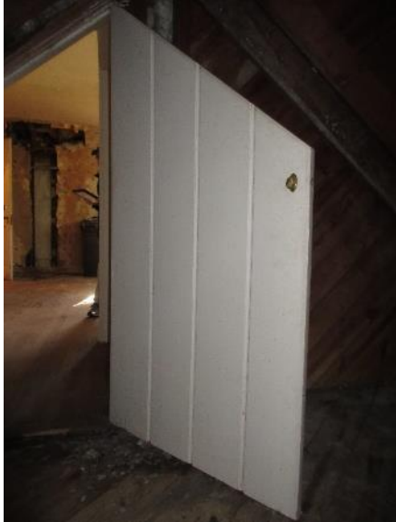
Figure 279. Door to storage room.
