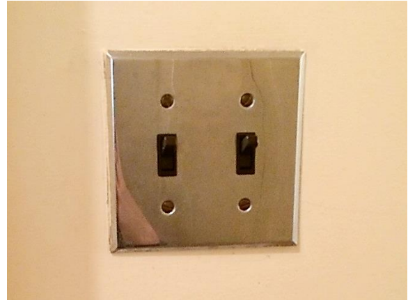
Figure 216. Typical metal switch plate.
