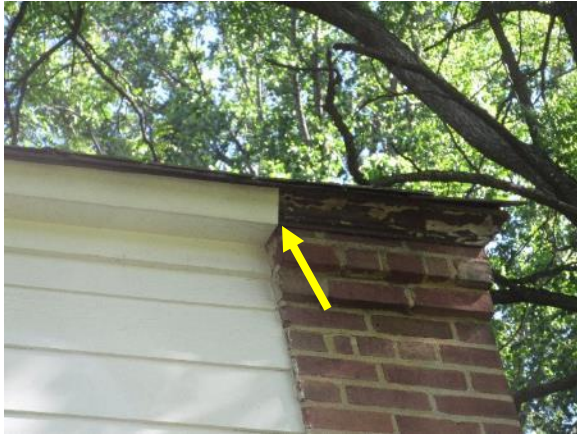
Figure 121. New trim covering old trim (north elevation).
