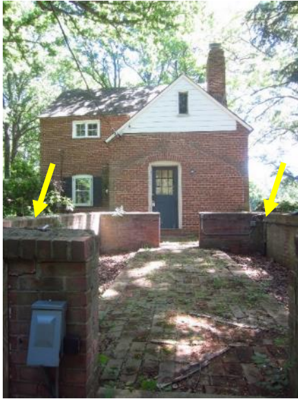
Figure 21. West wing and remains of previous greenhouse.
