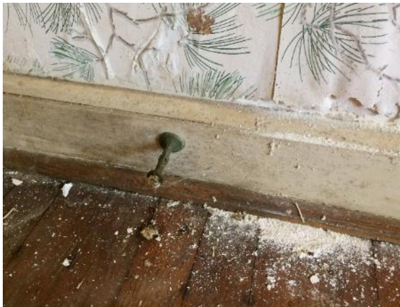
Figure 175. Baseboard in dining room. Baseboard profile is typical for all other baseboards in the home.
