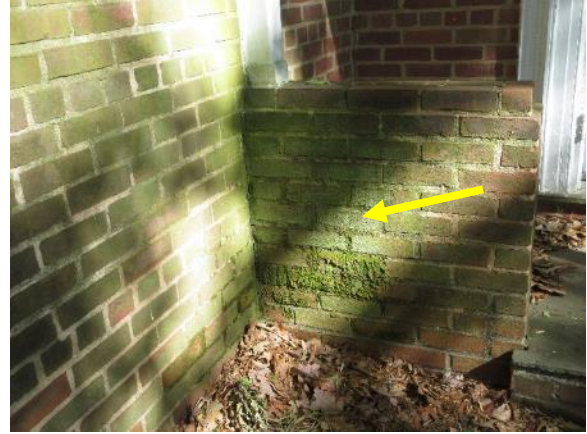
Figure 92. Biological growth and staining of brick at entryway corner.
