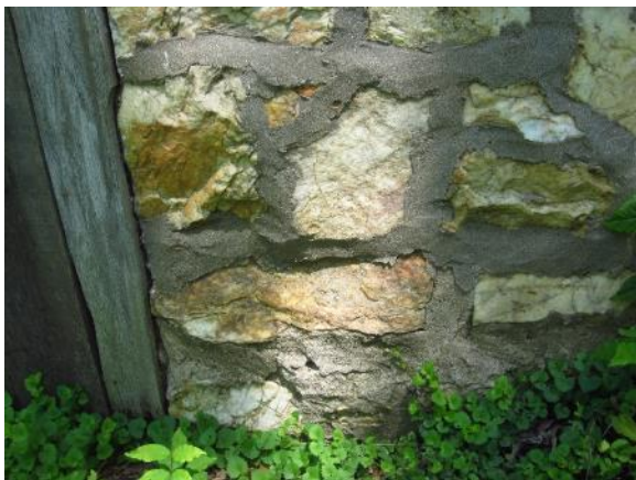
Figure 368. Mortar in fair condition on south side.
