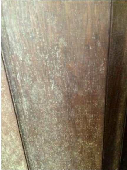
Figure 314. Potential microbial growth on surface of wood paneling in living room.
