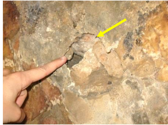
Figure 412. Typical debonded and weak mortar on stone foundation walls in basement.
