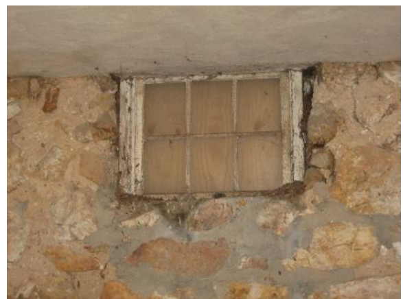
Figure 351. Typical fixed six lite window located in basement of barn.
