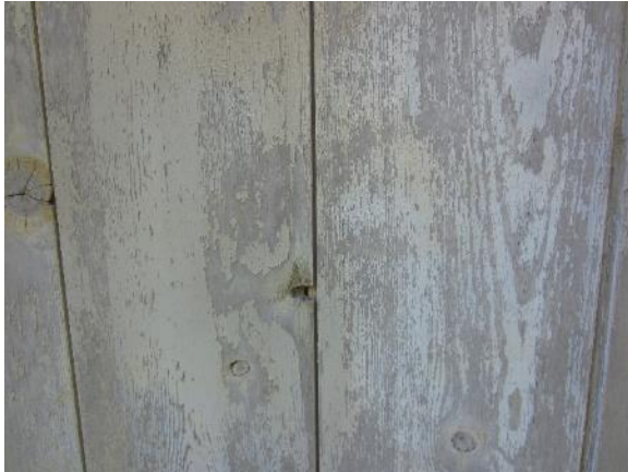
Figure 384. Typical coating deterioration of sliding door.
