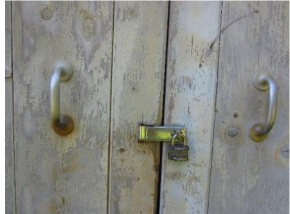
Figure 353. Silver metal handles and padlock at center of sliding barn doors on north side.
