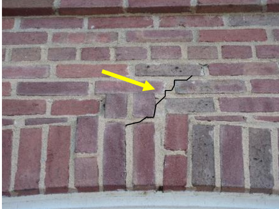
Figure 79. Stepped cracks in mortar above segmental arch. Crack traced for clarity.
