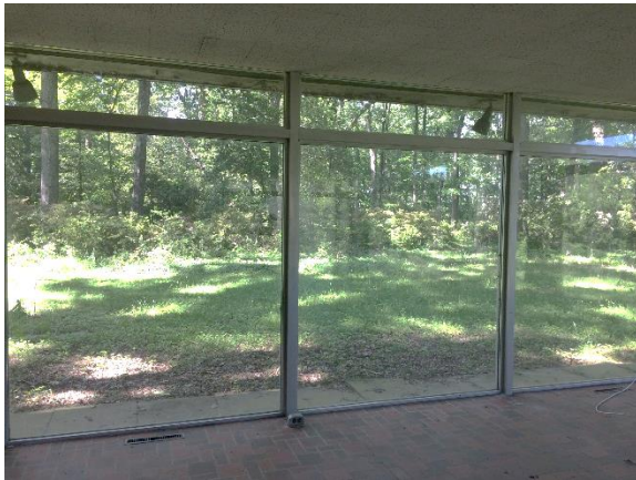
Figure 235. Typical storefront windows at glass porch, looking north.
