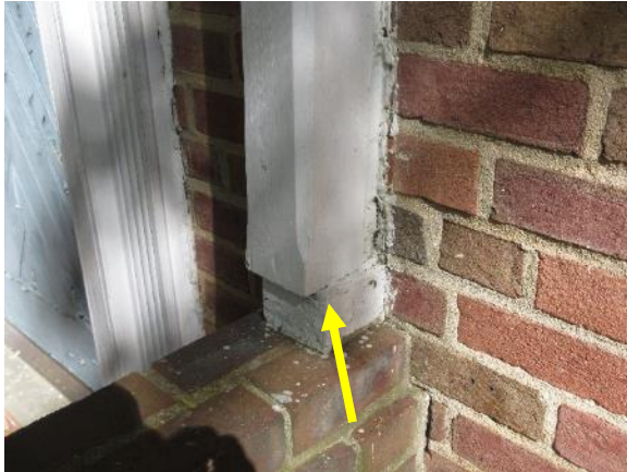
Figure 97. Undersized wood block under wood post at front entryway.
