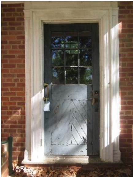
Figure 65. Front door of home, located on south facade under front entryway.
