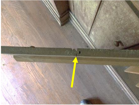
Figure 227. Detail view of tongue-and-groove construction of built-in cabinet doors, adjacent to fireplace in living room.
