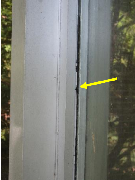
Figure 129. Typical deteriorated sealant at interface between IGU and aluminum framing at glass porch storefront.
