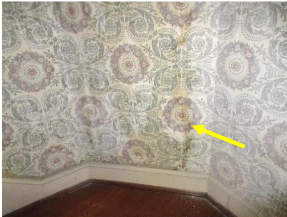
Figure 308. Stained wallpaper as evidence of water infiltration in the main stairwell between the first floor and the second floor.
