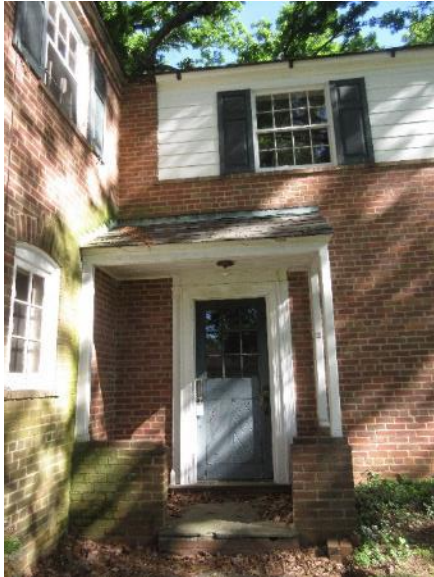
Figure 27. Front entryway on the south facade.
