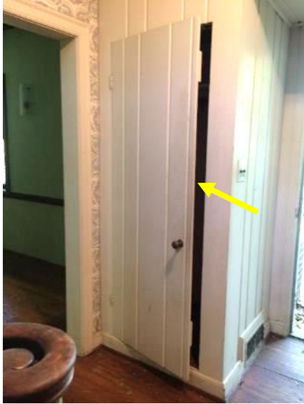
Figure 161. Foyer closet door with wood paneling to match south wall.
