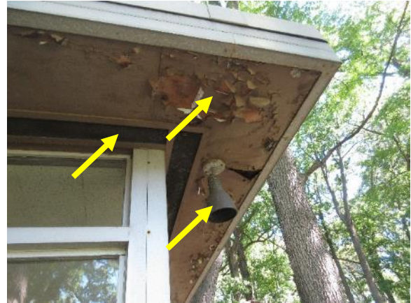
Figure 40. Glass porch soffit with 1/2 inch plywood and aluminum bird screen. Note aluminum light fixture on the corner.
