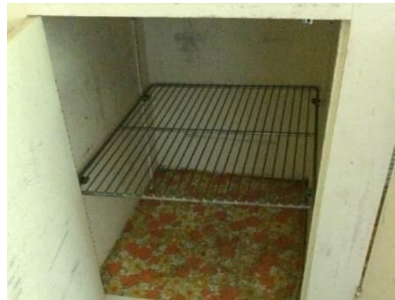
Figure 192. Metal racks are used in lieu of wood shelves in some of the original cabinets.
