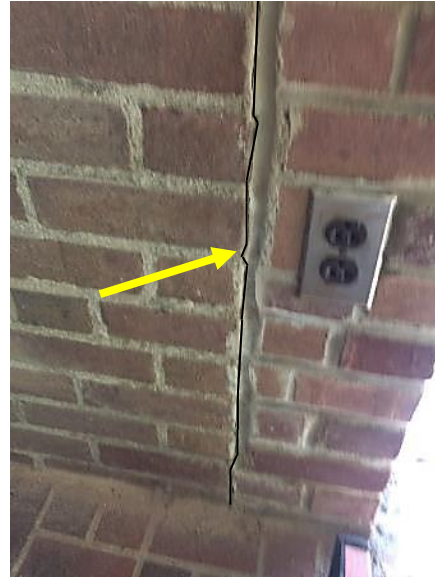
Figure 335. Bondline failure at interface between original brick facade and glass porch addition. Crack traced for clarity.
