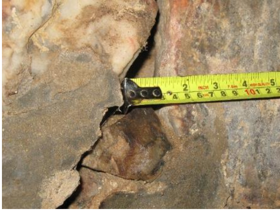
Figure 413. Displaced stone foundation walls and cracked mortar in northeast corner of basement.
