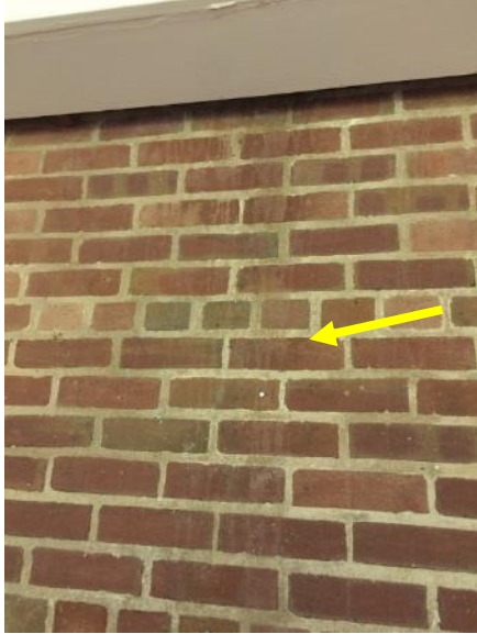
Figure 306. Streaking on brick in glass porch.
