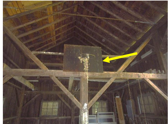
Figure 401. Basketball hoop installed over center post on west half of barn.
