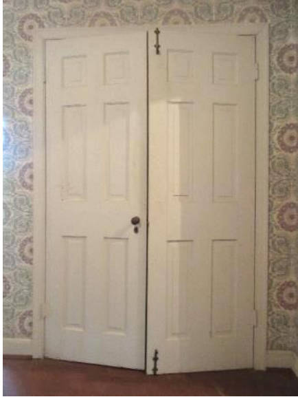
Figure 245. Six (6)-paneled closet French doors at second floor landing.
