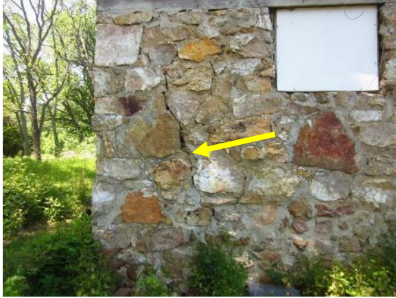
Figure 364. Multiple cracks and missing mortar in mortar of stone foundation at east end.
