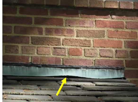
Figure 106. Warped copper flashing at front entryway roof.
