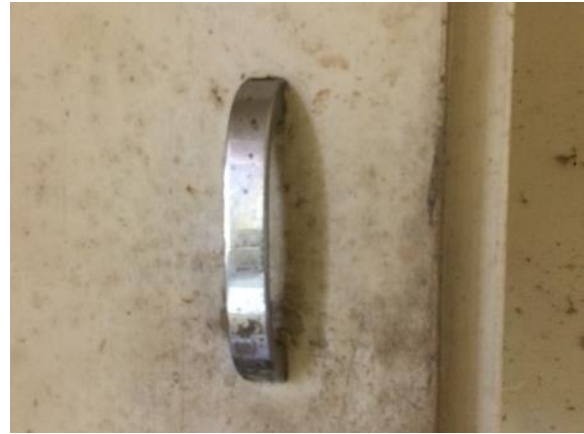
Figure 190. Original metal handles for lower cabinets and drawers in kitchen.
