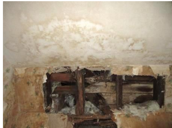
Figure 297. Missing and deteriorated plaster in Bedroom C revealing soft stud framing members.
