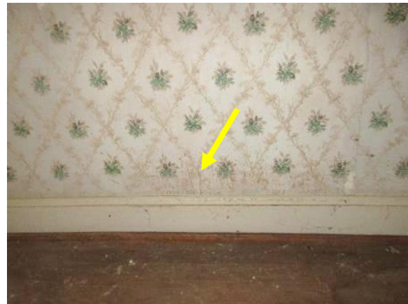
Figure 323. Scraped baseboard and wallpaper in Bedroom C.
