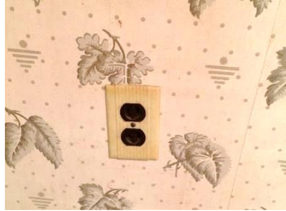
Figure 204. Typical white outlet plate. These were observed at isolated locations throughout the house.
