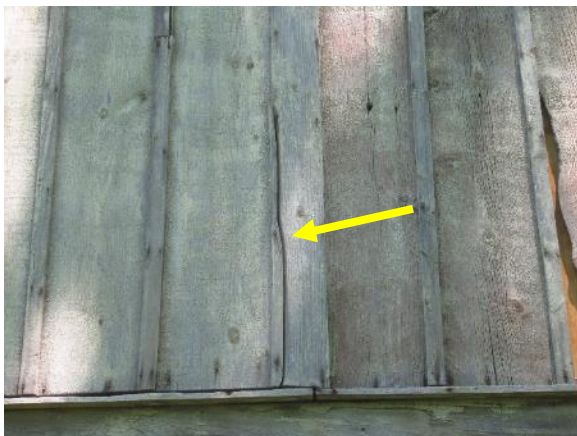
Figure 372. Split batten on south side.
