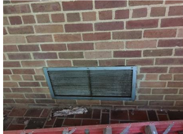
Figure 242. Large register located on interior south wall of glass porch, adjacent to the French doors that lead to the living room.
