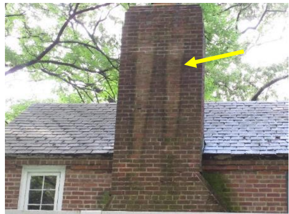
Figure 90. Surface staining of brick due to water runoff from chimney cap.
