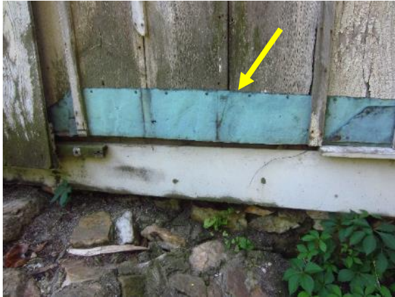
Figure 340. Copper sheet metal located on bottom of north side.
