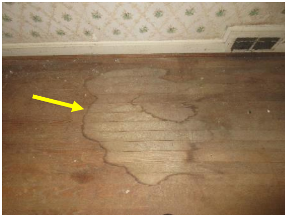
Figure 326. Water stain on wood floor in Bedroom C, not related to locations of exterior water infiltration.
