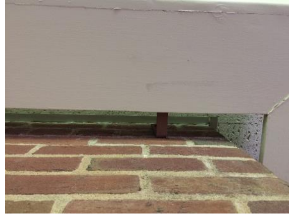
Figure 238. View of underside of white "lighting cove" that is installed on the perimeter of the brick face in the glass porch.
