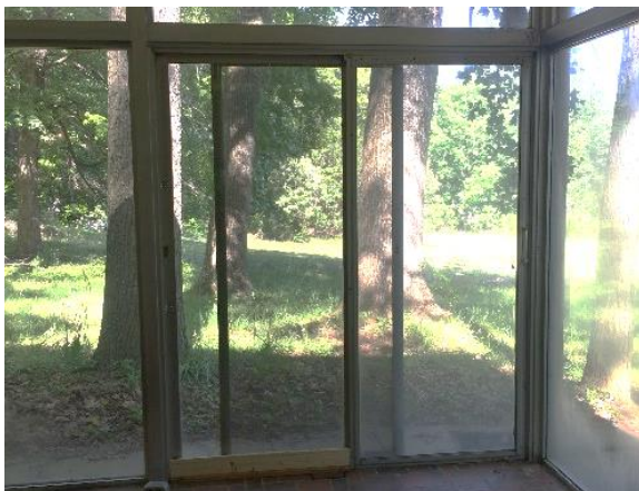
Figure 231. Sliding glass doors located on the east side of the glass porch.
