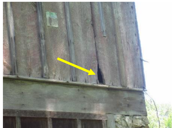
Figure 373. Hole in side of barn on south side.
