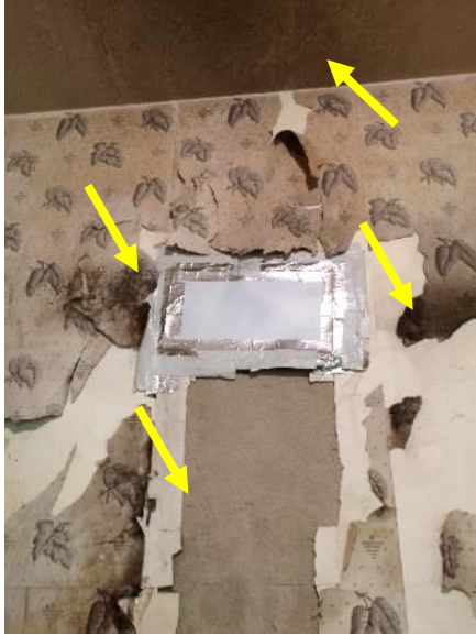
Figure 320. Dark surface staining and peeling/missing wallpaper and plaster around missing vent in Bedroom D.
