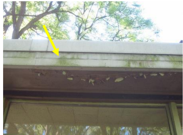
Figure 118. Typical biological growth along gutter of glass porch.
