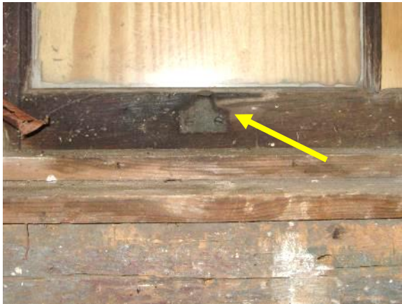
Figure 348. Metal pull located on interior of bottom rail at typical main level barn windows.
