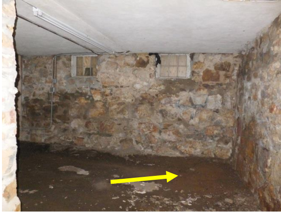
Figure 409. Standing water in the basement of the barn at the northwest corner during a rain event.
