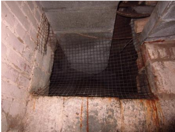
Figure 157. Hole through east CMU wall to allow air duct to reach the upper floors.
