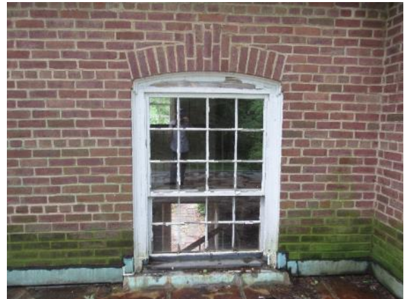
Figure 62. 12/8 double hung window at north facade above glass porch roof.
