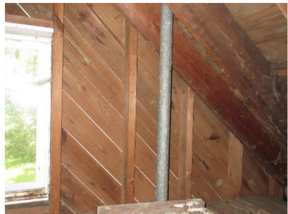
Figure 292. Diagonally-oriented wood boards at north gable end.
