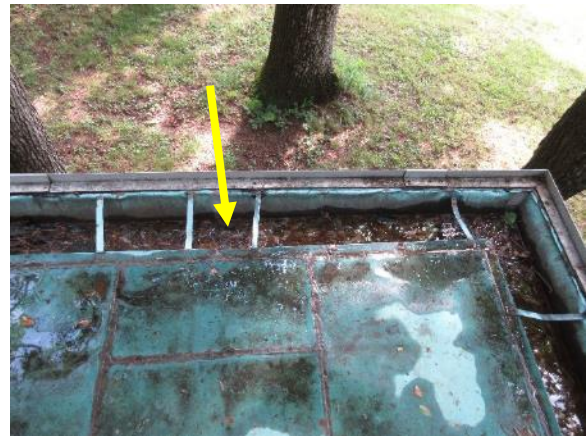
Figure 38. Metal-lined gutter with copper straps and aluminum edge metal.
