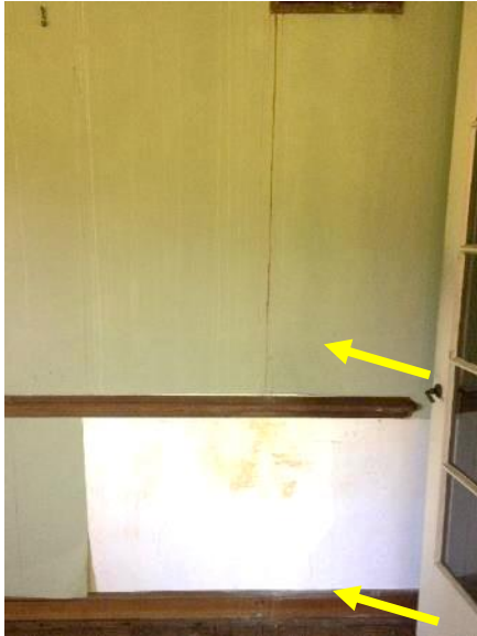
Figure 310. Streaked surface staining and missing wallpaper (living room).
