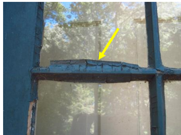
Figure 136. Typical cracked glazing putty at exterior doors.
