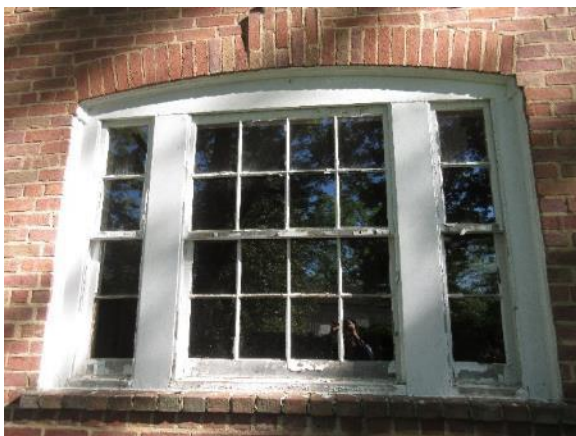
Figure 59. Double hung window assembly on south facade.
