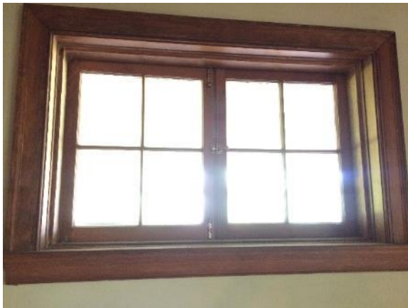
Figure 229. View of paired casement windows on east wall of living room.
