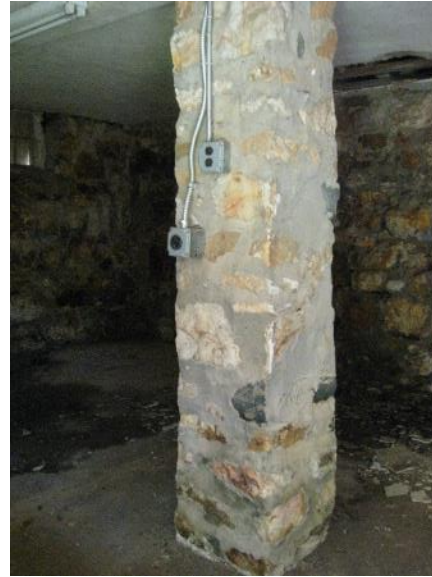
Figure 407. Stone column in basement. Repointing mortar and stone appear to match the south basement wall.
