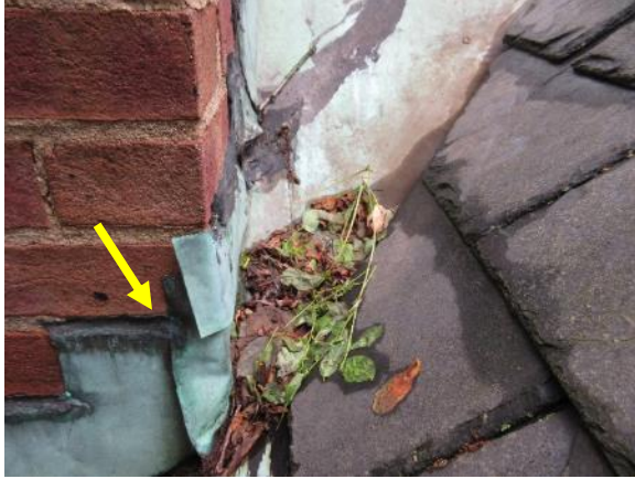
Figure 109. Copper flashing at north chimney. Note the mastic repairs and detached edges.
