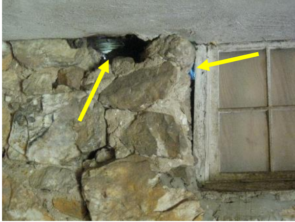
Figure 382. Void between window frame and stone and gap between stone and ceiling.
