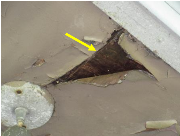
Figure 99. Glass porch soffit sagging from water infiltration.
