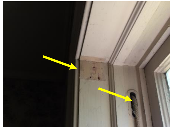
Figure 48. Typical abandoned anchor holes associated with previously installed window treatments. Note rope lifting hardware for double hung sash.
