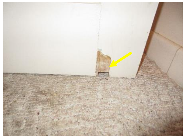
Figure 333. Chip at bottom of door to Bathroom B.
