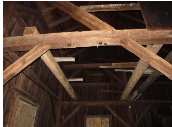
Figure 397. View of western portion of barn, showing the miscellaneous wood beams that sit on top of the tie beams.
