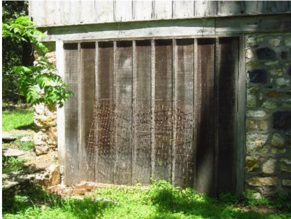
Figure 358. Opening on left side of south barn door that has been infilled with wood.
