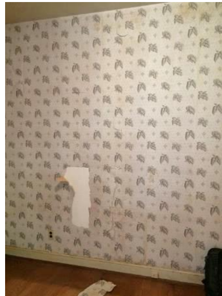
Figure 196. View of typical finishes on east wall in Bedroom D.
