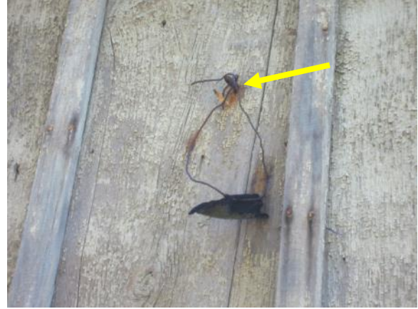
Figure 377. Typical metal hooks in wood boards.
