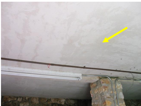
Figure 417. View of plaster ceiling in basement. Note the minor staining on the surface.
