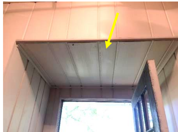
Figure 160. View of the lowered ceiling at the entryway to the foyer.
