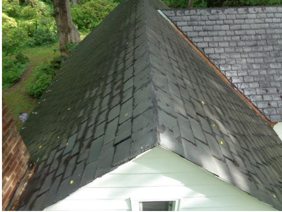
Figure 31. View of gable roof over center core of home and gable roof over east wing that intersects the center core.
