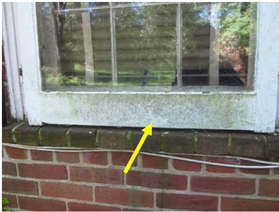
Figure 133. Typical biological growth on storm window and adjacent brick sill.
