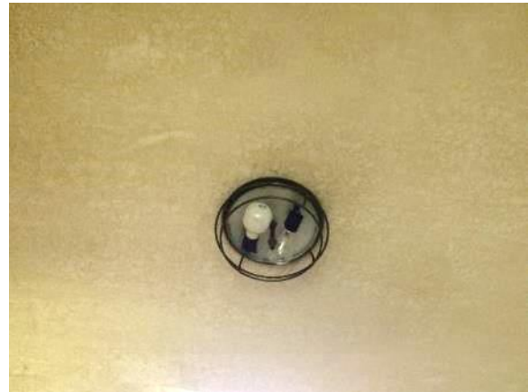
Figure 164. Circular light fixture in foyer with metal base and missing globe.
