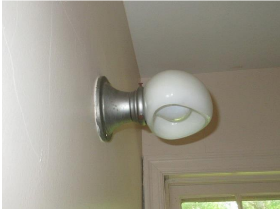
Figure 215. Original light fixture above sink. Typical for all bathrooms.
