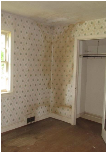
Figure 304. Water staining at plaster and wallpaper in southwest corner of Bedroom C.
