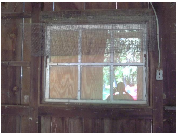
Figure 350. Center window on south wall of barn.
