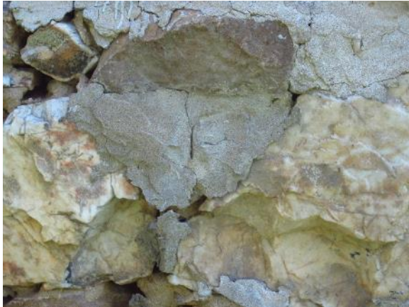
Figure 366. Typical debonded and cracked mortar of foundation walls.
