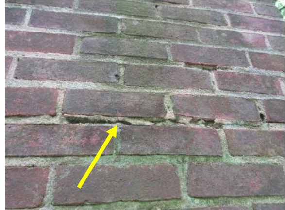
Figure 82. Missing and cracked mortar at chimney on north facade.
