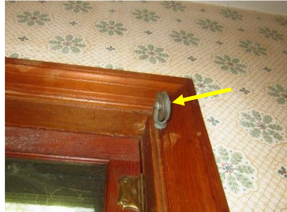
Figure 52. Pulley from previous window treatment attached to top corner of east window in Bedroom A.
