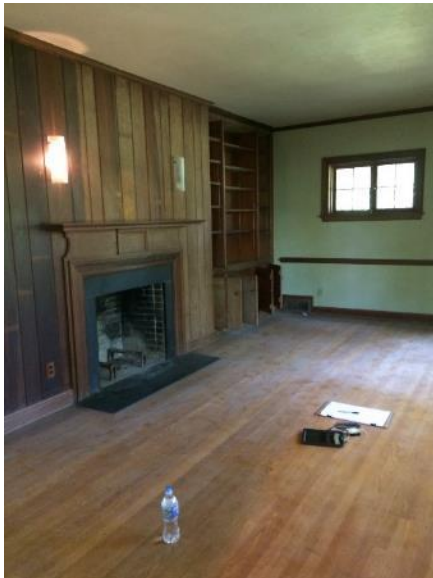
Figure 217. View of typical finishes in the living room, looking northeast.
