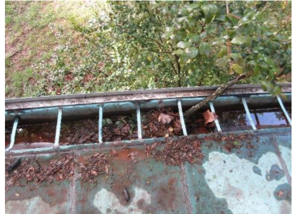
Figure 116. Glass porch gutters blocked with debris.
