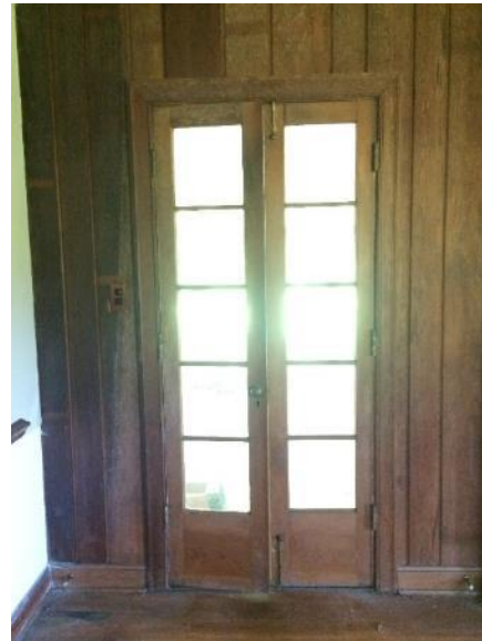
Figure 218. French doors from living room to glass porch, looking north.
