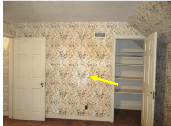
Figure 311. South wall of Bedroom B. Note typical discoloration of wallpaper. The door to the hallway is located on the left.
