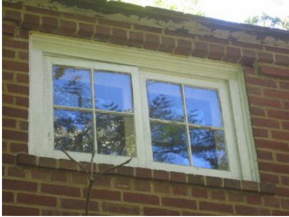
Figure 45. Paired casement window with four lites of glass in each sash, located on the second floor of the west facade.
