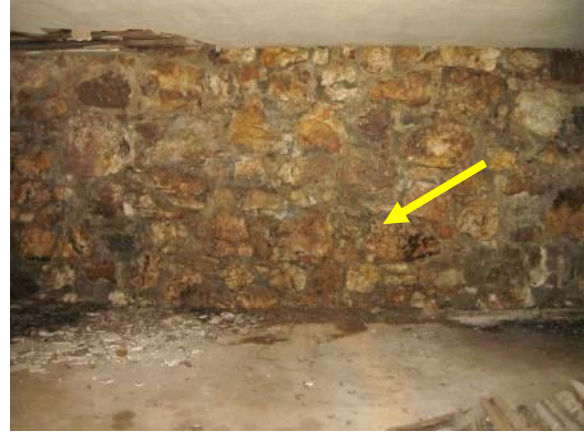
Figure 410. Moisture staining on stone foundation walls in basement.
