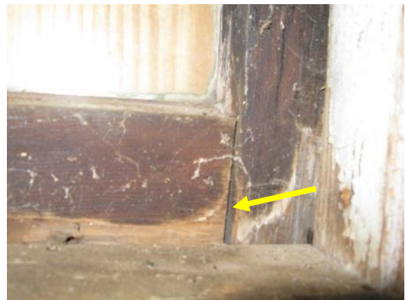
Figure 381. Typical separation between rail and stile at interior window. Note staining.
