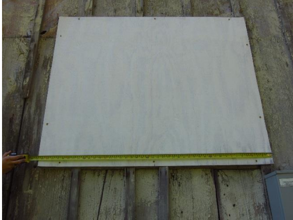
Figure 346. Typical white painted plywood covering awning windows.
