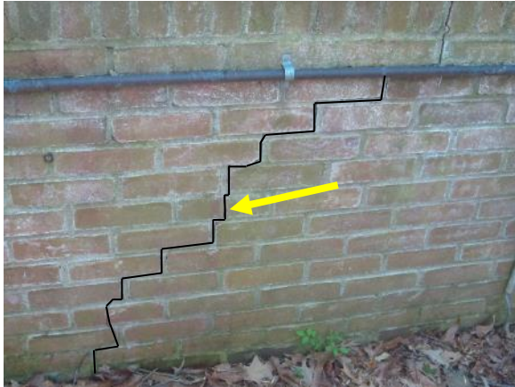
Figure 85. Crack pattern through mortar and brick on greenhouse wall. Crack traced for clarity.
