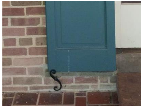
Figure 232. Original shutters with original shutter dogs framing the French Doors.
