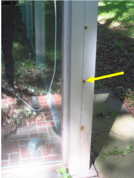
Figure 131. Typical corroding fasteners at glass porch window frame.
