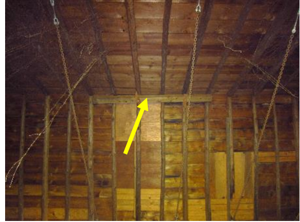
Figure 420. Partial ridge beam nailed in place.
