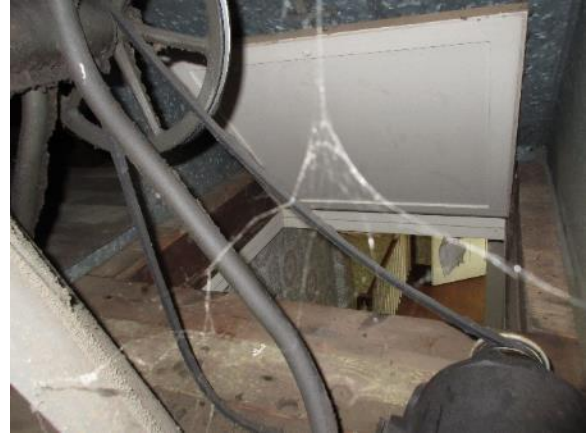
Figure 284. Attic hatch as viewed from attic through house fan.
