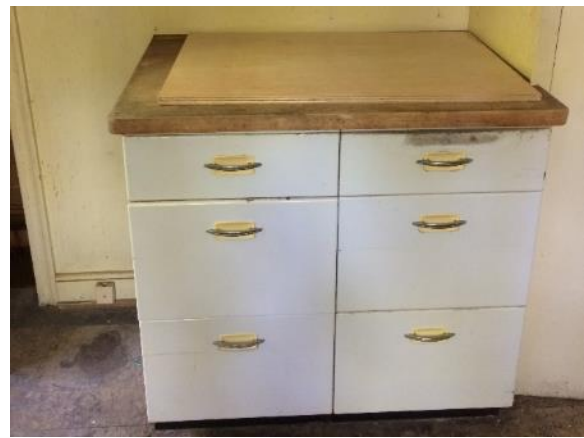
Figure 188. Lower replacement metal cabinets and drawers on north wall.
