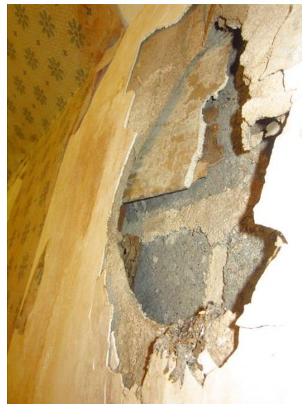
Figure 301. CMU chimney wall and layers of plaster at water damage in Bedroom A.
