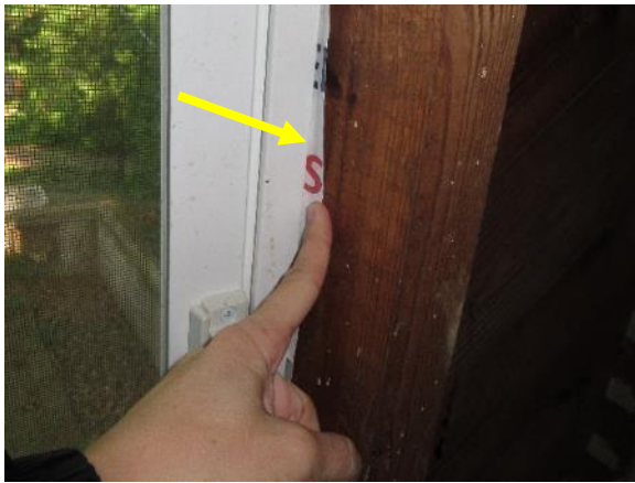
Figure 57. Contemporary weather-resistive barrier can be seen around frame of storage room window.
