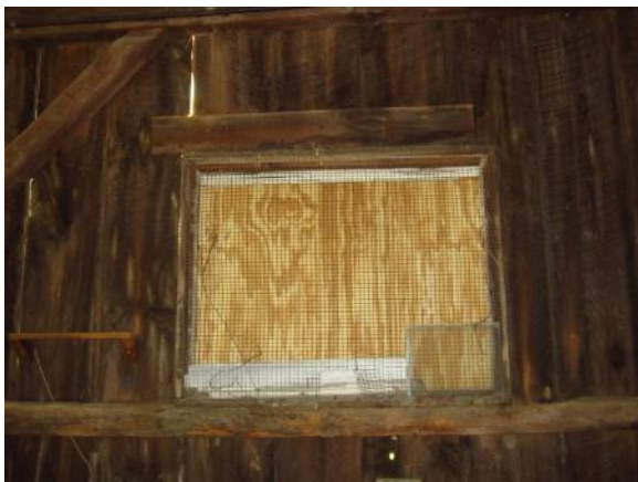
Figure 380. Missing window sash with several window components stacked between plywood and screen.
