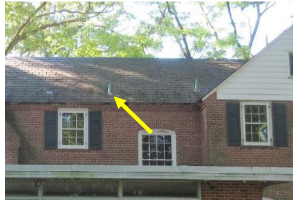
Figure 309. Pipe that penetrates roof above main staircase. This is a potential cause of water infiltration at this location.
