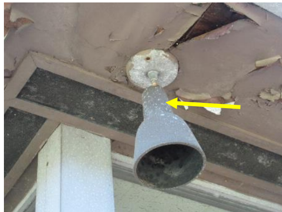
Figure 138. Typical oxidation of exterior glass porch light fixtures.
