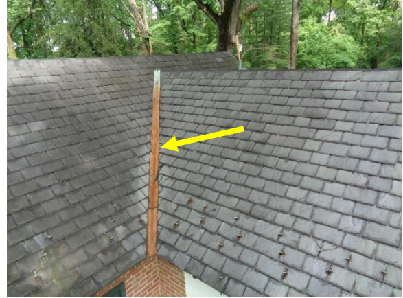
Figure 32. Open valley with copper flashing between core north-south gable and east wing.
