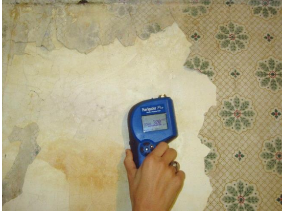
Figure 302. High moisture content detected by the moisture meter (300 out of 300).
