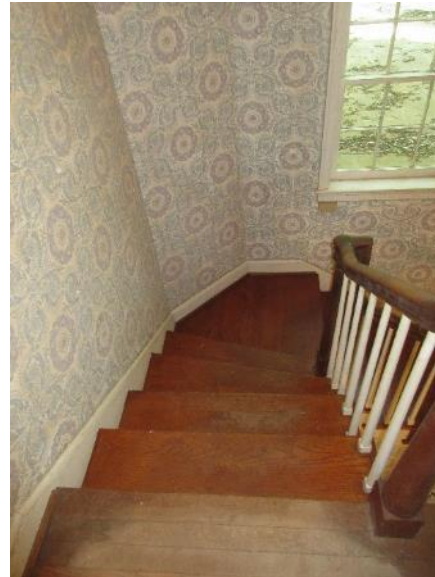
Figure 140. View of the main staircase from the second floor.
