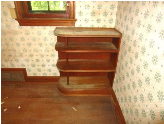
Figure 255. Built-in shelves at northeast and southeast corners of Bedroom A.
