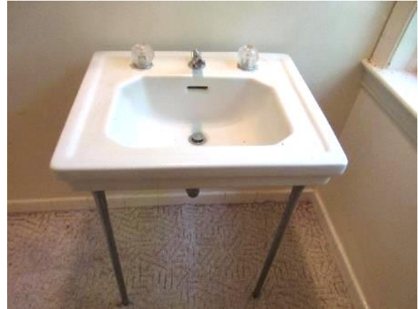
Figure 270. Porcelain console sink in Bathroom B. Note plastic replacement knobs for temperature control.
