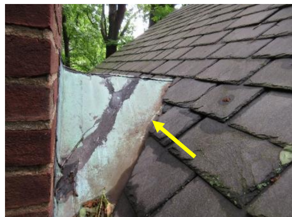
Figure 108. Copper cricket behind north chimney with mastic repairs.
