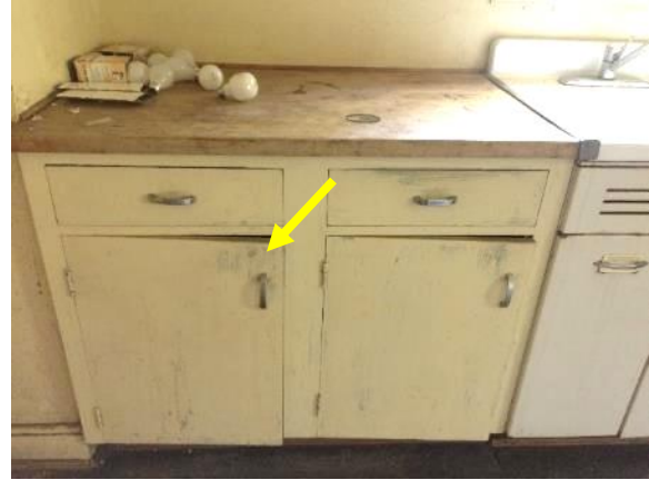
Figure 321. Paint scraped at cabinets in kitchen.
