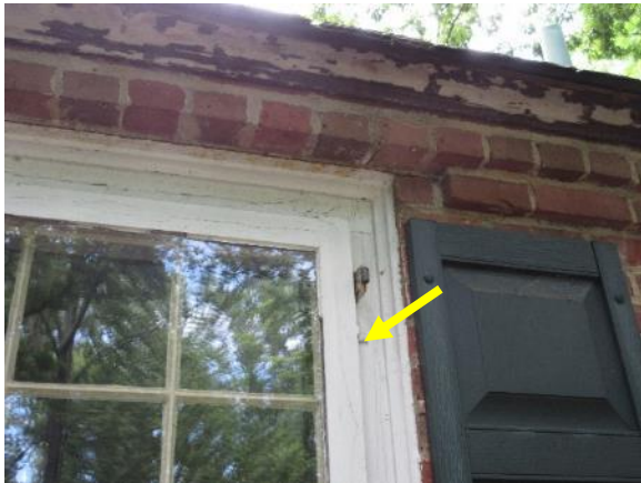
Figure 61. Storm window and typical "L" brackets (north facade).
