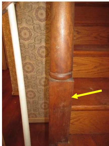
Figure 144. Typical base of newel posts on main staircase.
