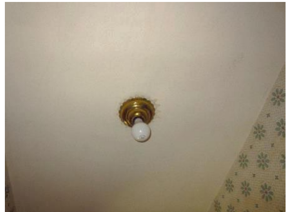
Figure 252. Light fixture with gold base and missing glass globe located in walk through closet to Bedroom A.
