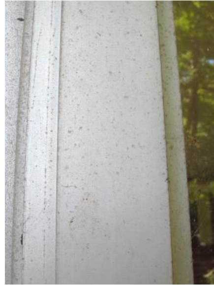
Figure 130. Typical oxidation of glass porch window frame.
