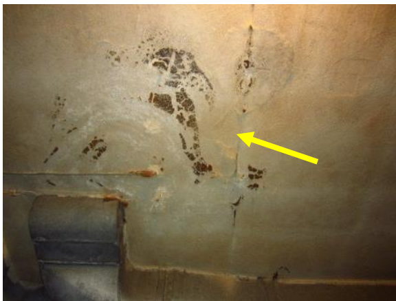
Figure 316. Potential microbial growth on plaster ceiling in basement.
