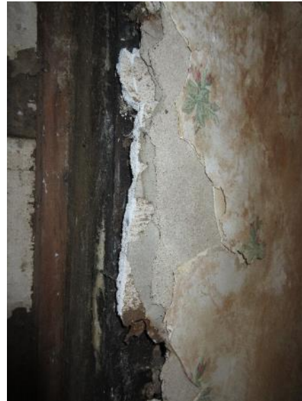
Figure 278. View of plaster layers at an existing hole in the wall.
