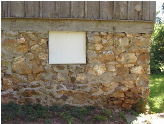
Figure 342. Typical fieldstone with tan mortar used for barn foundations.
