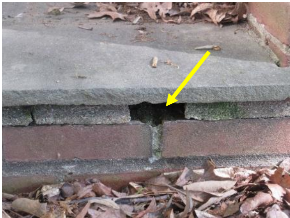
Figure 95. Setting mortar missing from underneath stone paver on front entryway.
