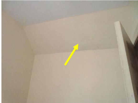
Figure 269. Northeast corner of Bathroom B. Note the sloped wall and painted white walls and ceilings.
