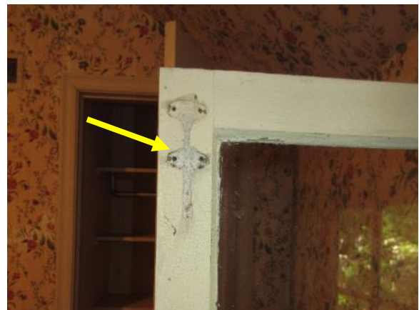
Figure 50. Missing sliding locks on interior storm windows of west window in Bedroom B.
