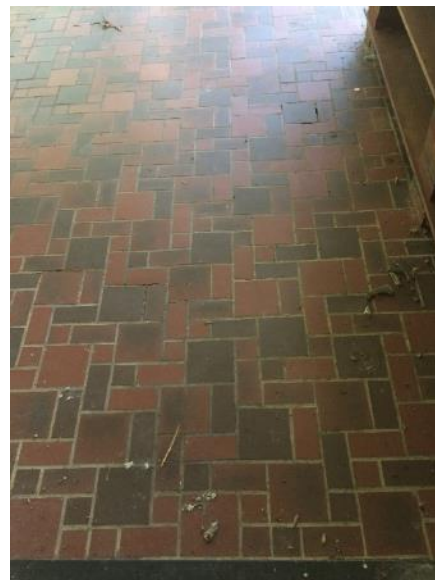
Figure 240. Brick pavers make up the flooring of the glass porch.
