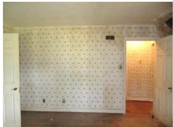
Figure 274. Typical finishes in Bedroom C, looking north.
