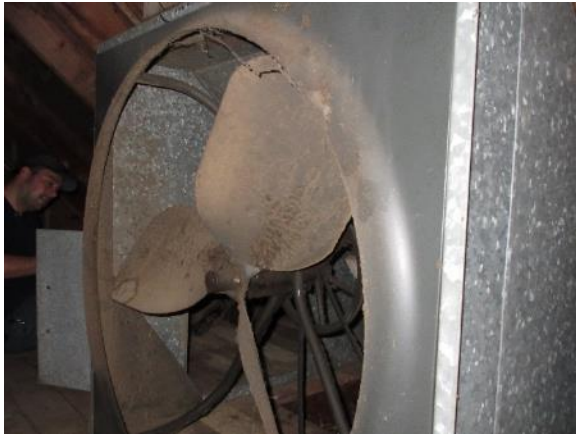
Figure 285. House fan located in metal duct over attic hatch.
