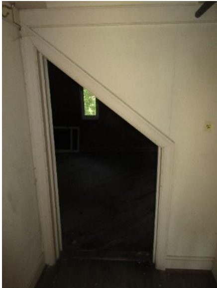
Figure 277. Angled doorframe to storage room through northwest closet of Bedroom C.
