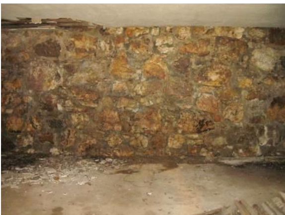
Figure 404. Typical fieldstone foundation walls and concrete floor in barn basement.
