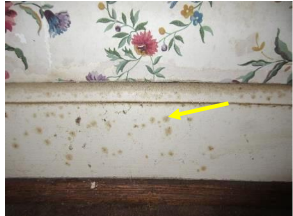
Figure 315. Typical potential microbial growth on baseboard.
