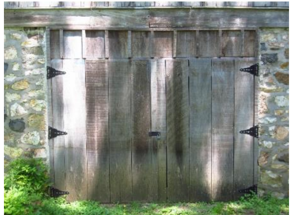
Figure 355. Hinged double doors on south side.
