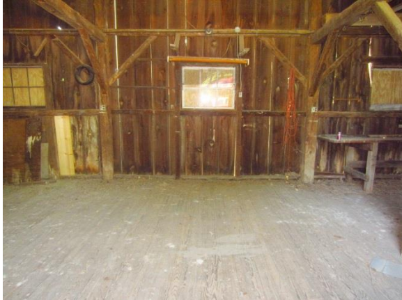
Figure 390. Interior view of south barn wall with exposed heavy timber framing.
