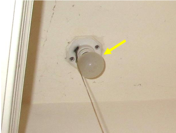
Figure 197. Typical bulb with pull chain located in closets throughout the home.
