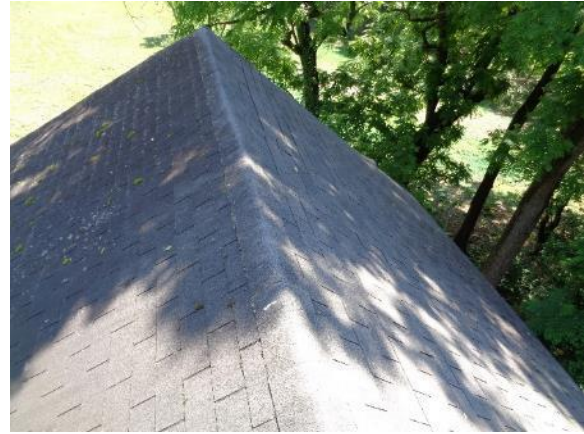
Figure 359. View of barn roof, comprised of asphalt shingles.
