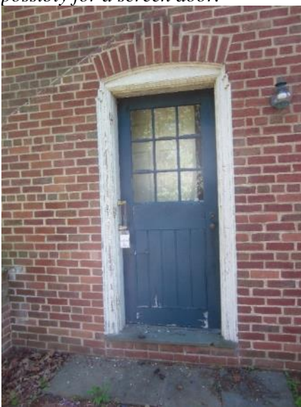
Figure 71. Exterior door on west facade.
