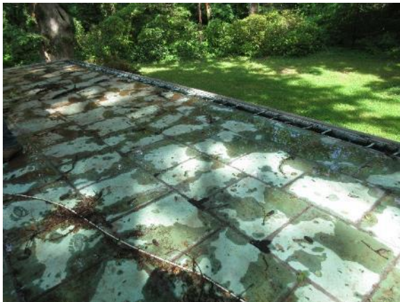
Figure 37. Copper flat-lock soldered seam roof located over the glass porch addition.
