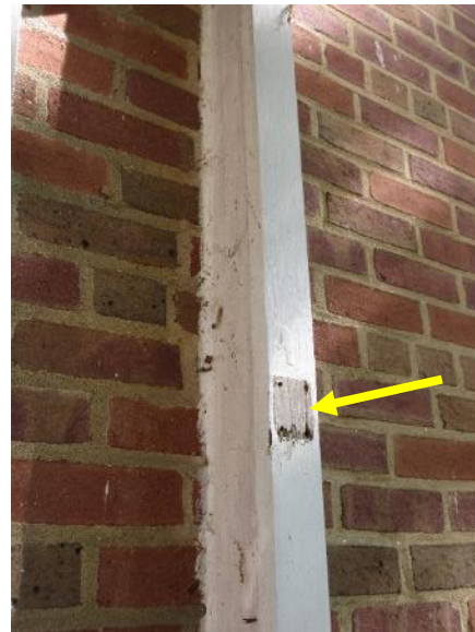
Figure 96. Typical holes in front porch wood post.
