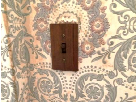
Figure 169. Typical wood switch plate.
