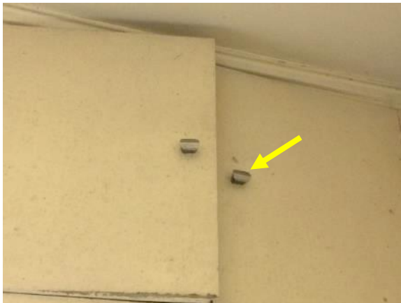
Figure 191. Original oval knobs for upper cabinetry in kitchen.
