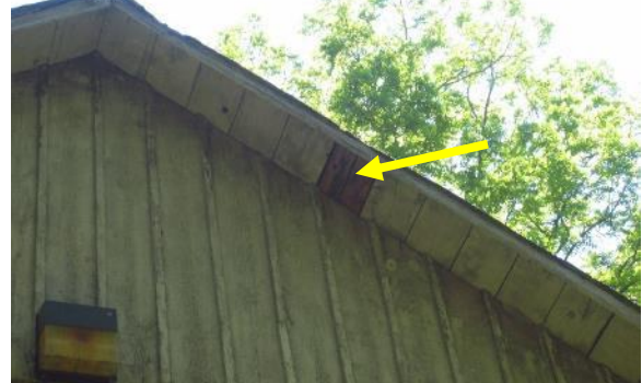
Figure 387. Replacement roof deck plank on west rake overhang.
