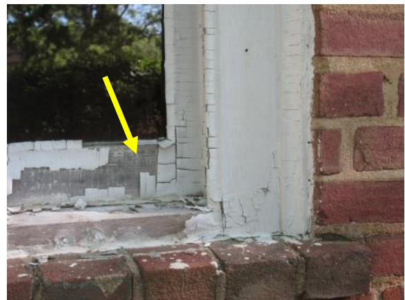
Figure 126. Typical cracked and peeling paint at exterior of window.
