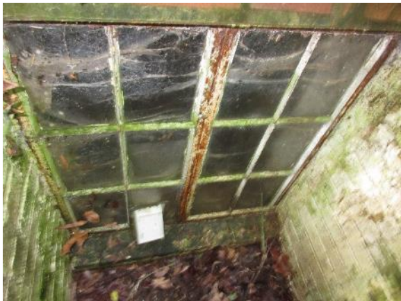
Figure 41. Typical paired casement basement window within a window well.
