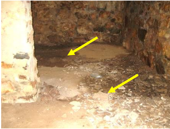
Figure 411. Moisture staining of concrete basement floors. Note plaster remnants on floor.
