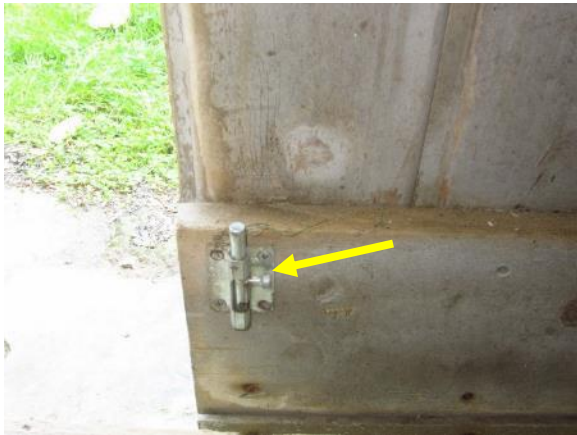
Figure 354. Metal sliding lock on east sliding barn door.
