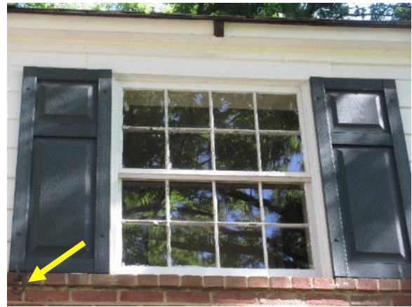
Figure 58. Typical 8/8 double hung window with fixed replacement shutters. Note abandoned shutter dog (yellow arrow).
