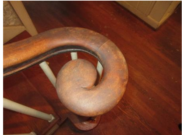
Figure 146. Railing detail at bottom of staircase, where handrail curls away from stairs.
