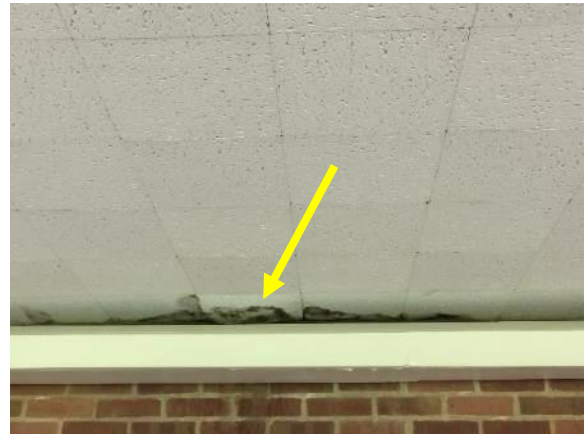
Figure 305. Water staining at acoustic ceiling tiles in glass porch.
