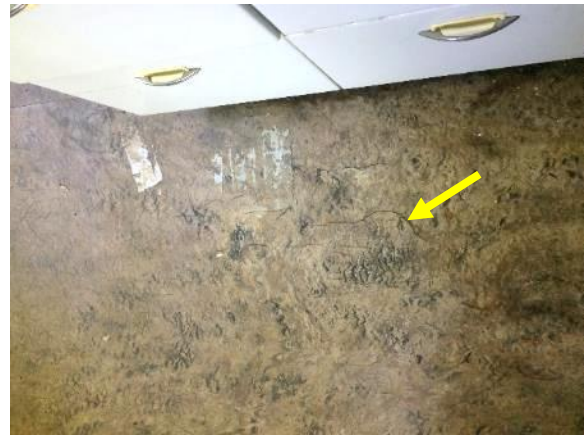
Figure 327. Cracked linoleum in the kitchen.
