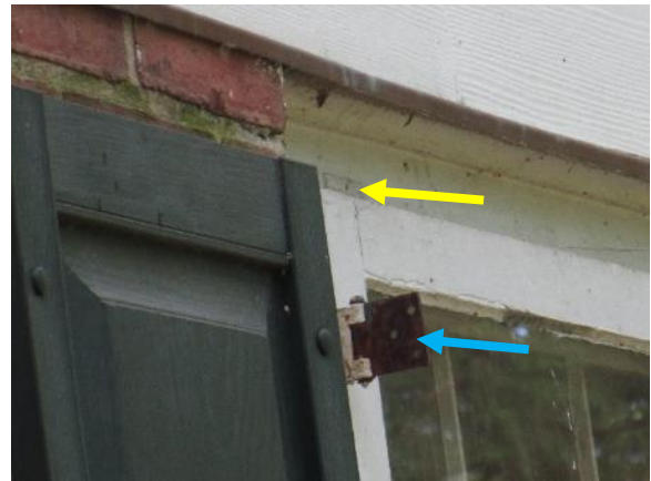
Figure 64. Exterior storm windows attached with hinges at the top of the frame. Abandoned hinge from original shutter (blue arrow).
