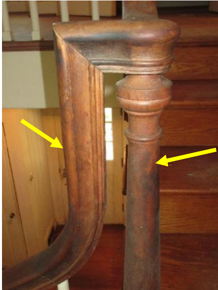
Figure 145. Typical top of newel posts and steep curve in handrail on main staircase.
