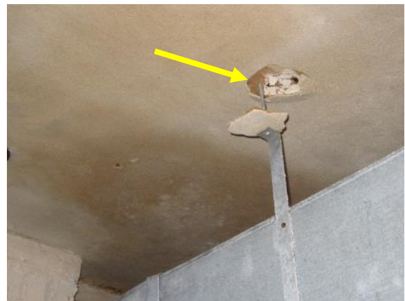
Figure 317. Hole in plaster ceiling of basement from detached ductwork anchorage.
