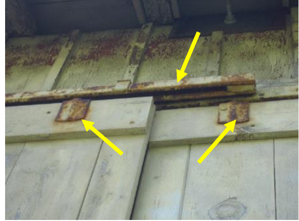
Figure 383. Rusted sliding door tracks and hardware
