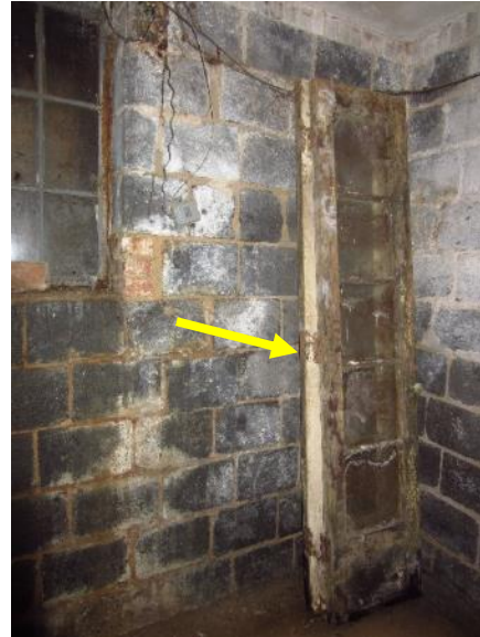
Figure 158. French doors stored in the basement.
