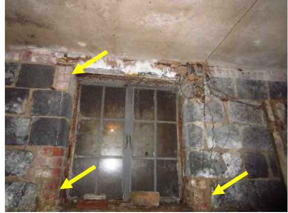
Figure 154. Window on west wall with brick at three corners of the window rough opening.
