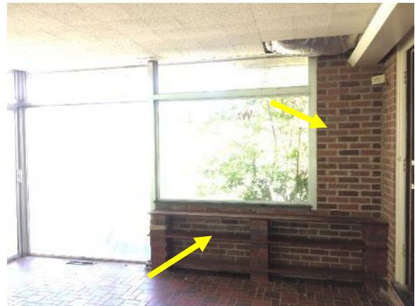
Figure 230. View of south wall of glass porch. Note the shelves adjacent to the storefront windows.
