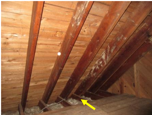
Figure 289. Roof rafters meet wood floor joists and insulation in attic.
