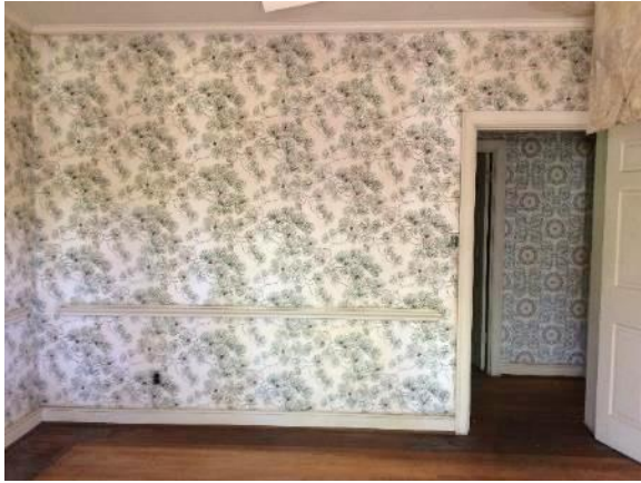
Figure 173. View of dining room, looking north. Note evergreen design wallpaper and typical painted chair rail, crown molding, and baseboards.
