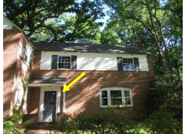
Figure 20. Front entryway at east wing of the home.
