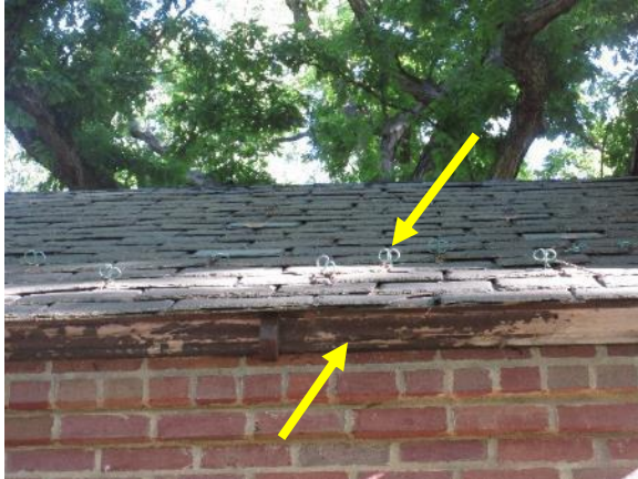
Figure 35. Side view of the slate roof. Note the copper snow guards on top of the roof and the wood trim below the roof.
