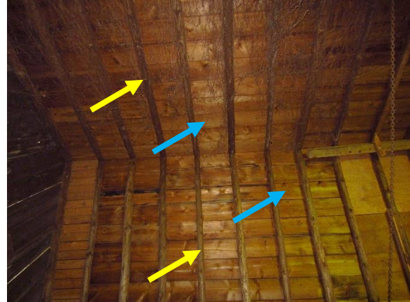
Figure 391. Interior view of barn roof structure. Note the wood rafters (yellow arrows) and wood sheathing (blue arrows). Note there is no continuous ridge beam.
