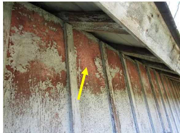
Figure 339. "Red" wood seen under eaves, indicating that the barn may have been stained red in the past.
