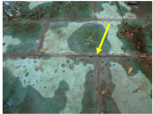
Figure 114. Cracked seams at expansion joint of copper roof over glass porch.
