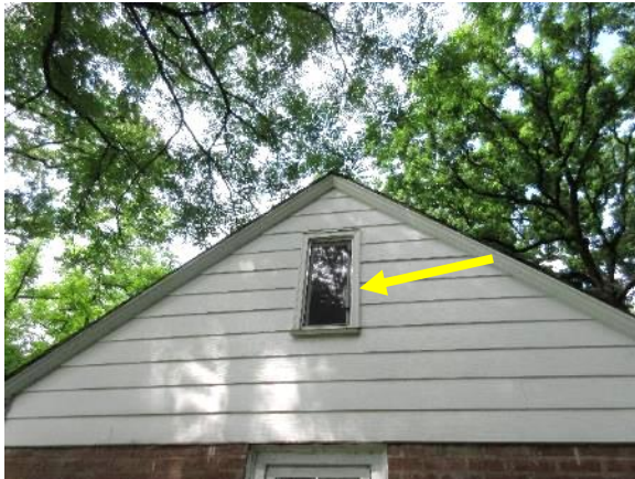
Figure 53. Typical replacement attic window.
