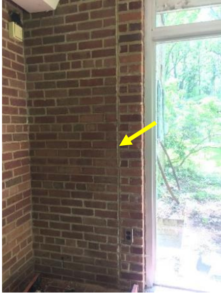
Figure 237. Southwest corner of glass porch. Note the vertical joint in the masonry between the original brick of the home and the brick added during construction of the glass porch.
