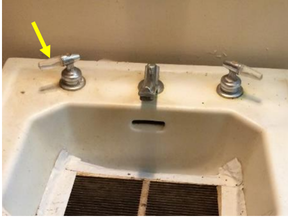
Figure 207. First floor bathroom sink details. Note the clear plastic tips on the ends of the flow and temperature controls.
