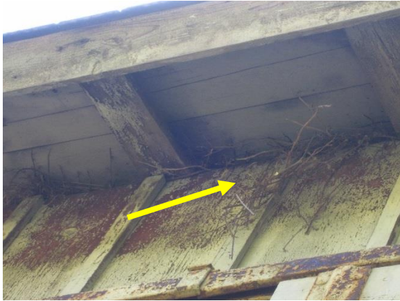
Figure 378. Vegetation growing from under roof on north side.
