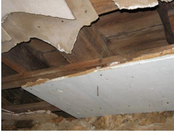
Figure 406. Hole in plaster ceiling of barn basement. The floor boards can be seen through the hole, as well as additional sawn lumber boards used as furring for the plaster.
