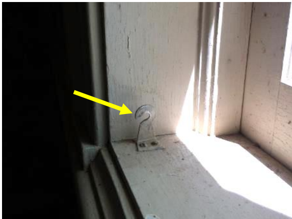
Figure 47. Typical abandoned hardware associated with previously installed window treatments.
