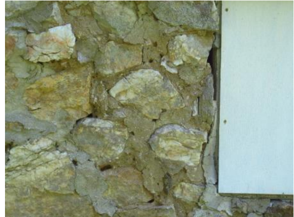
Figure 367. Typical debonded and missing mortar of foundation walls.
