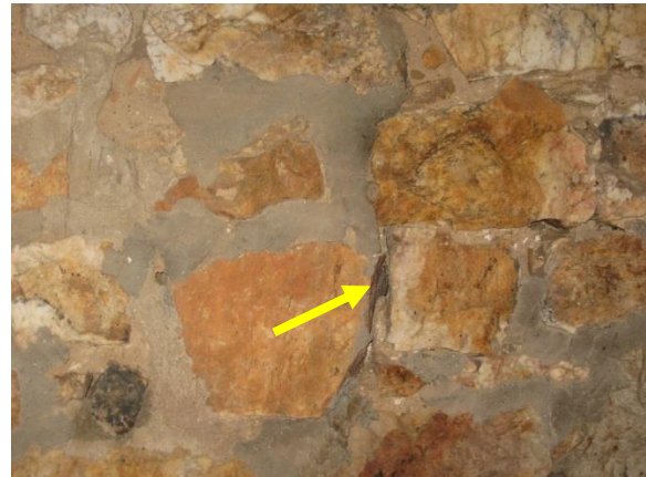
Figure 416. Typical debonded and missing mortar at interior surface of foundation walls.
