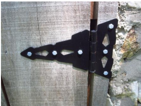
Figure 356. Detail view of metal hinges on south side.
