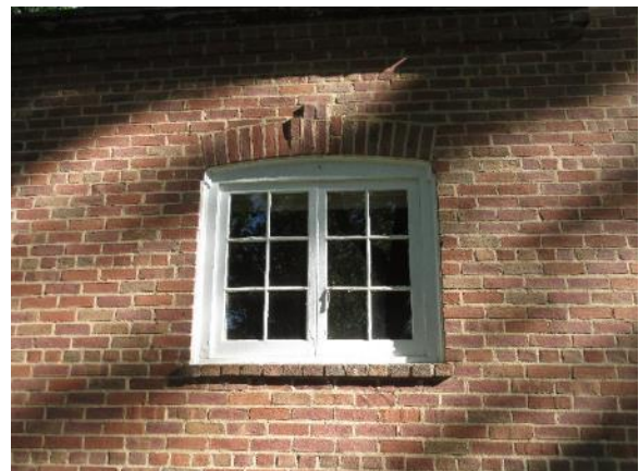
Figure 44. Paired casement window with six lites of glass in each sash at south facade.
