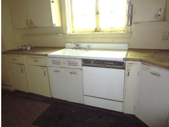
Figure 181. View of the kitchen south wall.
