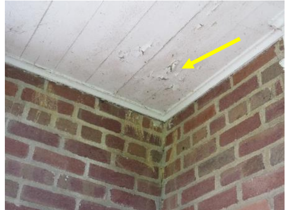
Figure 98. Typical cracked and peeling paint at front porch ceiling.
