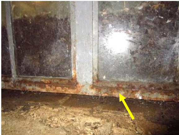
Figure 123. Corroded window casing and sash in basement.
