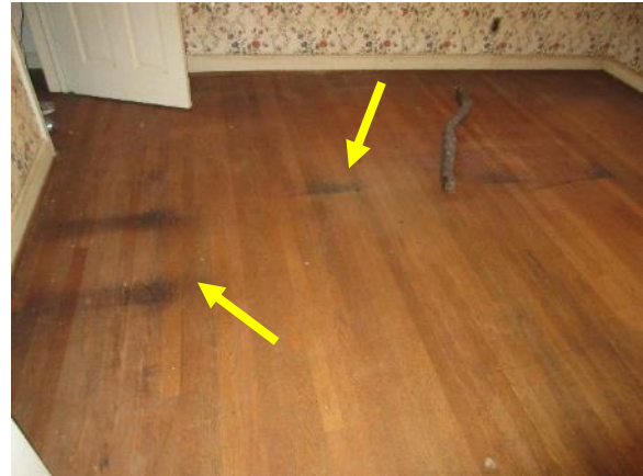
Figure 325. Dark marks on wood floor (Bedroom B).
