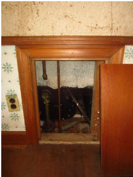
Figure 257. Access hatch for bathroom plumbing on west wall of Bedroom A.
