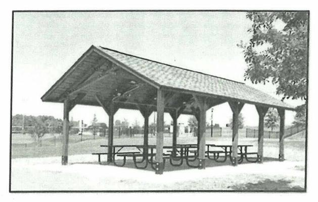
Please find the shelter and trail location in the attached Bowman Consulting site permit layout. See the RCP Shelters, Inc. rendering of the 24' x 24' custom scissor truss gable shelter with shingle roof with tables and accessible trails as recommended by the Planning & Development Division of FCPA.
