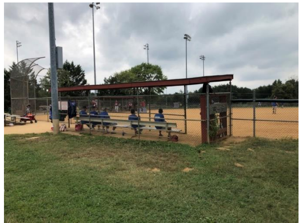
Figure 8: Braddock Park Dug Out Shelter
