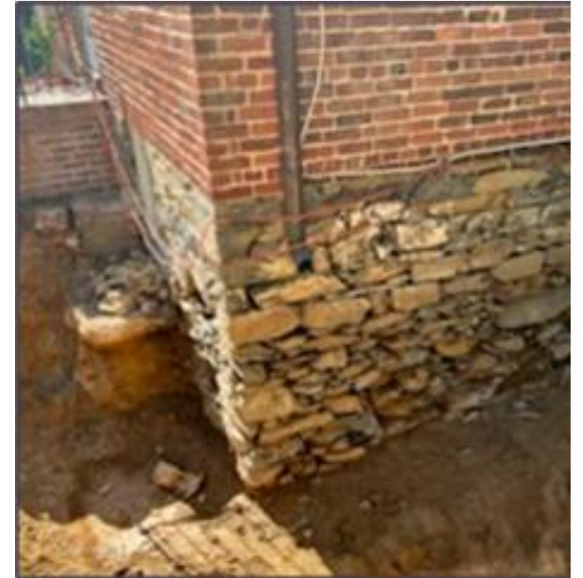
Lahey Lost Valley, Foundation Repairs
