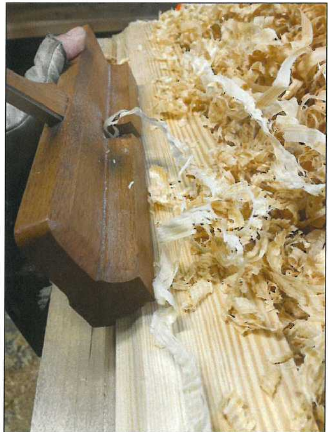
Running of moldings to match existing 18 th century examples in the Archives and in the Mansion.
