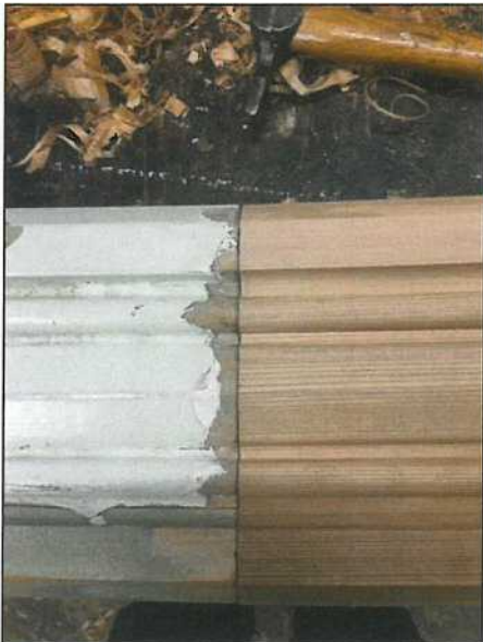
Existing molding on left. New run on the right
