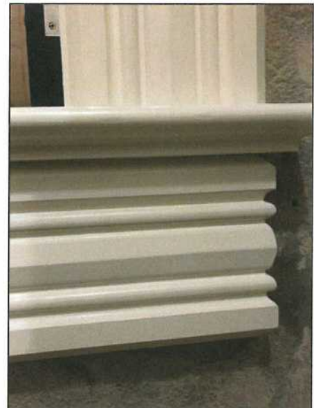
Molding installed in lighthouse.
