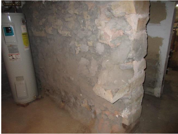
Figure 77. Deteriorated mortar and previous patch repairs at original stone foundation wall in cellar.
