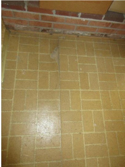
Figure 89. Delaminated and damaged linoleum flooring, typical.
