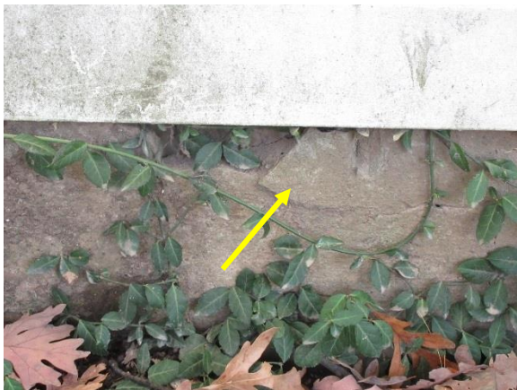
Figure 19. Typical crack and slight delamination in parge coat at original foundation.
