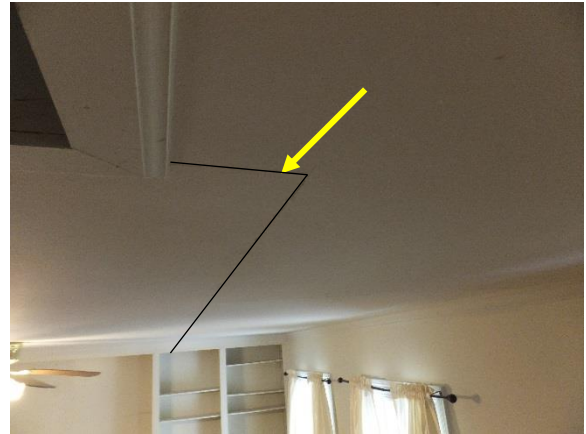
Figure 46. Cracking at ceiling (1st Floor) likely seams between drywall boards. Crack traced for clarity.
