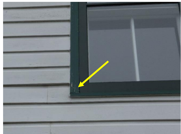
Figure 18. Flaked paint on window frame at southeast facade.
