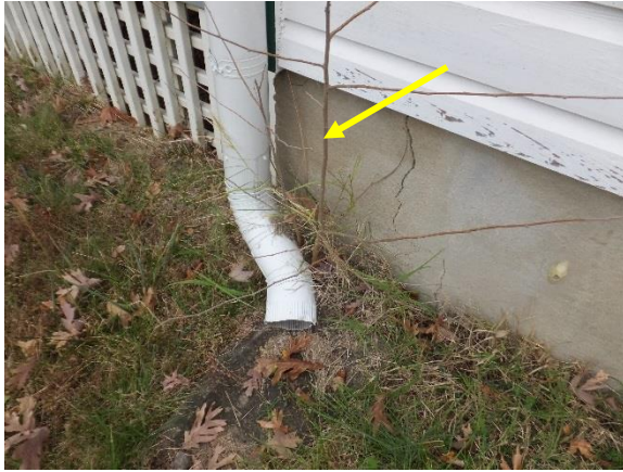
Figure 11. Vegetation along foundation at the southeast facade. Note close proximity of downspout to the house without splash pads and crack in foundation parge coat.
