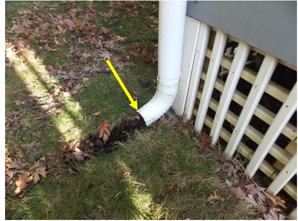
Figure 34. Downspouts terminate near the foundation without splash pads or extensions and have eroded the adjacent soil, typical.
