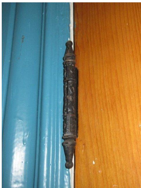
Figure 95. Original ornate steeple door hinge at D207.
