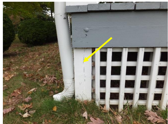
Figure 36. Vertical separation (checking) at wood porch column.
