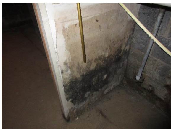
Figure 71. Potential microbial growth at drywall in cellar.
