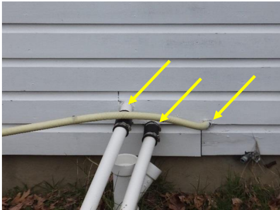
Figure 25. Partially sealed pipe penetrations on southeast facade.
