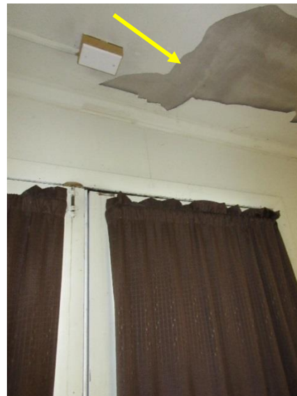
Figure 58. Drywall delamination at rear entryway.
