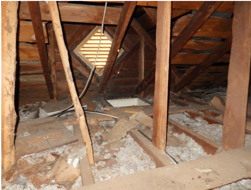
Figure 2. Framing of original attic access.
