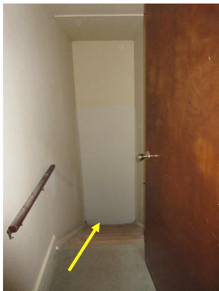
Figure 69. Terminated exterior access of stairwell at D205.
