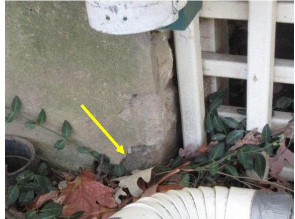
Figure 20. Spall in parge coat at original foundation exposing stone foundation.
