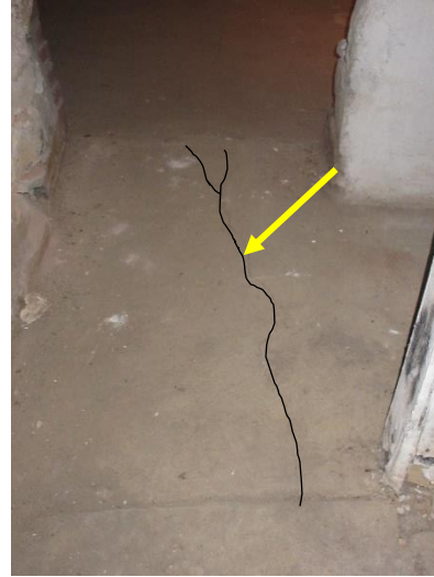
Figure 78. Cracking in concrete floor near the cellar entry. Crack traced for clarity.
