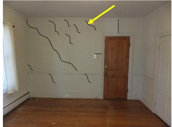
Figure 50. Diagonal and vertical cracking in room 102 (bedroom/family room). Cracks traced for clarity.
