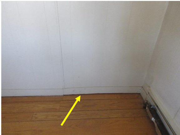
Figure 67. Bowed portion of wood siding panel in Room 210 (office).
