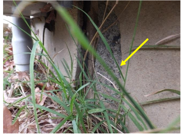
Figure 24. Delamination in parge coat exposing CMU foundation between ca. 1945 and 1984 additions on southeast facade.
