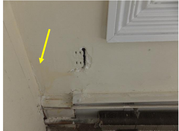
Figure 56. Stained plaster and potential previous repair. Note electrical outlet.
