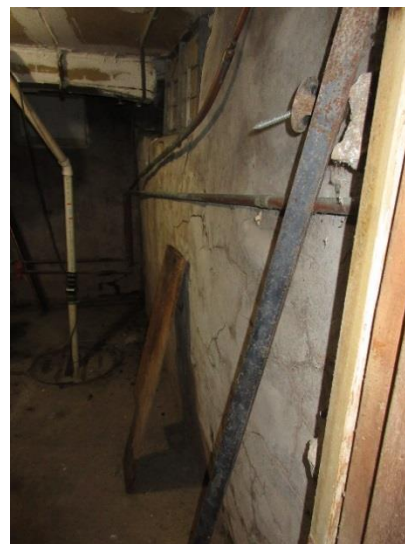
Figure 76. Northwest wall of cellar bowed out of plane and cracking in parge coat. Typical on northwest side of cellar.
