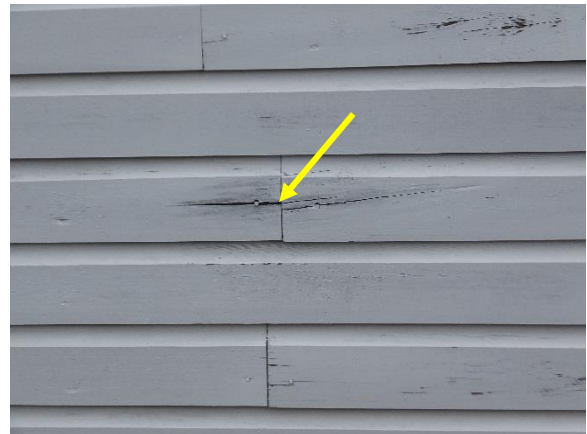
Figure 14. Typical cracking at fastener and end of boards.
