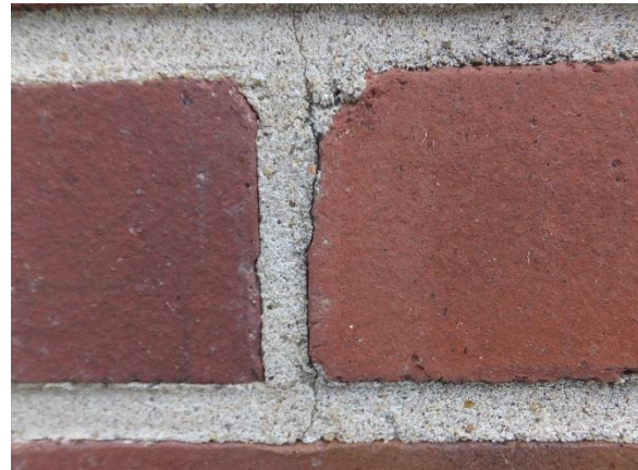
Figure 26. Cracking in mortar joint at chimney on southeast facade.
