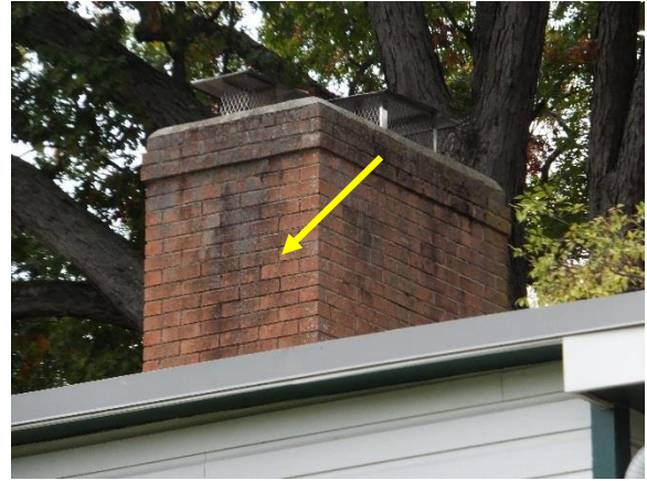
Figure 28. Staining at chimney located at the rear of the 1945 addition.
