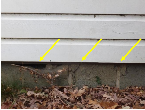
Figure 23. Typical spall and cracking in parge coating and CMU foundation at rear of additions.
