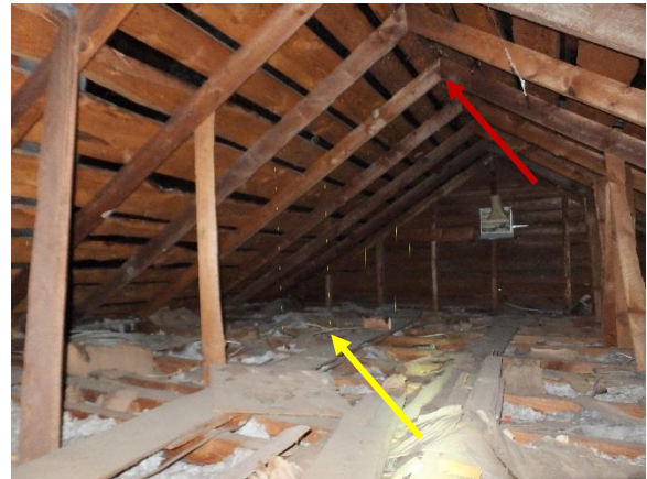
Figure 74. Rafter stud supports not continuous (yellow arrow) in attic and toe-nailed rafters (red arrow).
