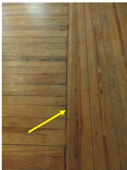
Figure 85. Area in room 101 (living room) where the original hallway wall was located.
