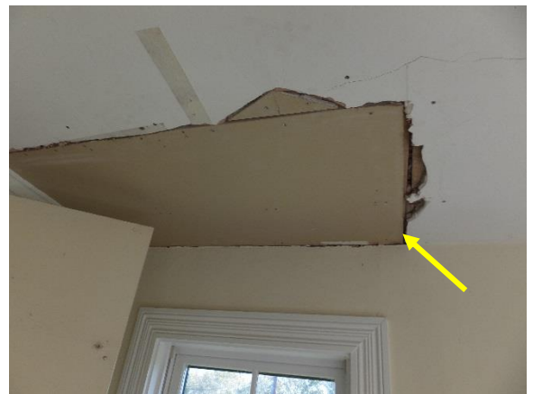
Figure 52. Removed area of plaster with drywall patch in room 201 (bedroom).
