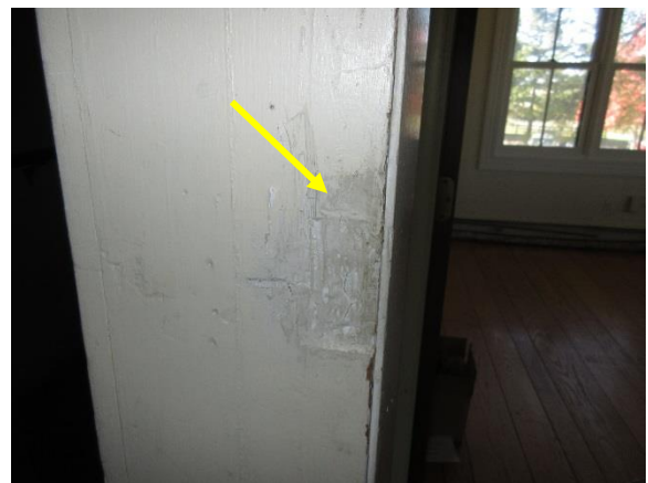
Figure 64 Tooling damage at wood siding panel at entry area adjacent to Room 209 & 210 (offices).
