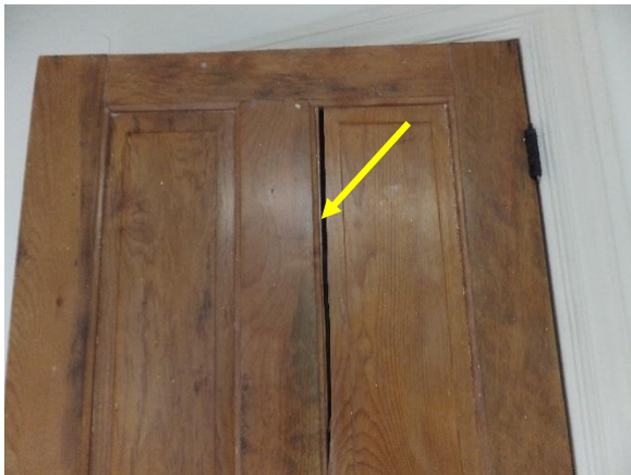
Figure 91. Cracking and missing wood at door panel at D205.
