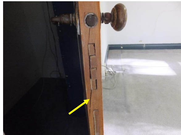
Figure 92. Splitting on stile of door facing latch, at D205.
