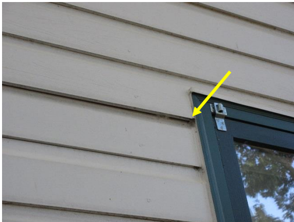
Figure 13. Displaced wood siding adjacent to window a northwest facade.
