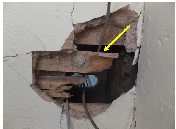
Figure 54. Hole through plaster and lathe for wiring.
