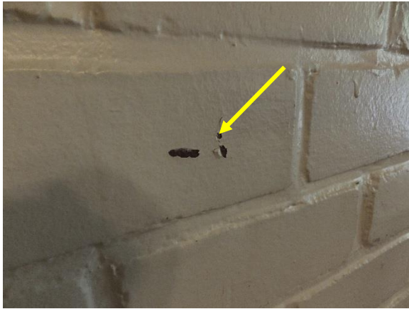
Figure 81. Flaked coating on fireplace brick in living room (room 101).
