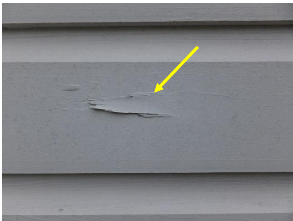
Figure 17. Typical flaked paint, and potentially damaged wood below, on wood siding.
