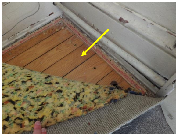
Figure 88. Original wood flooring under carpet.
