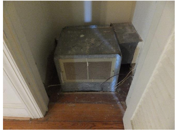
Figure 60. Ductwork installed at closet in stairwell.
