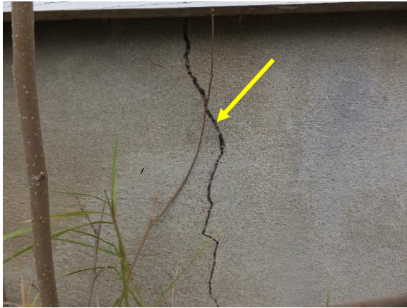
Figure 19. Typical crack and slight delamination in parge coat at original foundation.
