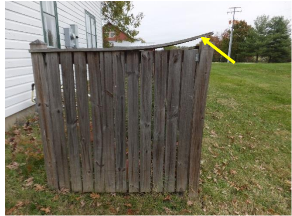
Figure 42. Bowed top rail of fence at southeast facade.
