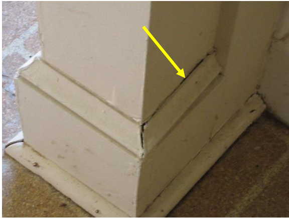
Figure 61. Gap and separation at crown molding, typical.
