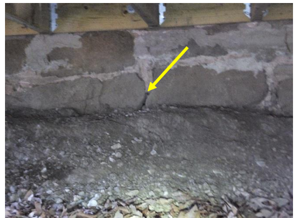
Figure 40. Missing mortar in stone foundation.
