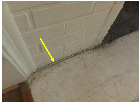
Figure 80. Deteriorated mortar joint between brick fireplace facing and the stone hearth/apron in living room (room 101).
