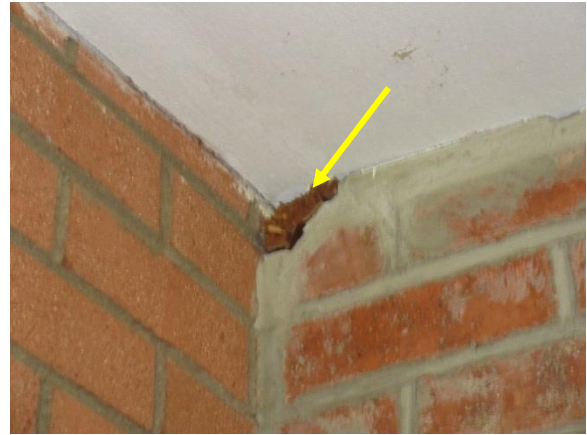
Figure 82. Spalled brick infilled with wood piece at Room 107 (bedroom).
