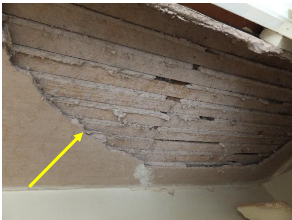
Figure 53. Missing plaster with wood lathe exposed at closet in room 201 (bedroom).
