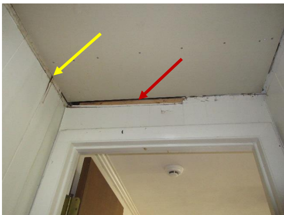
Figure 63. Cracked wood siding panel and gaps at ceiling (red arrow) at entry of Room 210 (office), typical.
