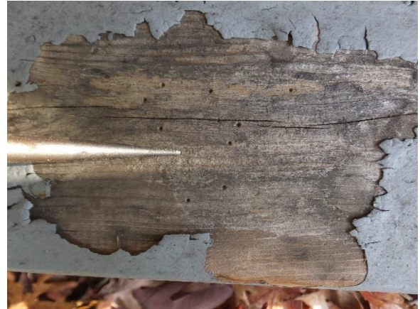
Figure 38. Paint and wood deterioration at porch stairs.
