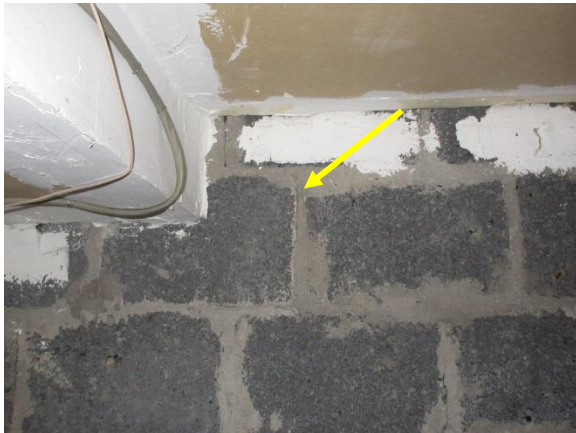
Figure 79. Bondline failure at CMU foundation wall in cellar.
