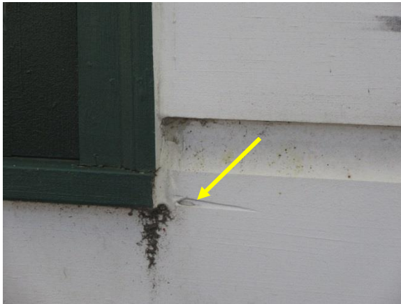
Figure 15. Chip in siding adjacent to a window corner. Typical on northwest facade.
