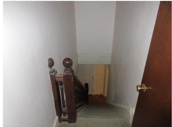
Figure 68. Drywall covering enclosing the historically open original stairwell and handrail.
