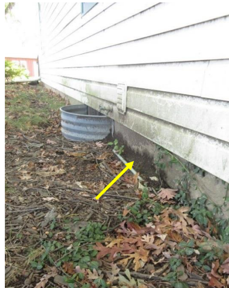
Figure 22. Foundation wall concave at original foundation. Note vegetative growth and staining at parge coat and above siding.
