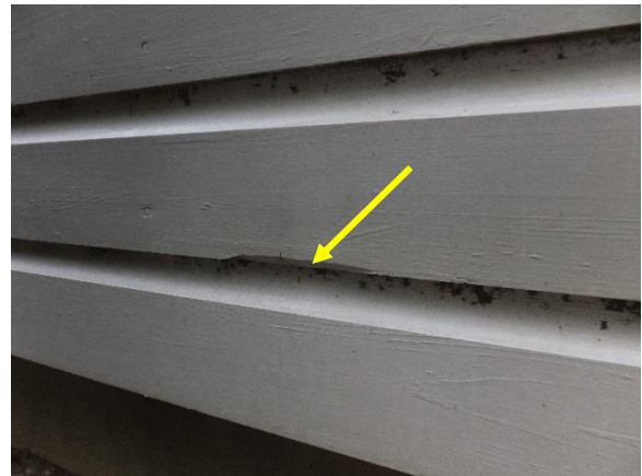
Figure 16. Chipped wood siding at base of siding at northeast facade.
