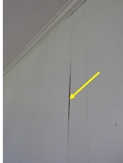
Figure 66. Displaced wood siding panel, typical.
