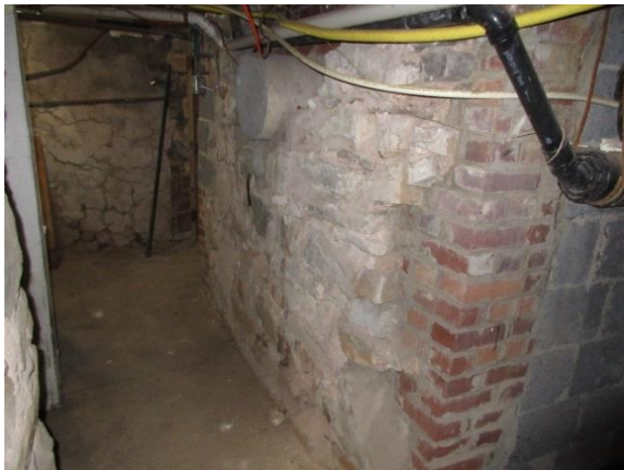
Figure 75. Different types of masonry construction in cellar fieldstone, brick, and CMU.
