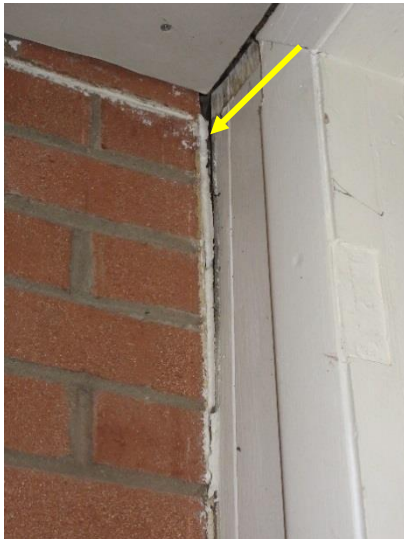
Figure 83. Separation between brick and adjacent wall, typical.
