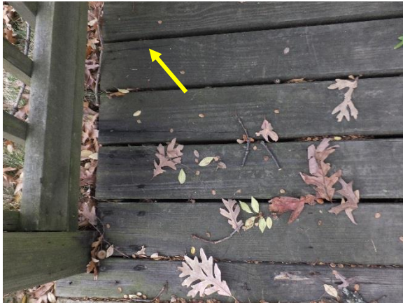
Figure 43. Multiple areas of splintered wood on wood deck at northeast facade.
