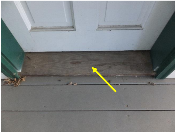
Figure 37. Uncoated wood door threshold at porch with minor areas of splintering.
