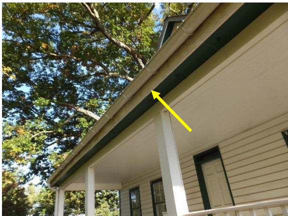
Figure 31. Soiling at fascia board behind gutter.
