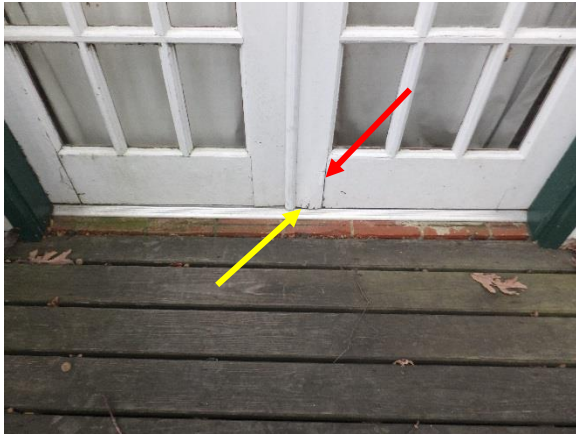
Figure 29. Splintered wood at base (yellow arrow) and separation of joinery (red arrow) at French doors.
