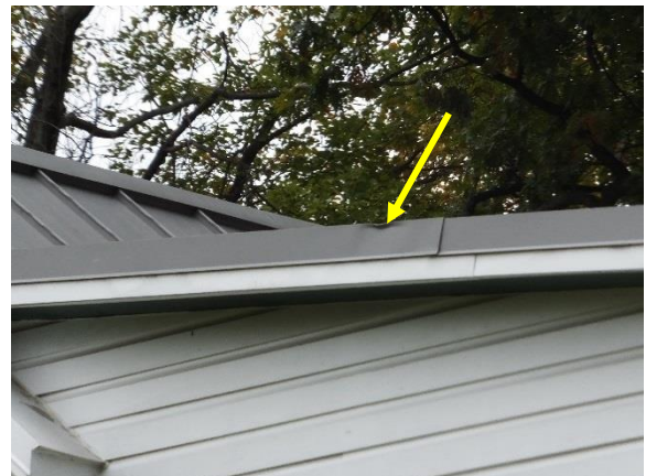
Figure 32. Dent in metal roof coping on southeast facade.
