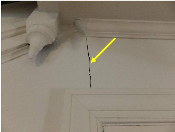
Figure 45. Cracked plaster/drywall above 1st floor doorframe, typical. Crack traced for clarity.
