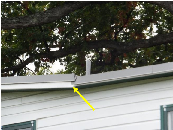
Figure 33. Displaced roof coping on southeast facade.
