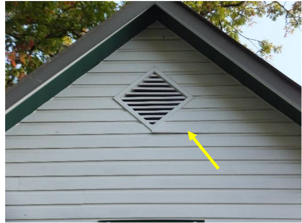
Figure 12. Example of displaced siding at southwest facade.
