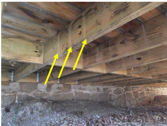
Figure 39. Wood joists under porch exhibiting staining, likely from water.
