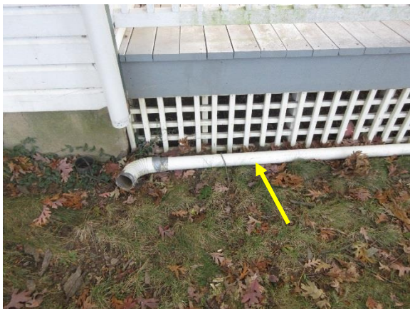
Figure 35. Disconnected downspout at northwest facade.
