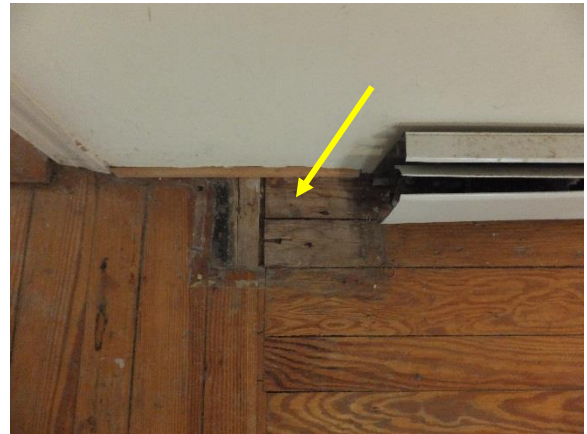
Figure 82. Spalled brick infilled with wood piece at Room 107 (bedroom).
