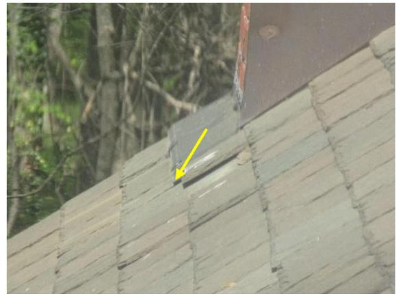
Figure 285. Lifted chimney flashing edge and adjacent slate shingle.
