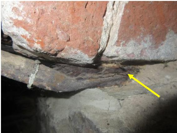
*Figure 380. Corrosion product accumulation at end of curved steel fireplace lintel.*
