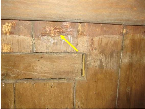
*Figure 378. Indentations and insect damage at subflooring of first floor Hall and Parlor.*
