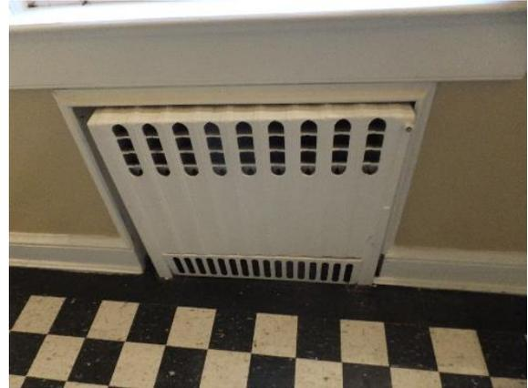
*Figure 151. Radiator below the window built into the wall. This configuration is typical in the 1941 addition at this level.*
