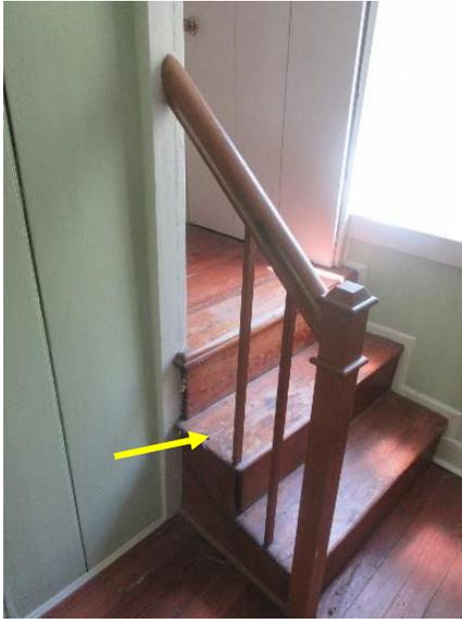
*Figure 368. Missing spindle at parlor staircase.*
