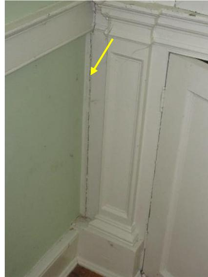
*Figure 339. Separation of seams at cabinetry.*
