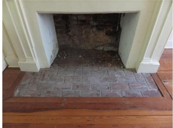
Figure 209. Parged sides of brick firebox. Note brick hearth.
