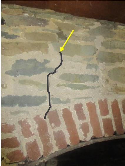
*Figure 354. Vertical cracking at mortar of fieldstone fireplace (crack traced for clarity).*
