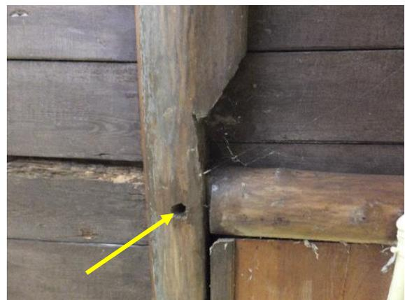
*Figure 125. Drilled beam location through tenon connection.*
