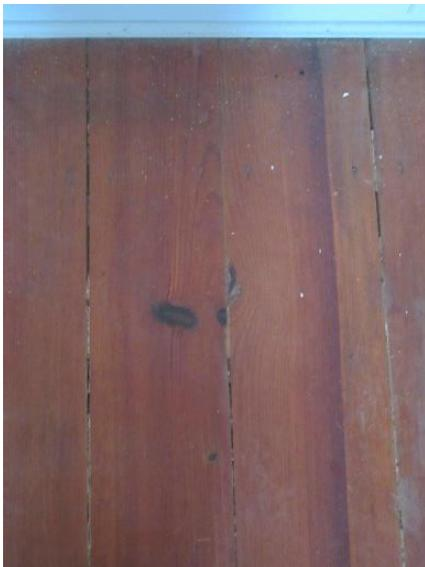
*Figure 384. Multiple areas of material accumulation at gaps between floor boards at the east and west lofts.*
