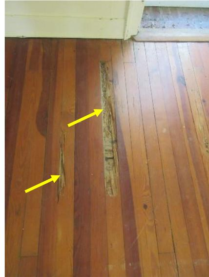
*Figure 381. Missing sections of floorboard in Hall.*
