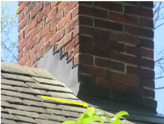
Figure 284. Overall of chimney flashing edges.
