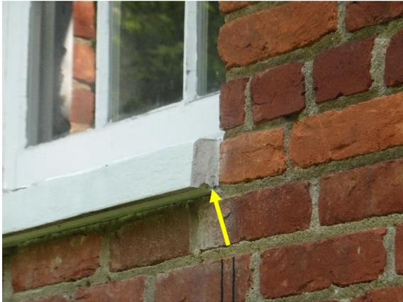
Figure 69. Wood sills at the addition with drip edges.
