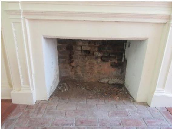
*Figure 350. Dark staining from fireplace use and mortar erosion at fireplace.*
