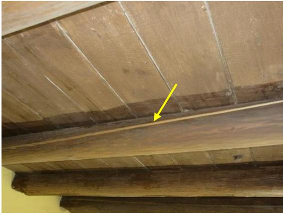
*Figure 374. Splitting at 3/4 round wood floor beams.*
