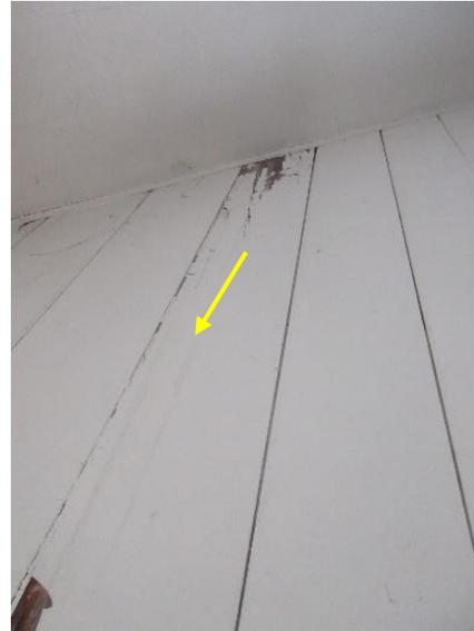
*Figure 345. Vertical cracking of paint at wood bead board panels.*
