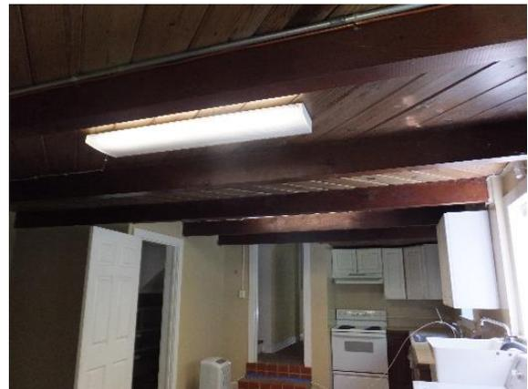
*Figure 107. Fluorescent light installed adjacent to floor beams.*
