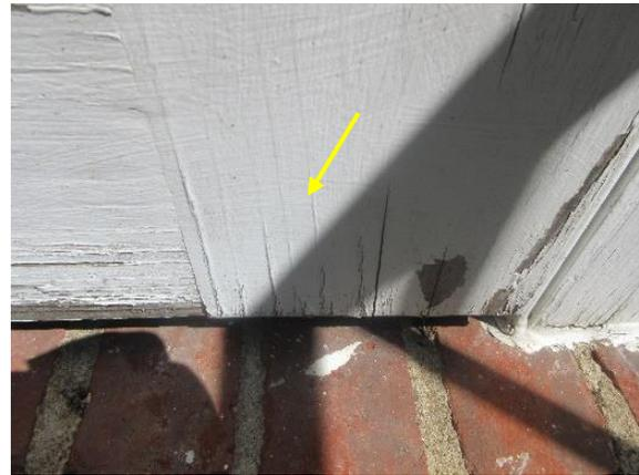
*Figure 305. Cracked paint at door base.*
