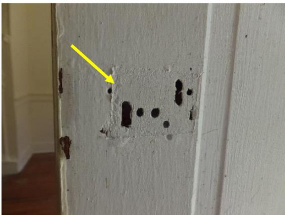
*Figure 218. Holes and ghosting from a removed surface mounted lock, such as a rim lock, at the south door.*
