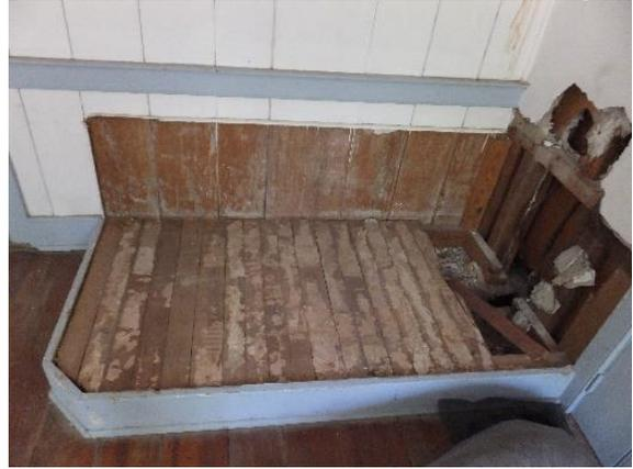
*Figure 240. Removed tub with resultant disrupted interior finishes.*
