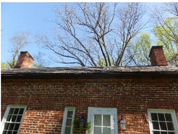
*Figure 87. Interior end chimneys at the original section of the home.*
