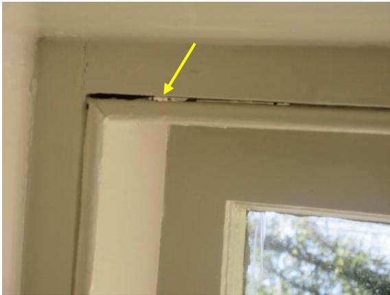
*Figure 300. Separation of frame joinery (interior).*
