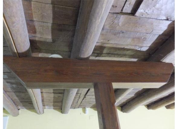
*Figure 127. Retrofit T-Shaped post centered in the cellar.*
