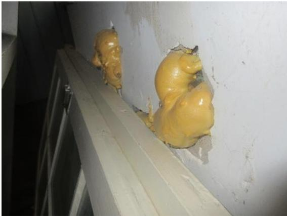
*Figure 392. Abandoned penetrations at west loft bathroom infilled with spray foam.*
