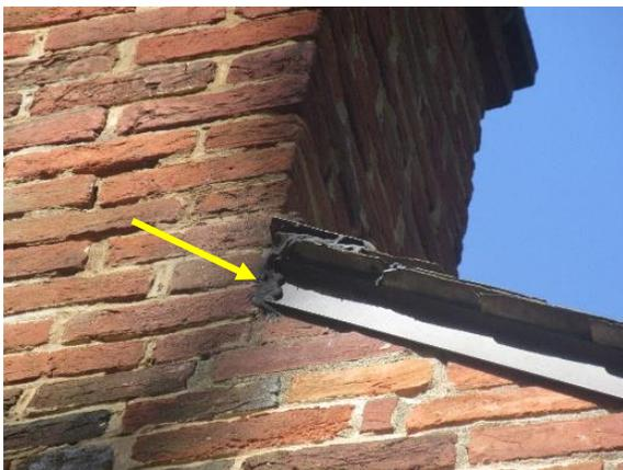
*Figure 280. Mastic at south rake edge.*
