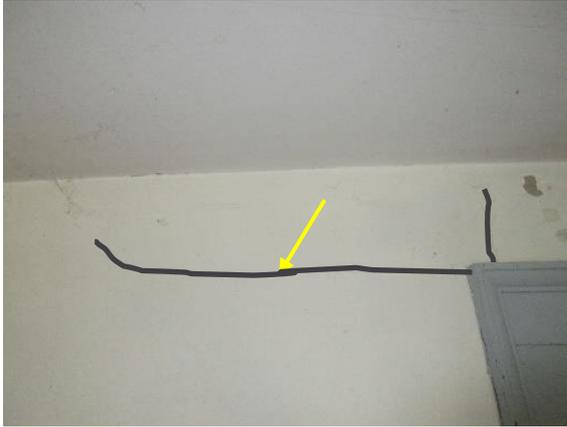
*Figure 318. Plaster cracking adjacent to board and batten door frame of east loft (crack traced for clarity).*
