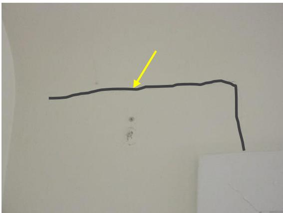
*Figure 316 Plaster cracking adjacent paneled door frame in parlor (crack traced for clarity).*
