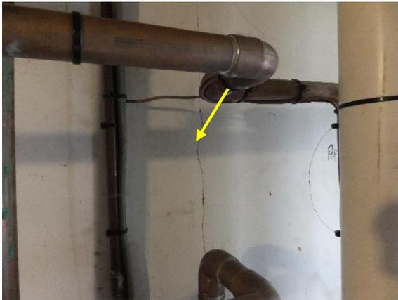
*Figure 320. Parge coating cracking in mechanical area.*
