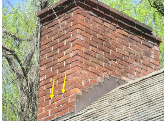
*Figure 269. Sealant at mortar joint.*
