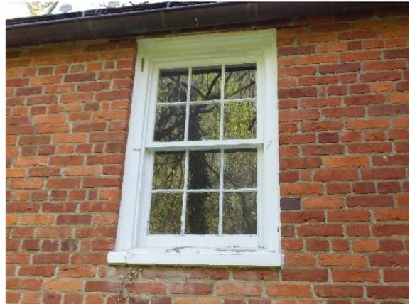
*Figure 62. 6/6 double hung window at the addition. Note pivot hardware.*
