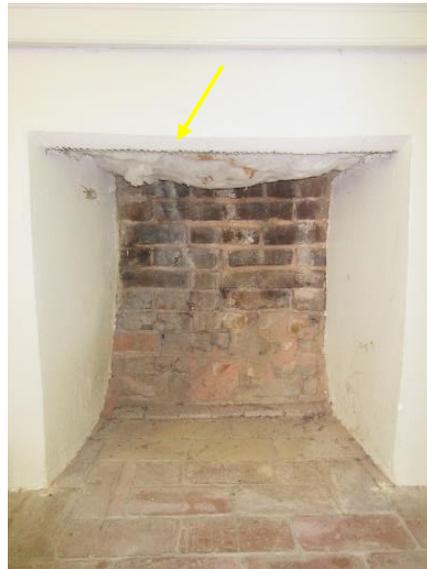
*Figure 351. Insulation installed at the throat of parlor fireplace.*
