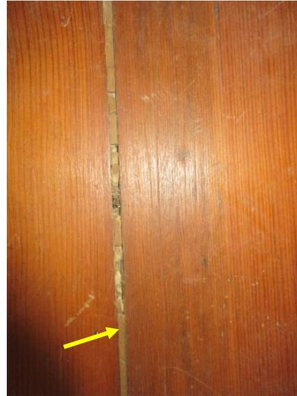
*Figure 383. Wood filler at gap between floor boards at east loft.*
