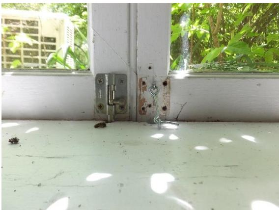
*Figure 65. Contemporary barrel lock and hook added to the bottom of casement windows.*
