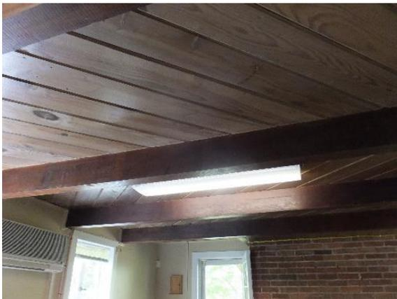
*Figure 106. Exposed floor beams and subfloor in kitchen.*
