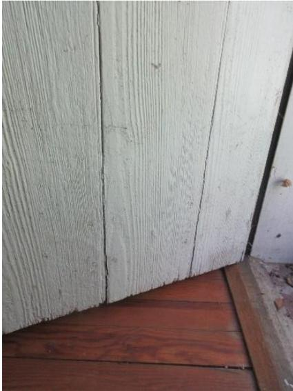
*Figure 356. Weather checking at board and batten bead door base.*
