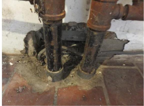
*Figure 325. Cut in parge coating for MEP in mechanical area.*
