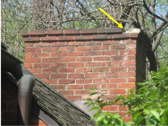
*Figure 276. Surface staining at chimney caps. Note missing brick at corner of chimney cap.*
