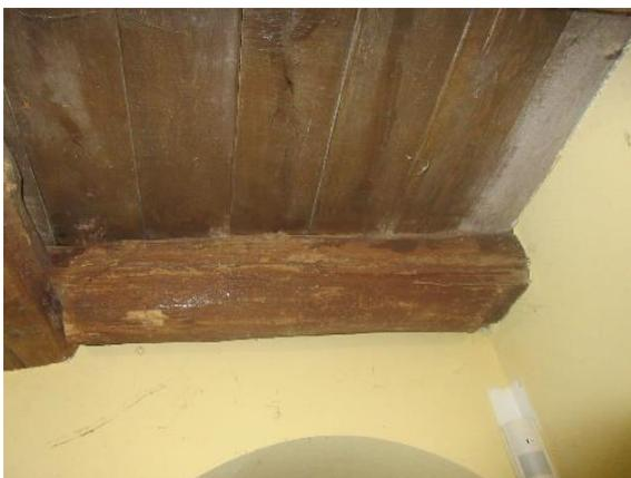
*Figure 124. Rough-hewn floor beam adjacent to fireplace and above interior entryway.*
