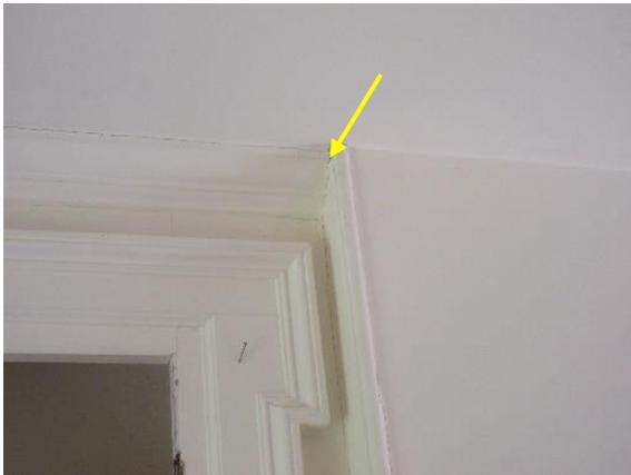
*Figure 338. Separation of joinery at cabinetry trim.*
