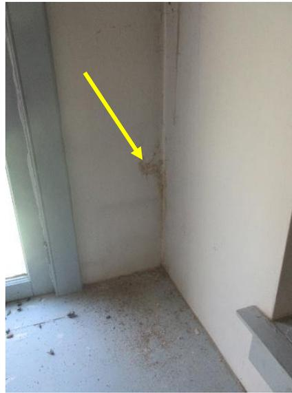
*Figure 327. Water staining, bubbling, and material loss of plaster at lower corner of west loft fireplace.*
