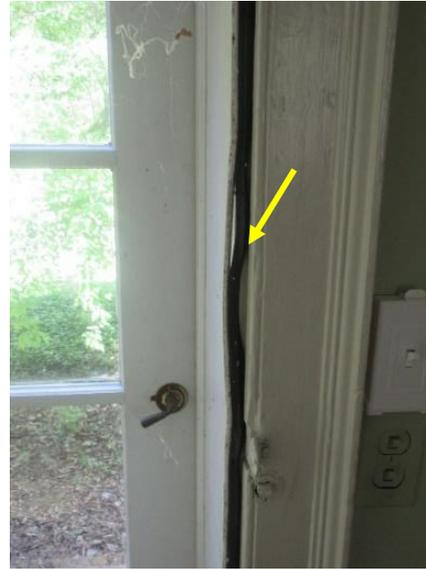
*Figure 311. Foam tape weatherstripping becoming detached at door jamb.*
