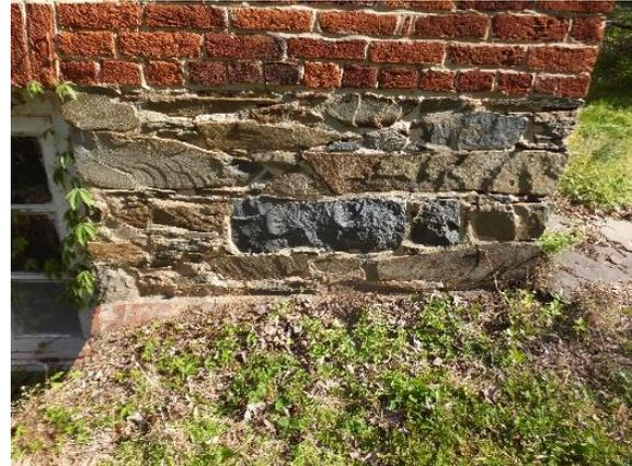
*Figure 44. Stone foundation exposed at the original section of the house.*
