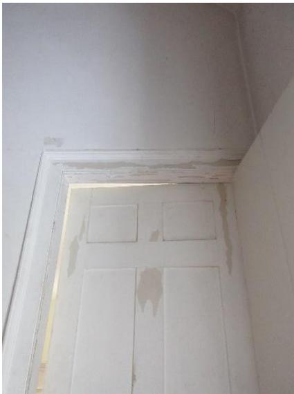
*Figure 346. Flaked paint at interior door.*
