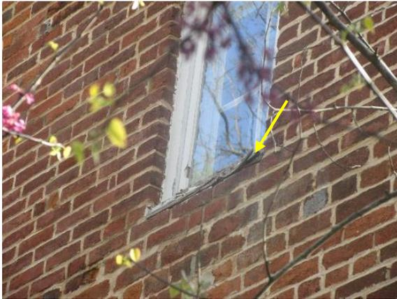
*Figure 298. Deteriorated window sill.*
