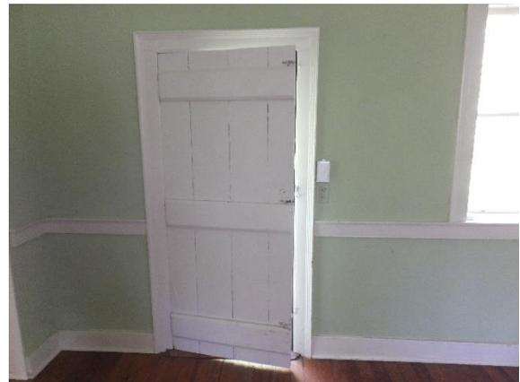
Figure 72. Interior view of the same board and batten door in the Parlor.
