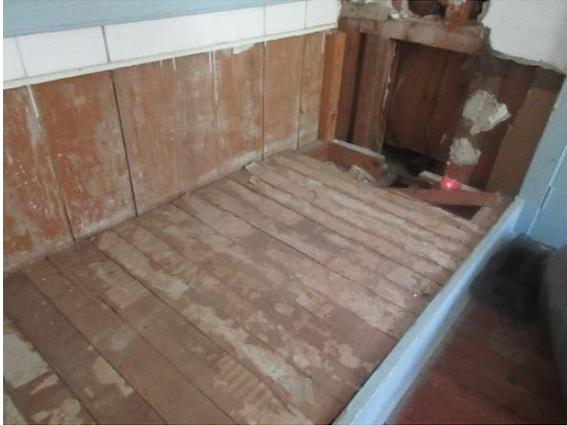
*Figure 372. Staining at wood bead board in tub area.*
