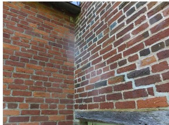
*Figure 48. Interface between the original section of the home (right) and 1941 addition (left).*
