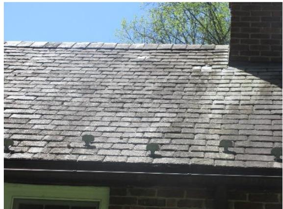
*Figure 52. Copper gutters and snow guards.*
