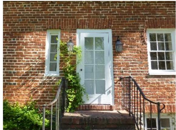
*Figure 76. 4-paneled door at the south facade with glass lite storm door.*
