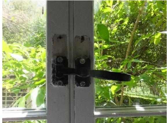
Figure 58. Casement latches at the ground floor windows.
