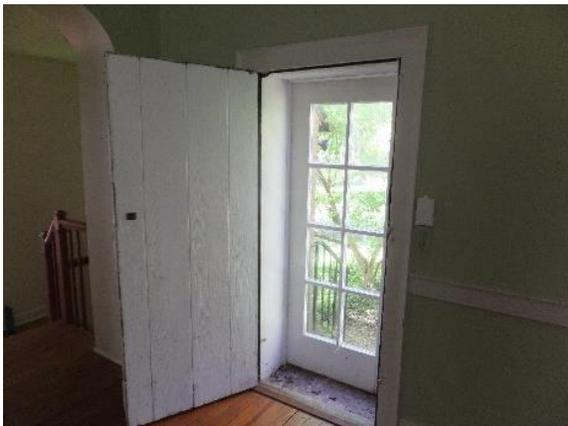
Figure 71. View of the exterior of the board and batten door in the Parlor with glass lite storm door.
