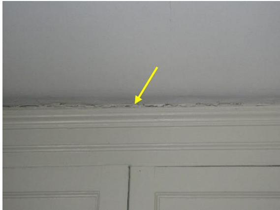
*Figure 340. Separation at ceiling and cabinetry seam.*
