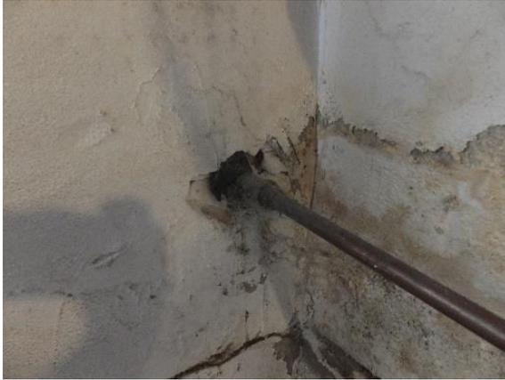
*Figure 332. Potential microbial growth at parge deterioration.*
