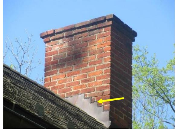
Figure 283. Mastic at copper chimney flashing.
