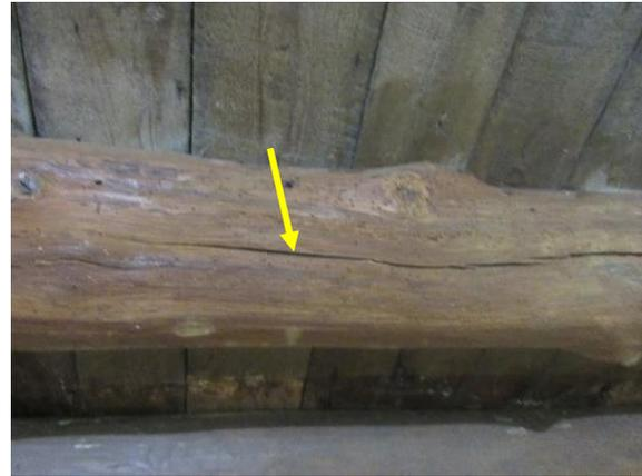
*Figure 375. Checking at original floor beam in cellar.*
