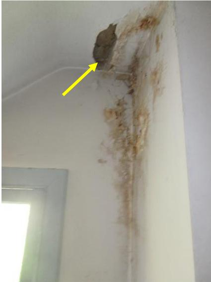
*Figure 328. Location of water infiltration with staining, bubbling, and material loss of plaster at upper corner of west loft fireplace.*
