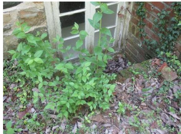
*Figure 291. Foliage and debris accumulation in window well.*
