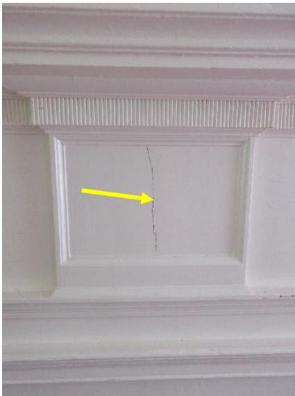
*Figure 370. Vertical crack in wood at mantle panel.*
