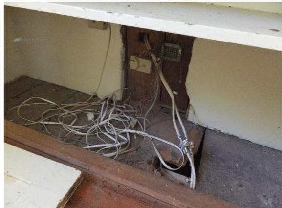
Figure 213. Interior finishes cut at east wall to accommodate wiring.
