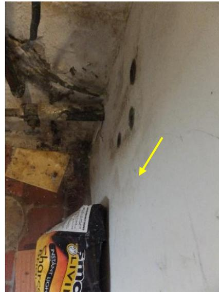
*Figure 335. Inward bow of parge coating at exterior wall in mechanical area.*
