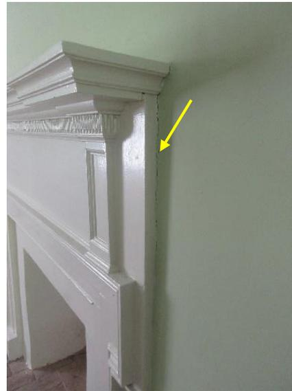
*Figure 341. Separation at wall and mantel seam.*
