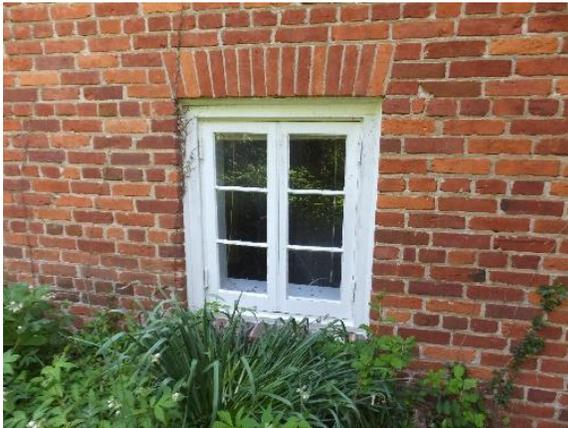
*Figure 61. Typical ground floor casement window at addition.*
