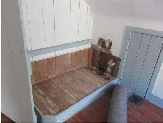
*Figure 324. Cut in plaster and beaded wood wall for plumbing in west loft.*
