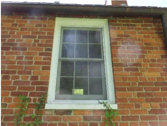
*Figure 63. 6/6 double hung window at the addition with installed screen.*
