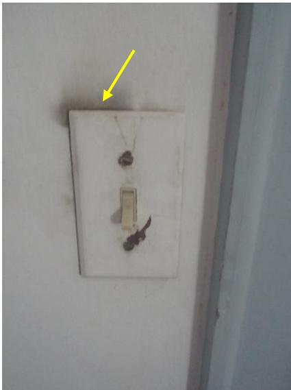
*Figure 330. Black burn marks at electrical switch.*
