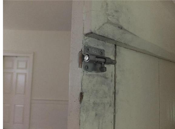
*Figure 215. Typical barrel locks added to the interior sides of first floor exterior doors.*
