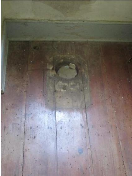
*Figure 386. Staining at cut in wood floor board for plumbing at the west loft.*
