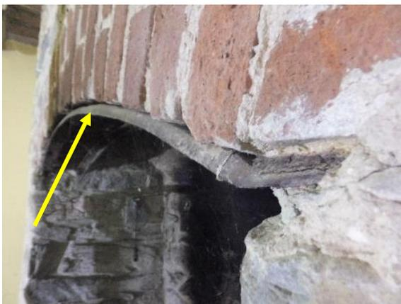
*Figure 134. Iron chimney bars.*
