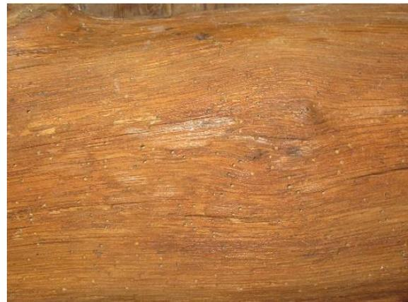
*Figure 377. Grain separation at original framing beams. Note pin holes in wood.*
