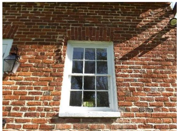
*Figure 54. Typical 6/6 double hung window at the original section of the home.*
