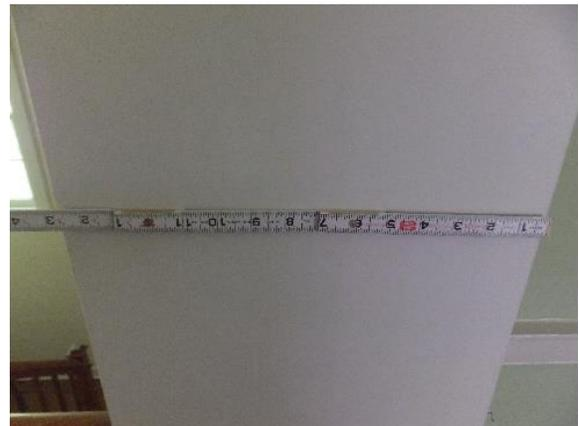
*Figure 173. The entryway is cut through the original brick exterior west wall and is 14-3/4 inches thick with interior finishes.*
