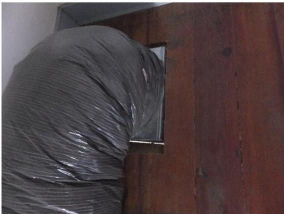
*Figure 255. Ductwork penetration through the wood floor was observed in both loft rooms.*
