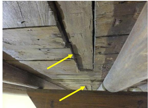
*Figure 129. Interruptions of subfloor that correspond with interior wall between the hall and parlor.*
