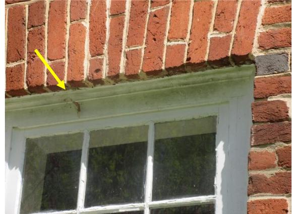
Figure 68. Steel lintel above windows at the addition.
