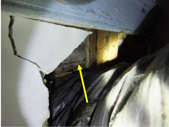
*Figure 257. Original plaster and wood lathe was observed in the interior wall ductwork penetration in the loft east room.*
