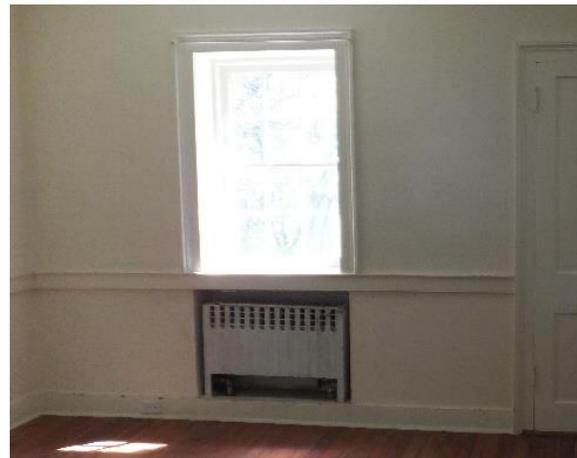
*Figure 219. Radiators located below windows.*
