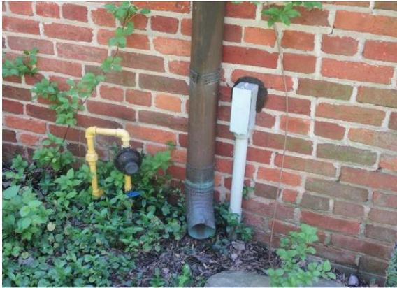
*Figure 288. Downspout close to masonry wall.*
