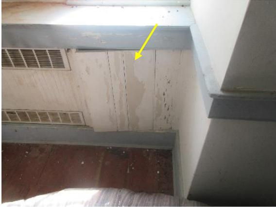
*Figure 348. Cracked and flaked paint at built-in cabinetry in loft spaces.*
