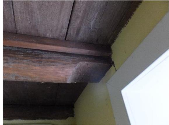
*Figure 123. Notching of floor beams to timber sill.*
