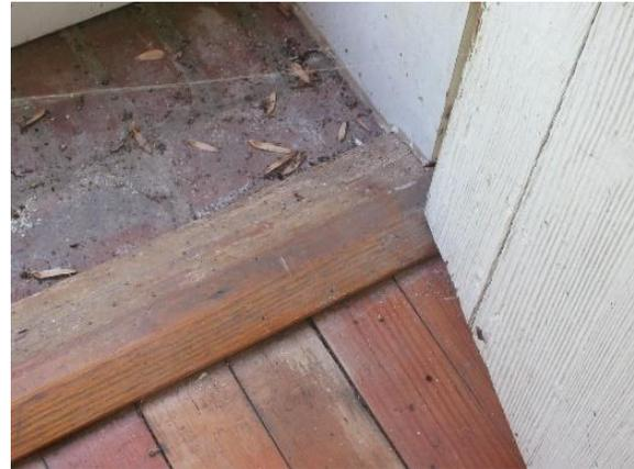
*Figure 365. Weather-checking and fading varnish at door threshold.*
