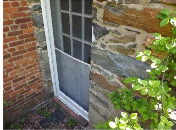
*Figure 74. Cellar door and metal screen door through stone foundation.*
