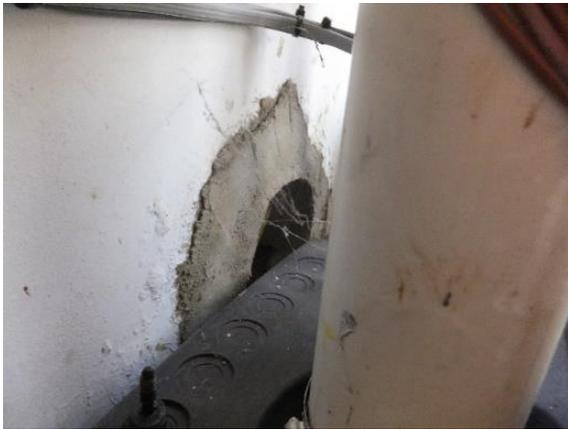
*Figure 326. Cementitious material at cut in parge coating for abandoned penetration.*
