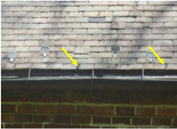
Figure 282. Mastic at slate joints.
