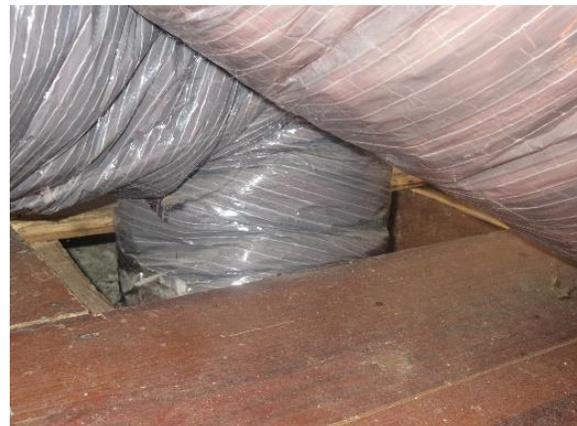
*Figure 385. Cut in wood flooring to accommodate ductwork at east loft.*
