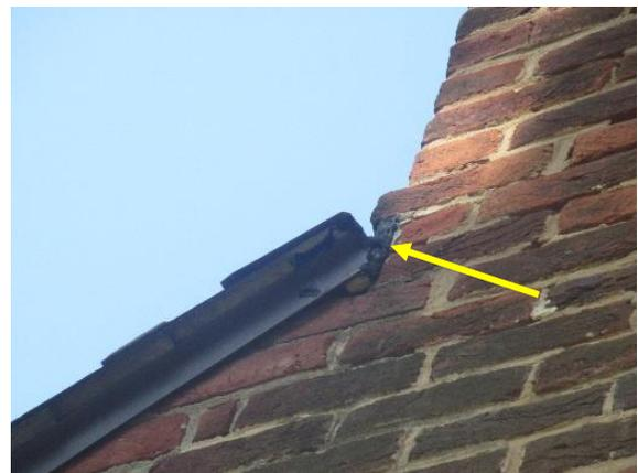
*Figure 281. Mastic at north rake edge.*
