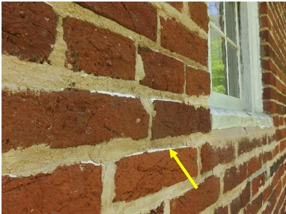
*Figure 41. Isolated remnants of white coating observed on the north facade at the exposed brick-to-mortar surfaces.*
