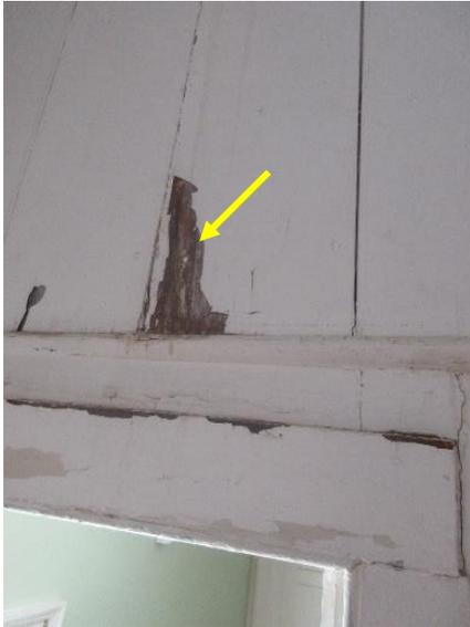
*Figure 344. Cracked and flaked paint and wood bead board panels*
