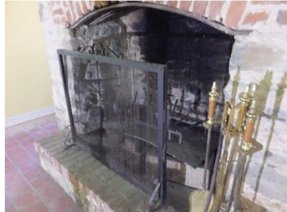
*Figure 133. Stone firebox with metal fire screen.*
