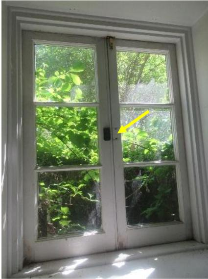
*Figure 302. Missing window interior lock (interior).*
