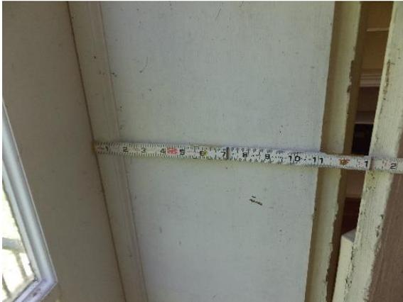
*Figure 216. Door casing that is 12 inches wide to accommodate the thickness of the brick wall.*
