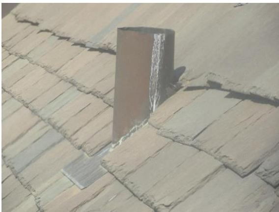
Figure 286. Pipe penetration through slate roof.
