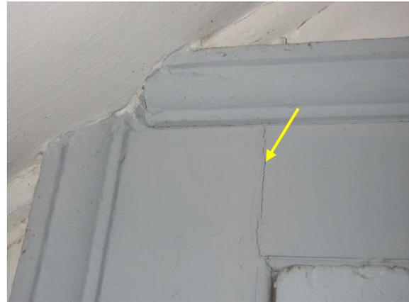
*Figure 357. Separation of joinery at board and batten door frame.*
