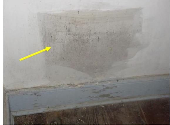
*Figure 337. Lack of paint coating from previously removed toilet location.*
