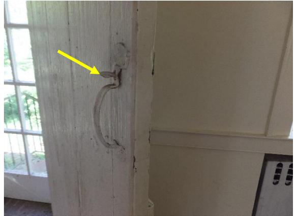
Figure 80. Thumb latch and handle remaining in Hall.
