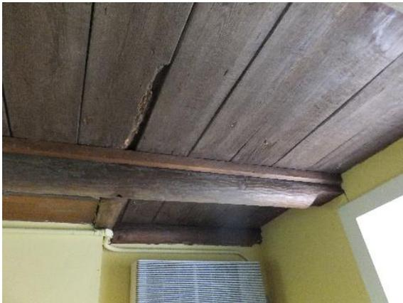
*Figure 128. Retrofit of wood member between beam and subfloor.*
