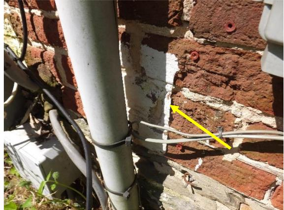
*Figure 40. Remnant white coating observed at the east facade behind conduit.*
