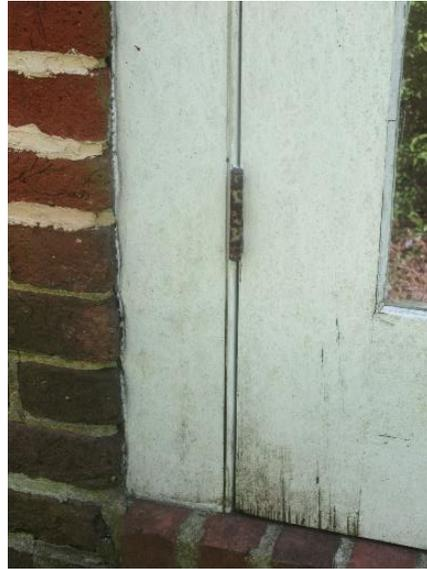
*Figure 307. Modest deterioration at the bottom of the wood storm door.*
