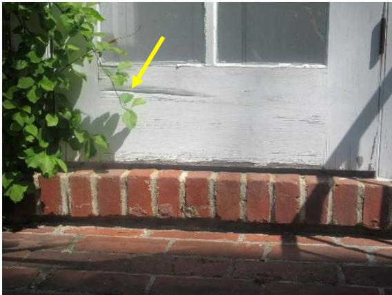
*Figure 308. Crack in wood at bottom rail of storm door.*
