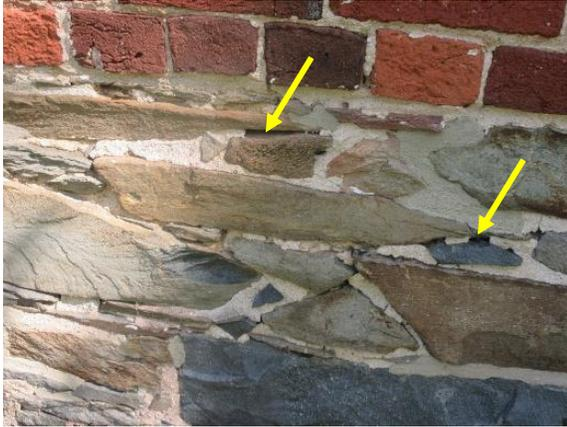
*Figure 258. Missing mortar locations at fieldstone foundation.*
