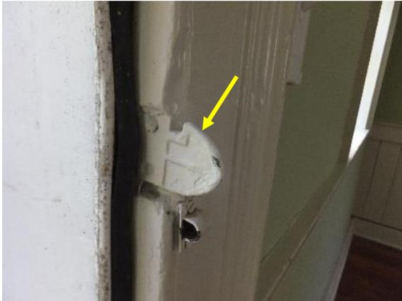
Figure 79. Metal catch remaining at trim in Parlor. Note added hasp for barrel lock.
