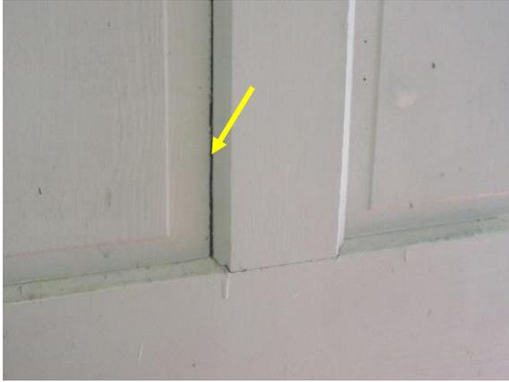
*Figure 360. Separation of joinery at center stile of paneled door.*
