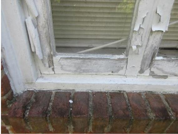
*Figure 292. Cracked and peeling paint at window.*
