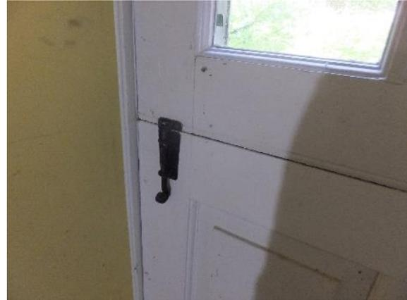
*Figure 84. Typical interior door hatch at dutch doors.*
