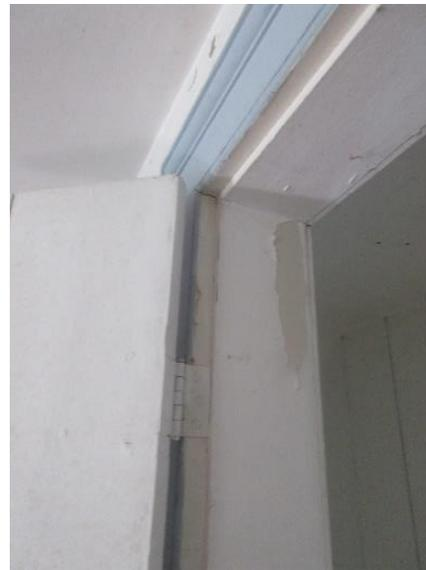
*Figure 347. Flaked paint at door frame.*
