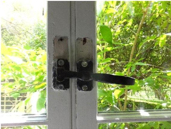
*Figure 304. Replaced window hardware.*
