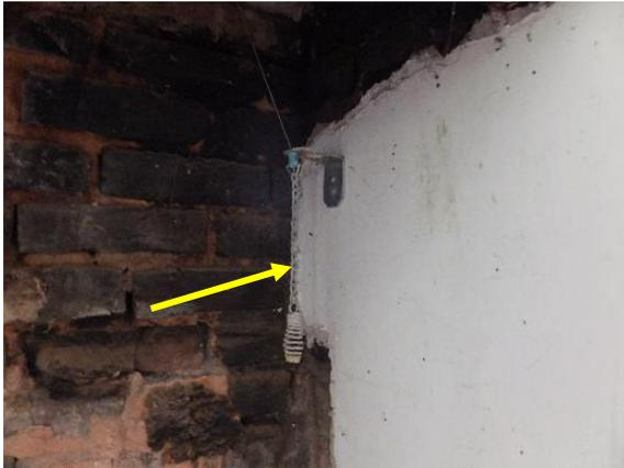
Figure 210. Typical damper pull chain.
