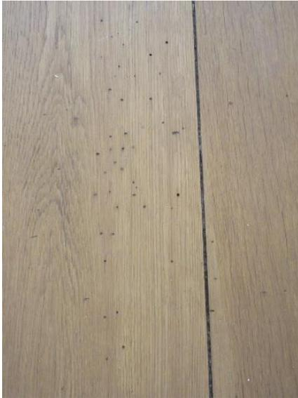
*Figure 382. Potential insect damage at floor board in the living room.*
