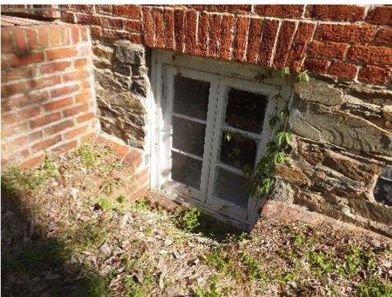
*Figure 53. Typical cellar paired casement window.*
