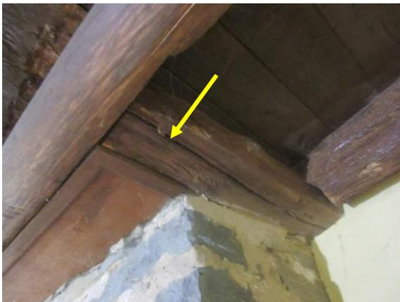
*Figure 376. Wood splintering/splitting at original beams framing the cellar fireplace.*
