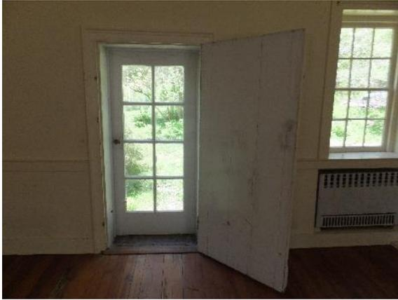
*Figure 73. View of the exterior of the board and batten door in the Hall with glass lite storm door.*
