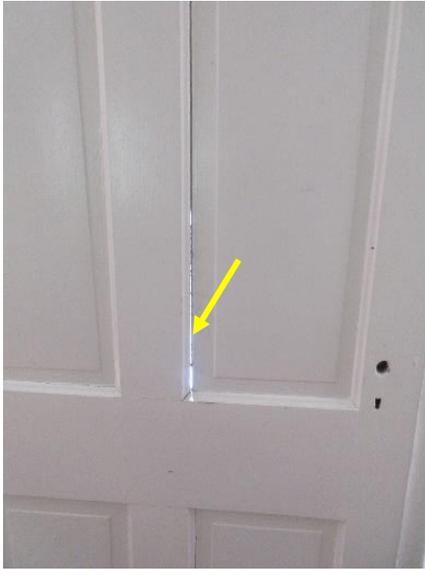
*Figure 310. Daylight observed at exterior door panel.*
