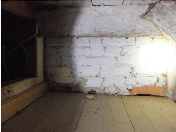
*Figure 196. White coating on south wall brick and continuation of wood floorboards.*
