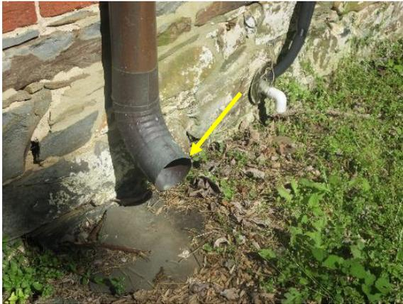
*Figure 264. Downspout without a splash pad or extension.*
