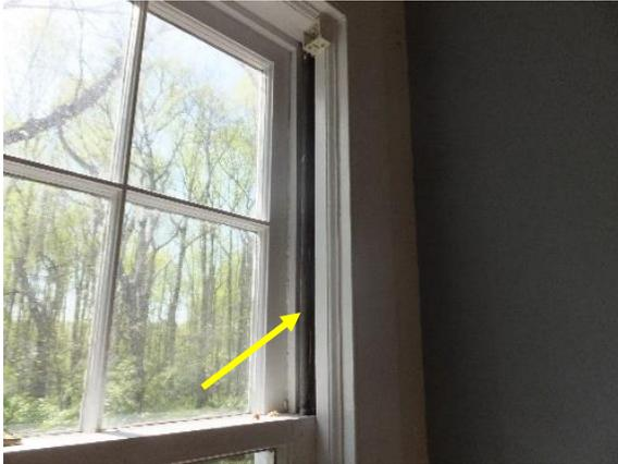
Figure 67. Spiral tube balance present at 6/9 double hung windows.
