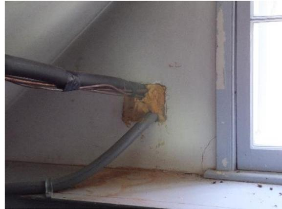
*Figure 254. Mechanical conduit penetration through the east wall.*
