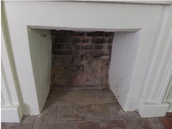
*Figure 180. Parged sides of firebox.*
