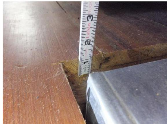
*Figure 256. Thickness of tongue-and-groove floorboards was observed at the ductwork cut in floor.*
