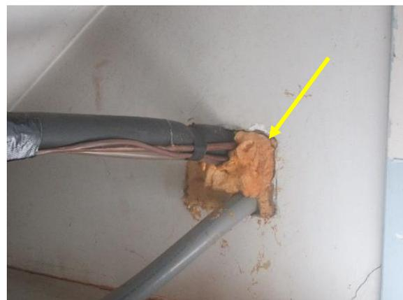
*Figure 323. Cut in plaster and spray foam for conduit penetrations at east loft exterior wall.*
