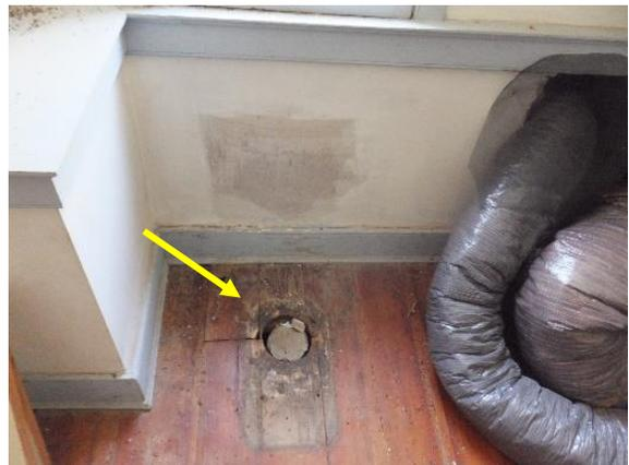
Figure 238. Area of a removed toilet.
