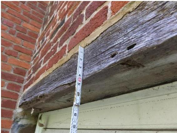
*Figure 45. Large timber lintel observed at the cellar door on the west facade.*
