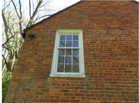
*Figure 64. Typical 6/9 double hung window.*
