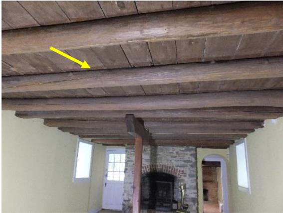
*Figure 122. Exposed 3/4 round floor beams run north-to-south. Note shadowing adjacent to beams.*
