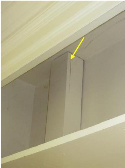
*Figure 364. Splitting at vertical support member in built in cabinetry.*
