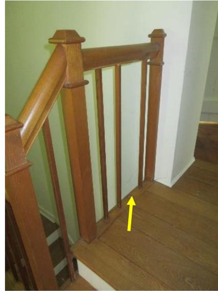
*Figure 369. Missing spindle at first floor staircase.*
