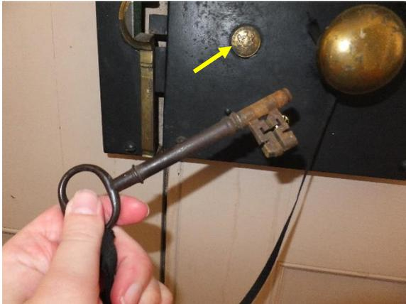
*Figure 60. Barrel key for the main door. Note Carpenter & Co. Patentees seal with British Royal Arms centered.*
