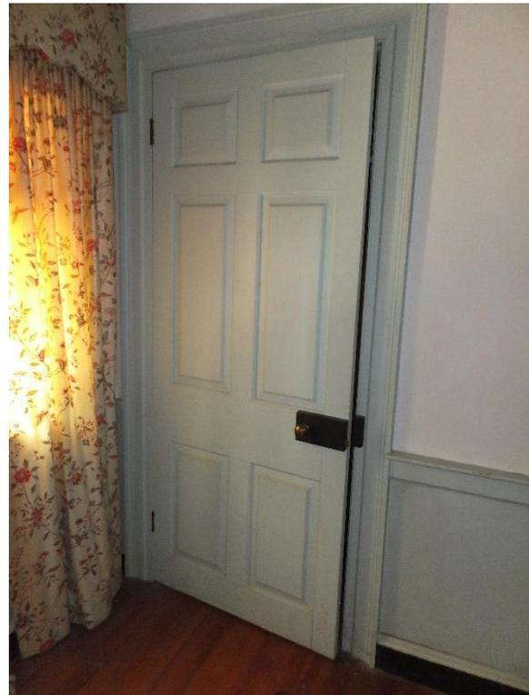
*Figure 185. Paneled closet door with horizontal rim lock.*
