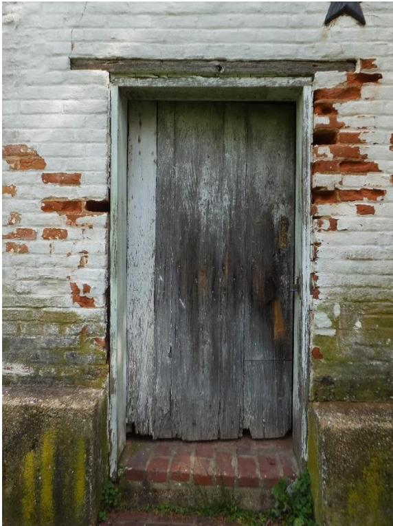
*Figure 293. Board and batten door at the south facade.*
