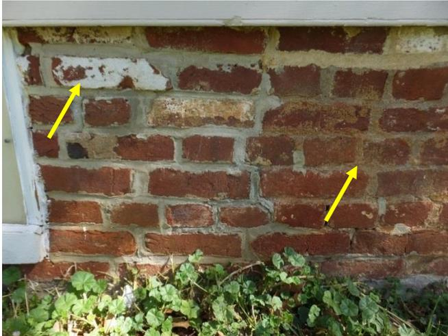
*Figure 47. Reddish tint at mortar. Note multiple campaigns of repointing visible through the differing mortar colors and white coated brick.*
