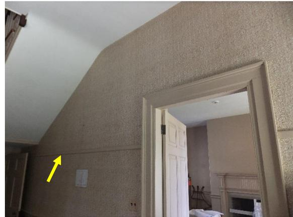
*Figure 137. Horizontal board added to the east wall. Note slope of ceiling as it transitions to room 104.*
