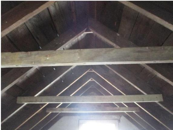
*Figure 325. Machine cut roofing members.*
