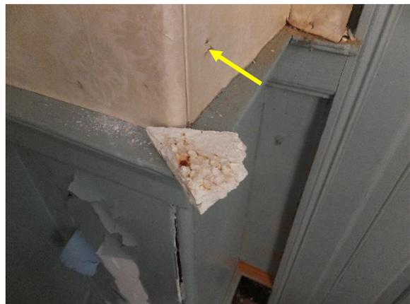
*Figure 161. Wall sheathing applied around fireplace evidenced by screws.*
