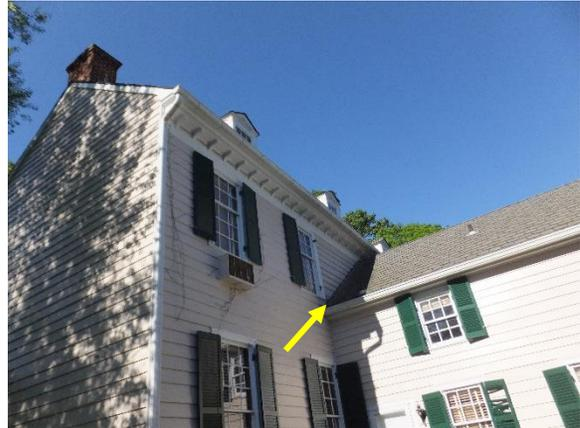
*Figure 44. Current intersection of the central gabled roof to the north facade does not show ghosting of a previous roofline as indicated in HABS drawings.*
