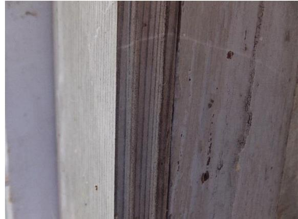
*Figure 292. Profiling of stop bead at the interior of the first floor windows.*
