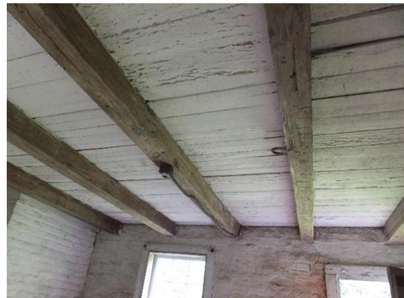
*Figure 314. Hand hewn floor beams running north to south.*
