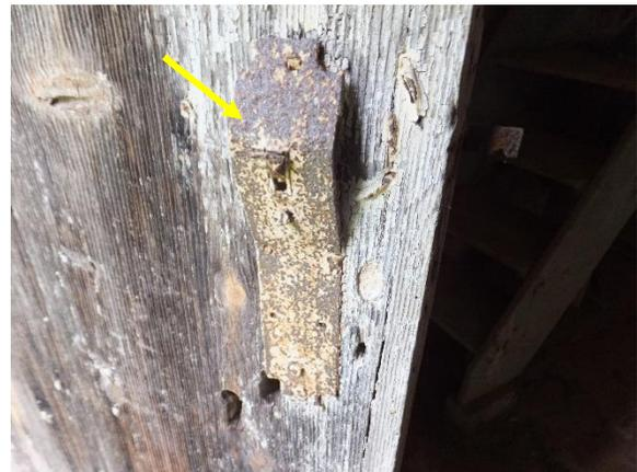
*Figure 294. Wrought iron thumb latch.*
