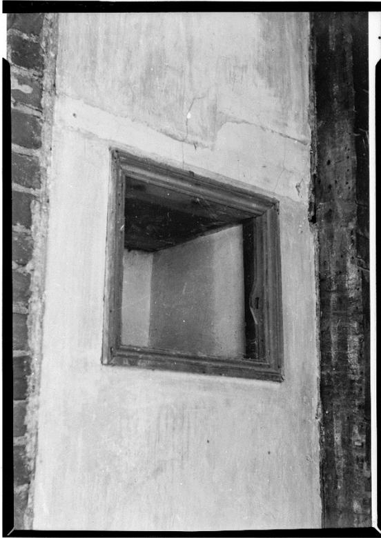
*Figure 104. View of the warming cupboard at the south side of the fireplace in room 102 ca. 1960. (Photo courtesy of HABS).*
