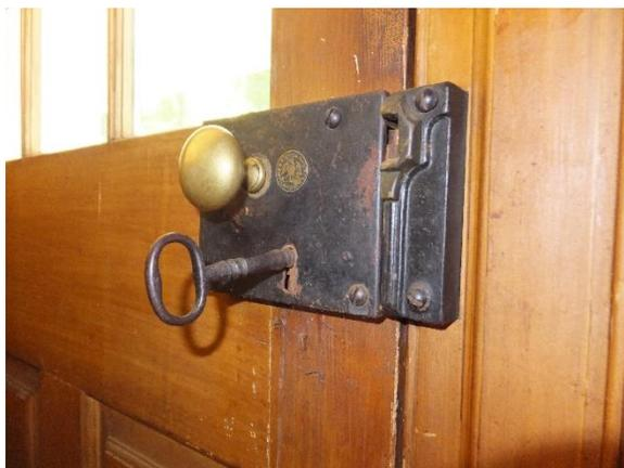
*Figure 68. "No. 60 Improved Rim Lock" with barrel key at the kitchen door. This lock predates the current kitchen structure.*
