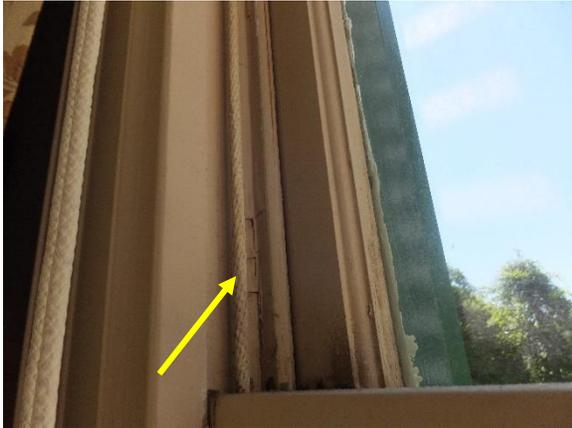
*Figure 54. Rope lift located at a window at the south facade.*
