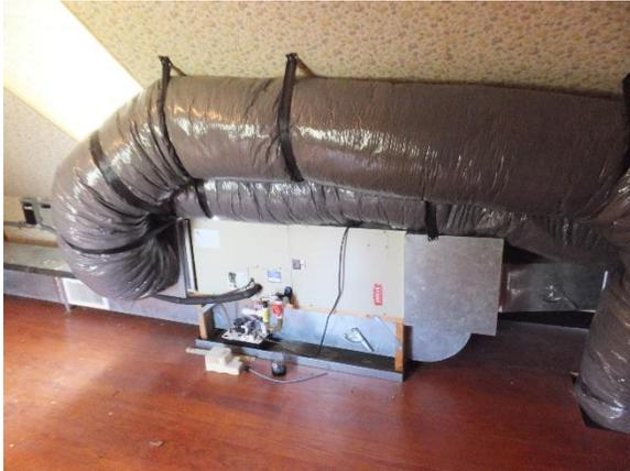
*Figure 240. Mechanical unit located at the south wall. Ductwork penetrates through the flooring and walls.*
