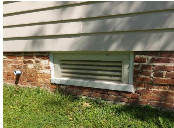
*Figure 31. Detailing of wood timber sill on top of the brick foundation with ventilation louver centered in 2017.*
