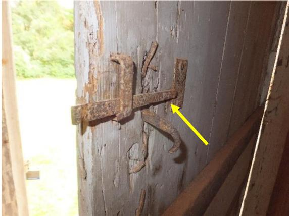
*Figure 295. Thumb latch at exterior activated lever at the interior.*
