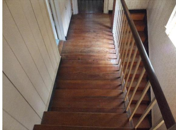
*Figure 225. Flooring in room 204 runs east to west rather than north to south as reflected on the HABS drawings.*
