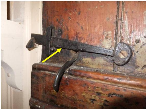
*Figure 64. Wrought iron latch at the interior of the board and batten door.*
