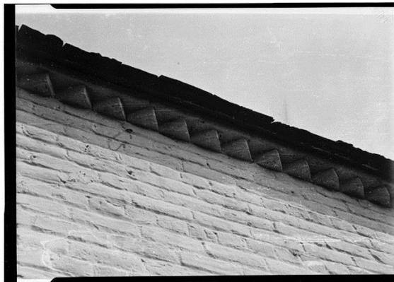
*Figure 276. View of dog-toothed brick cornice ca. 1960. (Photo courtesy of LOC)*
