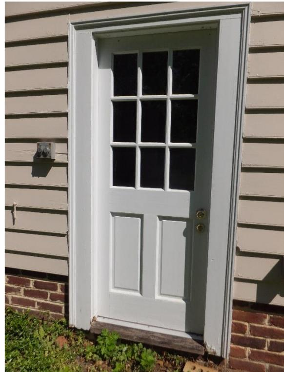
*Figure 65. Typical upper divided light exterior doors at the garage.*
