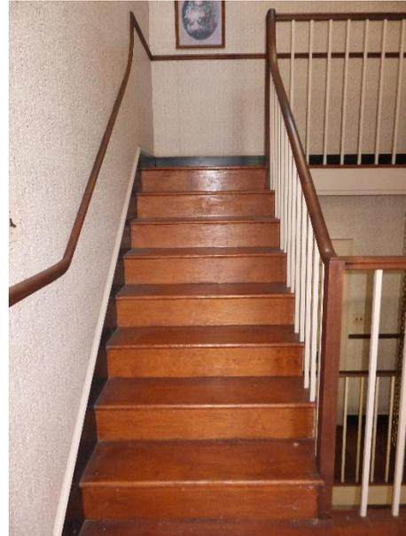
*Figure 233. Treads and risers are of differing dimensions as below levels.*
