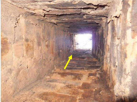
*Figure 246. View into chimney looking up. Note wire mesh in chimney.*
