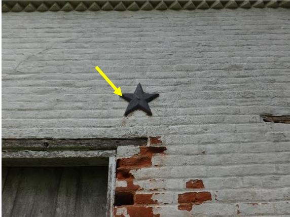
Figure 281. Star anchor plates and associated tie rods.
