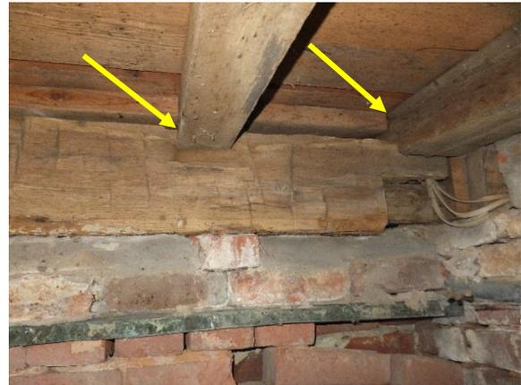
*Figure 151. View of floor beams notched to a timber sill looking west.*
