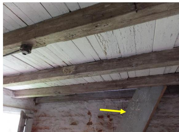
*Figure 316. Ladder stairs nestled between floor beams at the west wall.*
