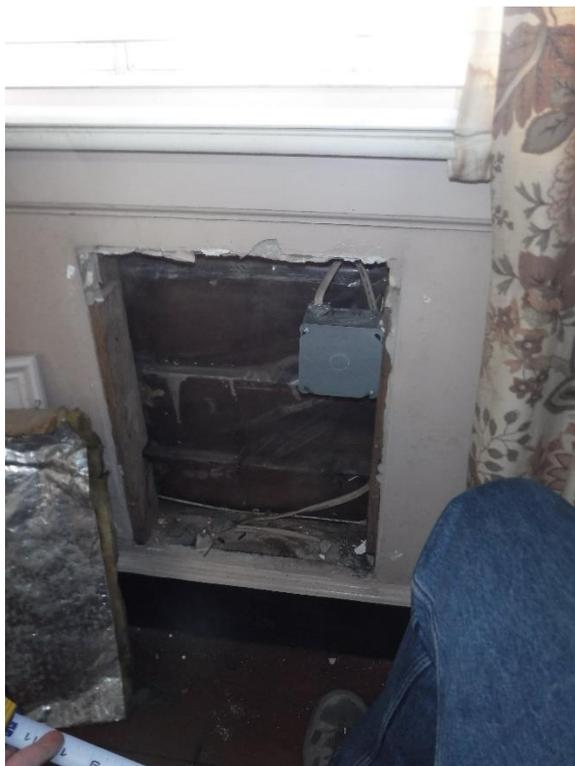
*Figure 152. Access hatch removed in room 102 revealing backside of clapboard siding.*
