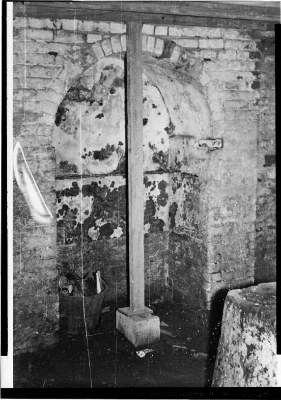
*Figure 106. View of the brick masonry arch support for the east fireplace in room 102 ca. 1960. (Photo courtesy of HABS).*
