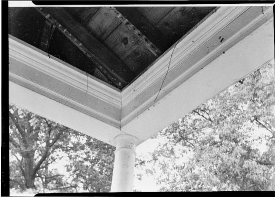
*Figure 24. Detailing of the southwest corner of the portico cornice (note ceiling removed during restoration) ca. 1960. (Photo courtesy of HABS).*
