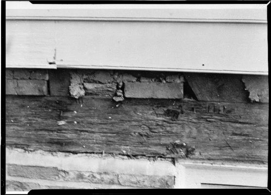
*Figure 28. Detailing of wood timber sill on top of the brick foundation exposed during the restoration work ca. 1960. (Photo courtesy of HABS).*
