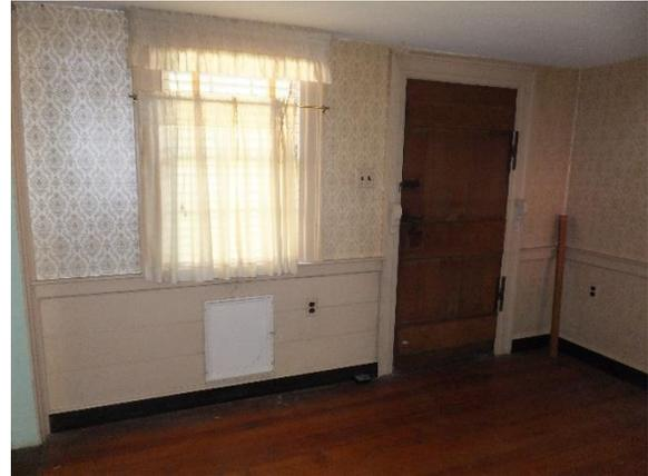
*Figure 173. View of east wall of wallpaper, chair rail, and shiplap.*
