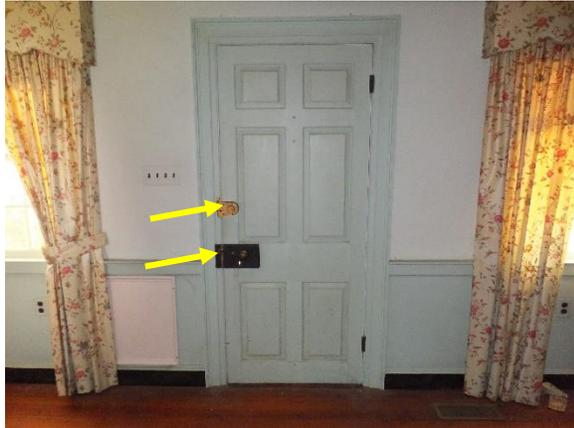
*Figure 70. Carpenter lock and Yale lock in place at the exterior door of room 105.*
