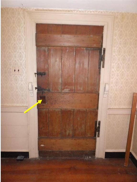
*Figure 62. Interior of east facade board and batten door with door pull and wrought iron latch.*
