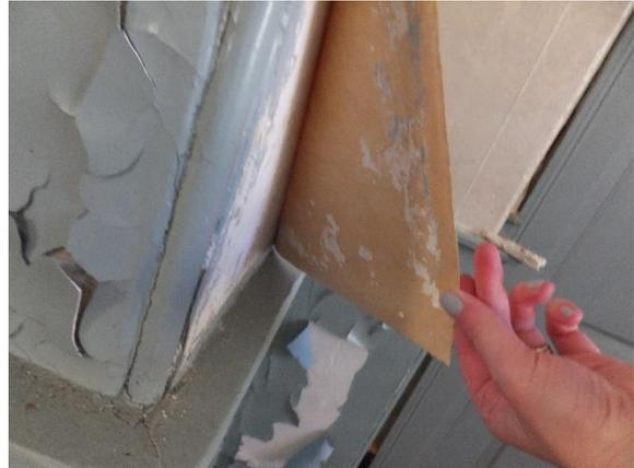
*Figure 157. Backside of wallpaper where peeling from wall at the northwest corner of the room.*
