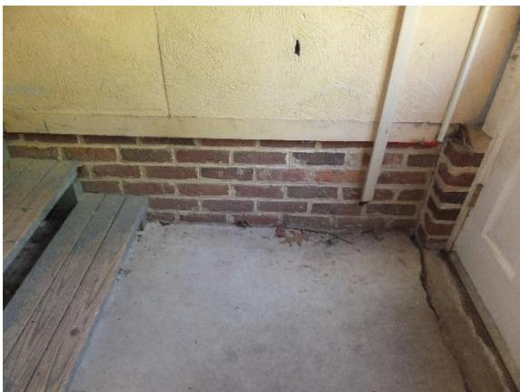
Figure 198. Brick foundation visible at the west wall of the garage.
