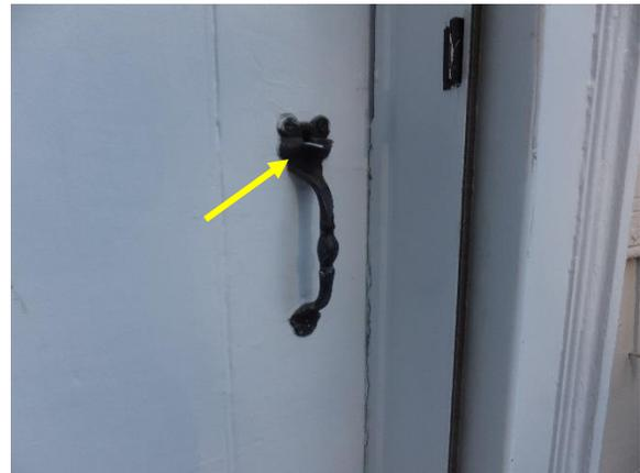
*Figure 63. Thumb latch at the exterior of the board and batten door.*
