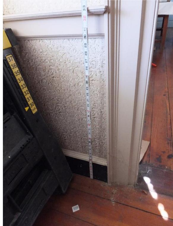
*Figure 131. View of typical chair rail and baseboard profiling and orientation throughout the majority of the house.*
