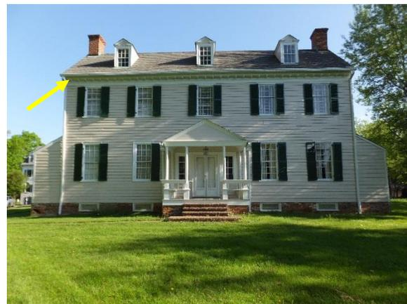
*Figure 49. View of the south facade in 2017 revealing 37 modillions with 8 dentils between each modillion along the cornice.*
