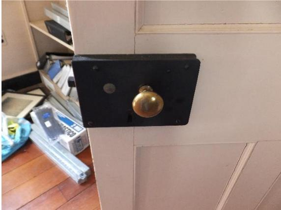
*Figure 142. Carpenter lock typically located on all prominent doors.*
