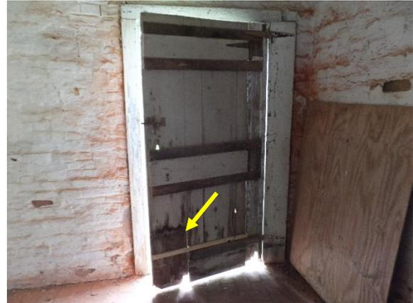
*Figure 296. Interior side of board and batten door reveals retrofits. Note the hinged section at the bottom left of door.*
