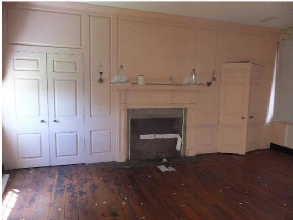
*Figure 216. Fireplace centered at fully paneled west wall. Note paneled closet (left) and contemporary bathroom (right) doors.*
