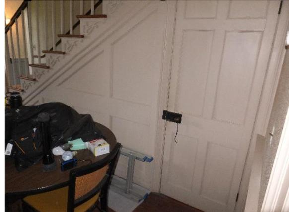
*Figure 135. Wood paneling below the treads and ornamentation tying into the paneling of the basement door.*
