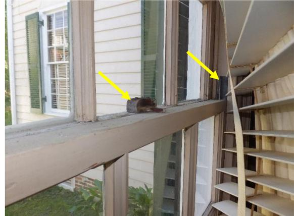
*Figure 55. Two-part interlocking weatherstripping at a window on the east facade. Note wood sash lock with pin.*
