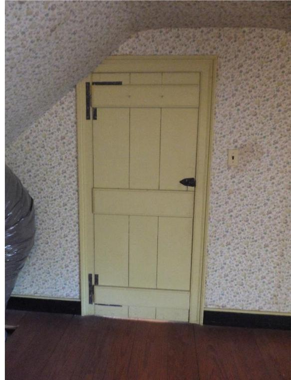
*Figure 237. Interior board and batten door to room 302.*
