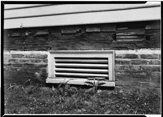
*Figure 30. Detailing of wood timber sill on top of the brick foundation with ventilation louver centered ca. 1960. (Photo courtesy of HABS),*
