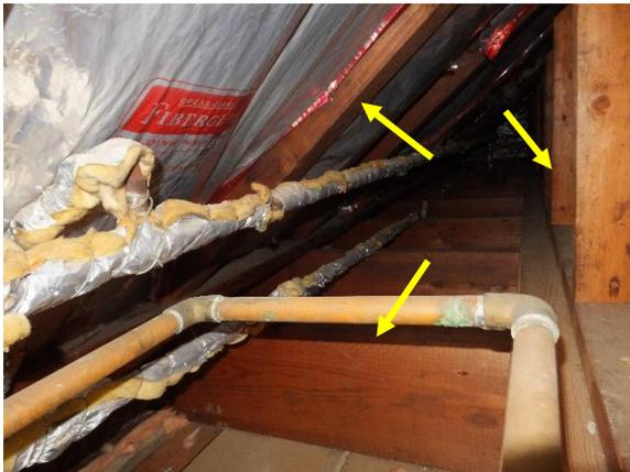
*Figure 242. View into the access hatch looking east reveals machine cut rafters, stud framing, and joists.*
