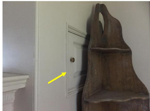
*Figure 147. Warming cupboard at the south face of the chimney.*
