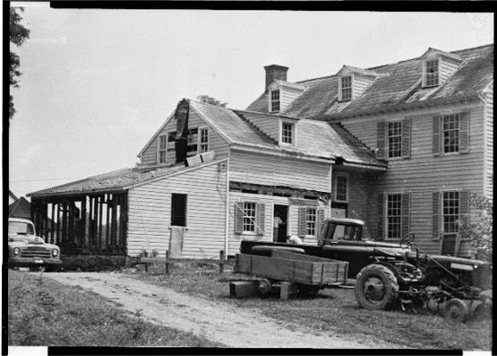
*Figure 34. View of the house from the northwest ca. 1960. Note restoration work underway and previous kitchen structure to the north (left). (Photo courtesy of HABS).*
