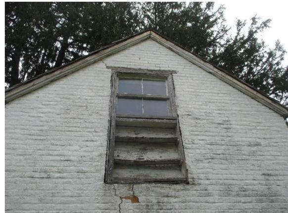
*Figure 290. 2/2 wood window at the second floor west facade with wood shelves below.*
