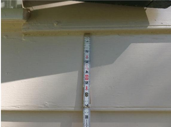
*Figure 43. Example of exposed weathering height of the beaded clapboard.*
