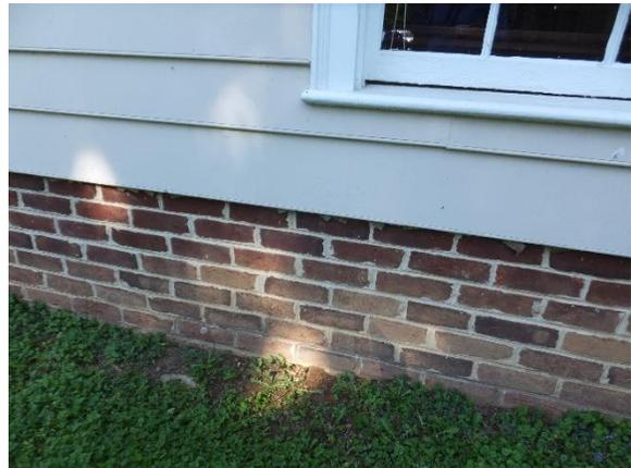
*Figure 46. Exposed brick at the garage addition with grapevine tooled mortar.*
