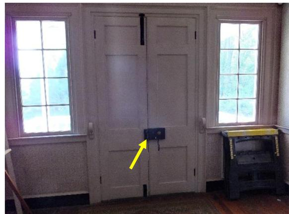
*Figure 59. Historic Carpenter's lock with barrel key still in place.*
