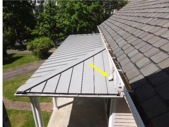
*Figure 51. West patio roof interface with central section of the home. Downspout from central section gutter deposits water directly onto patio roof.*
