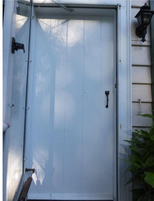
*Figure 61. Board and batten door at the east facade.*
