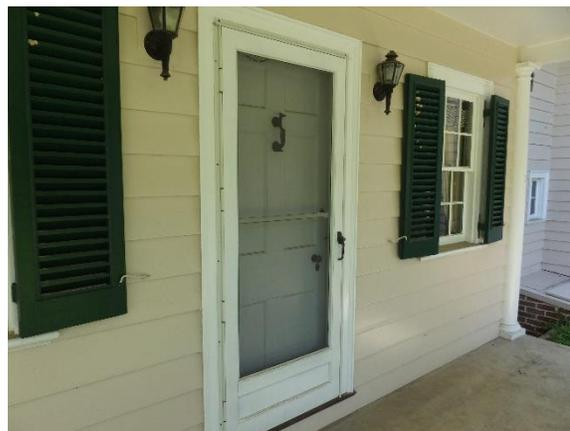
*Figure 67. Paneled exterior door at room 105, west facade.*
