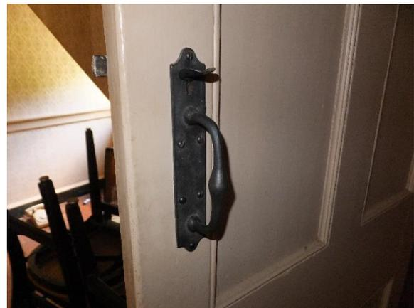
*Figure 177. Stair door has a thumb latch and door pull.*
