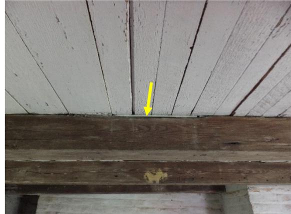
*Figure 318. Retrofit above floor beam and below second flooring.*
