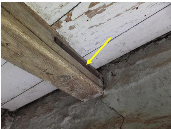
*Figure 315. Tie straps tying to star anchor plates at the exterior.*
