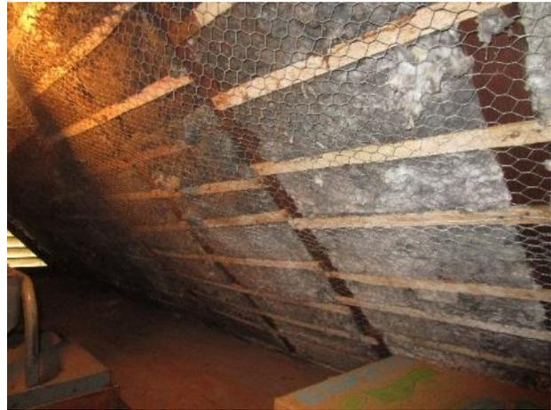
Figure 377. Loose fill insulation between the rafters is being held in place by chicken wire fastened to nailer boards.
