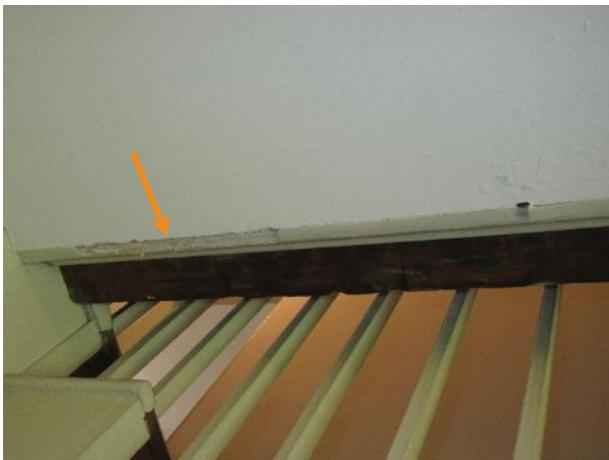
Figure 501. Missing section of wood molding along the stairwell.
