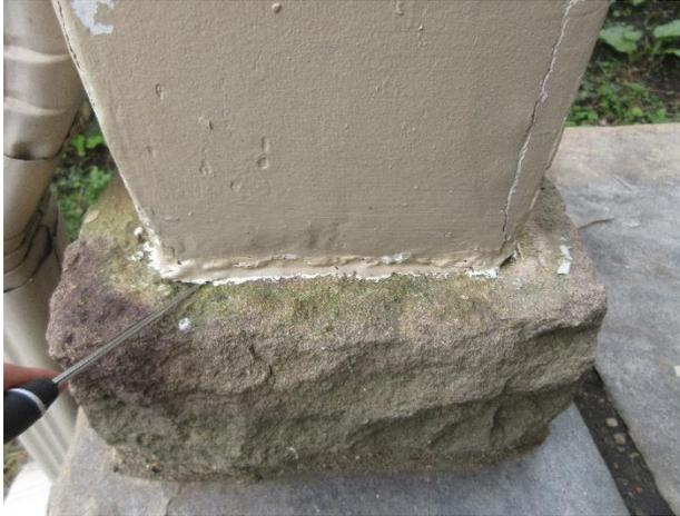
Figure 474. A small sealant fillet seal is in place at other north porch posts. The sealant joints typically had voids.
