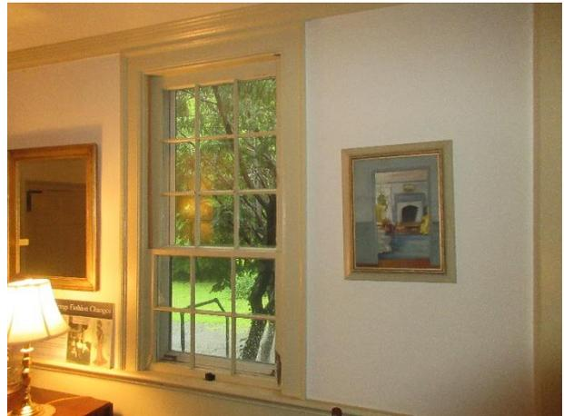
Figure 450. Dining room east window with missing and flaked paint and soft wood.
