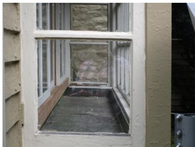
Figure 77. Copper lined planter box extends full length of garden bay window.
