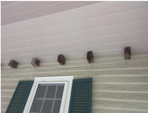
Figure 60. Second floor joists protrude beyond the clapboard, north porch.
