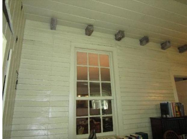
Figure 265. This north wall of the south enclosed porch was historically exposed to the exterior.
