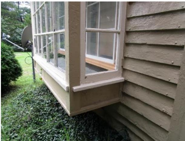
Figure 76. Copper lined planter box extends full length of garden bay window.
