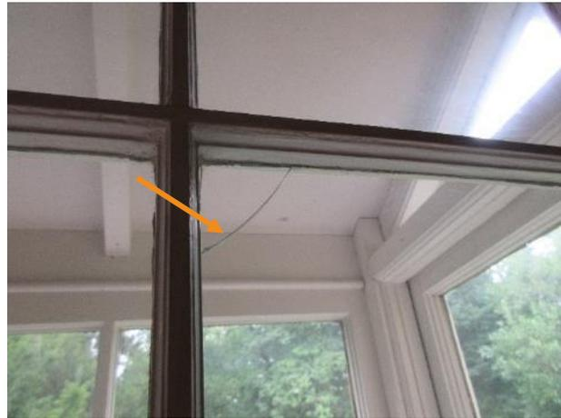
Figure 515. Cracked glazing lite at interior side of the garden window.
