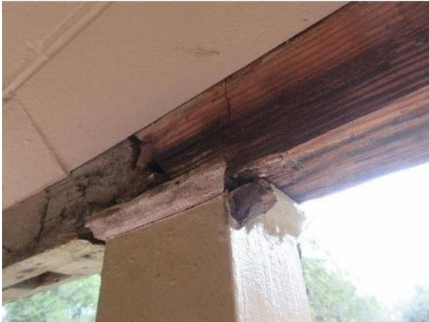
Figure 472. Soft and rotted wood found using a probe at the top of a north porch post.
