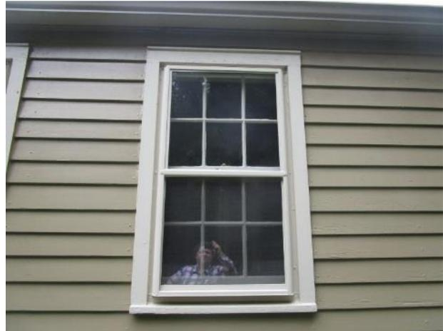
Figure 67. Typical 6/6 double hung wood window with no shutters, south enclosed porch.
