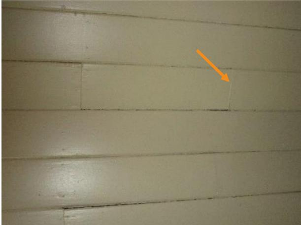
Figure 535. Separation between ceiling panels with one crack in the south enclosed porch.
