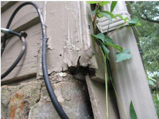
Figure 397. Wood section loss at the west corner of the south enclosed porch.
