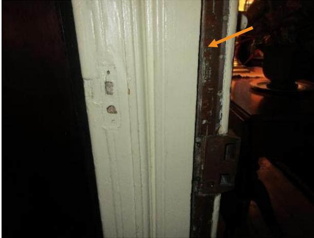
Figure 249. Copper weatherstripping along the door opening.
