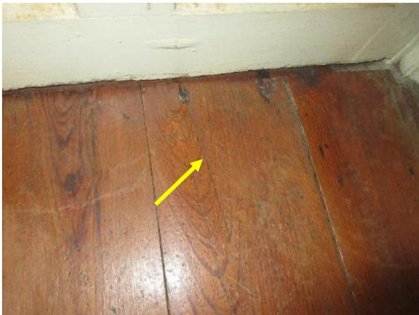
Figure 549. Crack in floorboard from fastener, closet shown.
