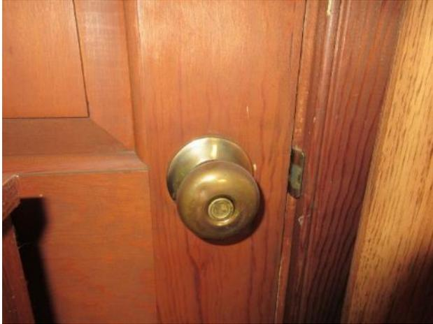
Figure 92. Interior view of non-historic brass hardware on study door, west addition.
