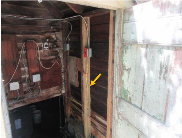
Figure 120. Contemporary 2x4 members sistered to vertical framing on north wall.
