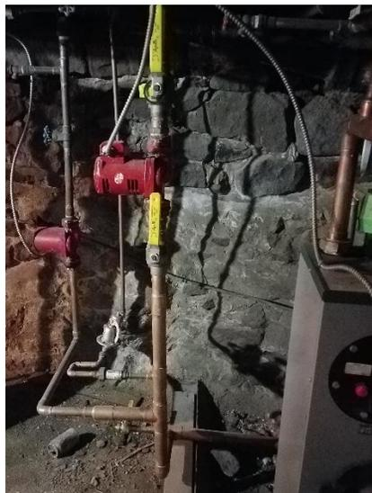
Photo 8: No piping insulation.
