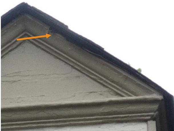
Figure 401. Section of wood section loss at a dormer pediment, north facade.
