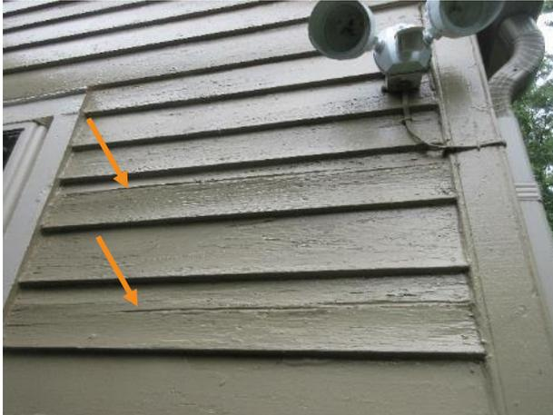
Figure 387. Clapboards with end splits extending longitudinally in the boards that have been painted over.
