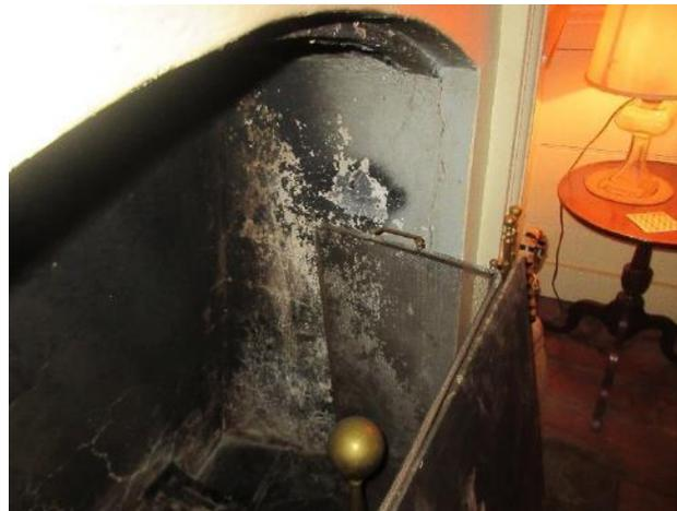
Figure 256. Firebox is lined with a cementitious coating.
