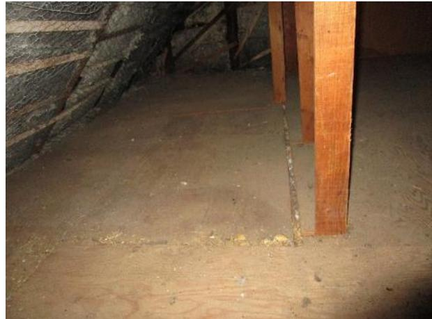
Figure 381. Plywood sheathing covering joists to provide walking surface.
