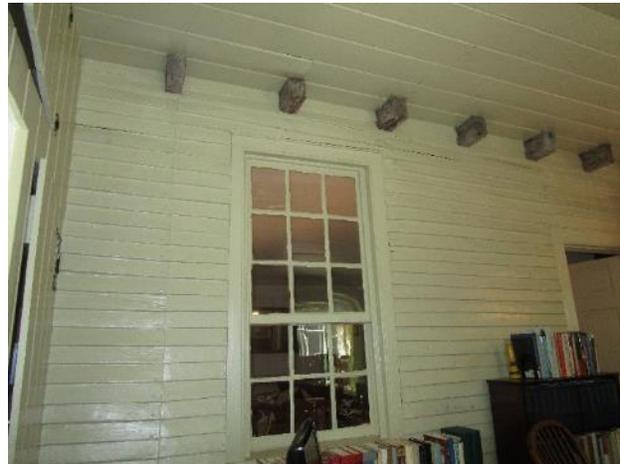
Figure 279. Typical 9/6 window at the north wall of the south enclosed porch. Note exposed joists at the ceiling.
