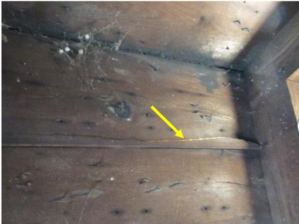
Figure 539. Longitudinal crack along wood paneling in the cellar access.
