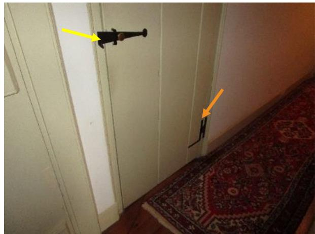
Figure 347. Closet door has a bar latch (yellow arrow) and typical HL-hinges (orange arrow).
