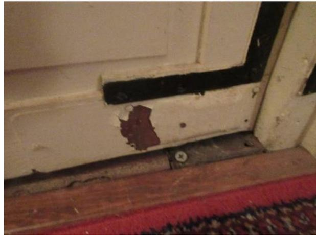
Figure 519. Peeling paint at the base of the kitchen door.
