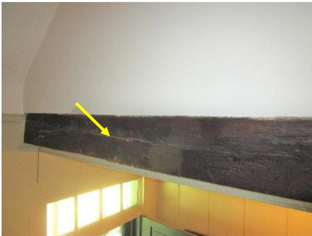
Figure 541. Season check along the exposed timber in the stairwell.
