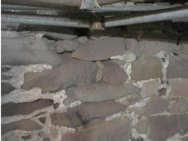
Figure 506. Crumbling and missing sections of mortar in the stone foundation wall.
