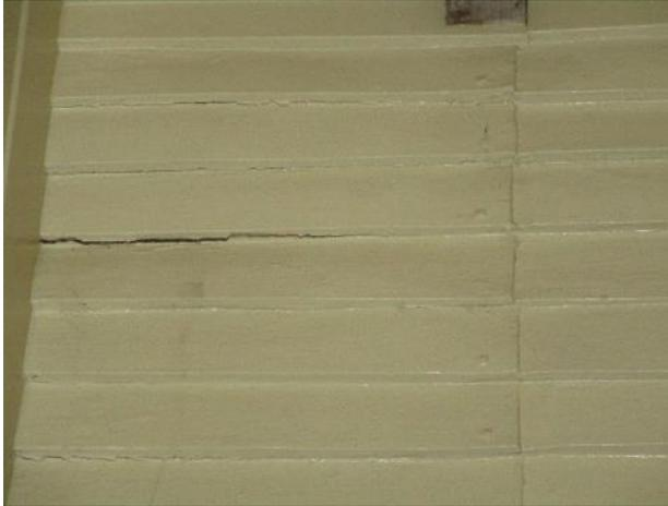
Figure 264. The south enclosed porch features the historic clapboard with rose head nails along the north wall.
