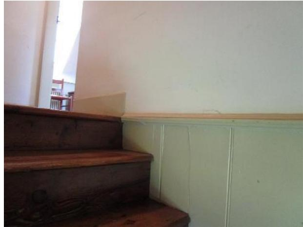
Figure 179. The staircase is lined with the typical wall paneling, which terminates at the top step. Plaster extends from the paneling to the ceiling.
