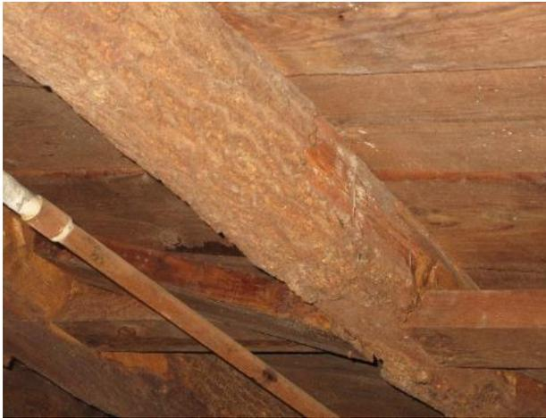
Figure 158. Log joists with cross bracing.
