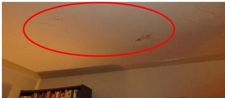
Photo 1: Water damage from leaking water closet wax seal on the second floor. The wax seal has been replaced and the water closet is no longer leaking.
