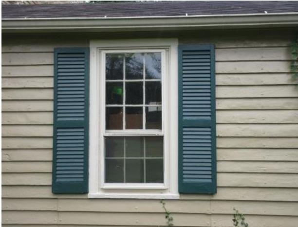
Figure 70. Typical 9/6 double hung wood window, west addition.
