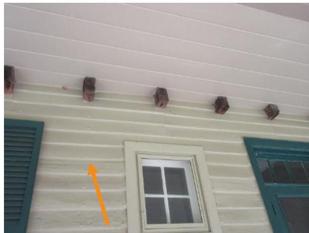
Figure 48. Wood dutchman section of clapboards, north porch roof.
