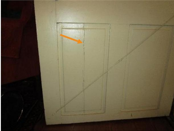
Figure 522. Crack full height of a door panel at the living room to south enclosed porch door.
