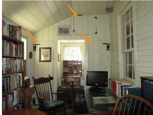
Figure 277. Several closets located along the west wall of the enclosed porch of similar construction at the wall paneling.
