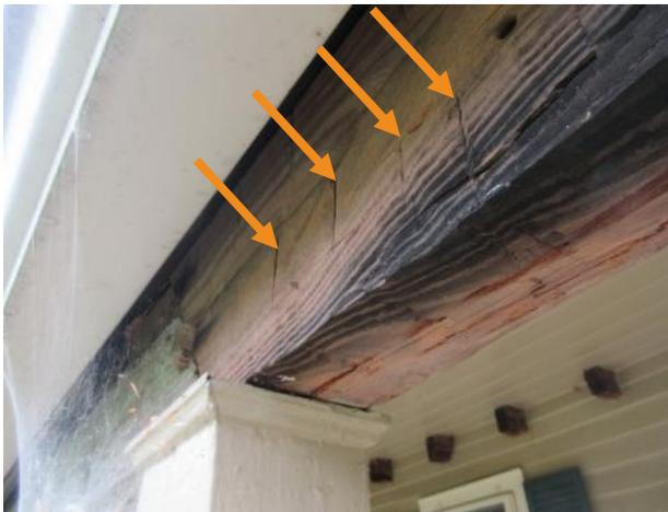
Figure 110. Adze marks on replacement beam(arrows).
