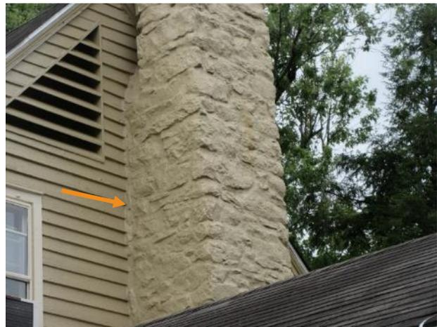
Figure 98. No metal flashings were visible at west chimney-to-clapboard interface.
