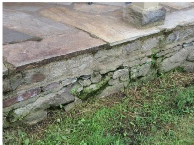
Figure 404. Missing sections of mortar at the north porch.
