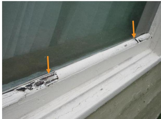
Figure 440. Paint is missing in sections and wood stop has deteriorated wood where exposed.
