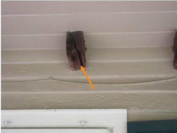
Figure 399. Wood section loss at an exposed wood joist, north facade.
