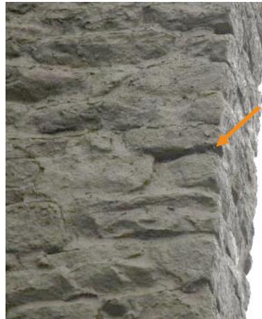
Figure 465. Missing section of mortar at the east chimney.
