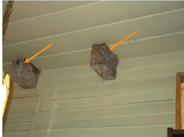
Figure 273. Exposed floor joists are visible through the enclosed porch, similar to the north porch.
