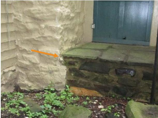
Figure 407. Mortar bondline failure at the interface between the east chimney and kitchen landing.
