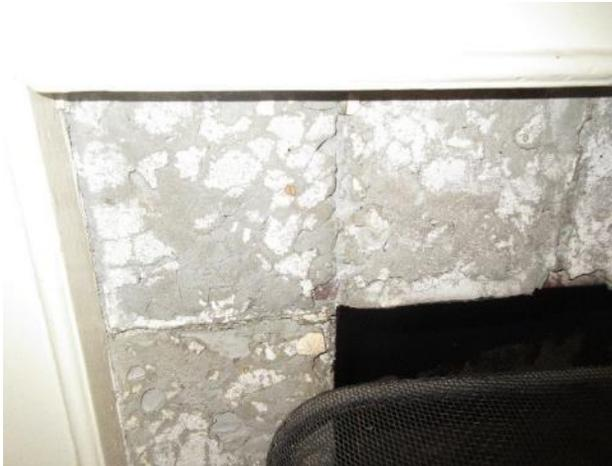
Figure 226. Tiles at the firebox surround have been removed.
