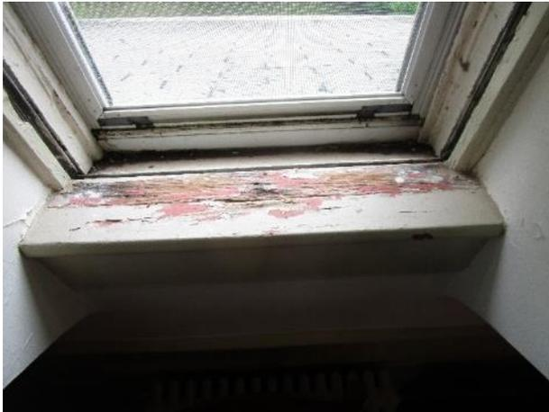
Figure 449. Missing paint with deteriorated wood where exposed at an interior stool, north dormer in guest bedroom.
