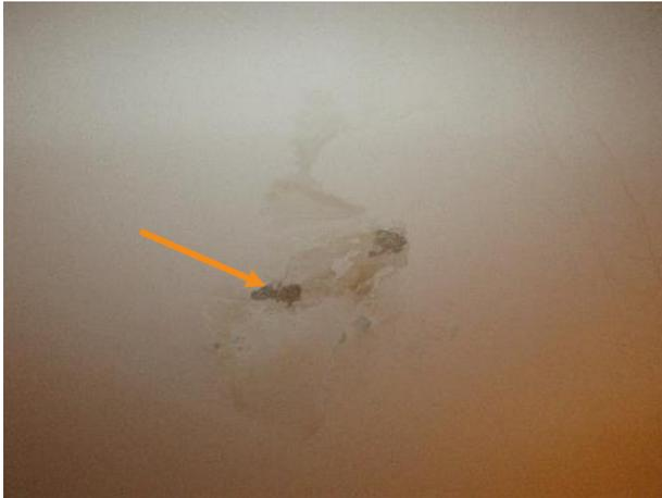
Figure 499. Area of blistered and stained plaster ceiling, living room shown.
