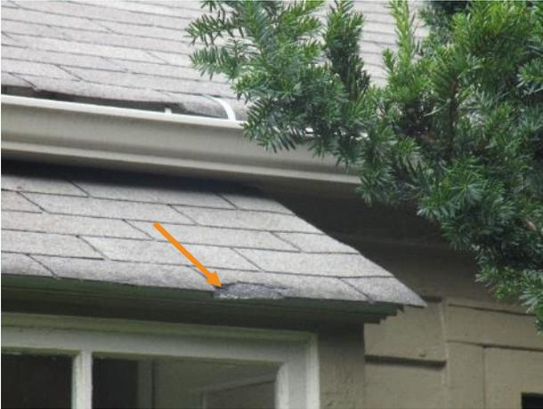
Figure 427. Broken shingle above garden window.
