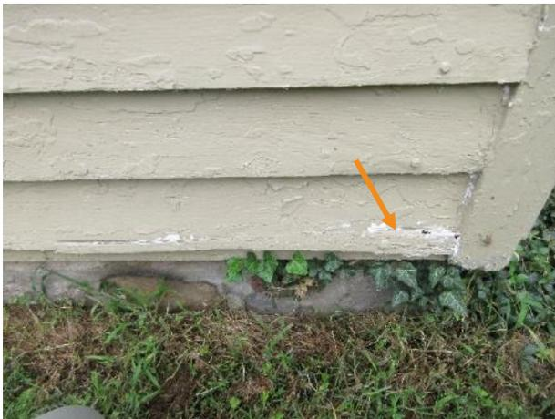
Figure 389. Previously repaired end split at the lowest clapboard at the west addition.
