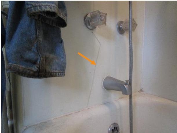
Figure 487. Several of the large shower tiles were cracked.
