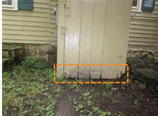
Figure 459. Wood section loss at the base of the cellar access door.
