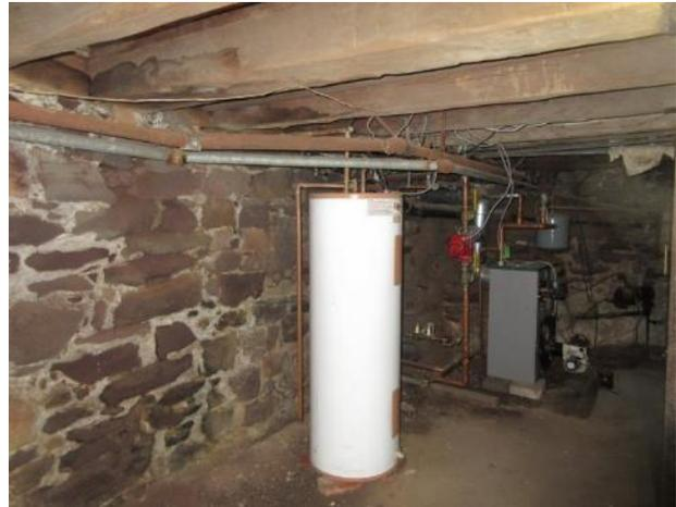
Figure 127. A water heater and furnace are installed in the northeast corner.
