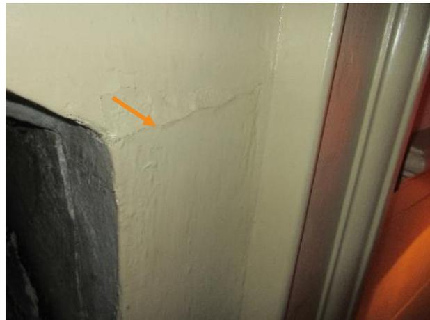
Figure 488. Crack, possible at a cold joint, of the cementitious crack at the living room fireplace.
