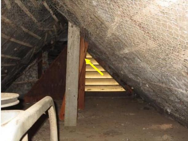
Figure 378. One of the north vertical rafter supports was observed to be out of plumb.
