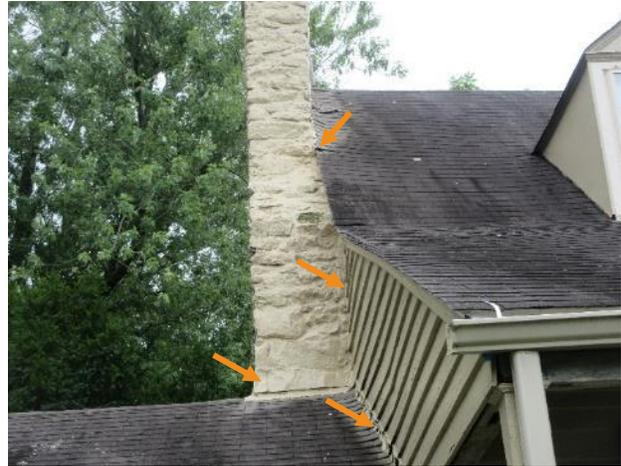
Figure 96. Painted metal flashings at the east chimney to the house clapboards and roof sections.
