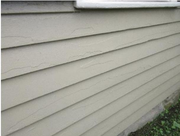
Figure 435. Paint has been applied over previous coating(s).
