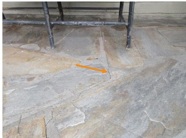
Figure 410. Full depth crack in mortar at the north porch.
