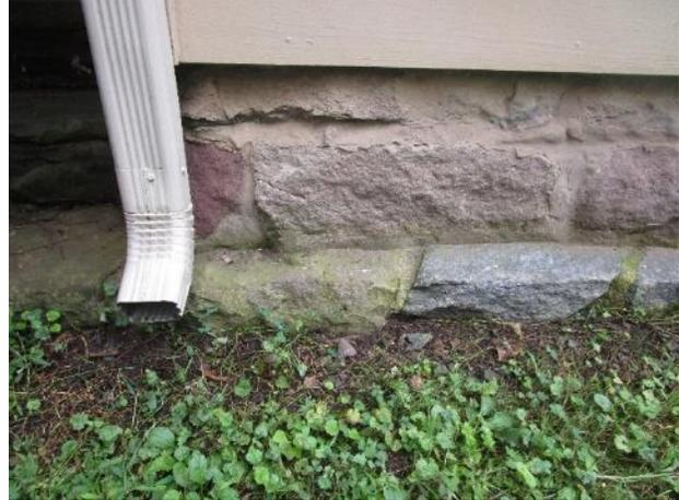
Figure 412. Biological staining on foundation stones adjacent to a downspout.
