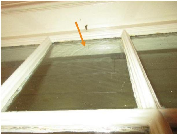
Figure 251. Glass lites at the south living room window appears indicative of crown glass with circular patterns.
