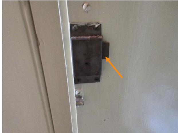
Figure 171. Interior view of cabinet hardware. The knob at the exterior would have been turned to activate the spring latch. This piece may also be installed opposite as protruding latch on the right would have engaged in a keep on the wall side (left).
