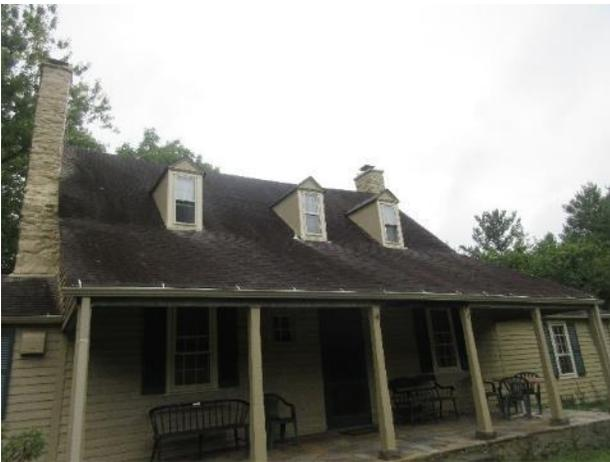
Figure 429. Typical dark staining on the north roof.
