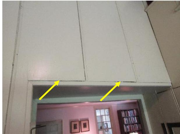
Figure 546. Cupped wood paneling in the hallway.
