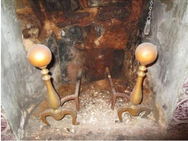
Figure 362. Stone firebox with parged sides. Two large brass andirons are located within the firebox.
