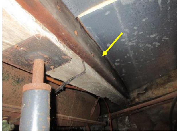
Figure 544. Sistered joist in the cellar.
