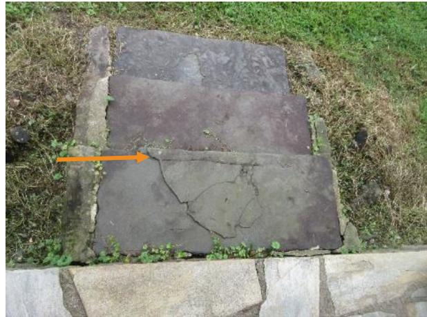
Figure 416. Scaling of stone unit at steps to the north porch.
