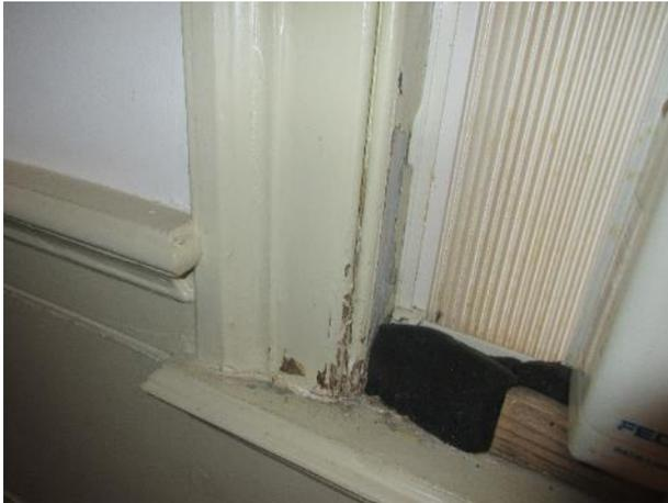
Figure 451. Missing paint at jamb trim with soft wood, living room west window.
