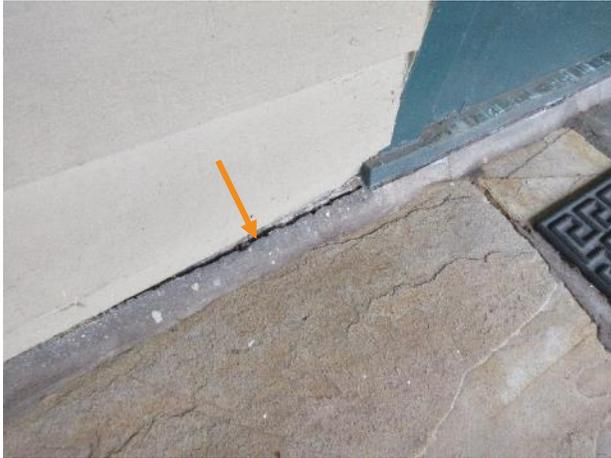
Figure 411. Separation of mortar along the wood clapboard and flagstone paver joint.
