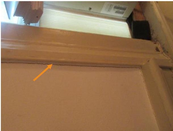
Figure 481. Typical cracking below wood window trim, living room shown.
