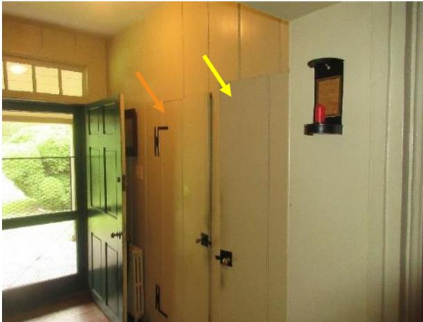
Figure 168. Doors leading to the powder room (orange arrow) and kitchen (yellow arrow) are typical board and batten doors with HL-hinges and bar latch hardware.
