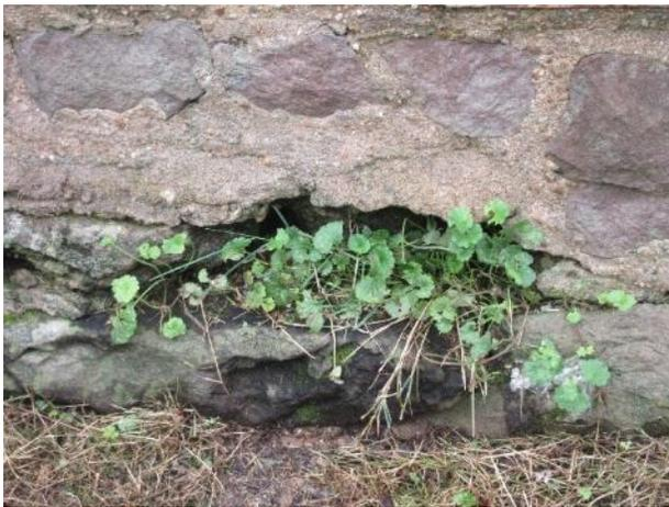
Figure 403. Missing mortar at the stone foundation with vegetative growth.
