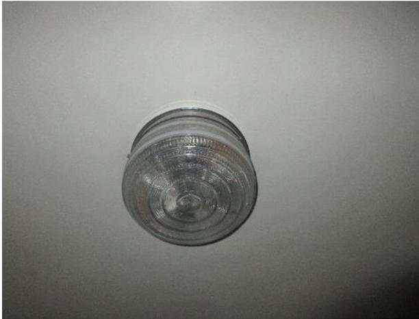
Figure 208. Typical ribbed ceiling mounted light fixture in the original section of the kitchen.
