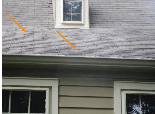
Figure 424. Displaced asphalt shingles, view from south.
