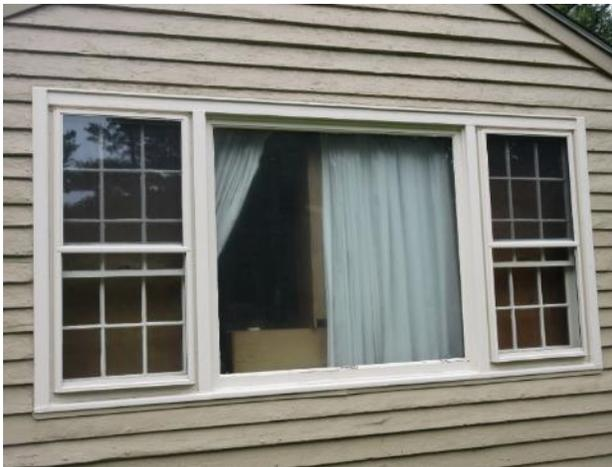
Figure 72. Picture window flanked by two 9/6 hung windows, west facade, west addition.
