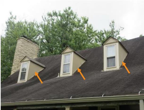
Figure 82. September 1, 2020 side view of dormers. Note flat surface of material.
