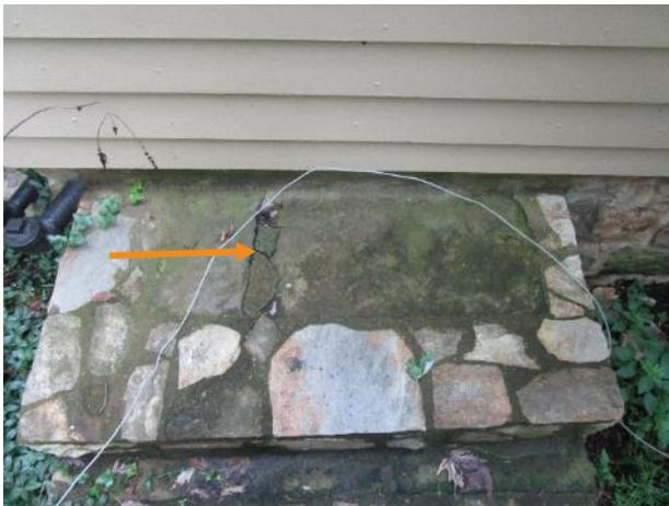
Figure 417. Weathering of stone units at abandoned steps to the south enclosed porch.
