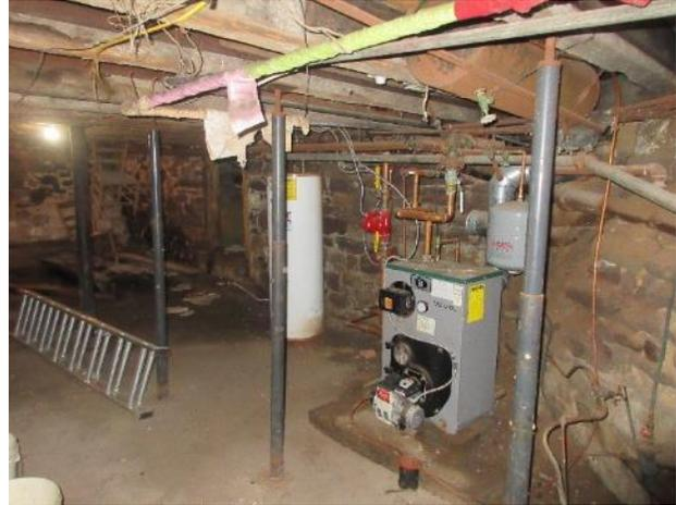
Figure 149. Looking north into the cellar from the access stairs. Furnace is installed atop a concrete pad.
