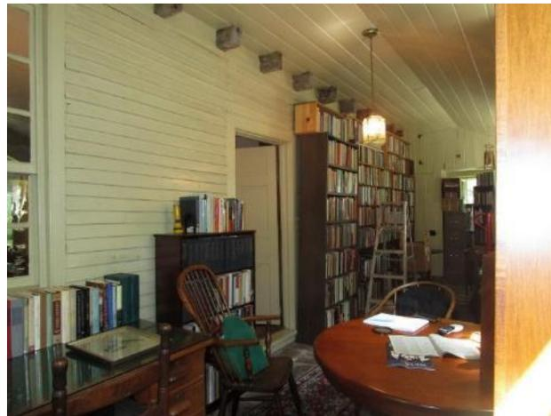
Figure 61. Second floor joists protrude beyond the clapboard, south enclosed porch.
