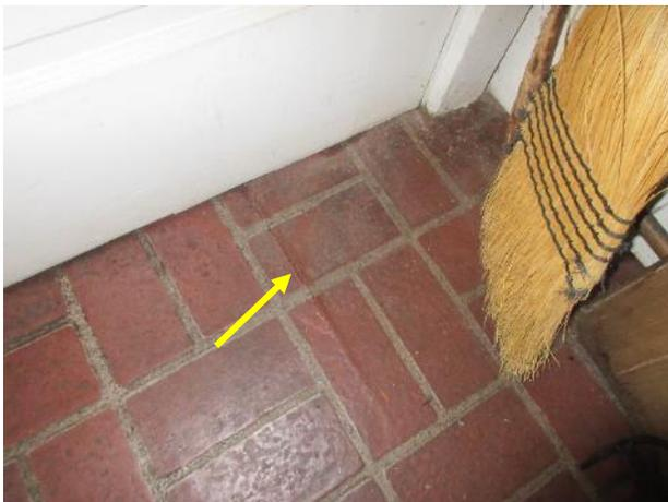
Figure 551. Crack in brick flooring of the kitchen.
