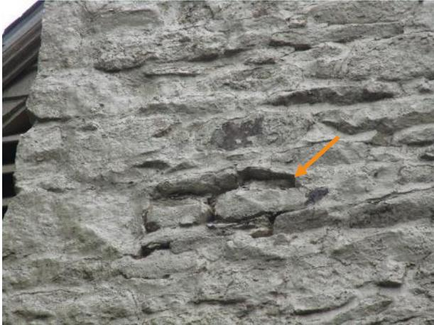
Figure 466. Section of recessed or missing mortar at the west chimney.
