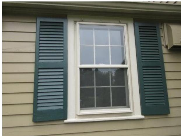
Figure 69. Typical 6/6 double hung wood window, east kitchen addition.
