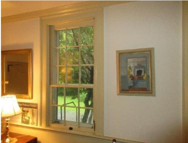
Figure 228. View at east wall of dining room with typical 9/6 window.
