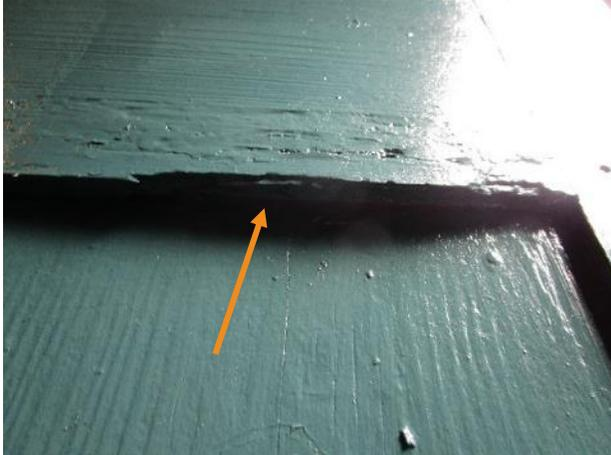
Figure 454. Separation between a lower panel and middle rail of the south enclosed porch door.
