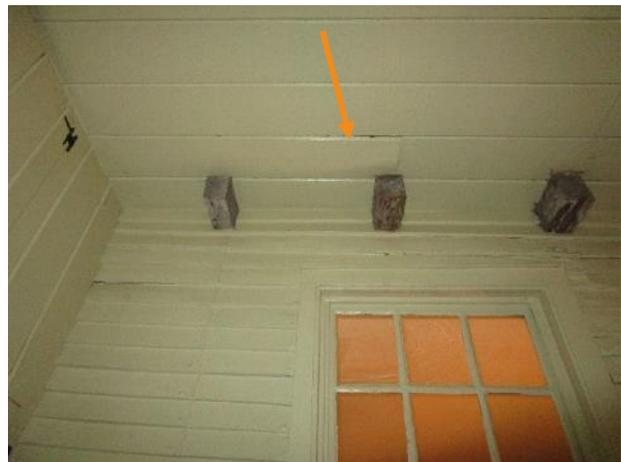
Figure 530. Displaced wood panel at the ceiling above the exposed joists.
