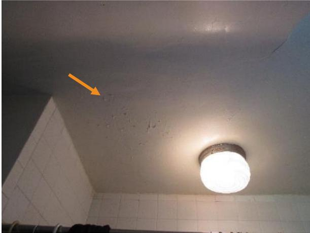
Figure 483. Blistered paint above the master bathroom shower
