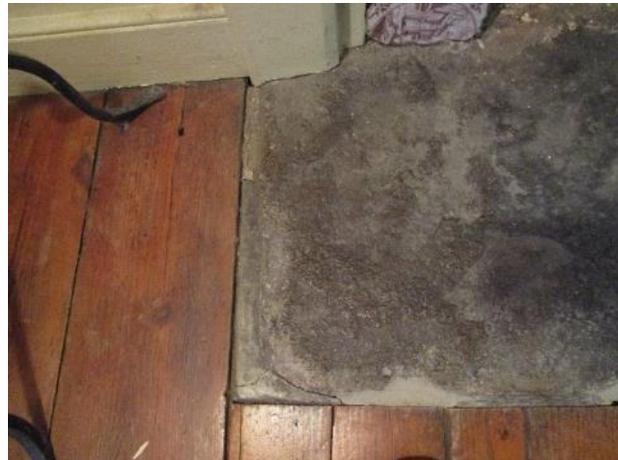
Figure 513. Crack in mortar at the bedroom fireplace hearth.
