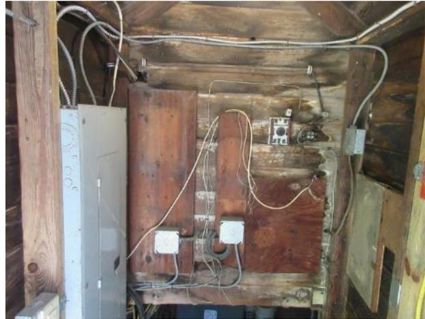
Figure 121. Electrical penetrations feed between house and cellar.
