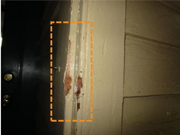
Figure 458. The east addition screen door is racked within the opening causing this impact damage to the trim.
