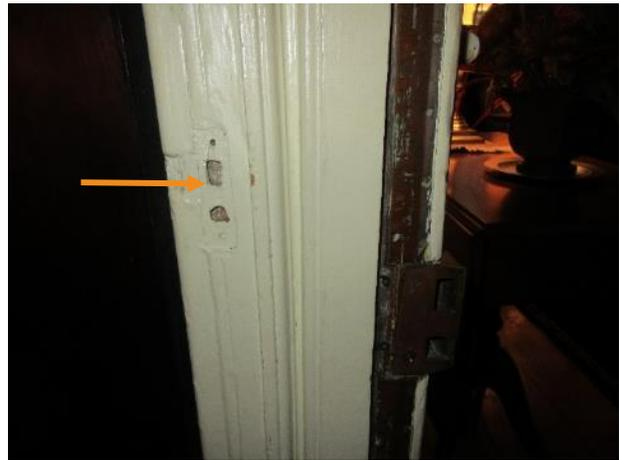
Figure 261. Evidence of a previously removed screen/storm door as chiseled section of latch strike remains on the south enclosed porch side.
