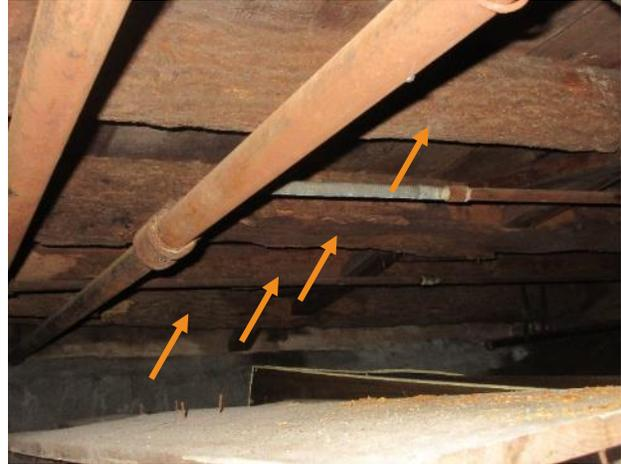
Figure 157. Westernmost floor joists in the crawl space still have bark on the log.
