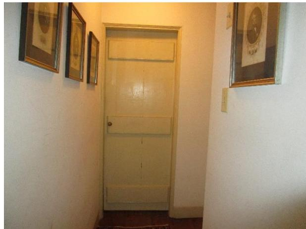
Figure 517. Door between the second floor hallway and guest bedroom doesn't fully close.
