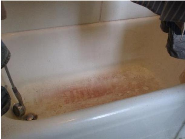
Figure 553. Staining within the master bathroom shower.
