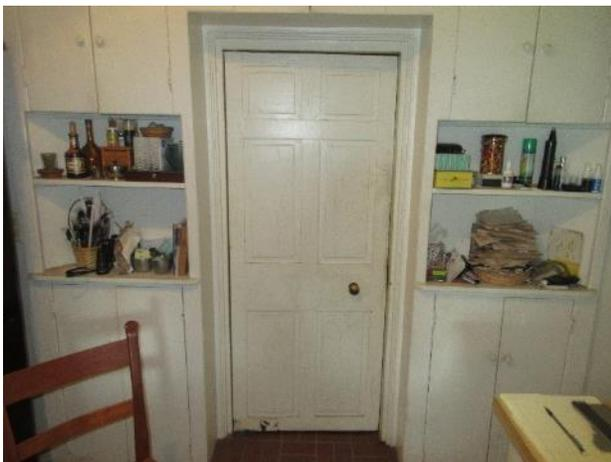
Figure 516. Door between the kitchen and dining room doesn't fully close.
