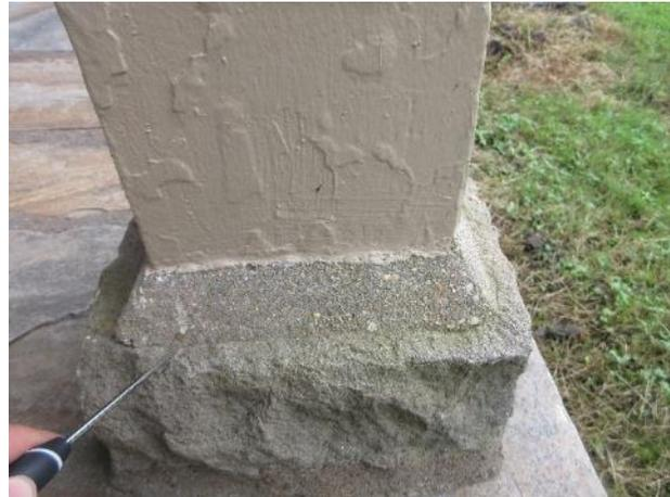
Figure 473. A sloped mortar wash exists on several north porch posts.
