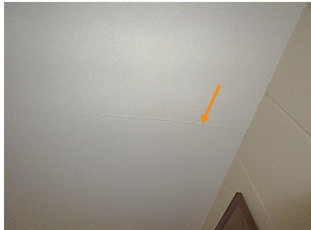
Figure 478. Typical cracking in the plaster ceiling-to-wall interface, guest bedroom shown.
