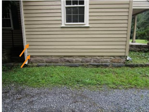
Figure 50. Wood replacement clapboards, kitchen addition at east facade.
