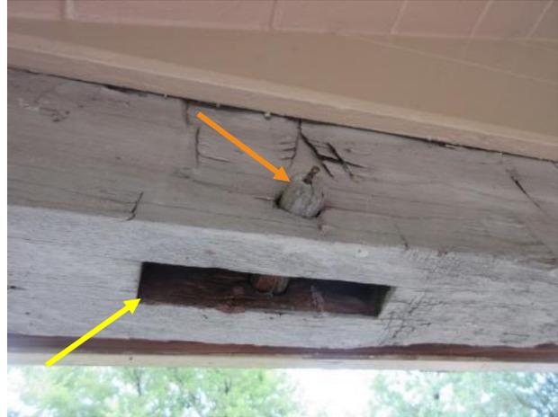
Figure 113. Close-up bottom view of end joist. Note notch (yellow arrow) and wood dowel (orange arrow) for mortise and tenon connections.
