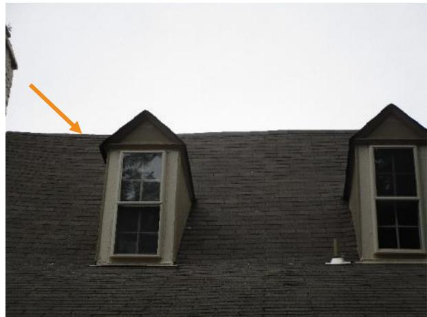
Figure 420. Sag at roof ridge, view from south.
