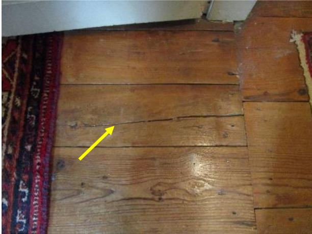
Figure 547. Crack in a floorboard at the guest room.
