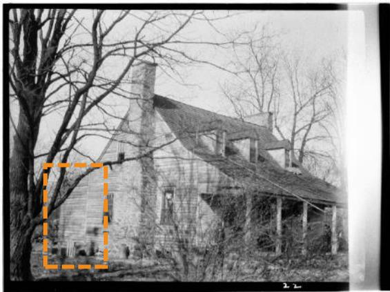
Figure 43. HABS photograph taken prior to Detwiler's restoration that shows clapboards at the north enclosure.
