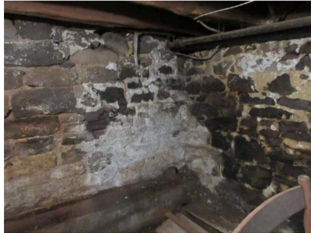
Figure 125. White coating remnant on cellar walls.
