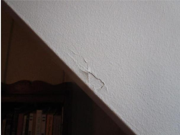
Figure 475. Typical blistered and cracked plaster at dormer wall, guest bedroom shown.
