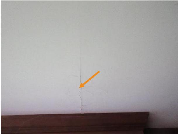
Figure 479. Typical cracking above wood trim, sitting room shown.
