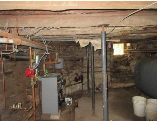
Figure 142. Four joists are supported by metal scaffold jacks.
