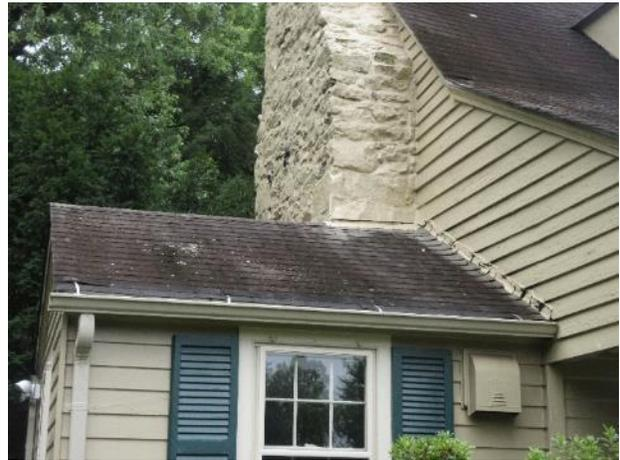
Figure 428. Typical dark staining on the north roof, east addition.
