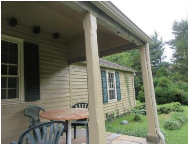
Figure 106. Posts have beveled edges that taper from top and transition to wider base.
