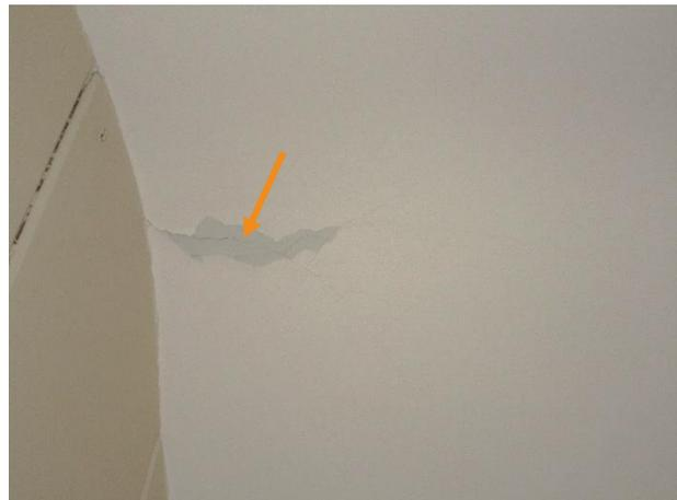
Figure 476. Typical cracking in the plaster ceiling-to-wall interface, guest bedroom shown.
