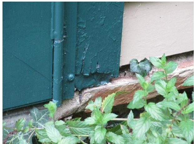
Figure 398. Wood section loss at the bottom of the south enclosed door trim.
