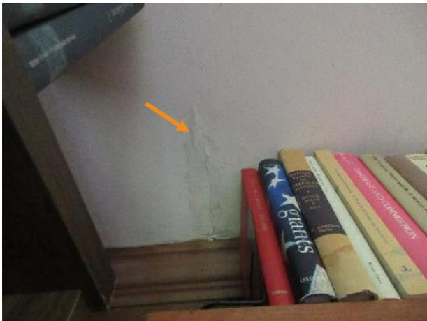
Figure 489. Crack in plaster with water staining at the east wall of the sitting room, possibly indicating an active source of water infiltration.
