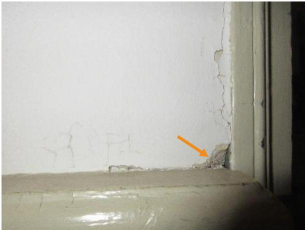
Figure 485. Section of plaster spalls above the chair rail in the dining room.
