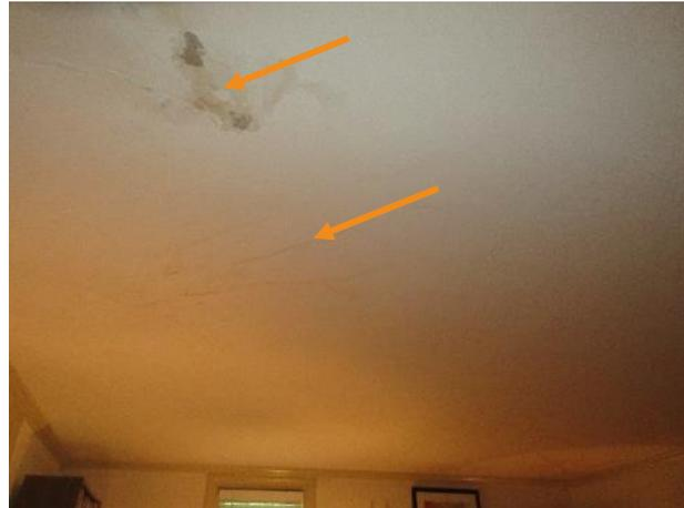
Figure 500. Area of blistered and stained plaster ceiling, living room shown.
