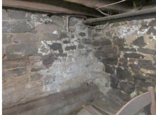
Figure 507. Area of repointing with a white coating at the foundation wall.
