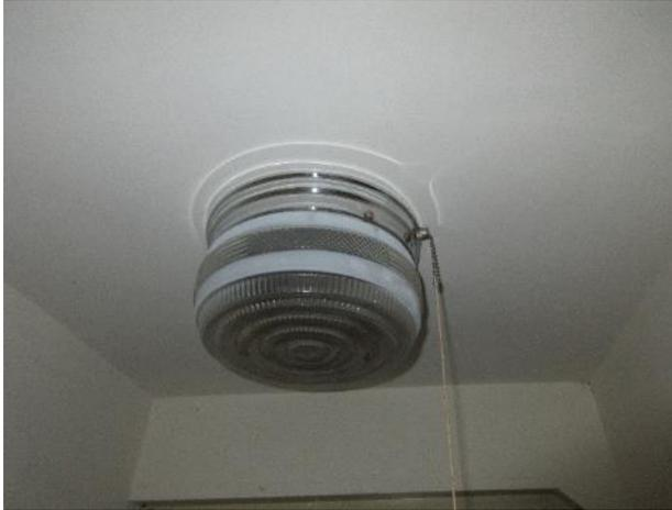
Figure 186. Ribbed ceiling mounted light fixture in the closet.
