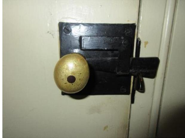
Figure 187. Typical bar latch hardware that is knob activated.
