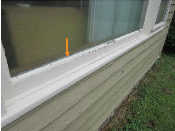
Figure 439. Wood glazing stop at the picture window, west addition.
