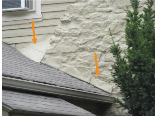
Figure 59. Asphaltic shingles and painted metal flashings (arrows) at roof.
