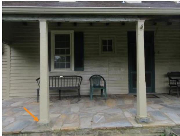
Figure 107. Posts are set on top of stone blocks. Note post at left has sloped mortar wash added along base.
