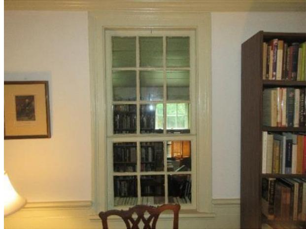
Figure 250. A typical 9/6 is located at the south wall of the dining room that used to be exposed to the exterior until the south porch was enclosed.
