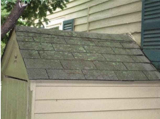
Figure 431. Typical biogrowth on the north roof, cellar access.
