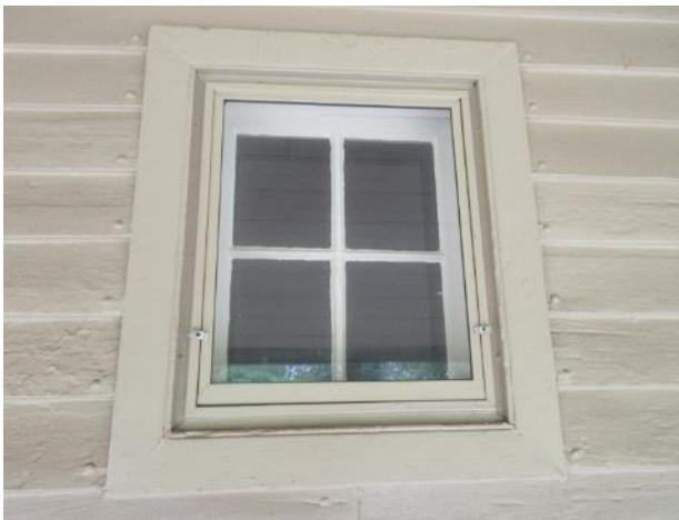
Figure 68. 4-lite casement window, east of north entry door.
