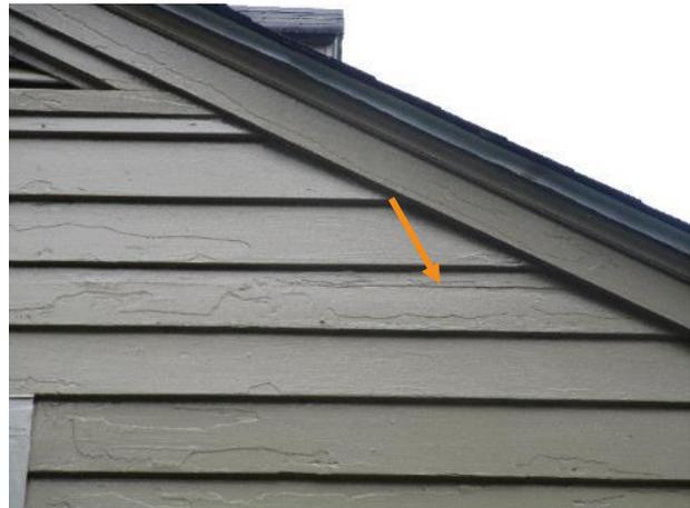
Figure 388. Typical end split in clapboards.
