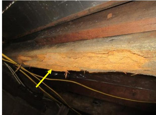
Figure 524. Typical insect damage along the bottoms of the exposed joists in the cellar.
