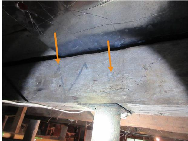
Figure 145. Markings observed on a hand hewn joist in the cellar.
