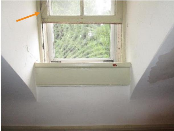
Figure 325. A rotating piece of wood on the sash sits into a slot along the jamb side of the sash channel to hold the window in the open position.
