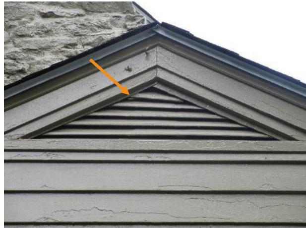
Figure 402. Displaced slat at the east addition louver.
