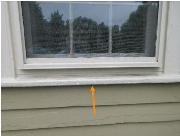
Figure 441. Soft section of wood below sill of east addition, north facade.
