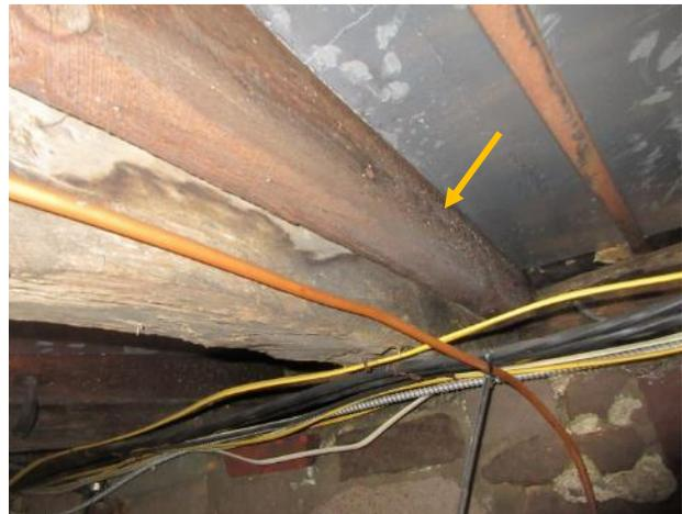
Figure 139. Contemporary sistered joist.
