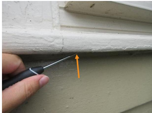
Figure 442. Soft section of wood below sill of east addition, north facade.
