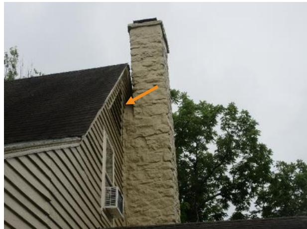
Figure 434. No visible flashings between the west chimney and house.
