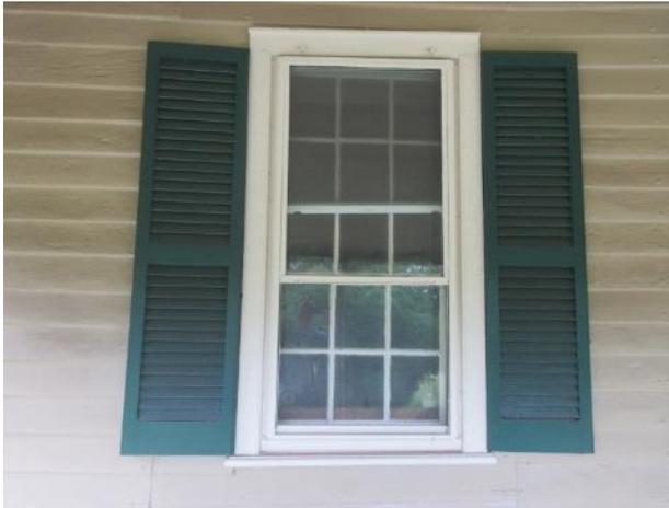
Figure 66. Typical 9/6 double hung window with wood slatted wood shutters, first floor, original section of house.
