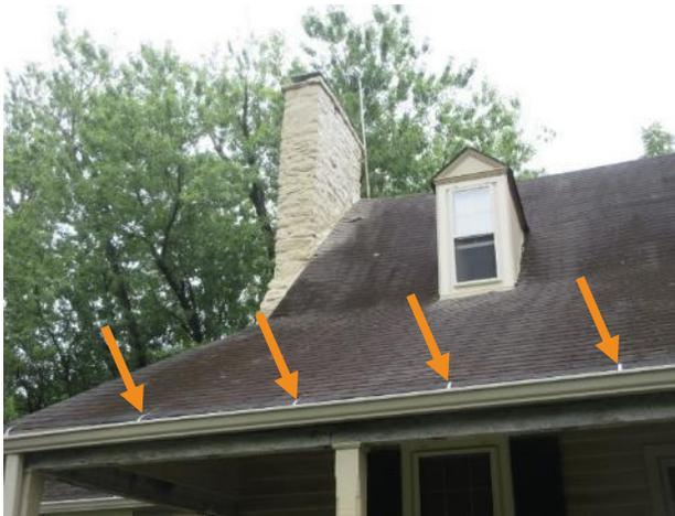
Figure 64. Gutter mounting brackets (arrows) at shingle surface.
