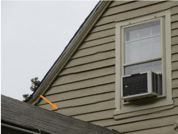
Figure 395. Isolated wood section loss at the west facade.
