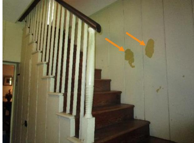
Figure 492. Typical peeling or missing tan paint at wood paneling in the stairwell, revealing a yellow undercoat.
