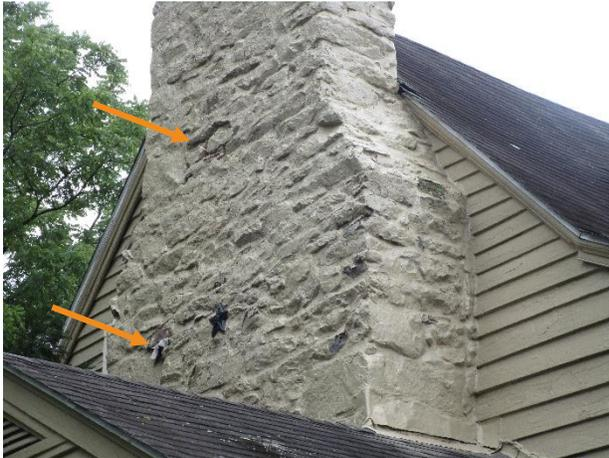
Figure 462. Typical peeling and cracking paint at the chimneys, east chimney shown.
