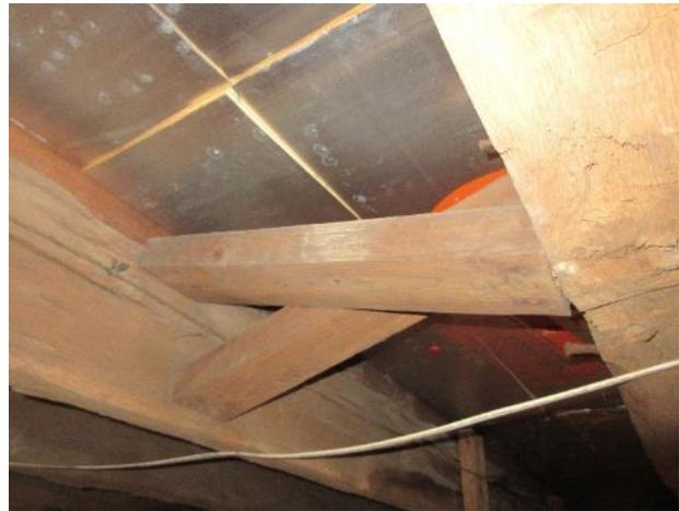
Figure 143. Cross bracing has been installed between several joists.
