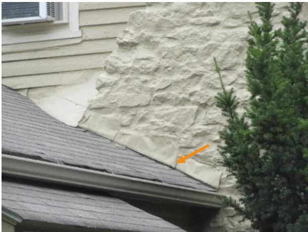
Figure 433. Unsealed laps of metal flashing between house and east addition.
