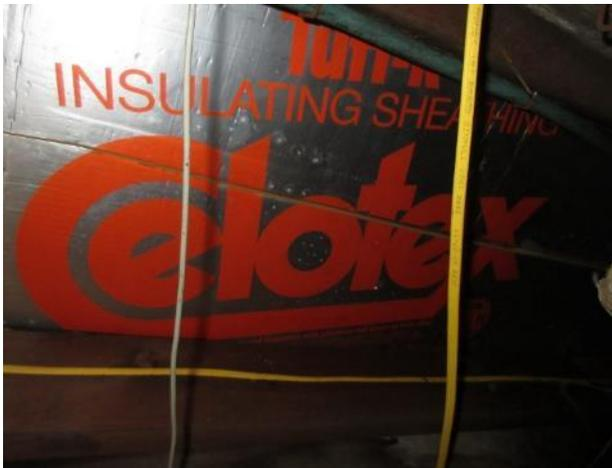
Figure 146. Celotex insulating sheathing installed below the floor boards, between joists.
