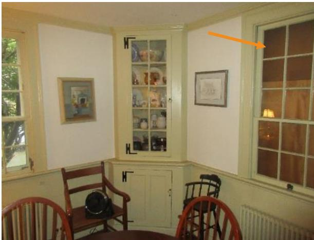
Figure 230. View southeast to original corner cabinet. Note previous exterior south window that is covered with a bookshelf at the south enclosed porch.
