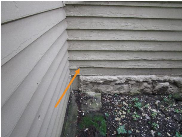
Figure 393. Isolated wood section loss at the east facade, to the north of the cellar access.
