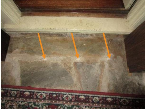
Figure 531. Filled mortar holes at the south enclosed porch from previous termite treatment.
