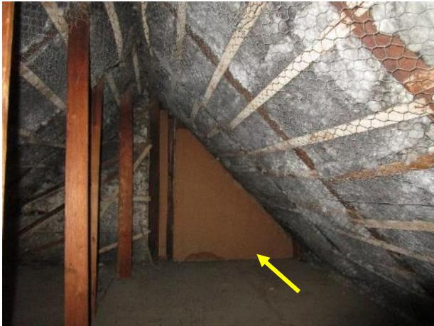
Figure 380. Gable vent on the east was closed with a similar hinged plywood door.
