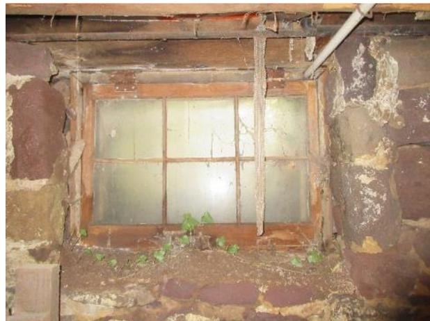
Figure 505. Vegetation growing into the cellar space from the west wall window. This window was not visible from the exterior.
