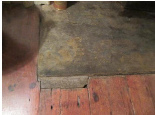
Figure 509. Cracked mortar at the stone hearth of the living room fireplace.
