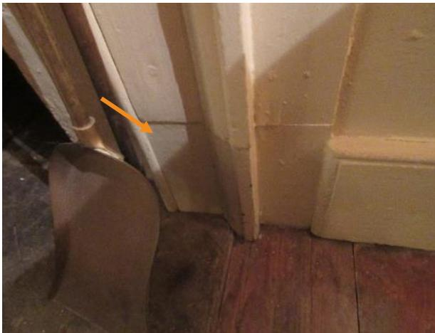
Figure 255. Wood dutchman observed at the base of the fireplace mantel legs.
