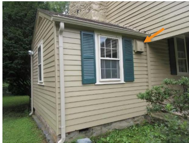
Figure 46. Oven vent (arrow) protruding west of window at north facade, east addition.
