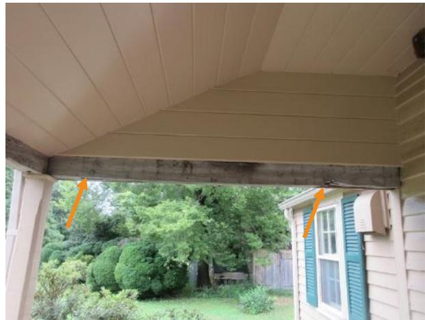
Figure 111. East end joist has widely spaced notches on bottom side. See Figure 113.
