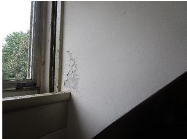
Figure 482. Blistered plaster at a dormer window, master bedroom shown.
