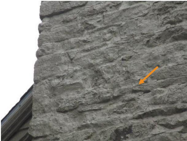
Figure 464. Typical bondline failure of mortar joints at chimneys, west chimney shown.
