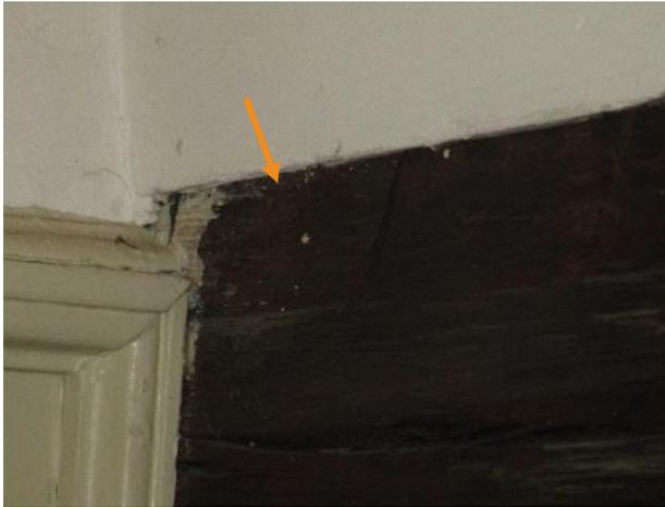
Figure 174. Exposed timber beam along the staircase. This north end has a partial dutchman.
