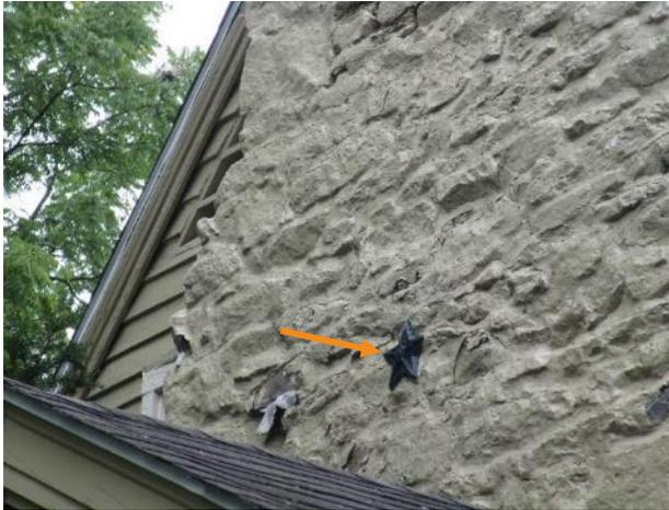
Figure 95. Black painted star faced tie rod, east chimney.
