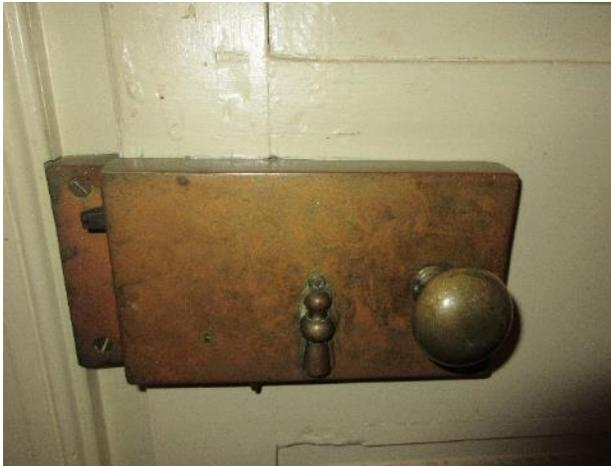
Figure 222. Large brass rim lock located at the dining room side of the door connecting to the kitchen.
