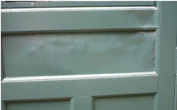
Figure 456. Denting in south enclosed porch storm door.
