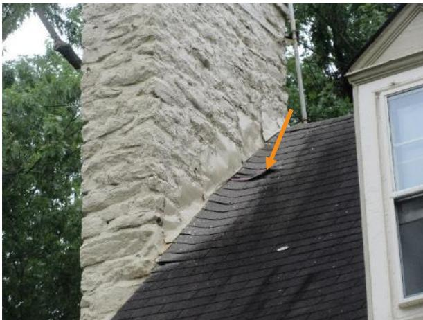
Figure 425. Displaced asphalt shingles at chimney flashing, view from north.
