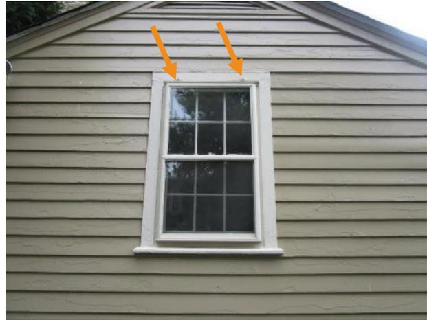
Figure 71. Hasps at top of window (arrows) indicate shutters may have been removed, east window, east addition.
