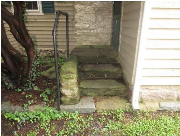
Figure 413. Biological staining on the kitchen steps and landing. Note adjacent tree, which overhangs this area.
