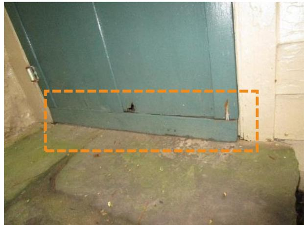
Figure 457. Wood section loss at the base of the east addition screen door.
