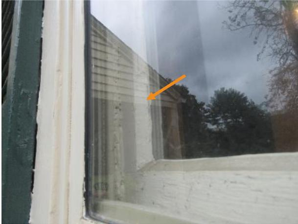
Figure 447. Cracked section of glazing putty at a north facade window. Storm windows are in place at this window.
