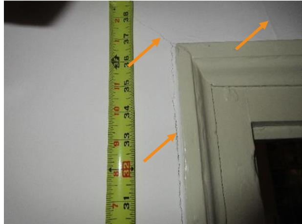
Figure 480. Typical cracking in plaster around and above door and trim, living room shown.
