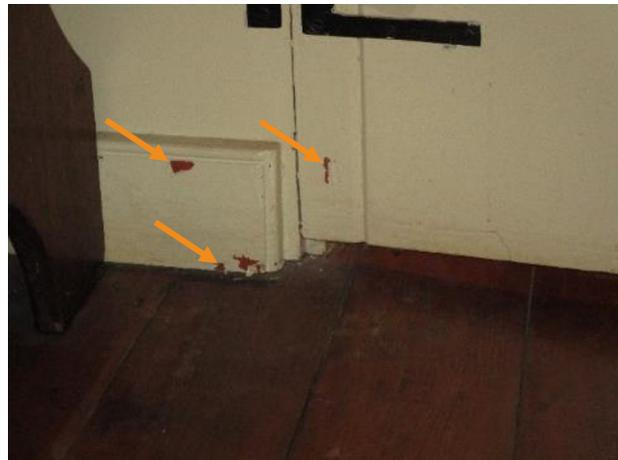
Figure 490. Typical peeling or missing tan paint at wood elements, revealing a red undercoat.
