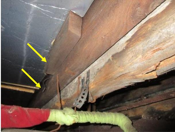
Figure 543. Partial sistering at a floor joist in the cellar.
