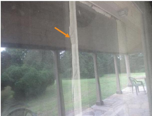
Figure 445. Cracked section of glazing putty at a north facade window. Storm windows are in place at this window.
