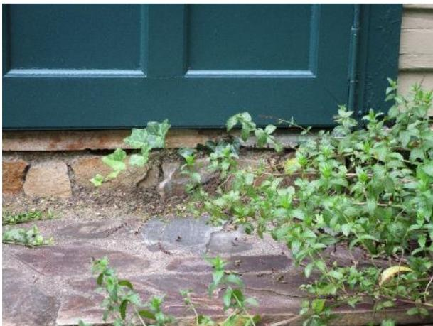
Figure 405. Missing mortar below the south enclosed porch door.
