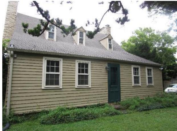
Figure 383. View of the south facade with vegetation around and in contact with the facade materials.
