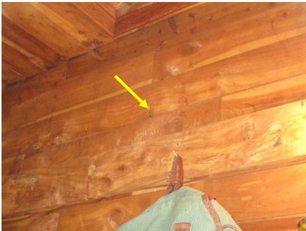
Figure 537. Crack in wood paneling within the hall closet.
