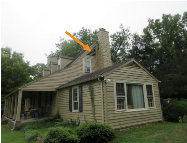
Figure 62. Gable end roof vent (arrow) on side of chimney, original section of house.
