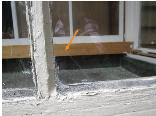
Figure 438. Cracked lite in the garden window.
