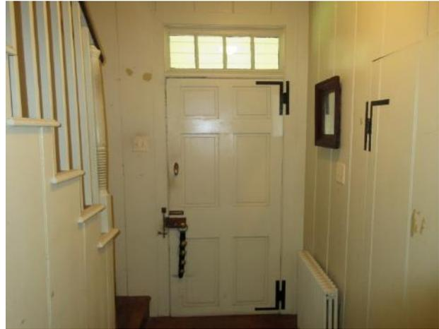
Figure 85. Interior view of exterior door, north facade. Note brass rim lock and knobs and HL-hinges.
