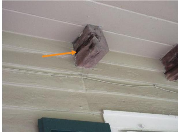
Figure 400. Wood section loss at an exposed wood joist, north facade.
