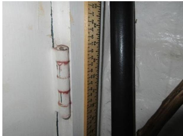
Figure 521. Surface corrosion observed at a kitchen door hinge.
