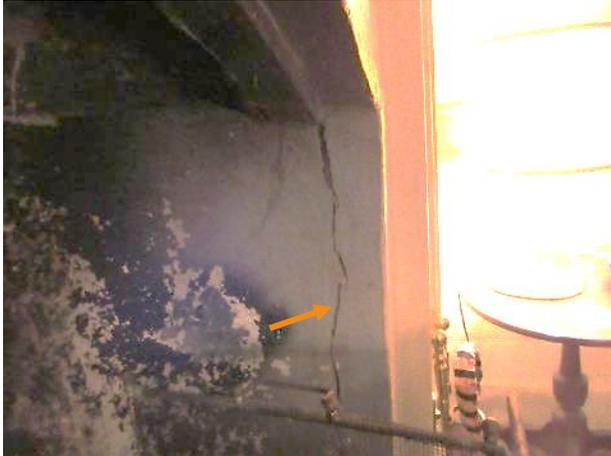
Figure 510. Crack within the cementitious parge coat of the living room firebox.
