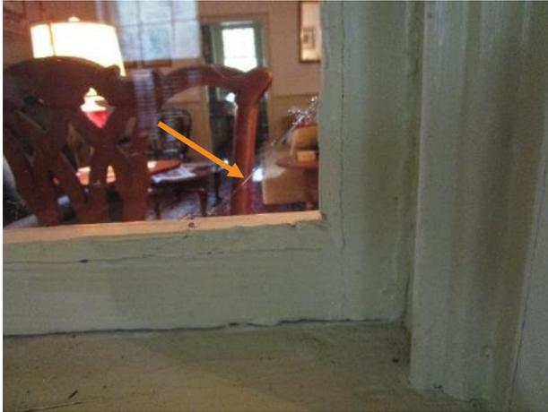
Figure 514. Cracked glazing lite at window between living room and south enclosed porch.
