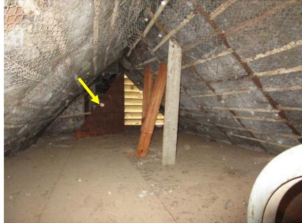
Figure 379. Gable vent fan at the west is open. Note hinged plywood door.
