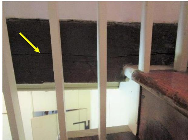
Figure 542. Season check along the exposed timber in the stairwell.
