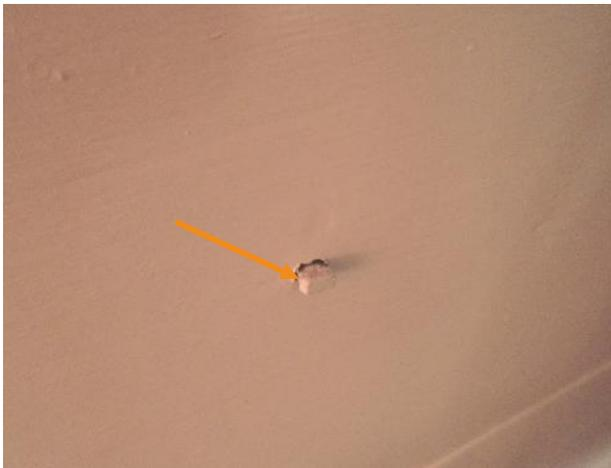
Figure 247. Headless cut nails were observed fastening to the wood wall paneling to studs.
