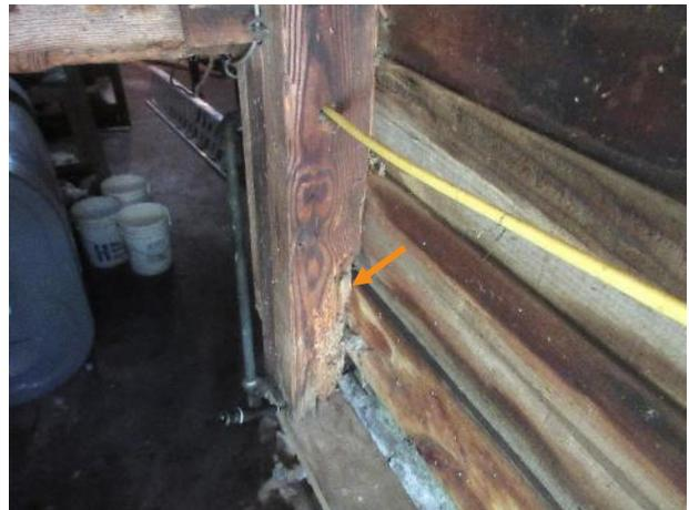
Figure 534. Wood section loss at the wood studs of the cellar access.
