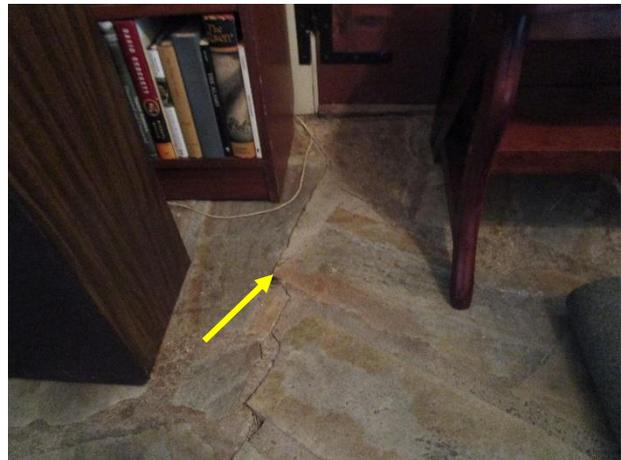
Figure 552. Crack full depth of the south enclosed porch.
