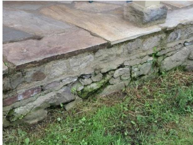
Figure 52. Stone varies in size and shape, including thin stone units, north porch.
