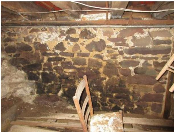
Figure 504. Staining at the foundation wall, viewed from the cellar.
