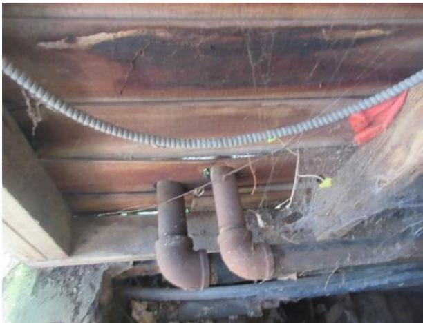
Figure 122. Plumbing penetrations, cellar access.
