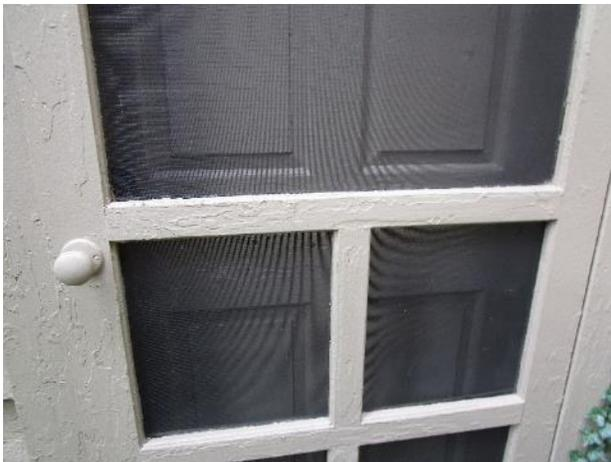
Figure 460. Screen door at the west addition could not be opened, possibly due to overpainting.
