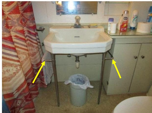
Figure 334. Typical 1930s era sink. This sink features integrated towel racks, which is unique to this space.
