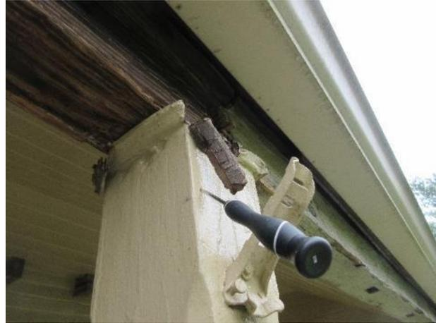
Figure 471. Soft and rotted wood found using a probe at the top of a north porch post.
