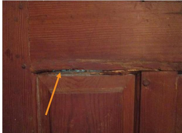
Figure 455. Separation between a lower panel and middle rail of the south enclosed porch door, view from interior to show daylight.
