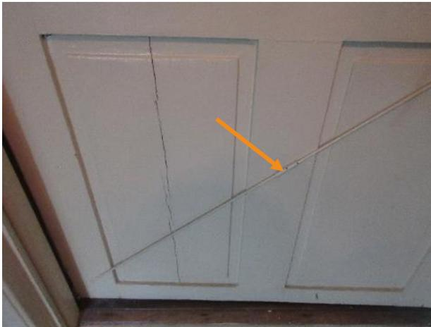
Figure 262. Torsion rod in place at the bottom half of the door leading to the dining room.
