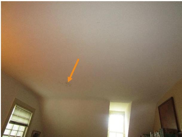
Figure 477. Typical peeling paint at second floor ceiling, guest bedroom shown.
