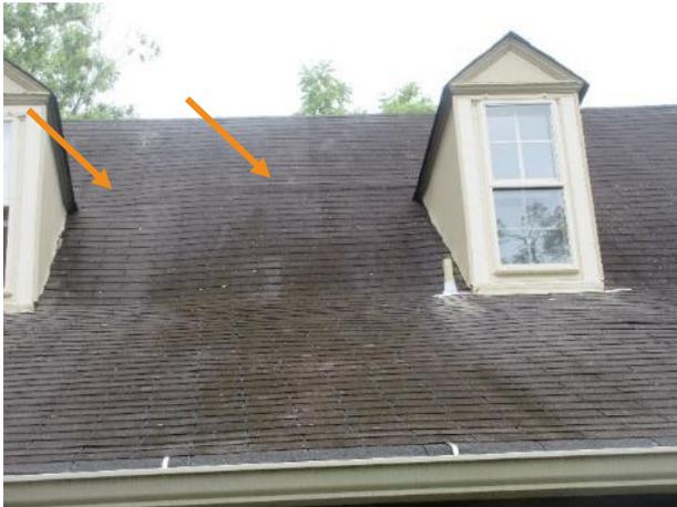
Figure 423. High point and sags between dormers, view from south.
