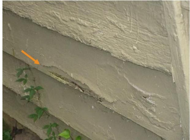
Figure 396. Isolated wood section loss at the west facade.
