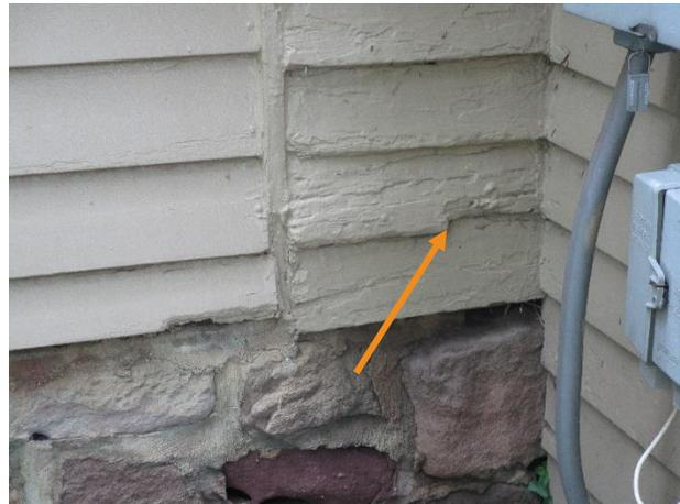
Figure 394. Isolated wood section loss at the east facade, to the south of the cellar access.
