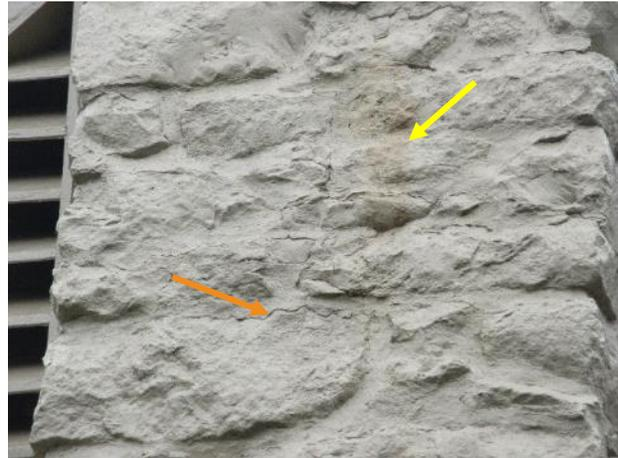
Figure 463. Typical bondline failure of mortar joints at chimneys (orange arrow), east chimney shown. Note adjacent staining (yellow arrow).
