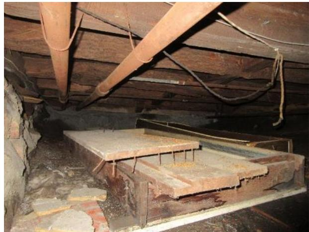
Figure 155. Wood materials and possibly door stored on the dirt in the crawl space.
