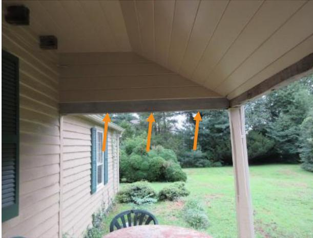
Figure 112. West end joist has notches on bottom side. See Figure 113.
