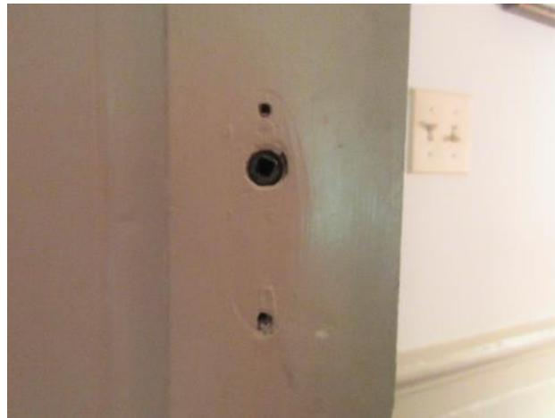
Figure 248. Evidence of removed hardware at the south dining room door leading to the south enclosed porch. The previous hardware is located above the existing hardware.
