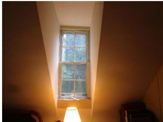
Figure 357. Dormer at the south wall is covered with plastic.
