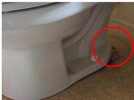
Photo 2: Footprint of the old water closet where the seal was already replaced.
