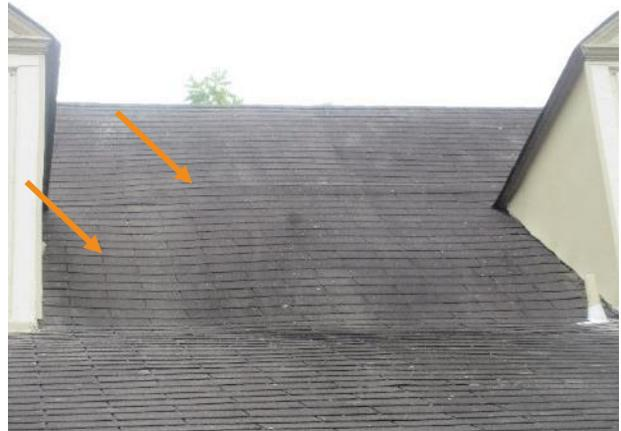
Figure 422. High point and sags between dormers, view from south.
