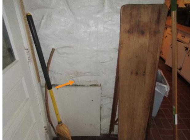
Figure 511. Crack in the mortar originating from an opening on the side of the masonry wall in the kitchen.
