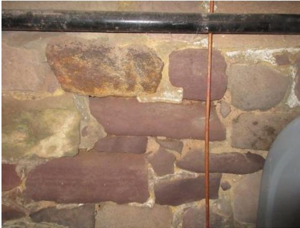
Figure 124. Cellar walls are made up of red sandstone with a sand and lime-based mortar.
