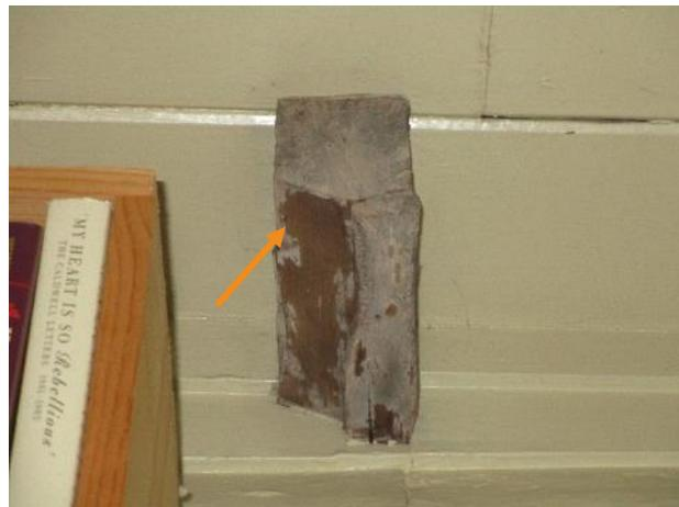
Figure 526. Wood section loss at exposed joists in the south enclosed porch.
