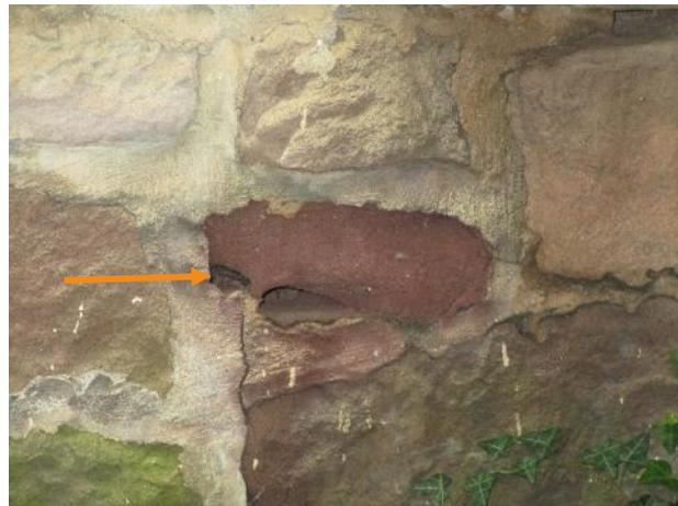
Figure 418. Erosion of a sandstone foundation unit, east facade.
