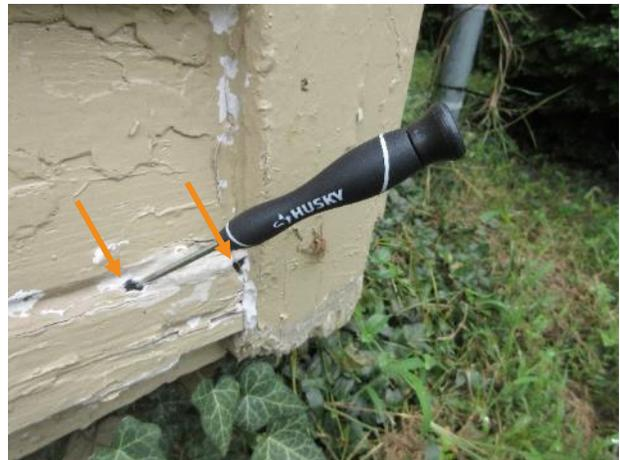
Figure 390. The repair was done with sealant, which contains voids.
