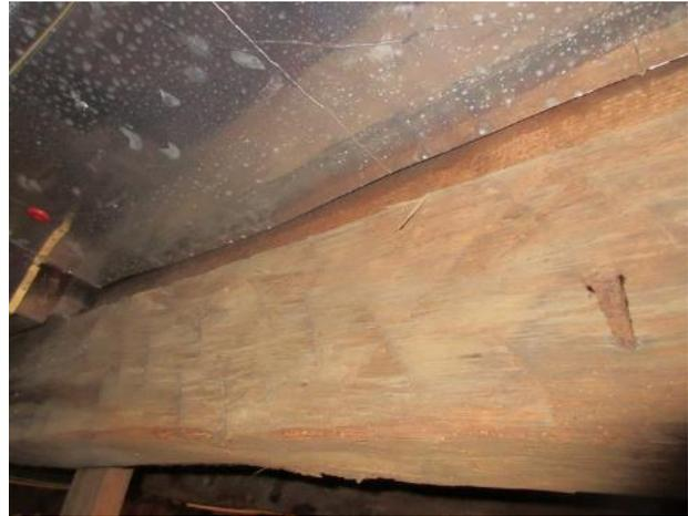
Figure 137. Close-up view of hand-adzed floor joist.
