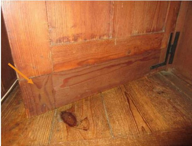
Figure 297. Lower rail of the door between the library and sitting room has been replaced.
