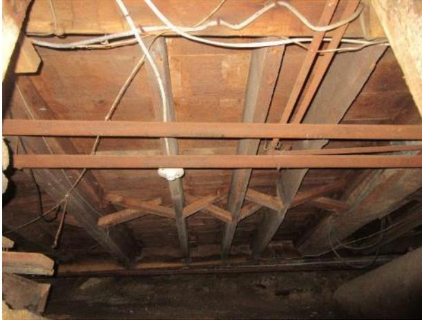
Figure 156. Joists in the crawl space are comprised of hand hewn and machine sawn.
