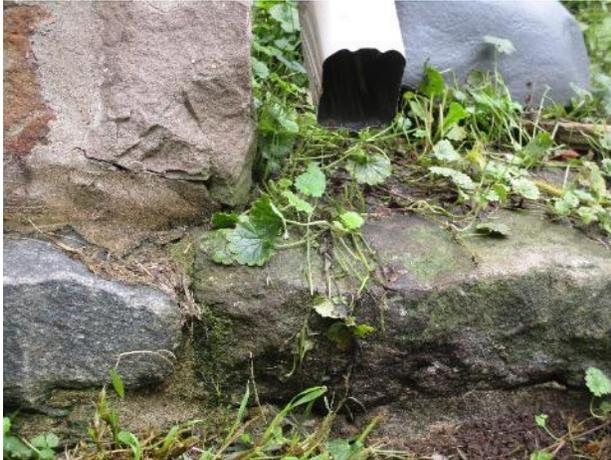
Figure 415. Biological staining on foundation stones adjacent to a downspout.
