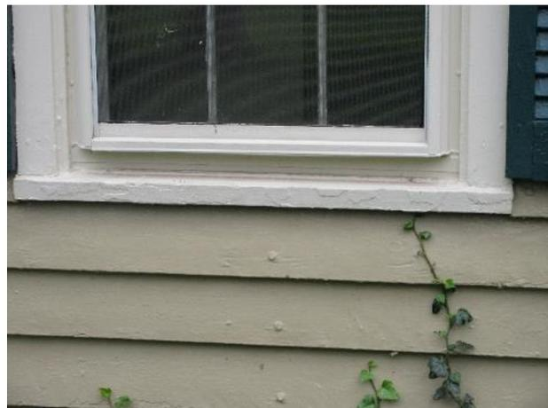
Figure 436. Paint has been applied over previous coating(s).
