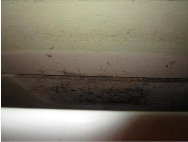
Figure 495. Black staining observed in bathrooms, indicating an issue with ventilation.
