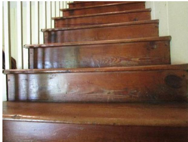
Figure 177. Typical finished wood risers and treads.
