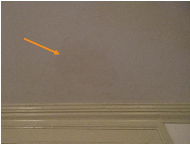
Figure 497. Area of plaster staining, dining room shown.
