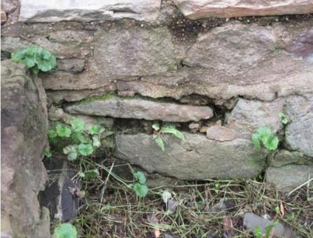
Figure 53. Stone varies in size and shape, including thin stone units, north porch.
