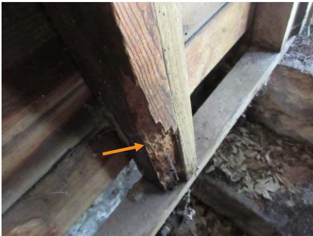
Figure 533. Wood section loss at the wood studs of the cellar access.
