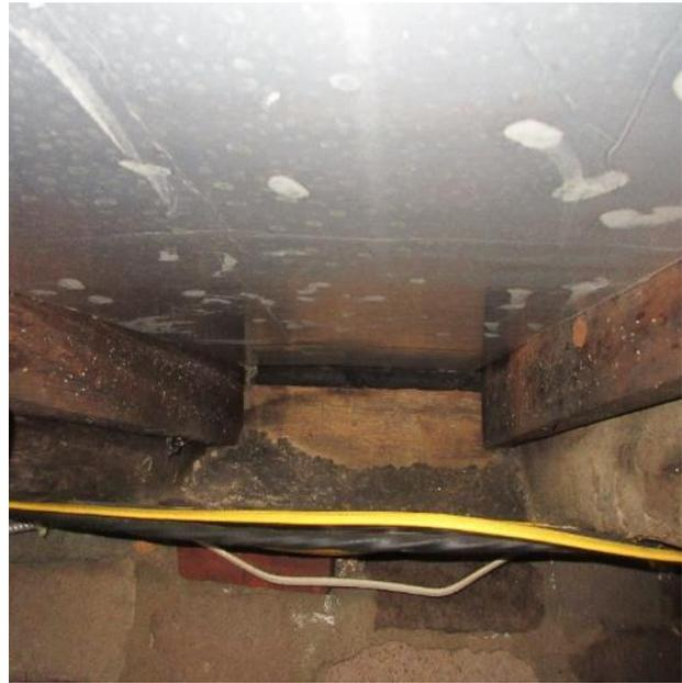
Figure 141. Joists are notched to ledger boards (or sill plate) that rests atop the masonry foundation wall.
