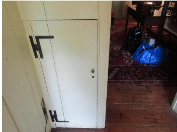
Figure 169. Small storage cabinet at the south wall of the hallway of similar construction of doors that blend with wall paneling.
