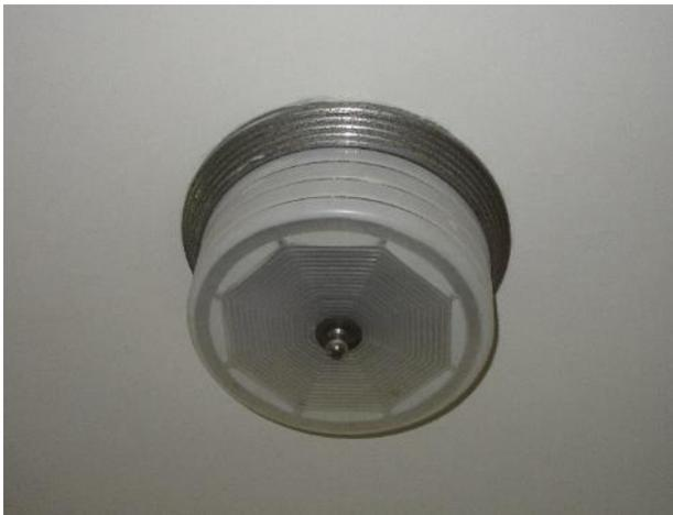
Figure 198. Ribbed milk glass ceiling mounted light fixture.
