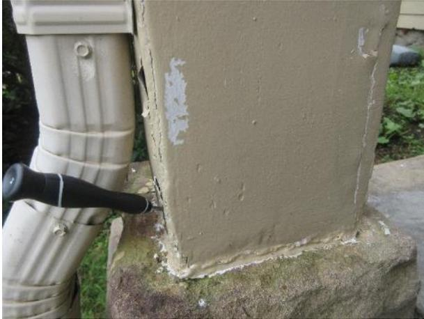
Figure 470. Soft and rotted wood found using a probe at the base of the north porch posts. Note downspout attached to this post.
