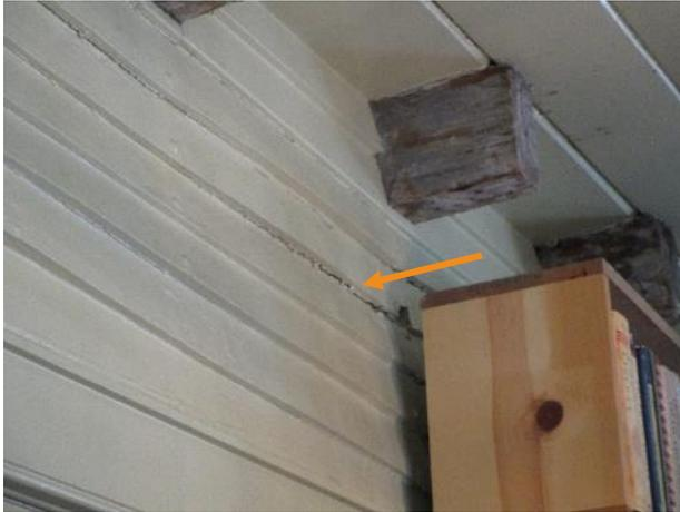
Figure 527. Uneven clapboards below the exposed joists.
