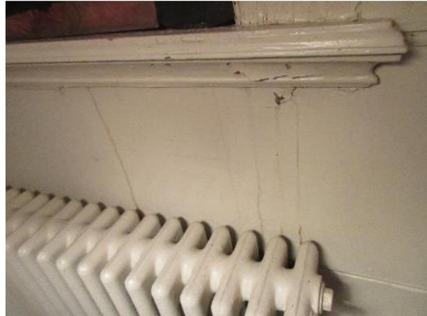
Figure 452. Water staining below the living room south window on the west facade.
