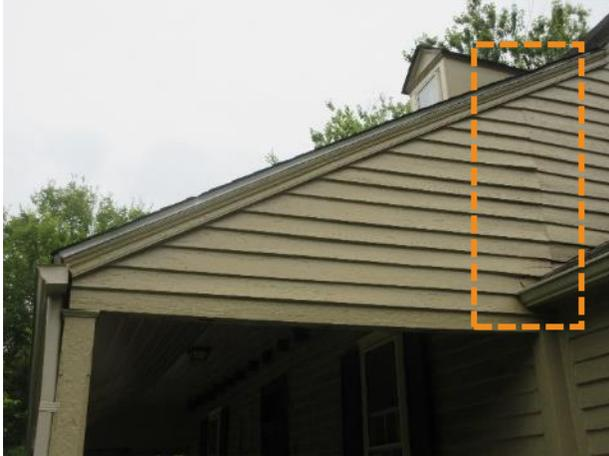
Figure 391. Section of clapboards at the west facade above the porch that is displaced.
