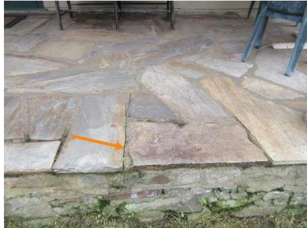
Figure 408. Full depth crack in mortar at the north porch.
