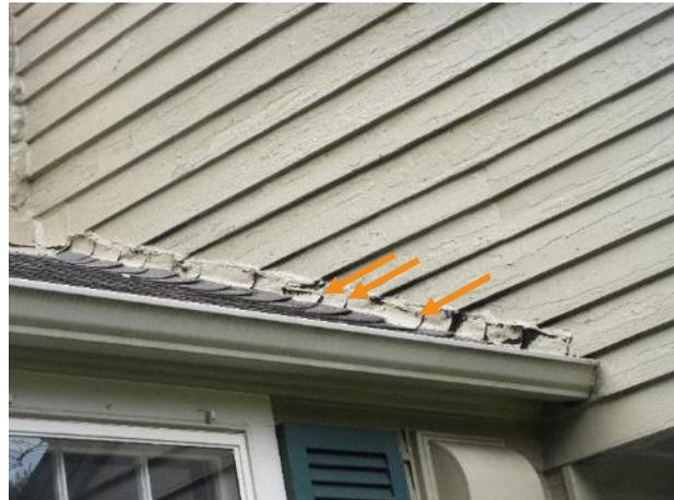
Figure 432. Unsealed laps of metal flashing between house and east addition.
