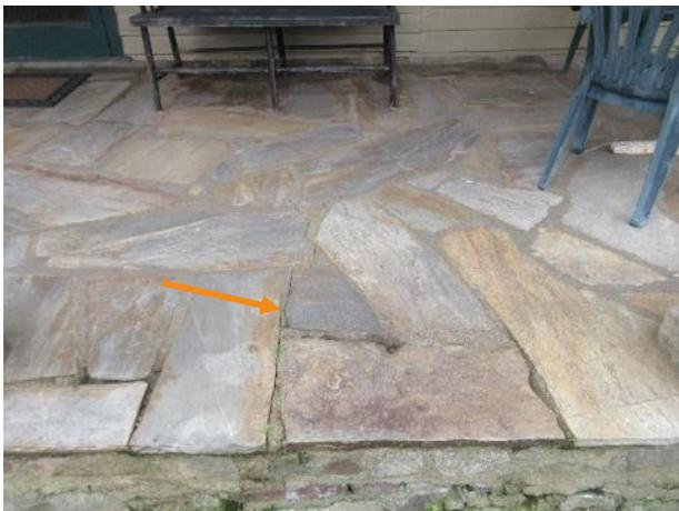
Figure 409. Full depth crack in mortar at the north porch.
