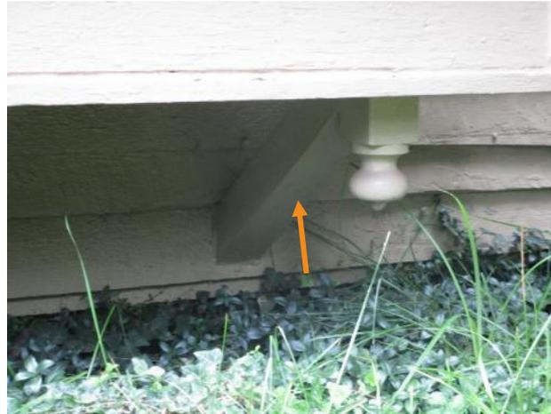
Figure 79. Close-up view of angled supports shown in Figure 78.
