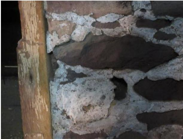
Figure 126. White coating remnants on cellar walls, at mortar joints.
