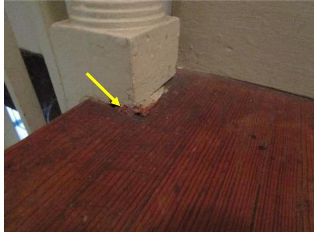
Figure 540. Crack in wood or shim at the base of the newel post.
