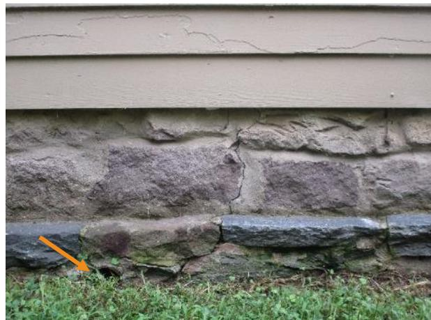
Figure 406. Crack in foundation mortar at the east addition. Note exposed pipe from where the crack originates.
