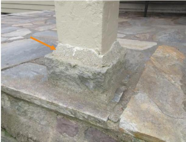
Figure 108. Close-up view of mortar wash at the base of the left post seen in Figure 107.
