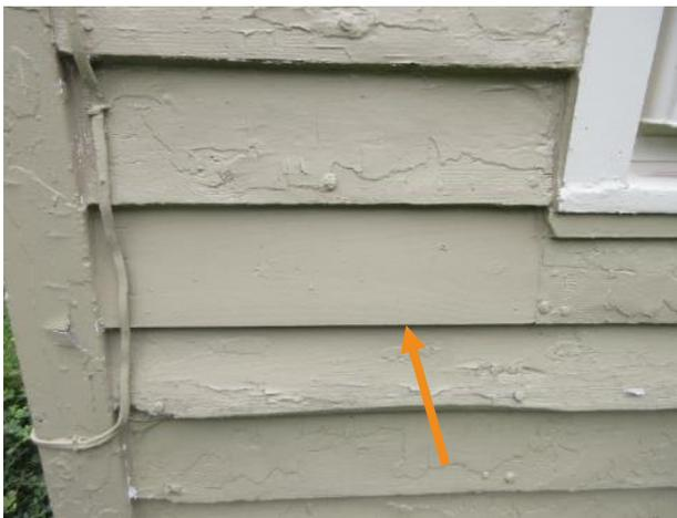
Figure 47. Wood dutchman section of clapboard, north facade study addition.
