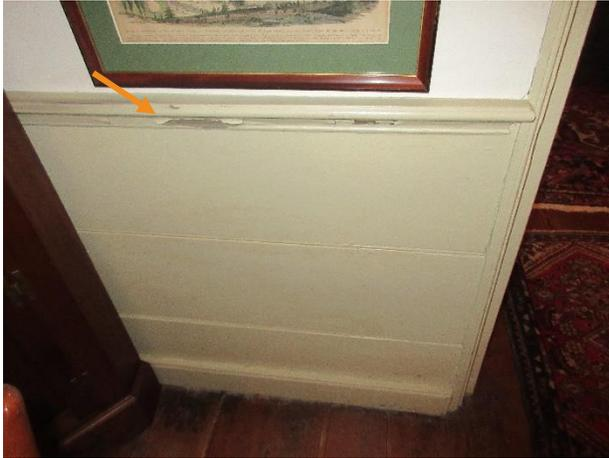
Figure 491. Typical peeling or missing tan paint at wood elements, dining room west wall shown.
