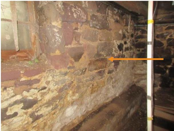
Figure 508. The west wall appeared to be out of plumb.
