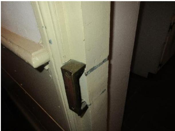
Figure 520. Missing paint at the casing from door abrasion, dining room shown.
