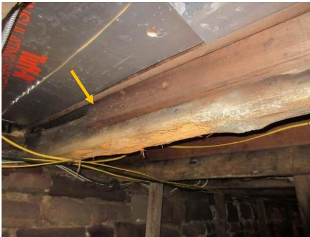
Figure 138. Contemporary sistered joist, partial length of the hand hewn joist.
