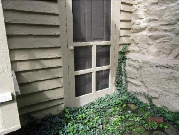
Figure 386. Vegetative growth onto the west addition door and house facade materials.
