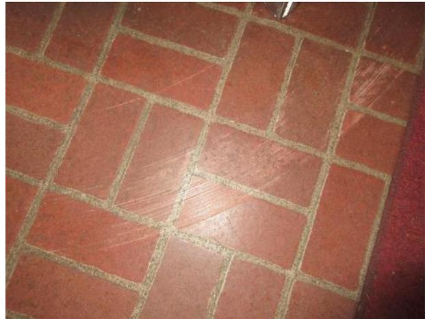
Figure 207. Basket weave brick paver flooring in the kitchen.
