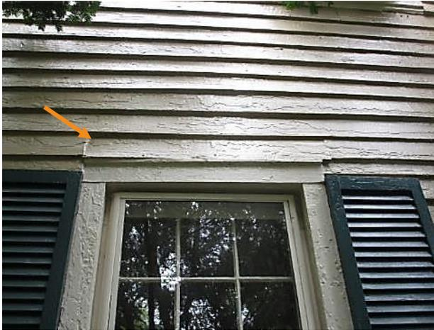
Figure 49. Wood dutchman section of clapboard, first floor southern window at east facade.
