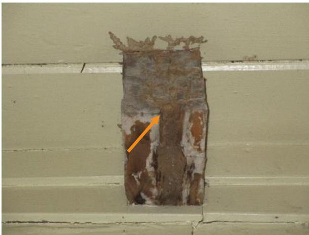
Figure 525. Wood section loss at exposed joists in the south enclosed porch.
