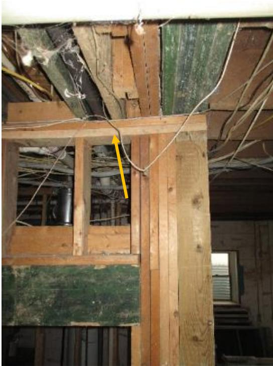
Figure 16. Deflection of header at interior partition wall.
