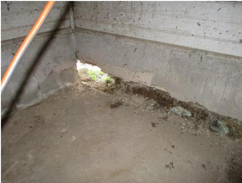
*Figure 89. Deteriorated finish at base of interior walls.*
