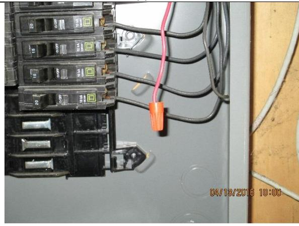
Photo 6: Unsecured conductor in basement panel
