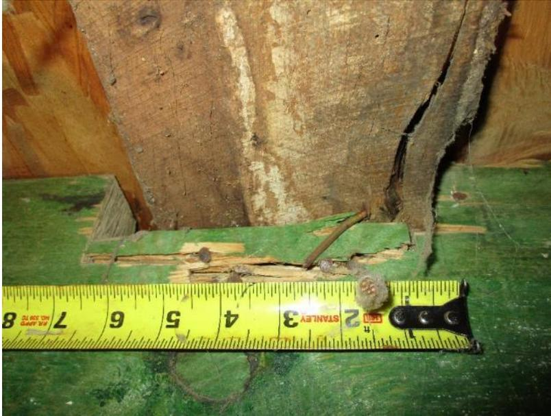
*Figure 19. SCL joists are notched at their tops at what appears to be an old perimeter beam, which runs perpendicular to the joists.*
