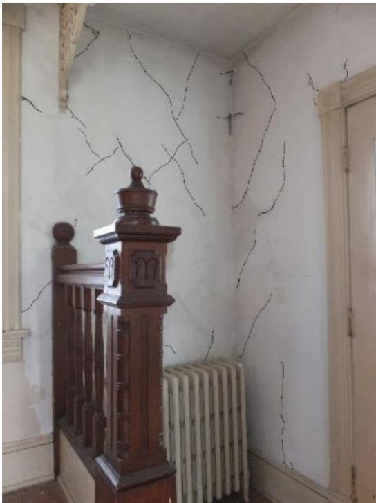
*Figure 9. Example of cracking at the entryway at the northwest corner. Cracks have been traced for clarity.*
