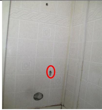
Photo 30: Mid-level hall bath shower enclosure with damage evident
