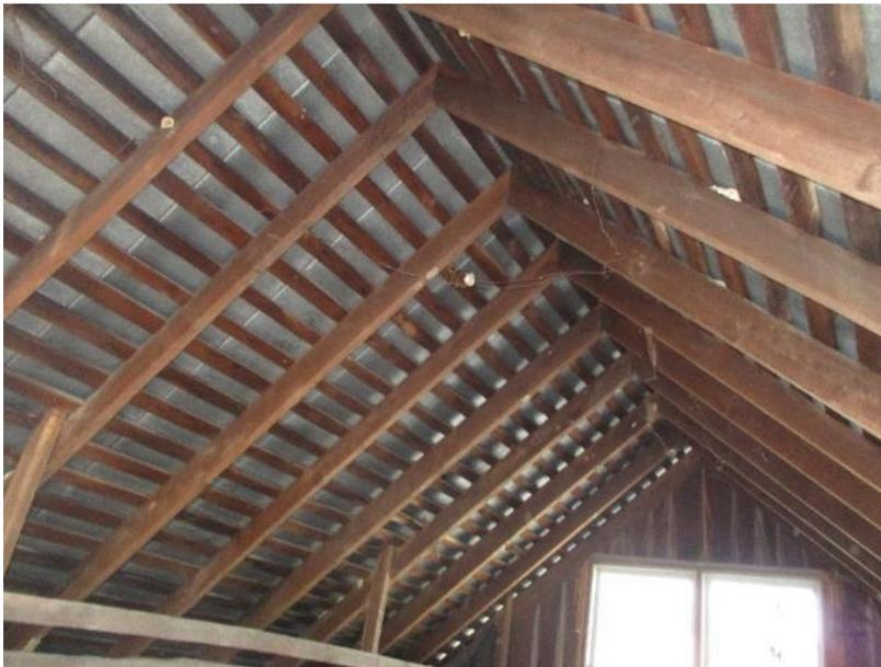
*Figure 74. Roof framing as viewed from the loft.*
