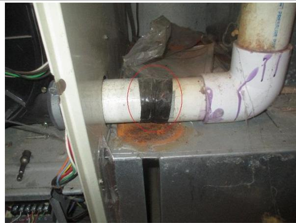
Photo 21: Taped pipe joint on exhaust
