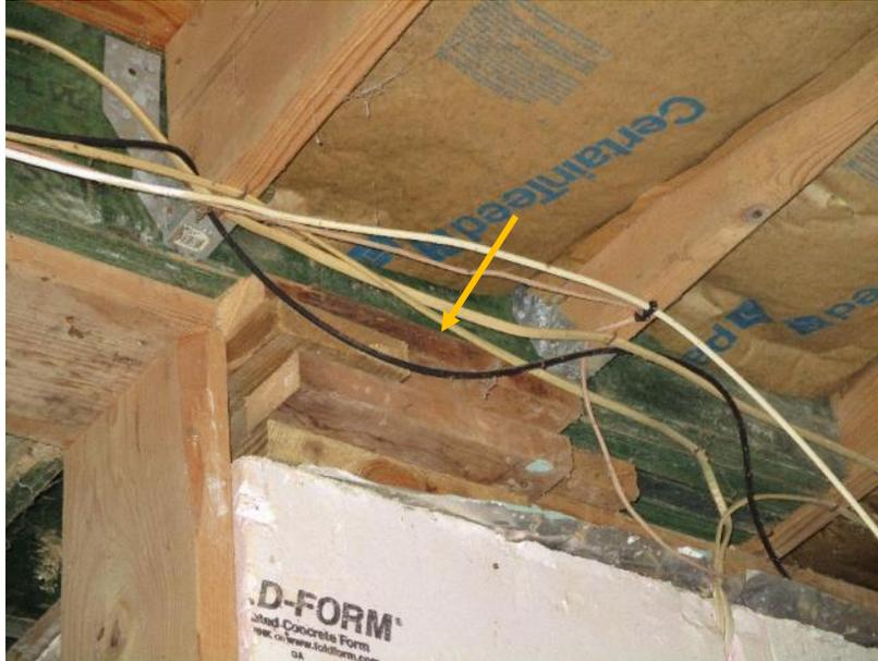
*Figure 17. Built up wood blocking.*
