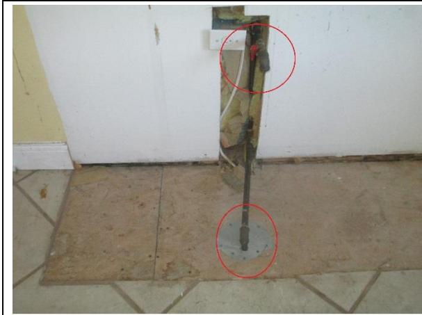
Photo 7: Kitchen gas piping through floor
