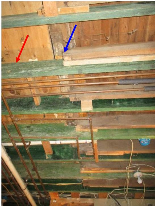
*Figure 18. New framing members span the entire width of the south addition (red arrow). Original framing is no longer supported at west ends (blue arrow).*
