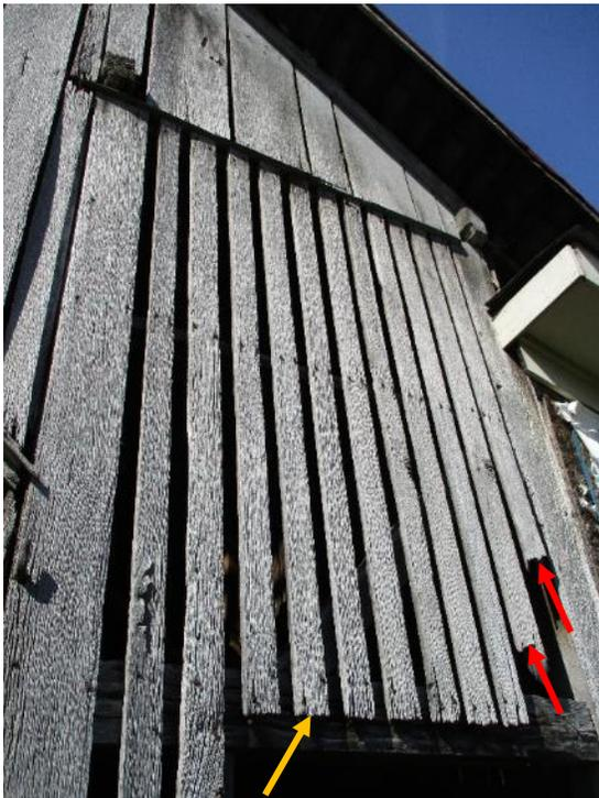
*Figure 76. Splintering at the ends of the wood slats (orange arrow) on the south elevation along with two fractured slats (red arrows).*
