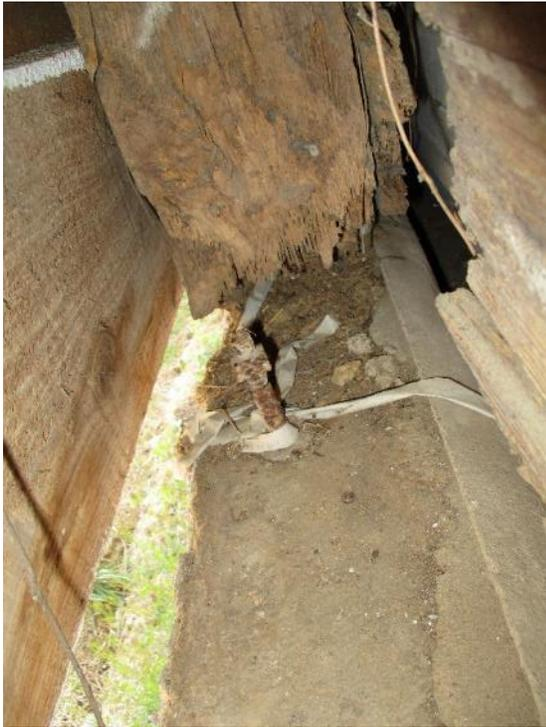
*Figure 90. Loss of bearing at wood column.*
