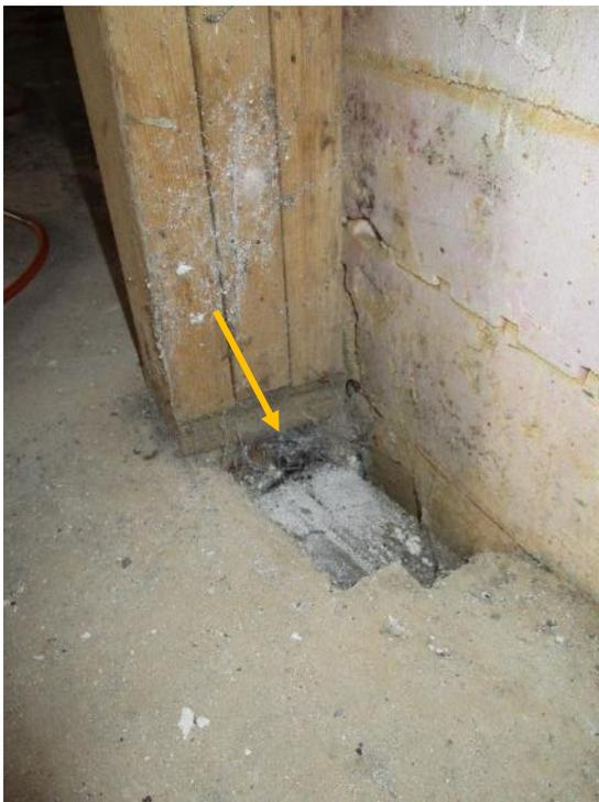
*Figure 20. Void in concrete slab below column.*
