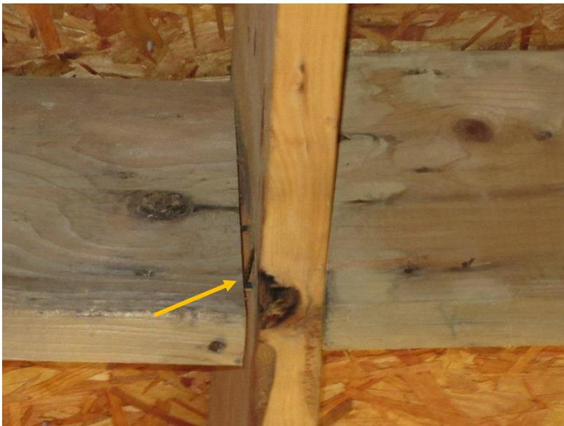
*Figure 53. Gap is present between end of wood bridging and joist.*
