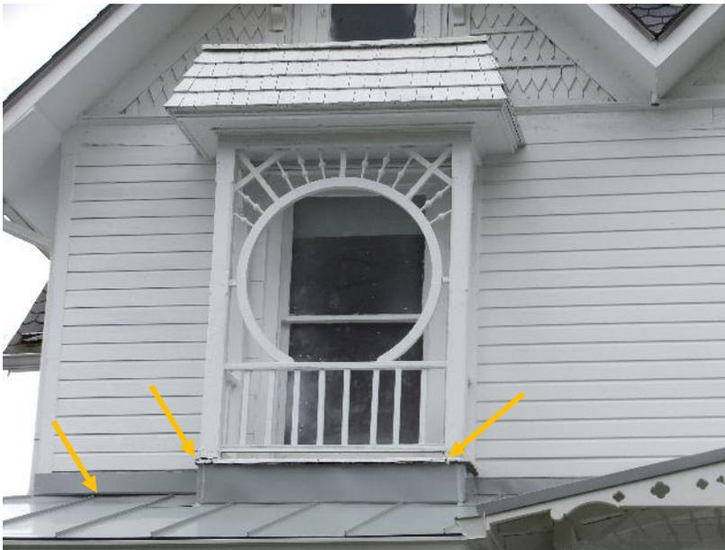
*Figure 37. Lifted and separated flashing at Juliet balcony. Note gap between second floor flashing and porch roof.*
