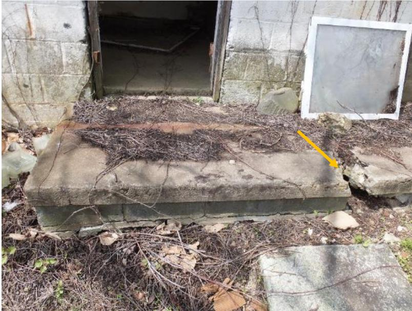
*Figure 82. Large crack through concrete landing and deterioration of the supporting CMU.*
