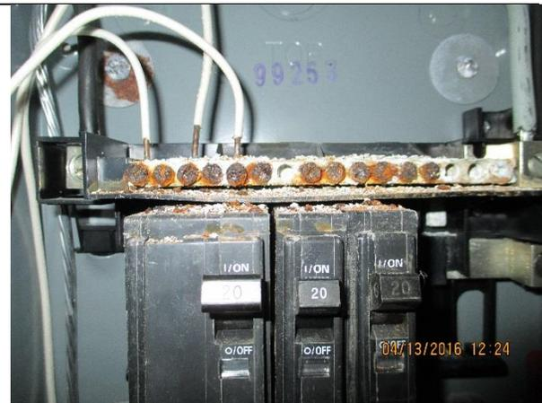
Photo 42: Oxidation/rust at terminations in panel inside the Dairy Barn
