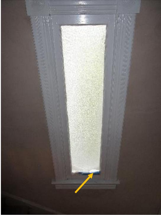
*Figure 34. Broken glazing in stairwell fixed window.*
