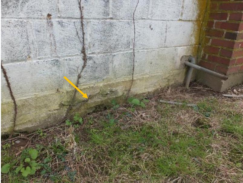
*Figure 80. A small spall is present in the concrete foundation wall.*
