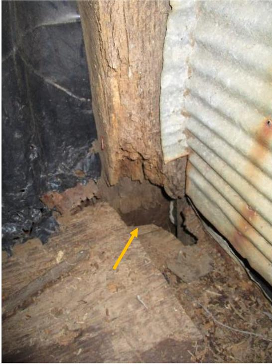
*Figure 70. Nearly complete loss of bearing at the northeast corner column in the east crib.*
