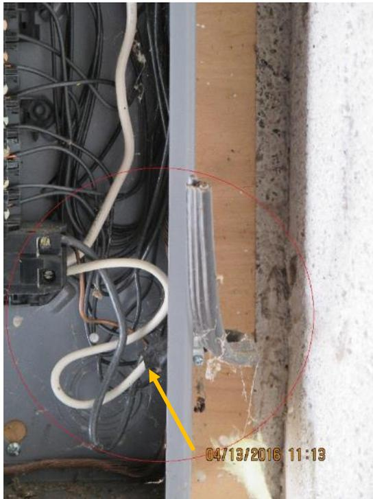
*Figure 54. Improperly terminated electrical lines. Photo courtesy of MBP.*
