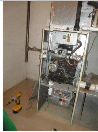
Photo 26: Condensate pump removed (lower left)
