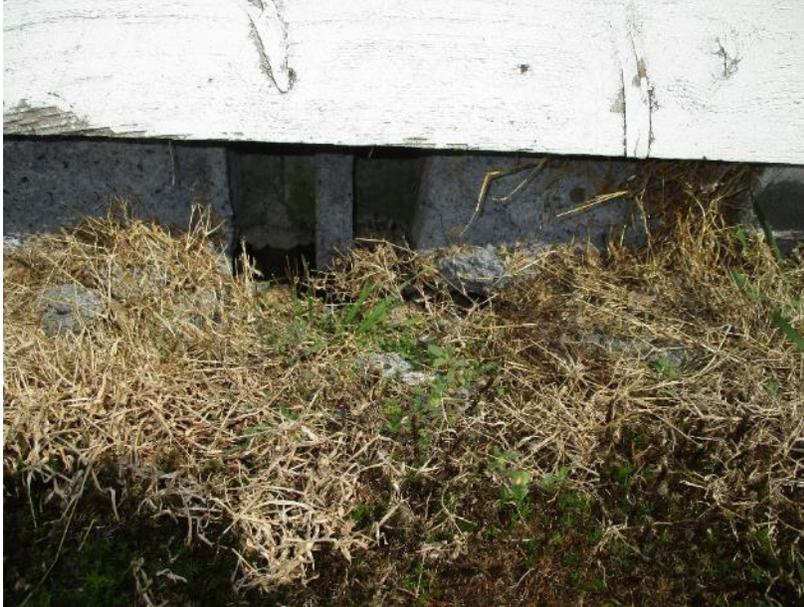
*Figure 88. CMU present at foundation wall along west elevation.*
