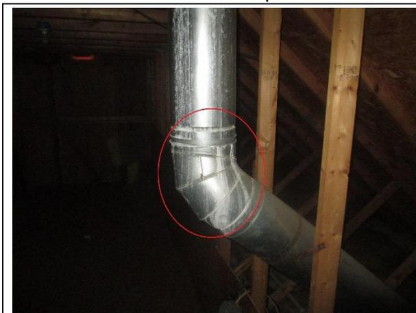
Photo 9: Flue vent with water stains
