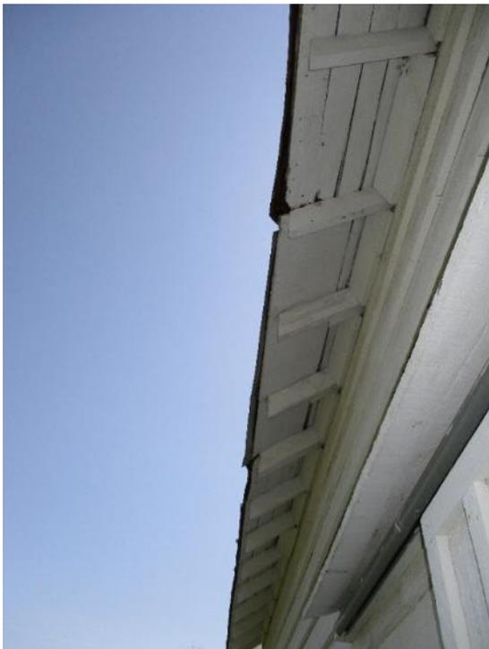
*Figure 100. Painted plywood installed at isolated area of soffit.*
