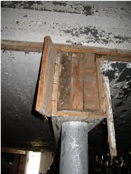
*Figure 93. Ends of built up interior beam appear to be in good condition.*
