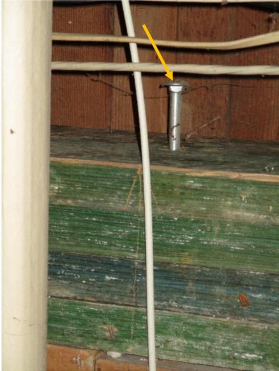
*Figure 21. Disengaged bolt in built-up member.*
