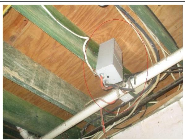
Photo 2: Abandoned box and wires in basement
