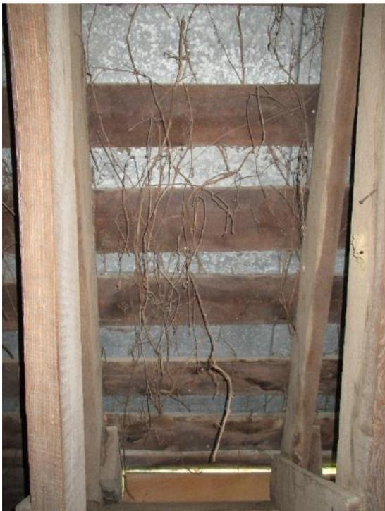
*Figure 98. Vegetation between the roof framing and the metal roof.*
