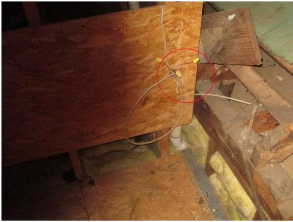
Photo 3: Unsecured wires in attic
