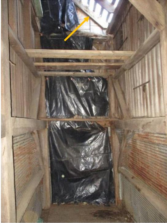
*Figure 69. A portion of the metal roof is missing at the northeast and corner of the original structure.*
