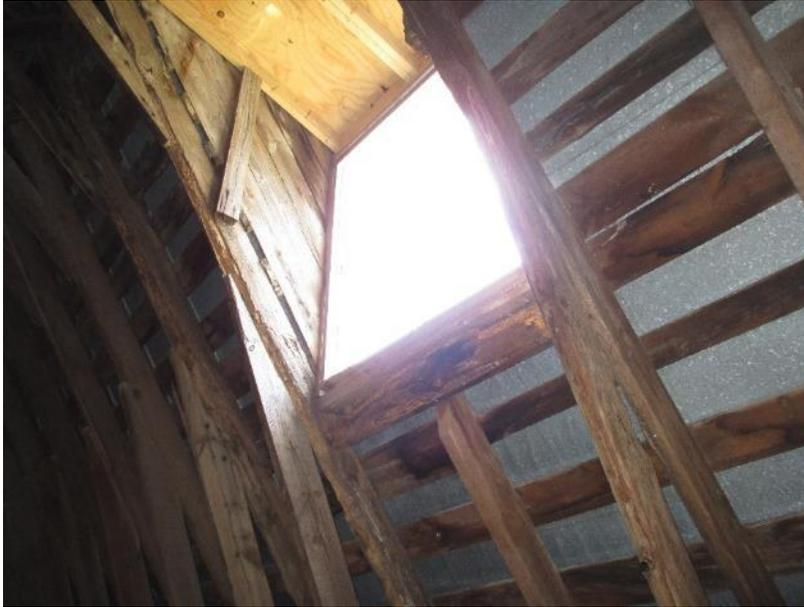
*Figure 94. Deterioration of the wood framing at the central dormer along the west elevation.*
