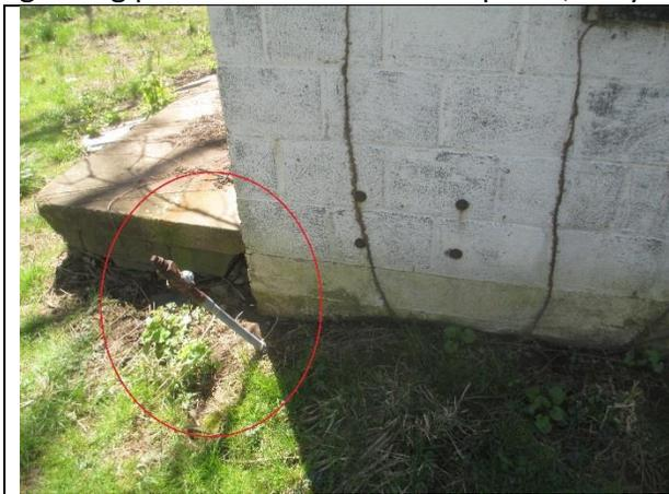
Photo 39: Damaged utility gas piping at NE corner
