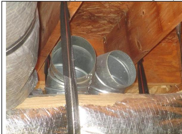
Photo 27: Duct fittings without dampers/diffusers
