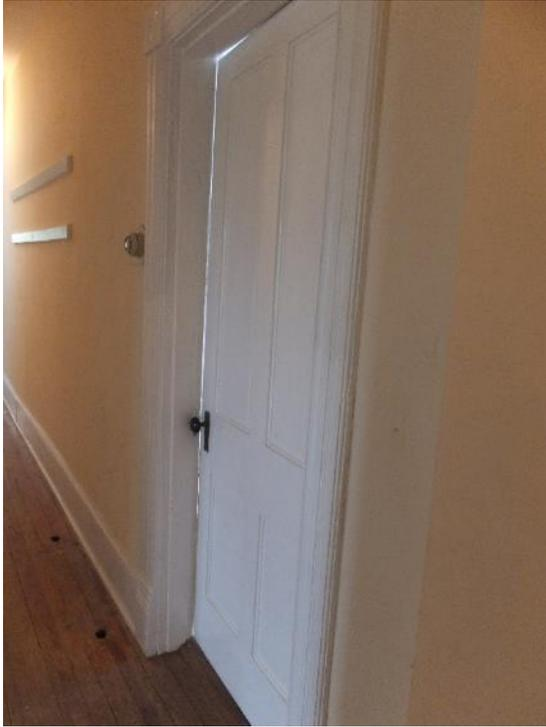
*Figure 10. Door leading into room 102 does not fully close.*
