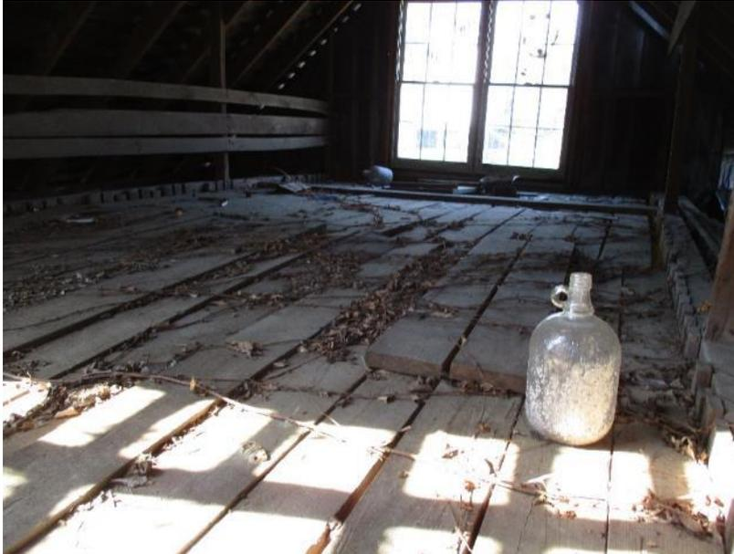
*Figure 73. Rough sawn planks in loft.*
