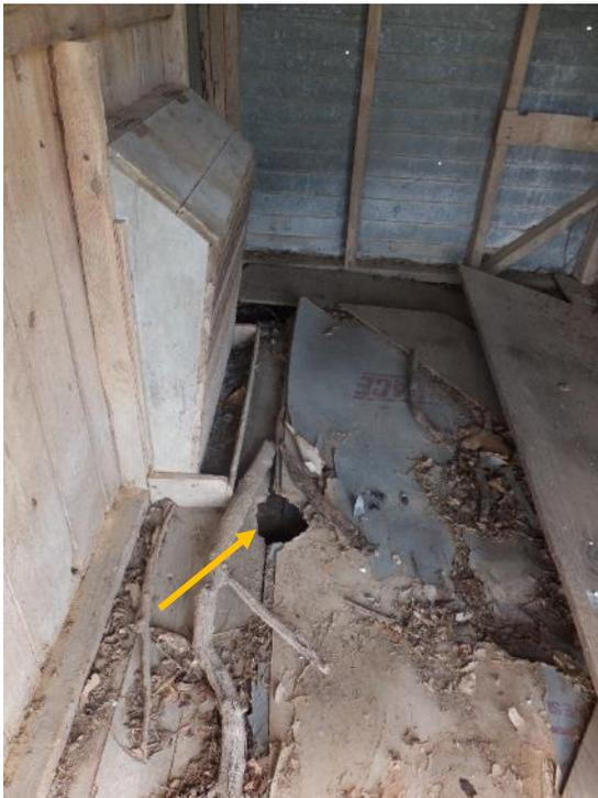
*Figure 60. Complete section loss of the plank members along with the presence of an animal habitat, as evidenced by chew marks in a wood plank (orange arrow).*
