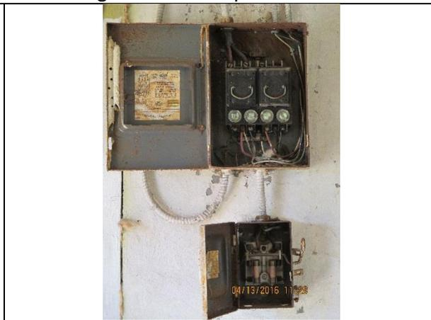
Photo 40: Derelict fuse box and wiring
