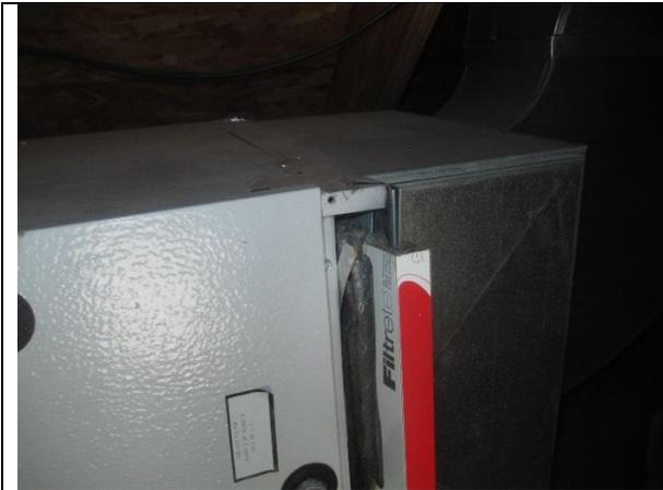
Photo 33: Ill-fitting filter at upper level heat pump unit
