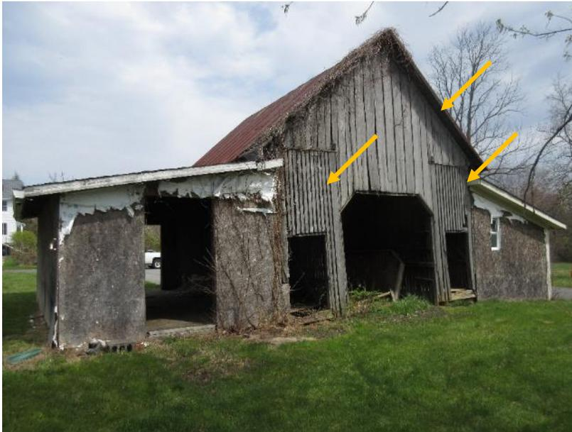
*Figure 64. South elevation of the crib barn as viewed from the southwest. Note the historic wood slats and siding.*
