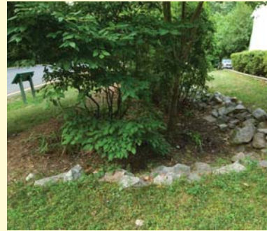
Rain gardens are designed to clean stormwater, slow runoff and increase ground water through infiltration. Vegetation and engineered soils act together to improve water quality throughout Fairfax County.
