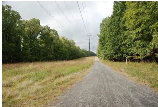
Figure 13: Photograph Illustrating Existing Maintenance Regime for Utility Corridor
