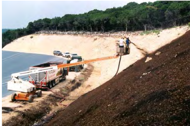
Application of a 2 inch-thick blanket to a 1:1 rock slope using a pneumatic blower (Austin, Texas, 2002). Source: McCoy, Texas Commission on Environmental Quality (TCEQ), 2005.
